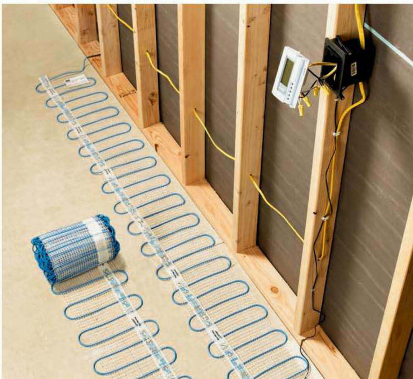
A radiant floor-warming system employs electric heating mats that are covered with floor tile to create a floor that's cozy underfoot.
