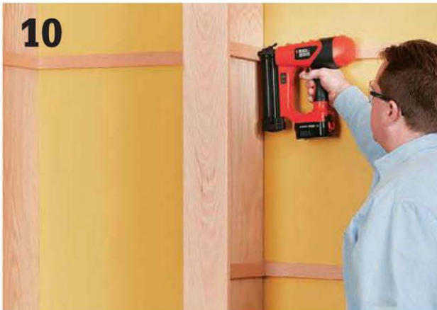
10 Attach the shelf cleats to the uprights, being careful to drive fasteners straight to prevent damage to the upright panels.
