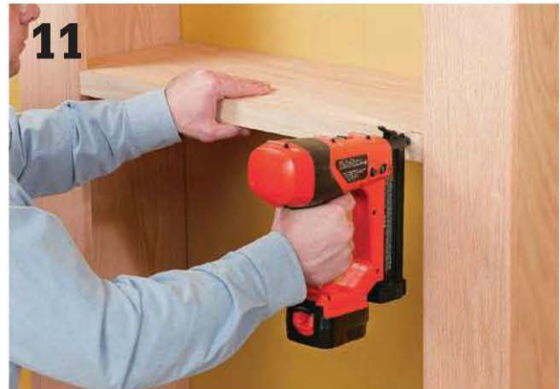
11 Edge the red oak shelves with 1 × 2 red oak nosing that's bonded to the shelves with glue and finish nails.
