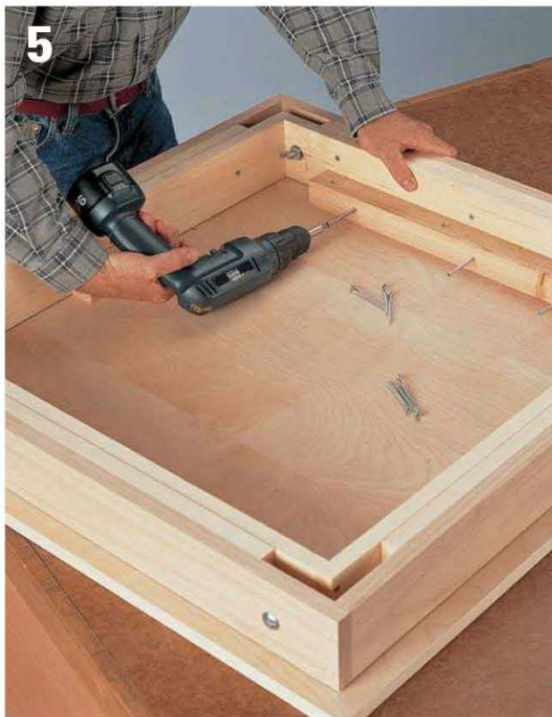
Fasten the main top to the liner by driving screws through the main cleats and short cleats and into the liner and filler blocks.
