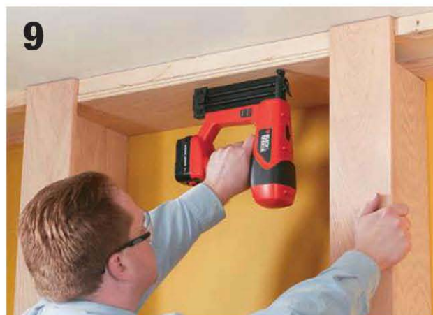
Attach a shelf at the top of each bay to conceal the framework attached to the ceiling.
