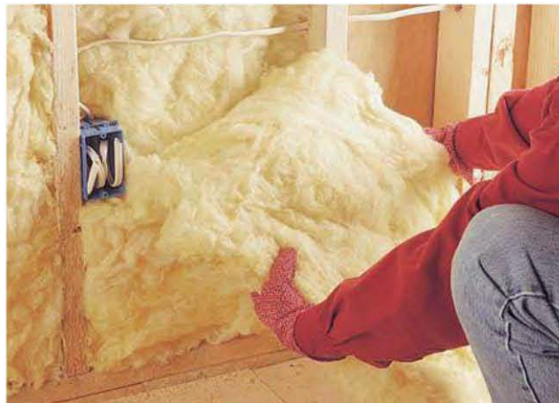
Insulate walls and ceilings of your new wine cellar to help you control the temperature and humidity and save energy.
