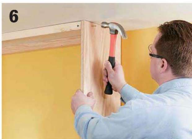
Nail the outer uprights to the ends of the nailing frame attached to the ceiling.
