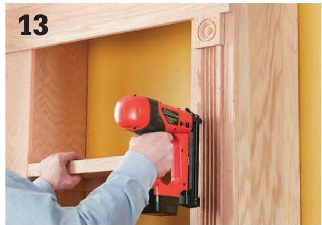
13 Attach the plinth blocks, rosettes, and fluted case moldings to complete the trimwork installation.
