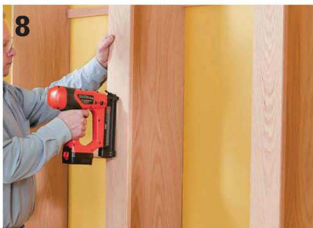
Attach the upright backers to the front edges of the inner uprights with pneumatic or hand-driven finish nails.
