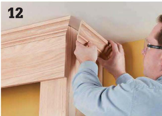
12 Conceal the gap between the top of the bookcase and ceiling with crown molding or sprung cove molding. Installing crown molding can get complicated. Consult a trim carpentry book if you are unsure how to work with crown molding.
