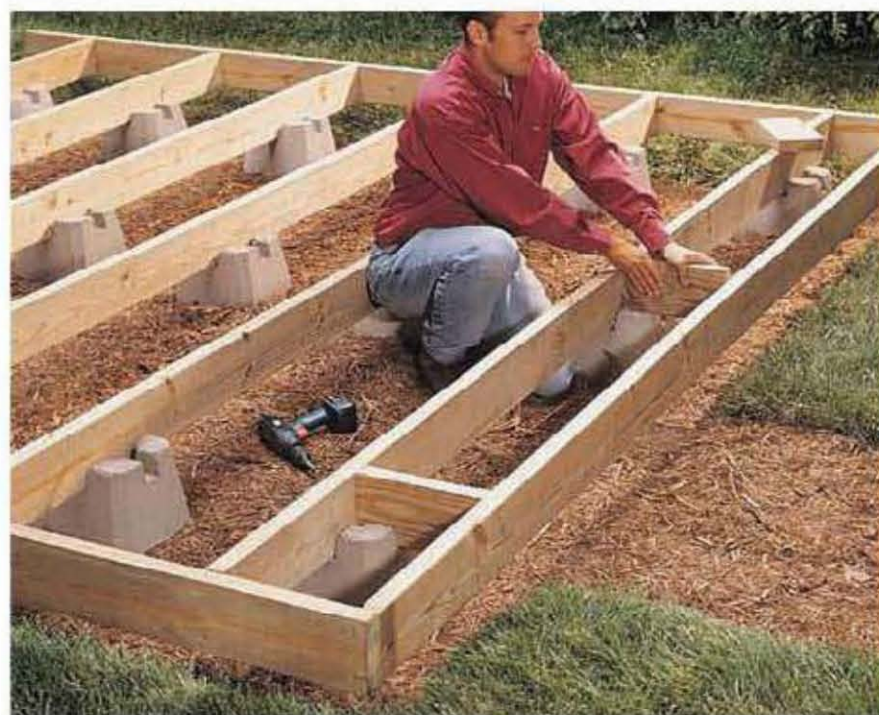
Position the sleepers in the slots of the footings , then attach them to both joists with pairs of deck screws.
