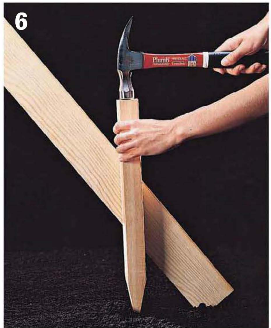
6 Drive a pointed 2 × 2 stake into the ground next to the end of the brace.
