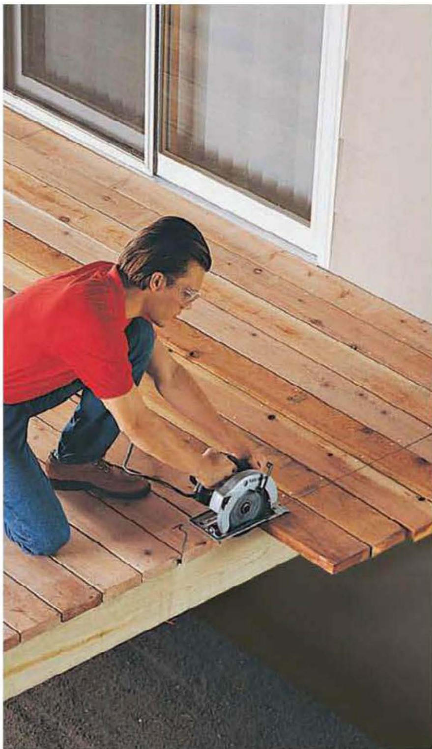
Snap a chalk line flush with the outside edge of the deck, and cut off overhanging deck boards with a circular saw.
