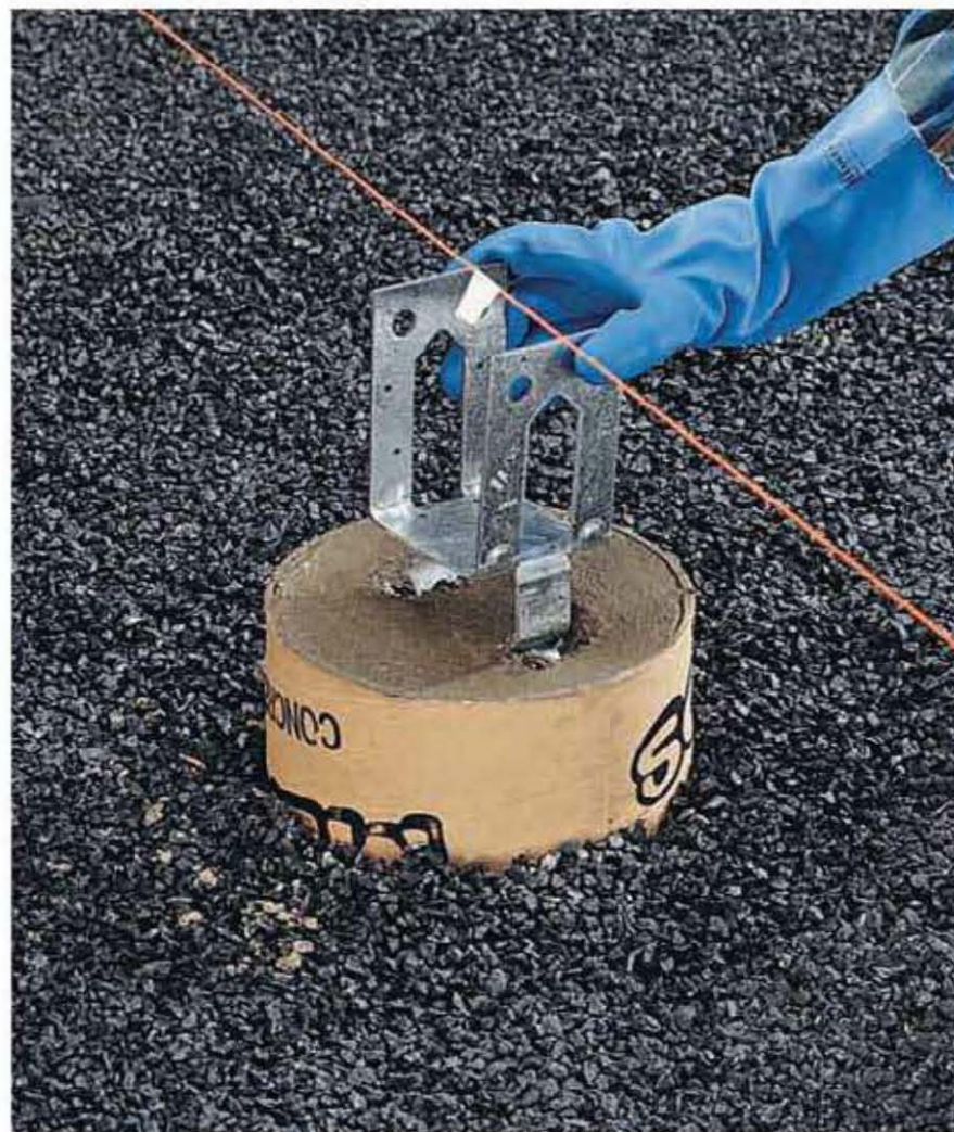
Direct bearing footing connectors attach beams directly to footings on low profile decks.
