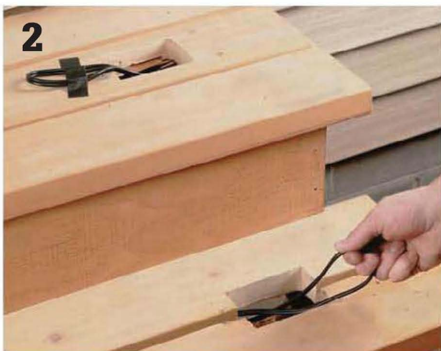
Run the cable from an existing low-voltage system or from a new transformer to the stair location.
