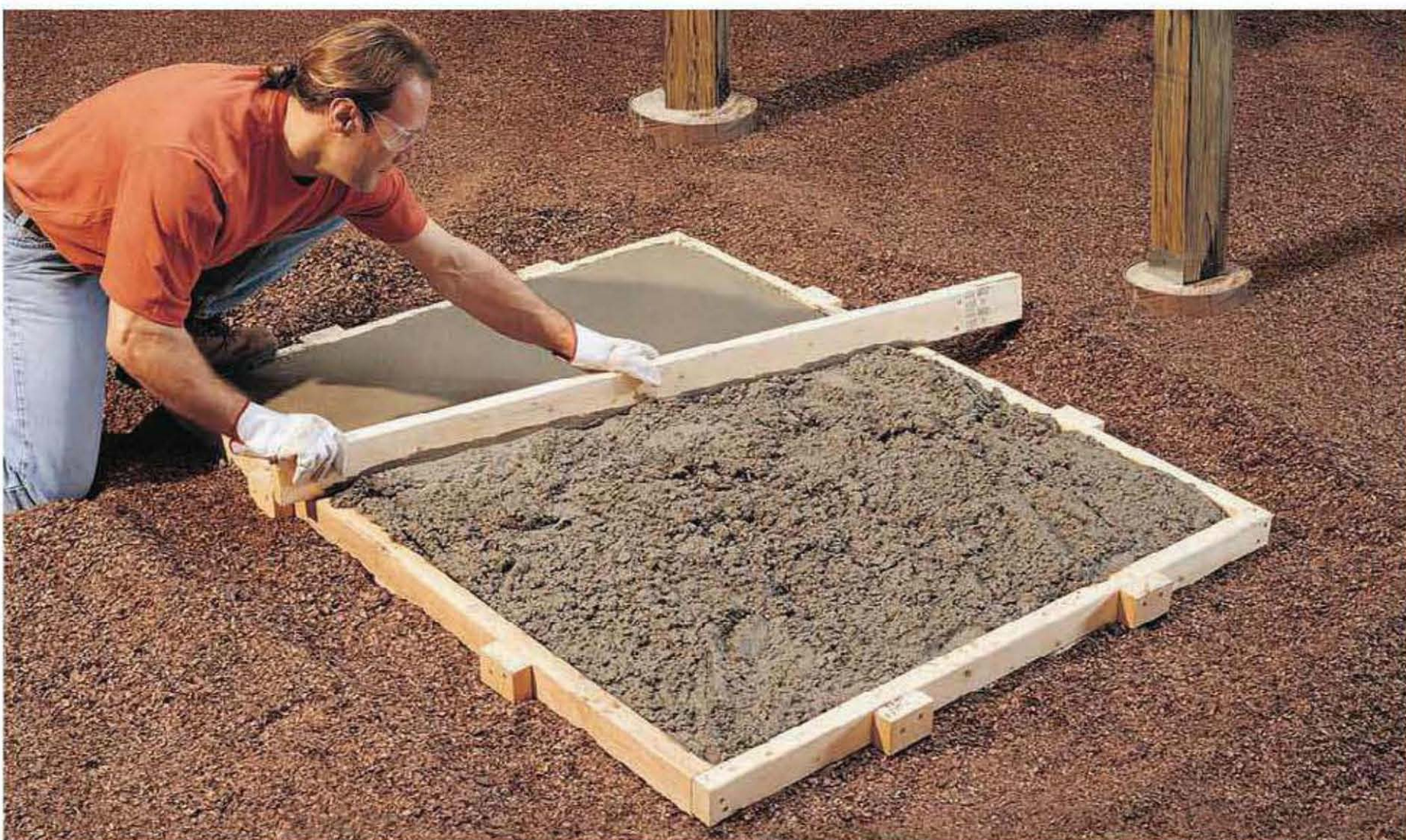
Pour the concrete into the staircase pad form , and screed flush, using a straight 2 × 4. If local codes require, pour concrete footings first.
