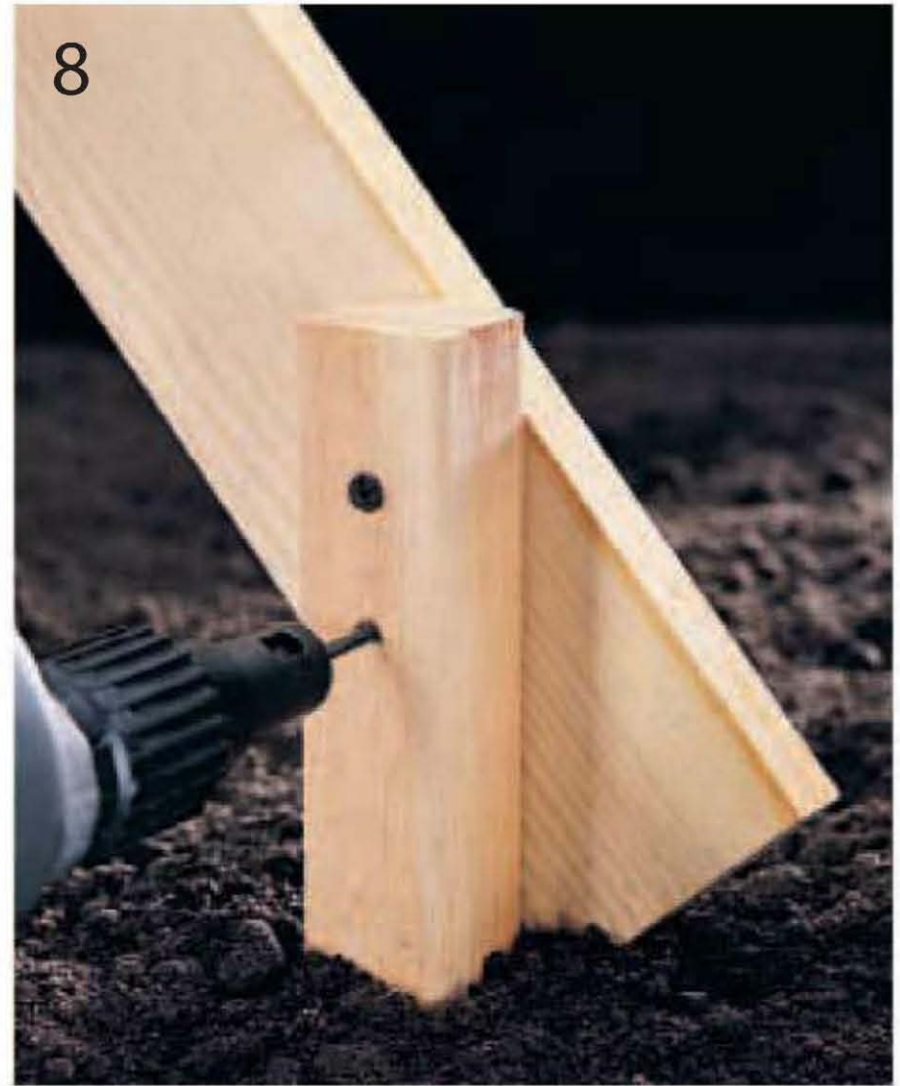
Attach the brace to the stake with two 2" wallboard screws.
