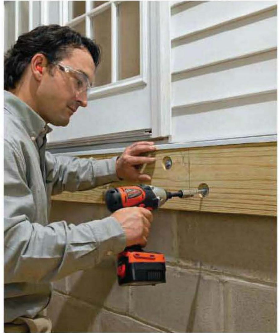
Galvanized or stainless steel lag bolts and washers are the correct fasteners for installing ledgers to the band joist of a house. You can also use them for making other wood-to-wood connections.
