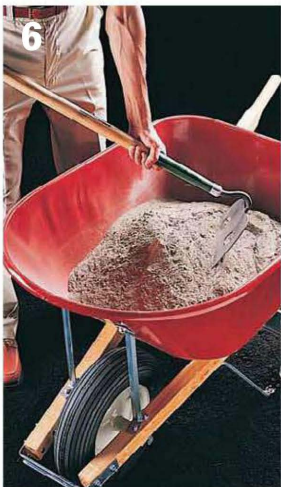
6 Mix dry ingredients for concrete in a wheelbarrow, using a hoe.
