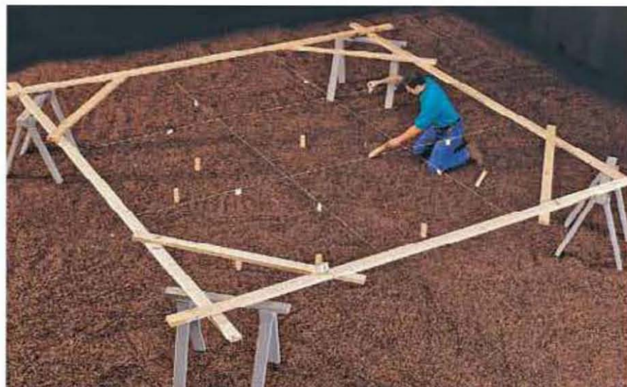
Locate the deck footings by stretching mason's strings across the site chooser, marking footing locations with tape, and dropping a plumb bob from each mark.
