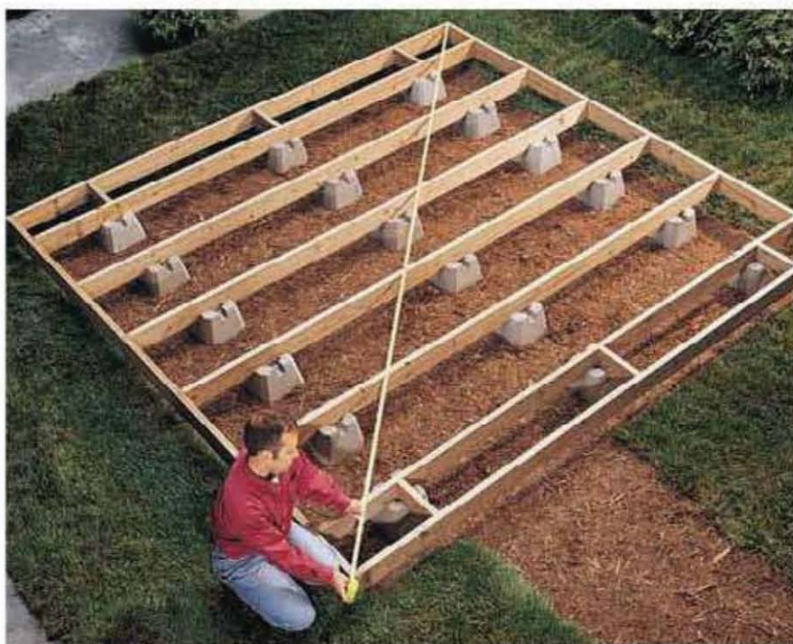
After the framing is completed , measure the diagonals and adjust the frame until it's square.
