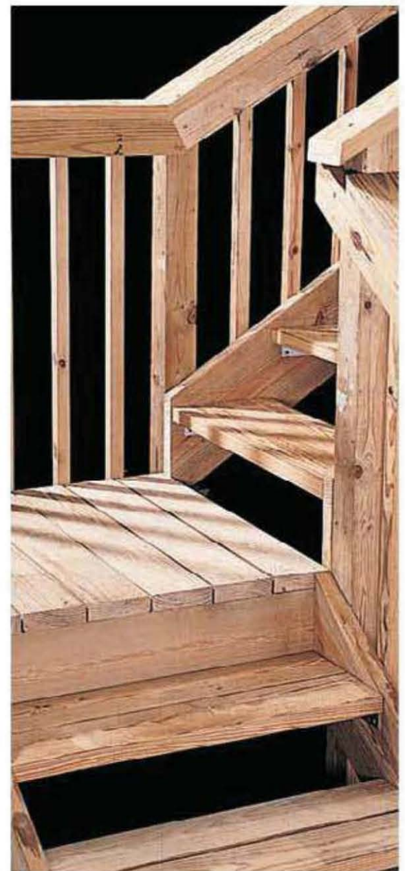
Long stairways sometimes require landings. A landing is a small platform to which both flights of stairs are attached (see pages 128 to 137).
