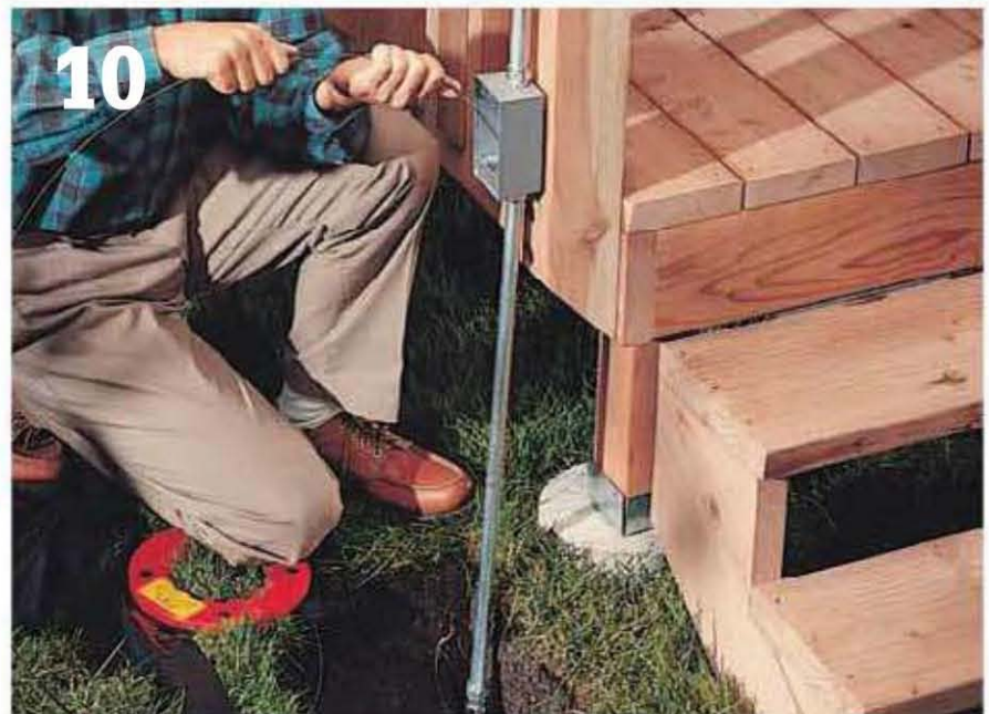
At the deck, use the fish tape to pull cable through the conduit and into the receptacle box and switch box.
