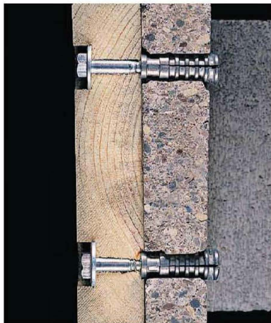
Soft metal shield anchors expand when lag screws are driven into them. They make suitable connections in either solid concrete or hollow block foundations.
