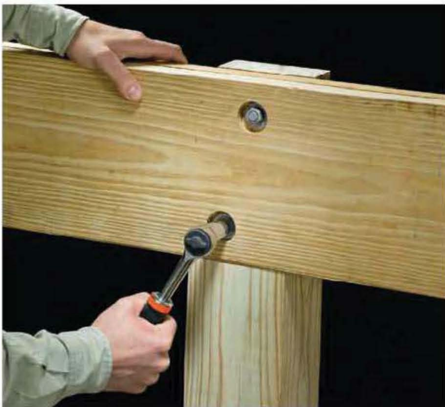
Use ½"-diameter or larger through bolts , washers and nuts for fastening beams to posts or railing posts to joists. They should be galvanized or made of stainless steel for corrosion resistance.
