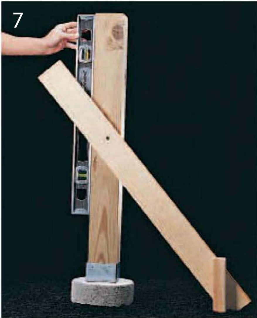
Use a level to make sure the post is plumb. Adjust the post, if necessary.
