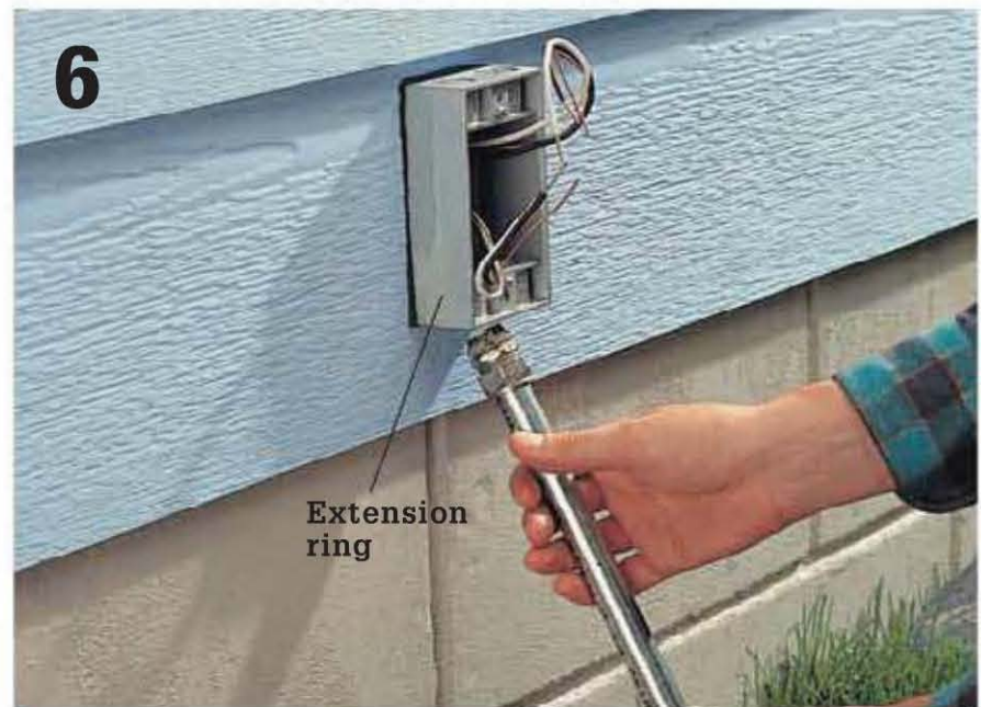
At the house, install conduit so it extends from the bottom of the extension ring to 4" from the bottom of the trench.
