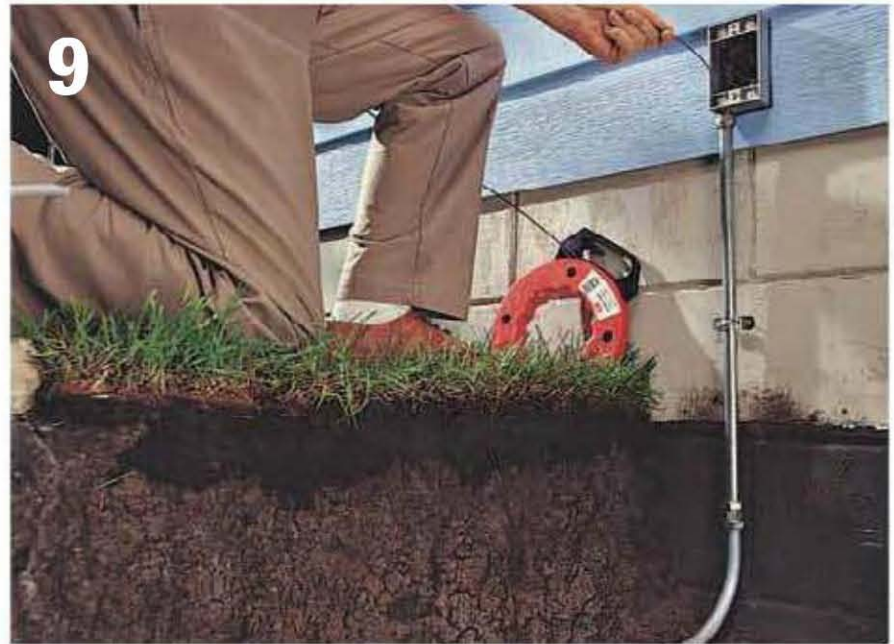
At the house, use fish tape to pull cable through the conduit and into the GFCI box.
