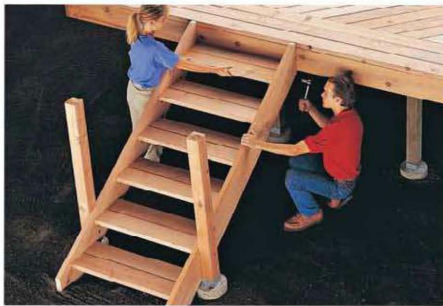
Fasten the stair to the deck with a ratchet wrench, using 4" lag screws.
