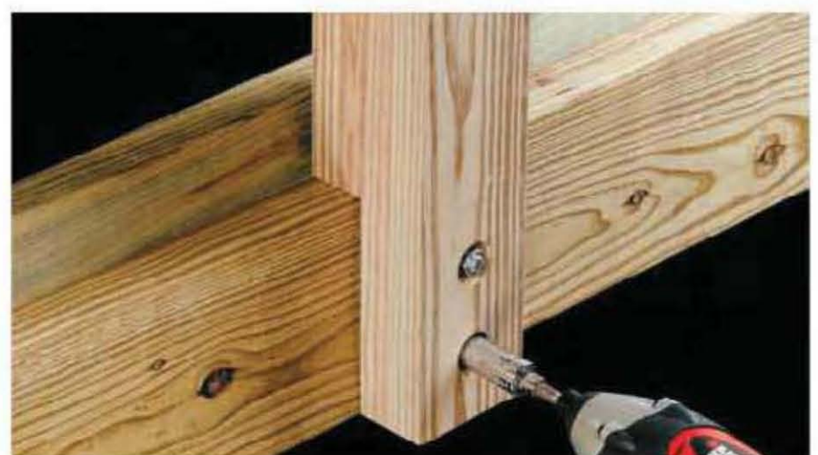
Attach the railing posts to the upper deck rim joists with carriage bolts, washers, and nuts.
