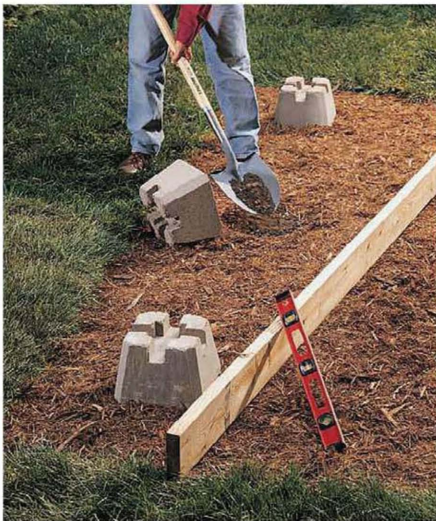
Position the corner footings and the center footing for the back joist. Remove or add soil beneath the footings to level them.
