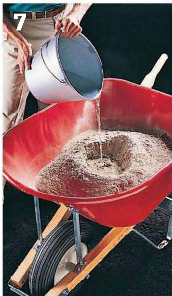
7 Form a hollow in center of dry concrete mixture. Slowly pour a small amount of water into hollow, and blend in dry mixture with a hoe.
