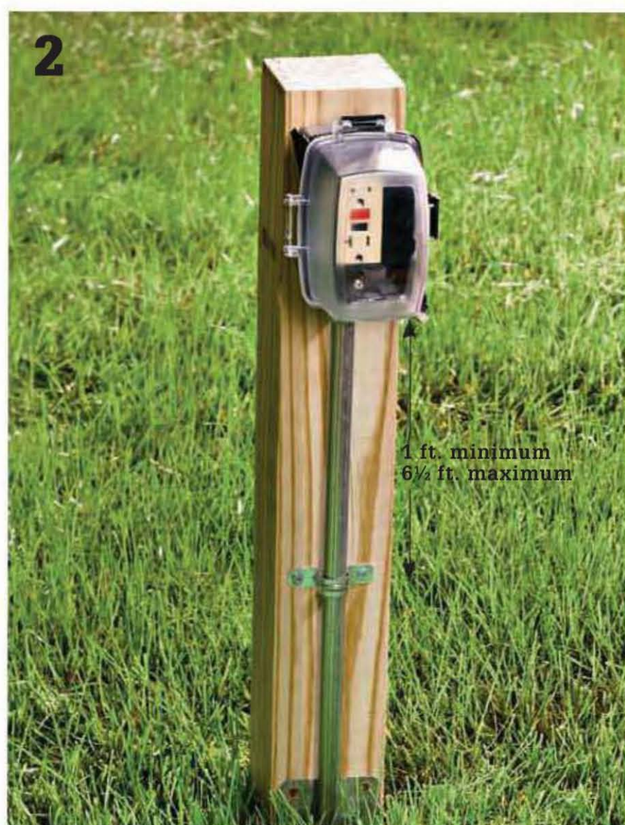
Install GFCI receptacles in weatherproof electrical boxes at least 1 ft.—and no more than 6½ ft.—above ground level.
