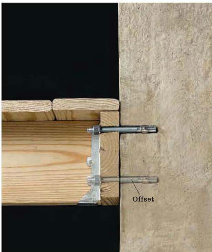
Wedge or sleeve anchors draw a wedge through a hollow sleeve, expanding it to form a tight fit in solid concrete. A nut and threaded end hold the ledger boards in place.
