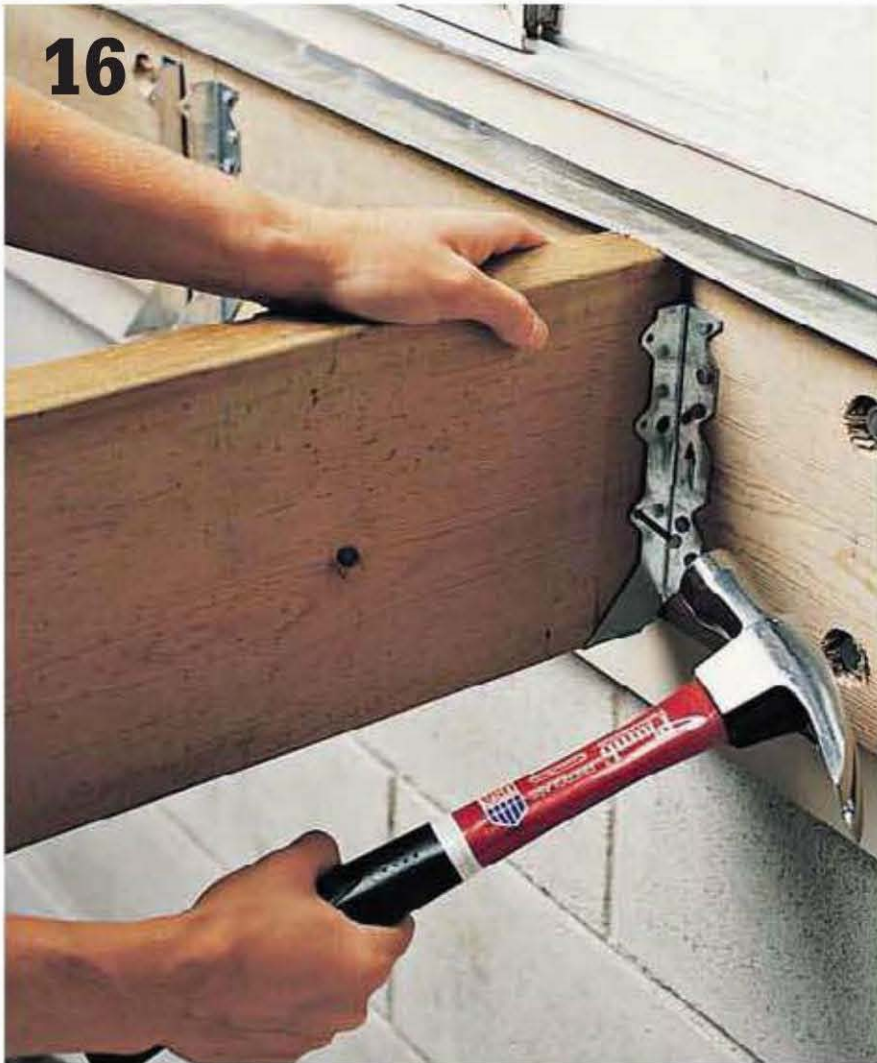
Attach the ledger joist hangers to the joists with joist hanger nails. Drive nails into both sides of each joist.
