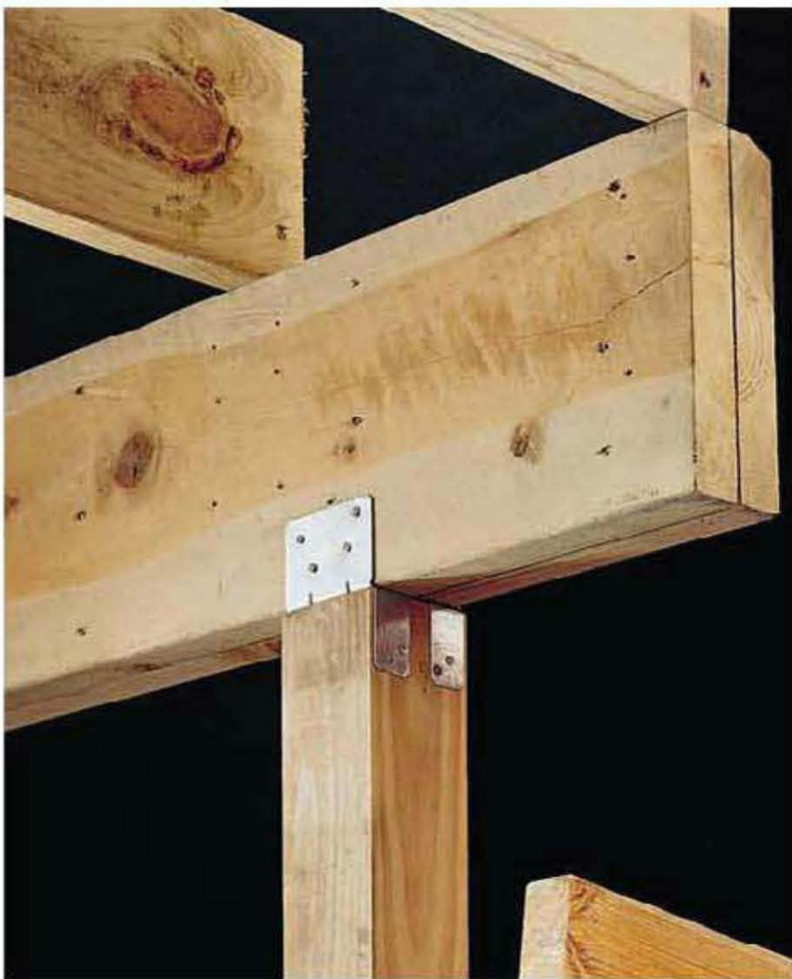
Post-beam caps secure beams on top of posts and are available in one-piece or adjustable styles.
