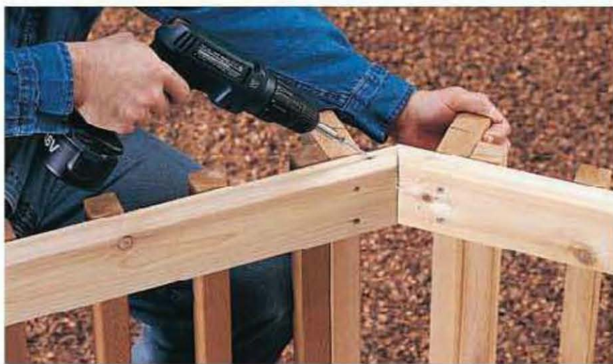
Drill \frac{1}{8} " pilot holes , then screw the top rail sections together where they meet at the corners.
