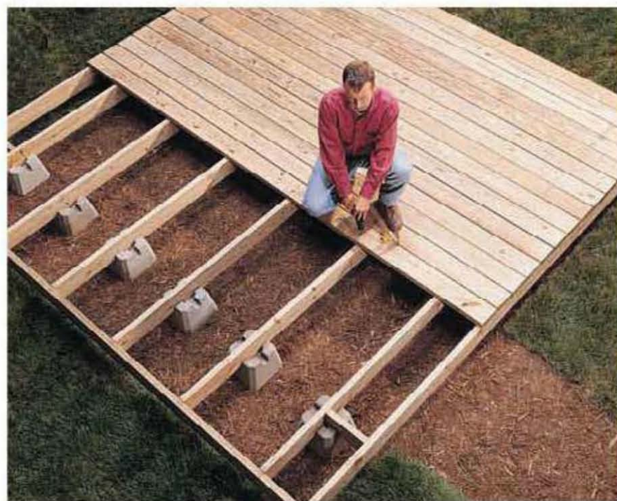
Install the decking by driving a pair of screws into each joist. Use a framing square to leave a 1/8" space between boards.
