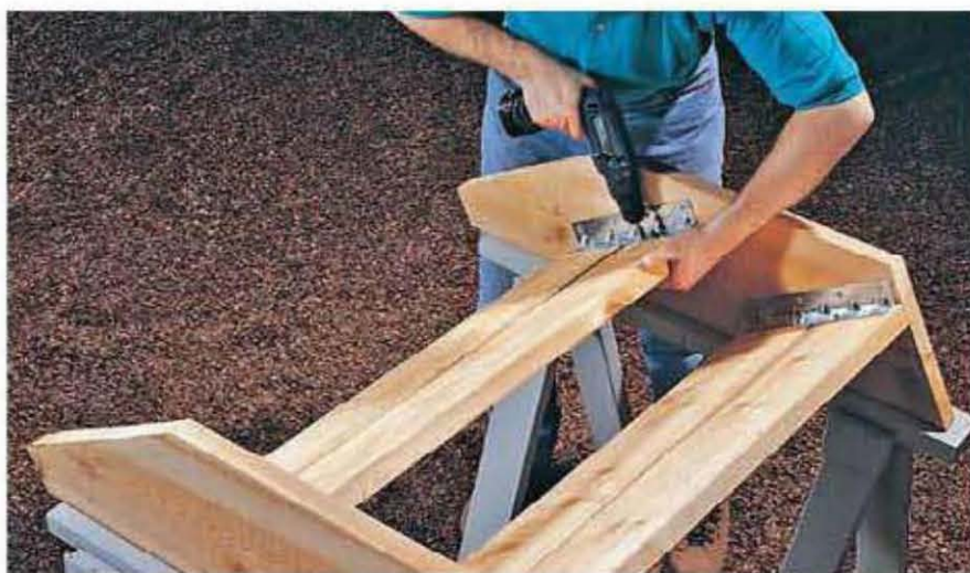
After attaching angle brackets , turn stringers upside down and install treads, using 1\frac{1}{4} " lag screws.
