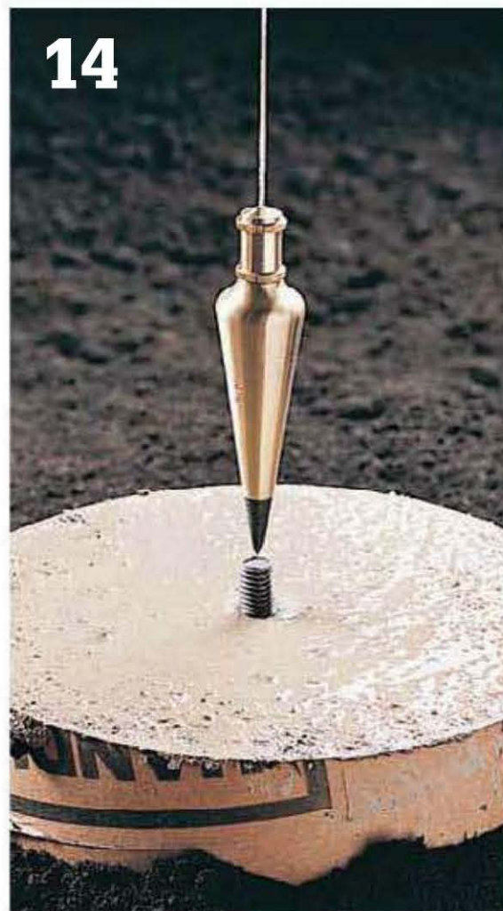
14 Use a plumb bob to make sure the J-bolt is positioned exactly at center of post location.
