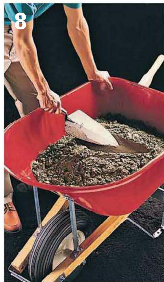
8 Add more water gradually, mixing thoroughly until concrete is firm enough to hold its shape when sliced with a trowel.
