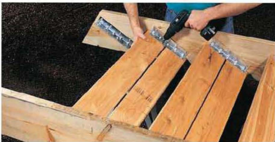
Drill pilot holes and then attach the treads to the stringers, using 1¼" lag screws and angle brackets.
