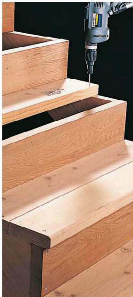
Boxed steps , built with notched stringers and solid risers, give a finished look to a deck stairway. Predrill ends of treads to prevent splitting.
