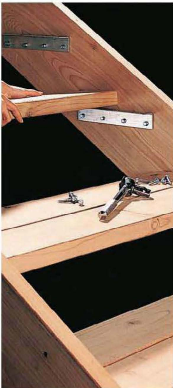
Open steps have metal cleats that hold the treads between the stringers. The treads on this stairway are built with 2 x 6s to match the surface decking.
