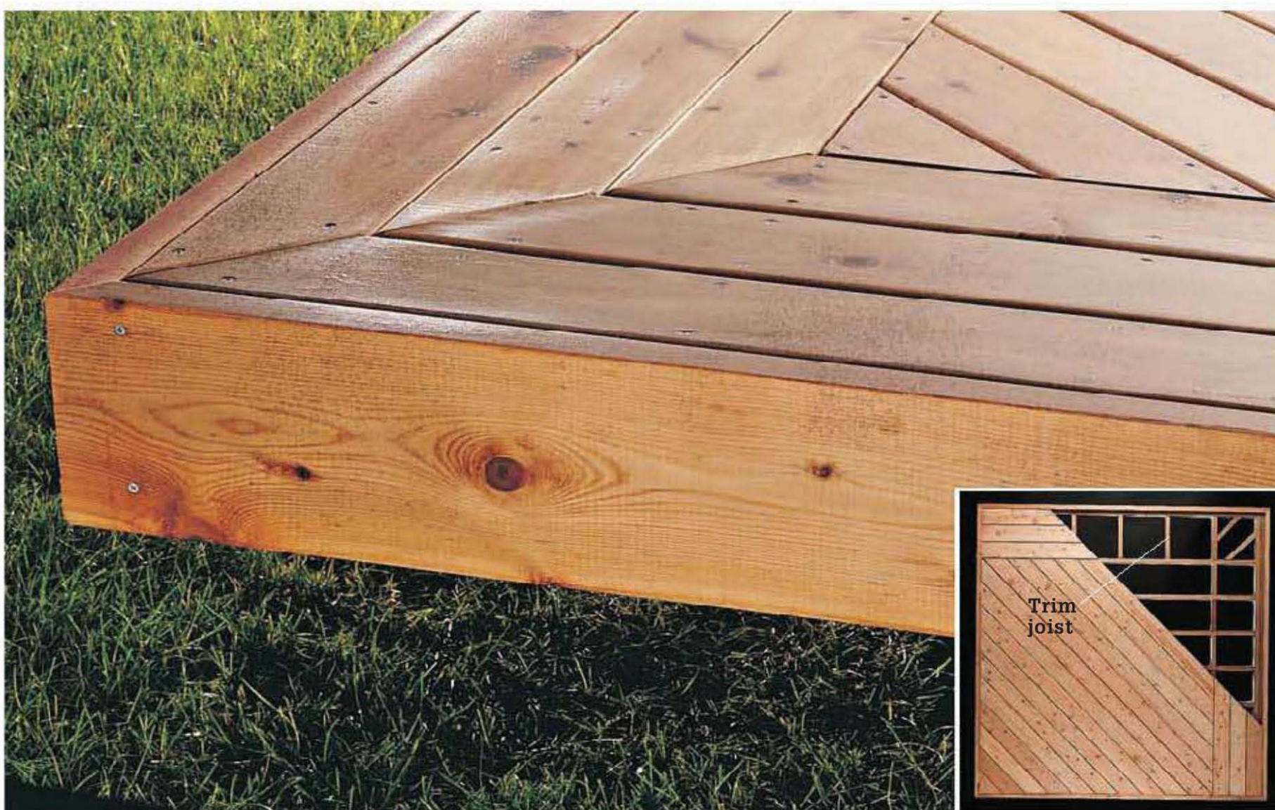
Border pattern gives an elegant, finished look to a deck. Install trim joists to support the border decking.
