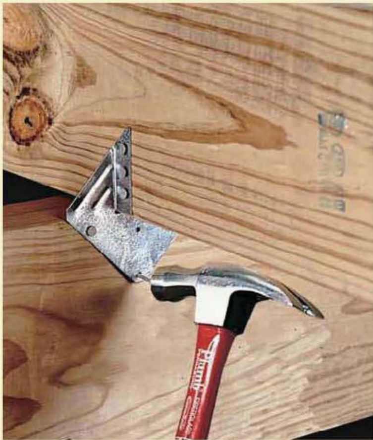
Fasten joists to beams using H-fit joist ties for strength and durability.
