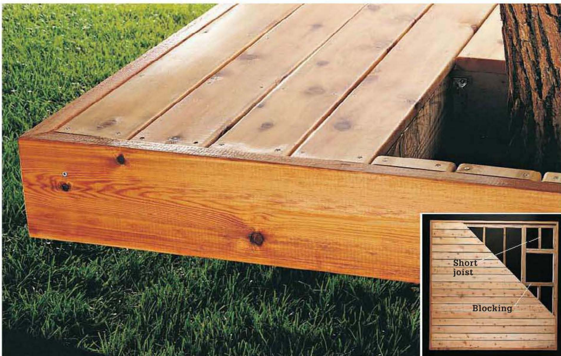
Framed opening for a tree requires extra blocking between joists. Short joists are attached to blocking with joist hangers.
