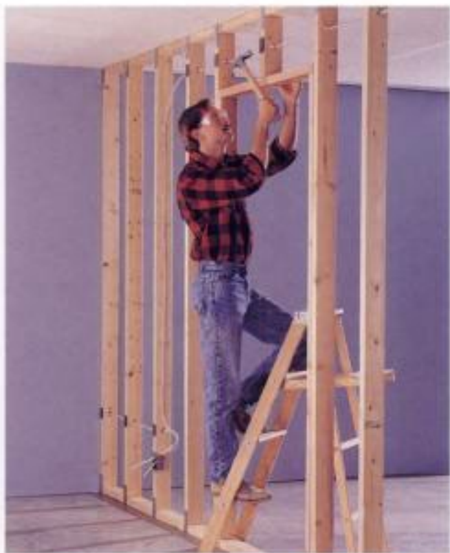
5 Drill holes and run any water pipes or wiring through the framed wall. Protect mechanicals from nail or screw punctures by covering them with flat metal plates.
