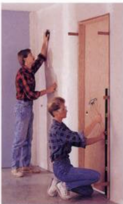
7 Install a prehung door. Prehung doors come complete with jambs.
