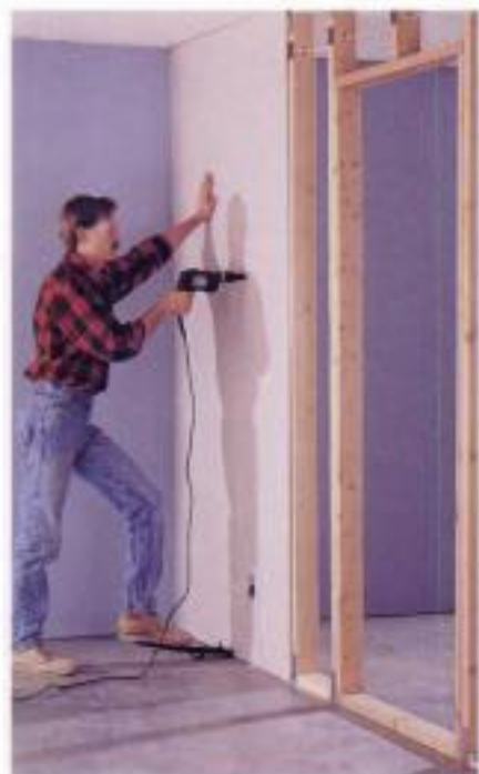
6 Install the wallboard, using \frac{1}{2} " wallboard for most applications. Finish the wallboard.
