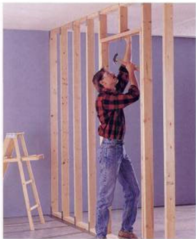
4 Frame for a prehung door. Frame the door opening \frac{1}{2} " larger on each side than the door unit.
