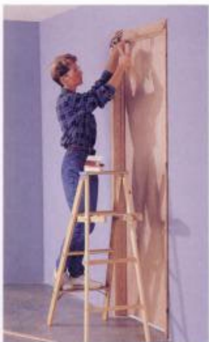
8 Cut and install the door casings. Stain or paint the trim pieces as desired.
