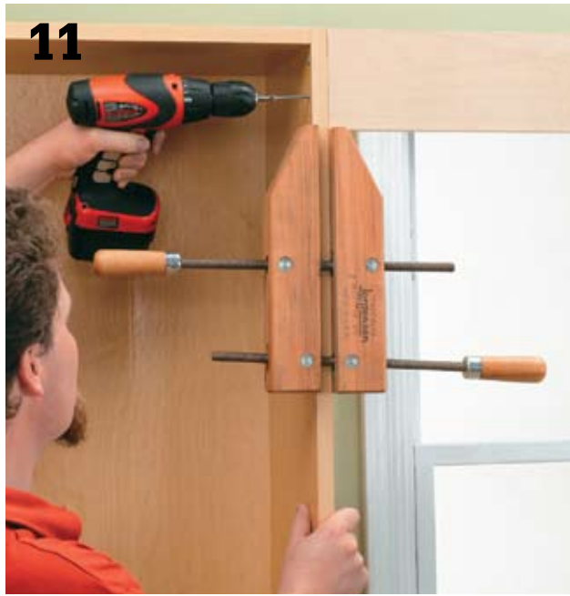
11 Attach decorative valance above the sink. Clamp the valance to the edge of cabinet frames and drill counterbored pilot holes through the cabinet frames and into the end of the valance. Attach with sheet-metal screws.
