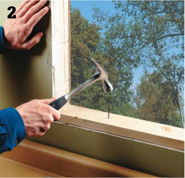
Check the rough opening measurements to verify the correct window sizing. The rough opening should be about ½" larger than the window height and width. If necessary, attach wood strips to the rough framing as spacers to bring the opening to the required size.
