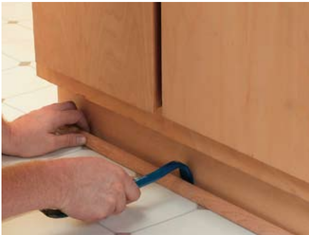
Remove base shoe from cabinet base if the molding is attached to the floor.
