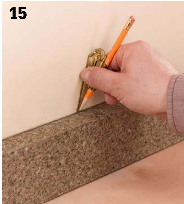
Test-fit the countertop and backplash. Because your walls may be uneven, use a compass to trace the wall outline onto the backplash-scribing strip. Use a belt sander to grind backplash to the scribe line (see page 94).
