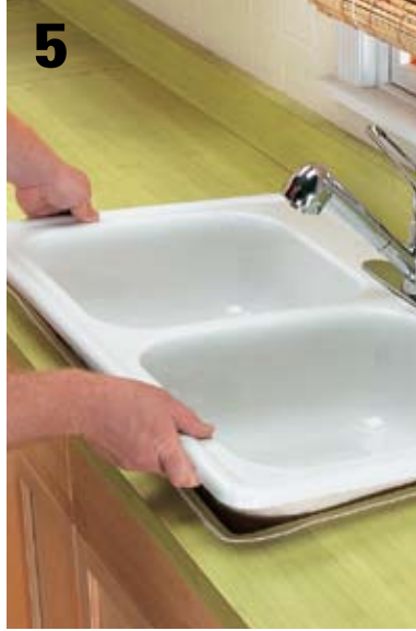
5 Place the sink in the opening. Try to get the sink centered right away so you don't need to move it around and disturb the caulk, which can break the seal. If you are installing a heavy cast-iron sink, it's best to leave the strainers off so you can grab onto the sink at the drain openings.
