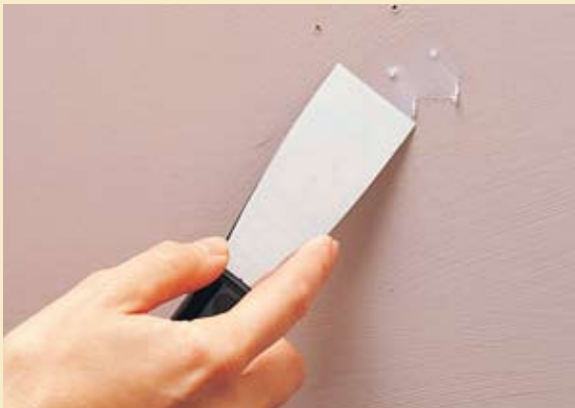
Apply lightweight spackle to holes with a putty knife or your fingertip. This keeps repair areas small. Let the spackle dry. Sand until smooth.
