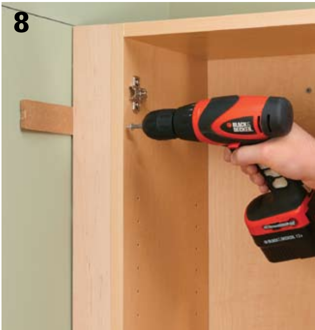
8 Fill the gaps between the cabinet and wall or neighboring appliance with a filler strip. Cut the filler strip to fit the space, then wedge wood shims between the filler and the wall to create a friction fit that holds it in place temporarily. Drill counterbored pilot holes through the side of the cabinet (or the edge of the face frame) and attach filler with screws.
