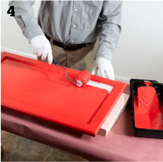
Apply a coat of latex enamel paint using 3"-wide short nap rollers. Make sure to smooth out any drips. Allow the paint to dry completely. Apply a second coat. Allow to dry thoroughly. Install the hardware and rehang the doors.
