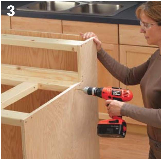
Cut the 2 × 4 cross supports to length and install them between the side panels at every corner, including the corners created by the L-shape cutout. Use 3" deck screws driven through the side panels and into the ends of the cross supports.
