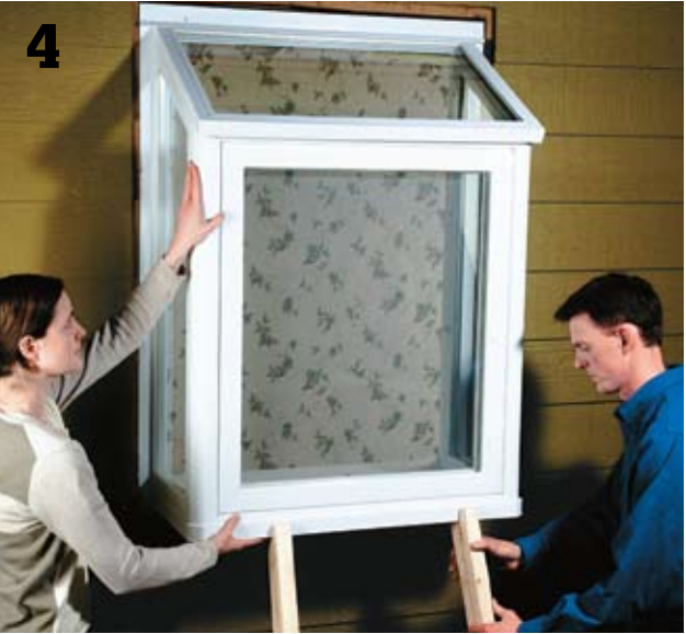
Insert the garden window into the opening, pressing it tight against the framing. Support the unit with notched 2 × 4s under the bottom edge of the window until it has been fastened securely to the framing.
