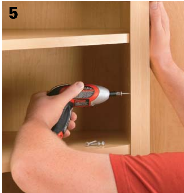
5 Attach the corner cabinet to the adjoining cabinet. From the inside corner cabinet, drill pilot holes through the face frame. Join the cabinets with sheet-metal screws.
