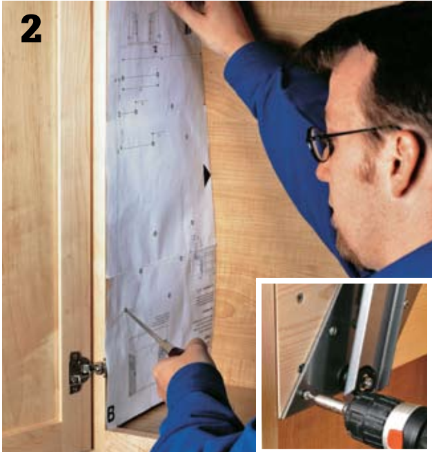
Use the template as a reference for marking the location of the swing arm mounting plates with a scratch awl. Drill a pilot hole at each mark. Fasten the swing arms to the custom spacers or cabinet sides with #8 panhead screws (inset). The screws should not go completely through the cabinet side.
