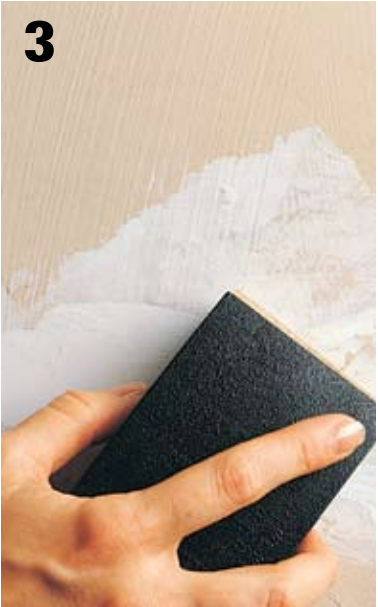
Sand the patch area with 150-grit production sandpaper. The patch area should feel smooth to the touch.
