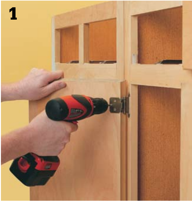
1 Remove doors and drawers to make it easier to get at interior spaces. You may need to scrape away old paint to expose hinge screws.
