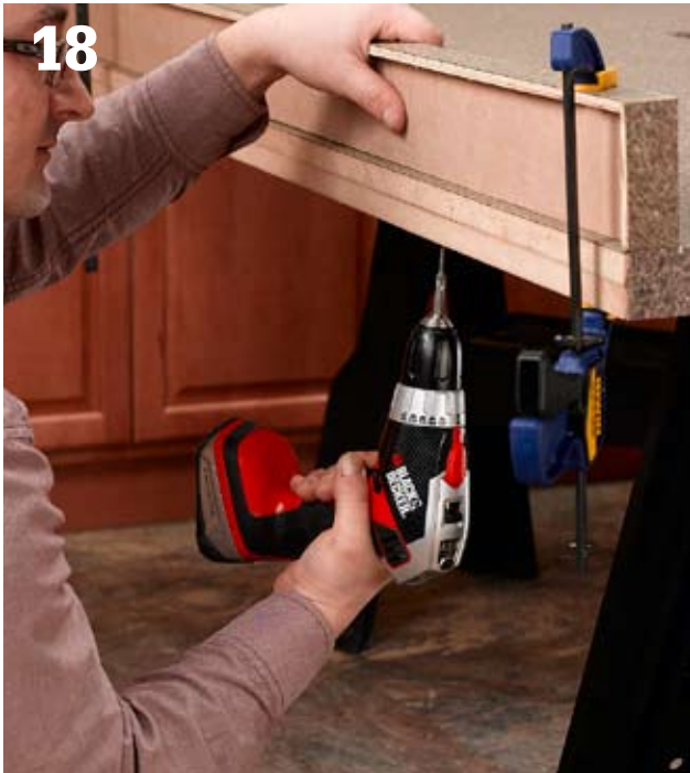
Screw 2" wallboard screws through the countertop and into the backplash core. Make sure the screw heads are countersunk completely for a tight fit against the base cabinet. Install the countertops.
