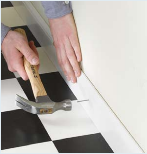
Drive nails into the wall surface —not through the vinyl flooring—when installing the baseboard or base shoe. Anchoring the flooring with perimeter nails may result in buckling of the vinyl surface when the floor expands or contracts. Also, do not press the molding down into the vinyl. Leave a small gap between the molding and the floor surface so the vinyl is not constricted.
