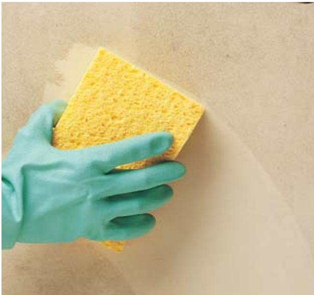
Wash kitchen walls thoroughly before painting. Grease and dirt will prevent paint from adhering fully.
