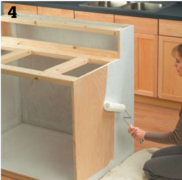
Prime and paint the cabinet interior and exterior.
