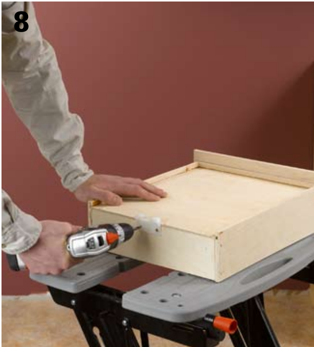
Install drawer slide hardware on the drawer. Slides may be center-mounted, as seen here, or side-mounted in pairs. Typically, side-mounted slides are rated for higher weight capacity.
