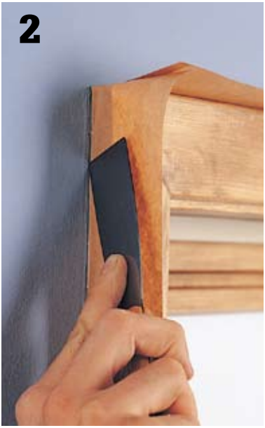
After applying the tape , run the tip of a putty knife along the inside edge of the tape to seal it against seeping paint. After painting, remove the tape as soon as the paint is too dry to run.
