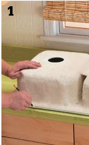
1 Invert the sink and trace around the edges as a reference for making the sink cutout cutting lines, which should be parallel to the outlines, but about 1" inside of them to create a 1" ledge. If the sink comes with a template for the cutout, use it.
