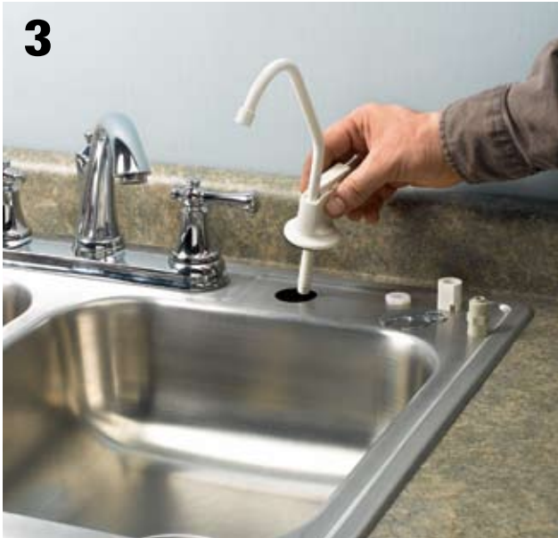
Remove the sprayer from the sink , if necessary, or cut a new hole through the countertop, following the countertop manufacturer's recommendations (some materials require a professional fabricator). Assemble the filter spout as directed, and then mount the spout into the sink hole, using plumber putty as a sealant.
