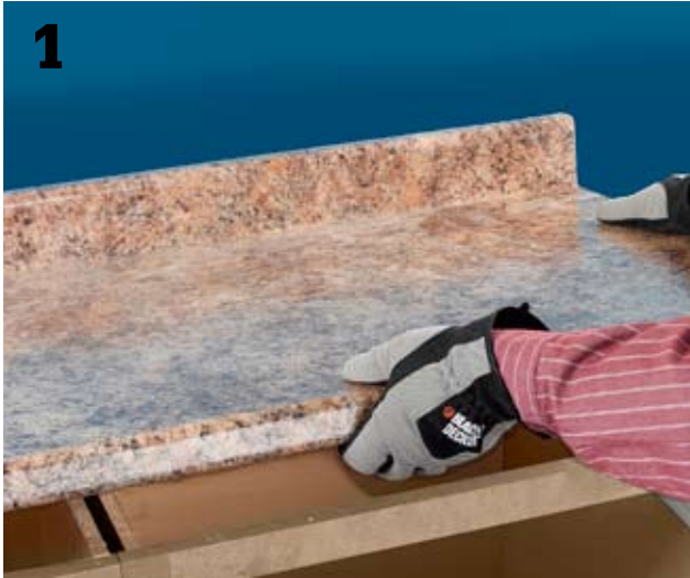
Remove the countertops. From inside the base cabinets, unscrew the screws holding the countertops to the cabinets. Unscrew take-up bolts on mitered sections of the countertop. Use a utility knife to cut through the caulk, if present. Countertops should lift off easily, but if they don't, you can use a prybar to carefully pry them away from the base cabinets. Note: In some cases you can install these tiles over old laminate countertops (see previous page).
