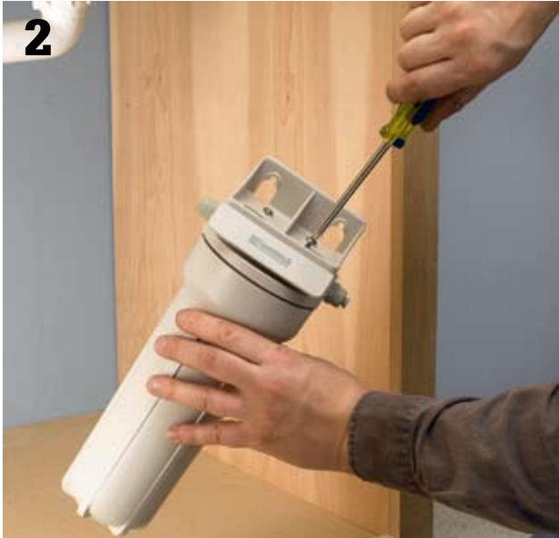
Secure the mounting bracket to the filter unit, then mount the unit at a convenient location under the sink, following the manufacturer's directions. Be sure to leave plenty of room for removing the filter housing for filter replacement.
