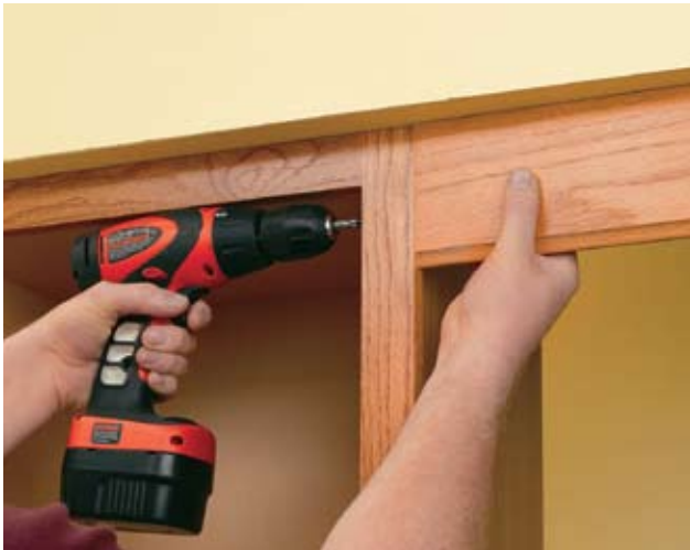
Remove valances above cabinets. Some valances are attached to the cabinets or soffits with screws. Others are nailed and must be pried loose.
