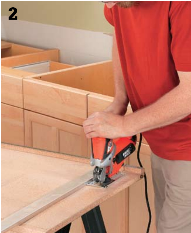
Use a framing square to mark a cutting line on the bottom surface of the countertop. Cut off the countertop with a jigsaw using a clamped straightedge as a guide.
