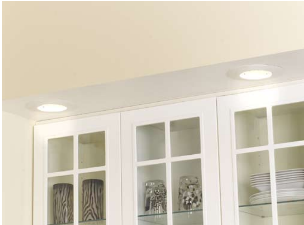
Build a soffit with framing lumber and drywall to open up new possibilities for installing task lighting or running ventilation ductwork.
