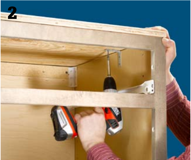
Prepare and install the subbase. Measure the cabinet bank from outside edges to outside edges on all sides and cut a piece of 5/8"-thick exterior grade plywood to fit. The edges of the plywood should be flush with the outside edges of the cabinet tops. Screw the plywood to the cabinet braces from underneath.
