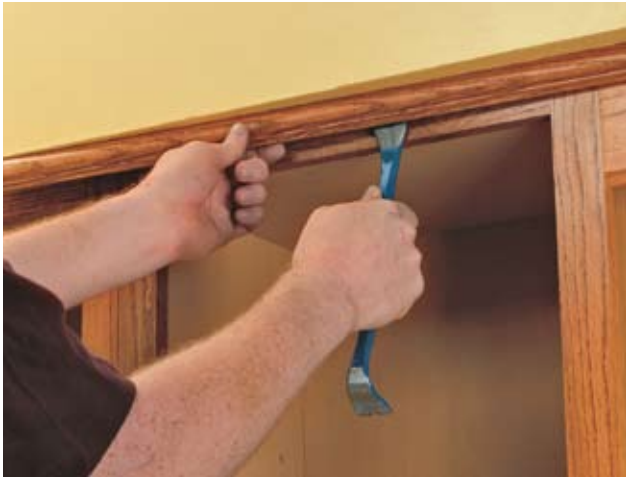
Remove trim moldings at the edges and tops of the cabinets with a flat pry bar or putty knife.
