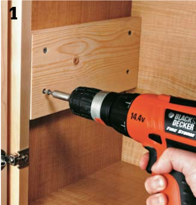
Use the shelf manufacturer's paper template to determine the general positions of the swing arms, then fasten the wood spacers to the inside faces of the cabinets with coarse-thread wallboard screws. The screws should not go completely through the cabinet side.
