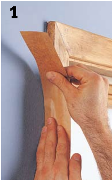
Use pregummed paper or wide masking tape to protect wood moldings from paint splatters. Leave the outside edge of the masking tape loose.
