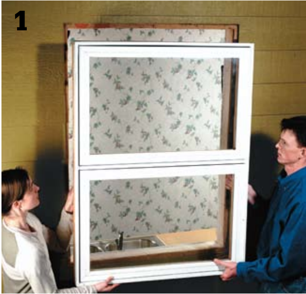
Prepare the project site and remove the interior and exterior trim, then remove the existing window.
