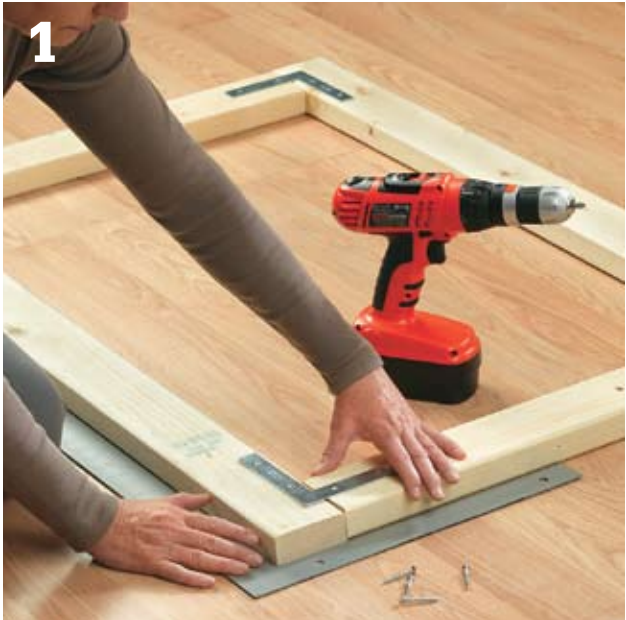
Build a 2 × 4 base for the island cabinet by cutting the 2 × 4s to length and joining them in a square frame that lays flat (wide sides down) on the floor. Use metal L-brackets to reinforce the joints. If you don't wish to move the island, fasten the frame to the floor in position with construction adhesive and/or deck screws.
