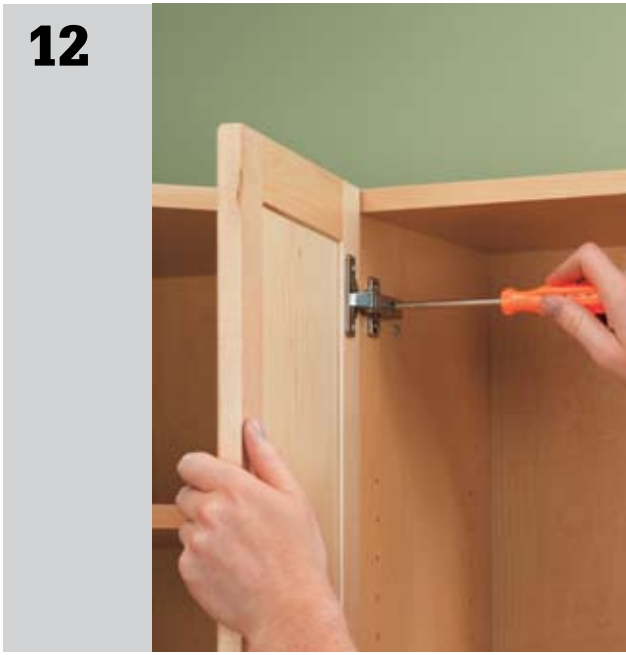
12 Install the cabinet doors. If necessary, adjust the hinges so that the doors are straight and plumb.
