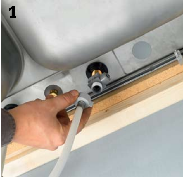
Shut off the cold water supply to the kitchen faucet at the fixture shutoff valve or the main house valve; drain the faucet. Remove the supply tubing from the faucet stud using a wrench. Wrap the stud with Teflon tape, then thread the filter's water supply fitting onto the stud and tighten carefully. Apply the tape and connect the supply tubing to the fitting.
