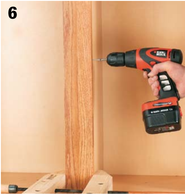
6 Position and attach each additional cabinet. Clamp frames together, and drill counterbored pilot holes through the side of the face frame. Join the cabinets with wood screws. Drill \frac{3}{16} " pilot holes in the hanging strips, and attach the cabinet to the studs with wood screws.
