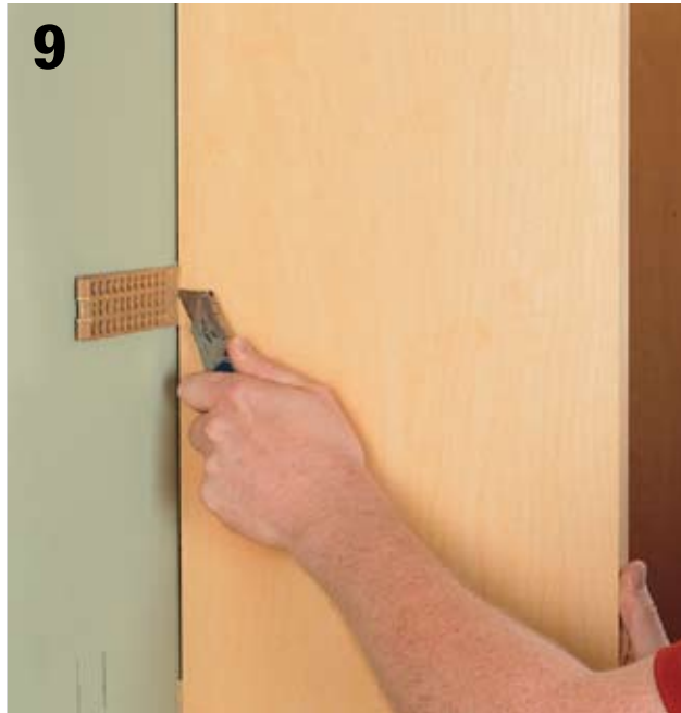
9 Remove the temporary ledger. Check the cabinet run for plumb, and adjust if necessary by placing wood shims behind the cabinet, near the stud locations. Tighten the wall screws completely. Cut off the shims with a utility knife.
