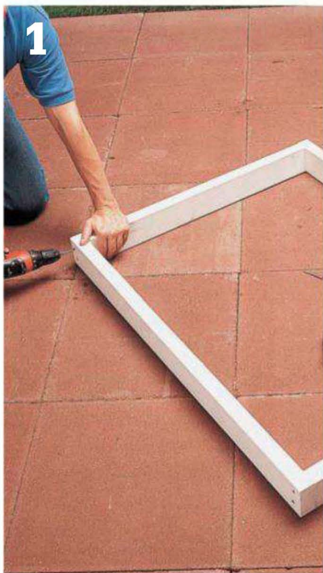
Make the frame. Determine the lengths of the horizontal and vertical braces of the frame then lay out the boards, check them for square, and secure the joints with 2½" deck screws.
