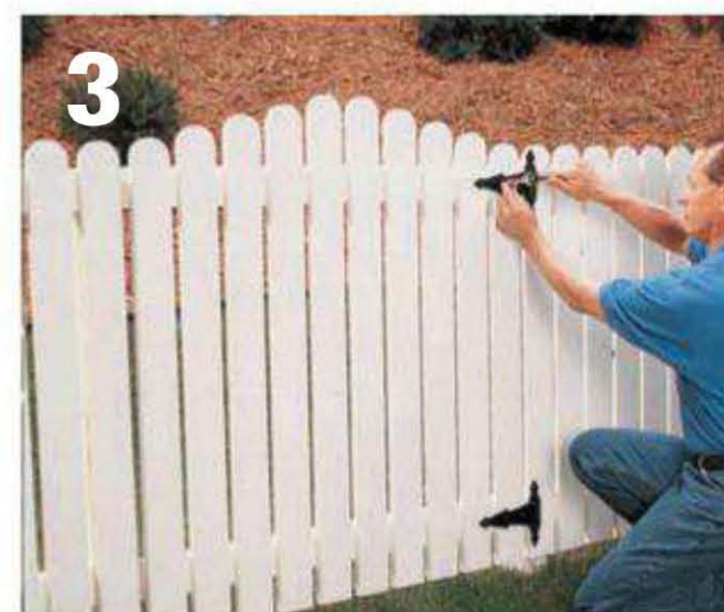
Install the gate. Shim the gate into place with blocking below and mark the position of the hardware on the gate and gateposts. Attach the hardware.
