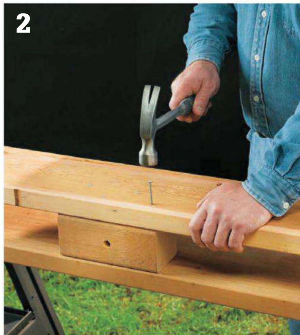
Sandwich the blocks between the main beams, and fasten the assemblies with exterior adhesive and 16d nails.
