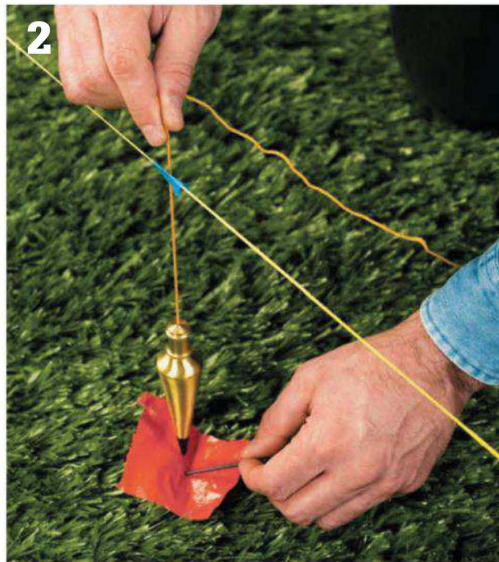
Transfer post locations from the string to the ground and mark them with pieces of plastic pinned to the turf.
