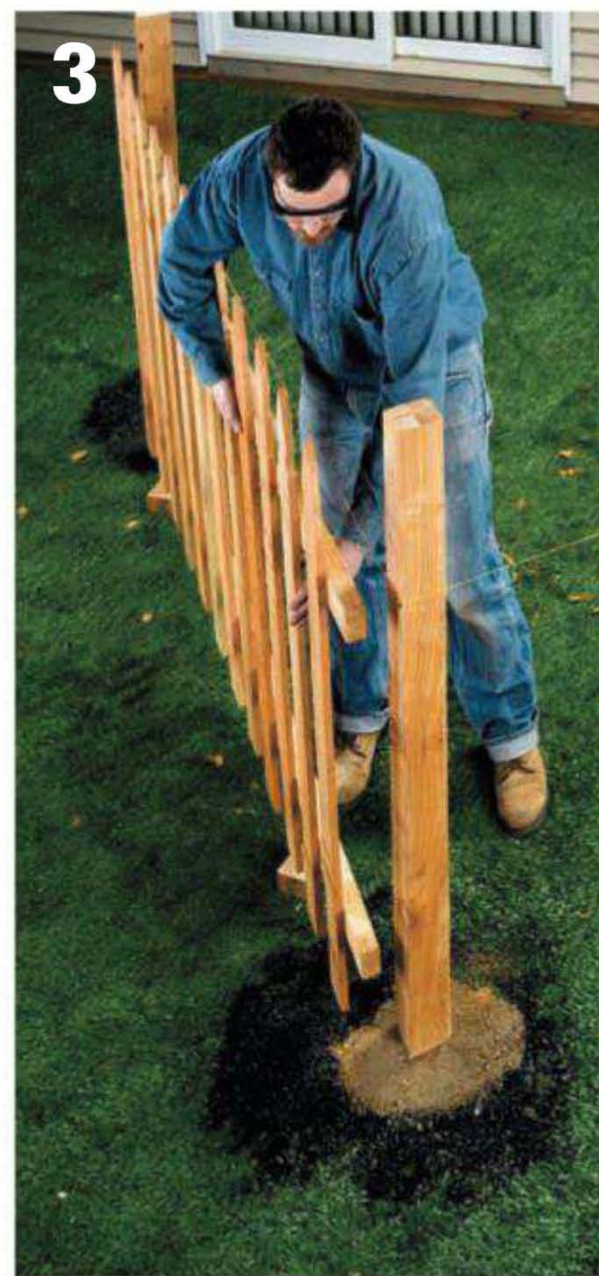
String a mason's line across all the posts to set the height for the stringers. Check with a line level. Position one of the panels against the posts it will attach to, resting on spacer blocks that are at least 2" high.
