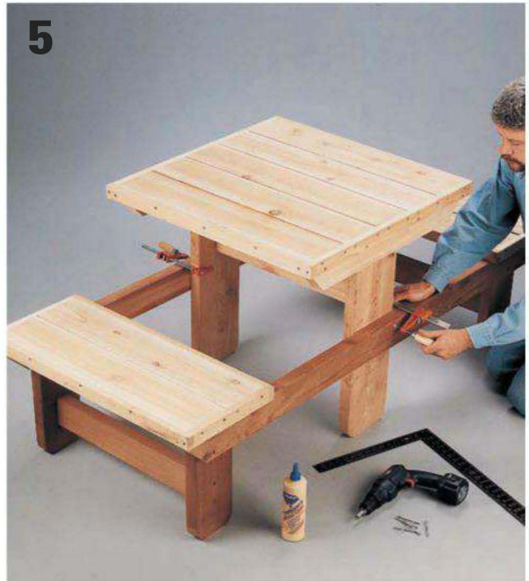
5 Center the table within the cross rails, and then clamp it in place. Secure the cross rails to the table legs with deck screws driven into counterbored pilot holes.
