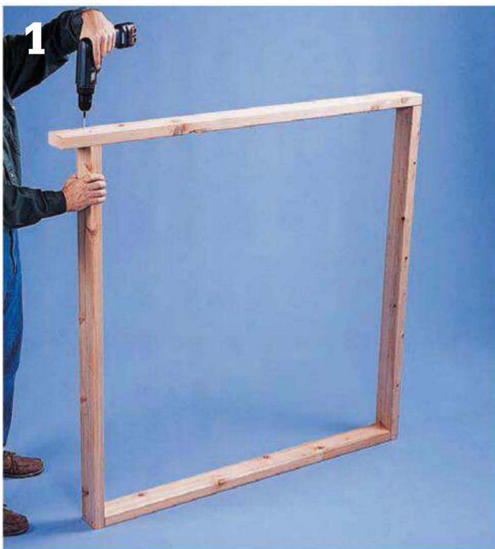
Attach the long rail at the top of one trellis frame with a 3\frac{1}{2} " overhang at one end to cover the post.
