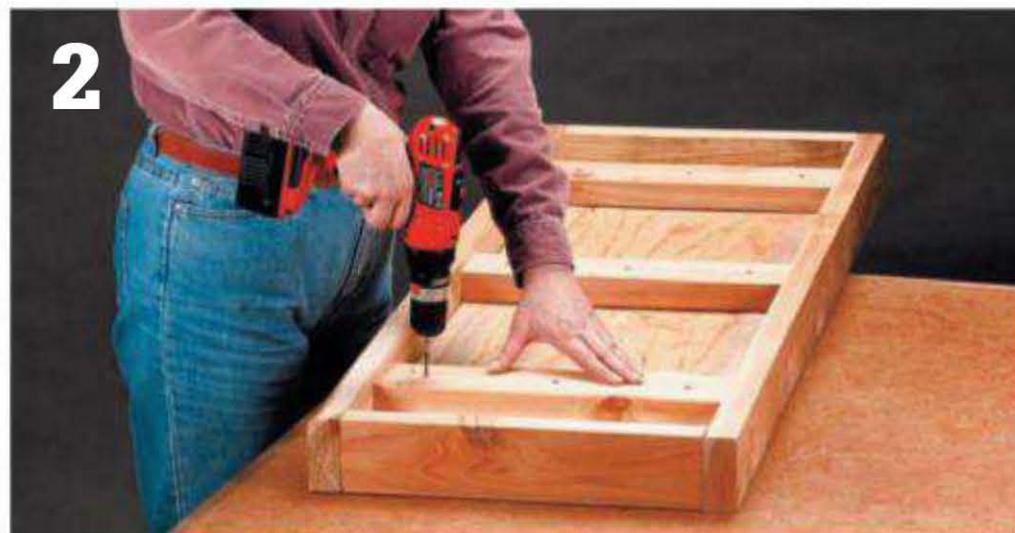
2 Position the frame over the subbase and fasten it by driving 2" deck screws through the stretchers and into the plywood. Also drive some screws down through the cementboard underlayment and plywood and into the stretchers.
