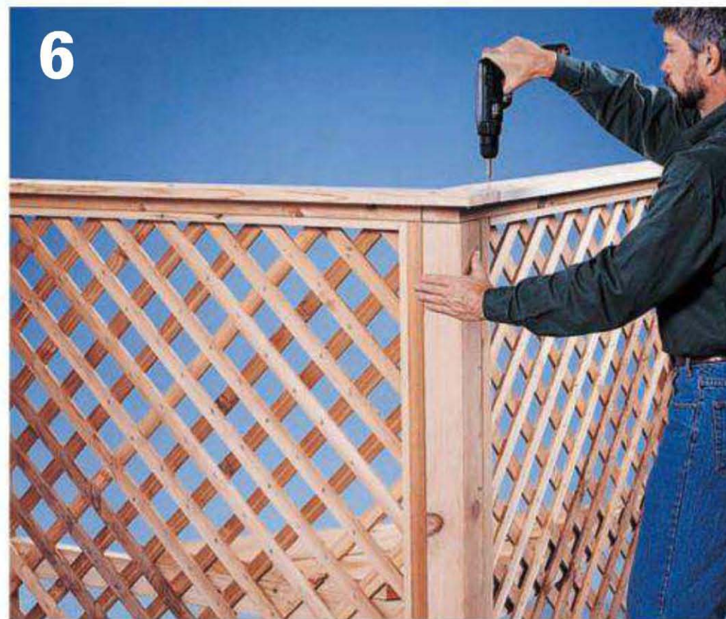
Attach the long and short caps to the tops of the trellis frames. The long cap overlaps the long rail and the post.
