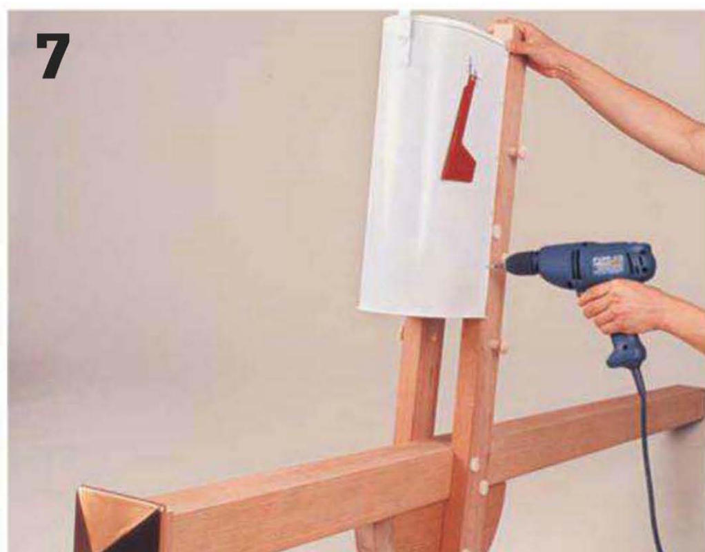
Attach the mailbox to the box shelf by driving screws through the side flanges of the mailbox.
