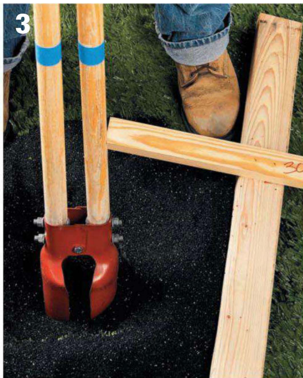
Dig a posthole at a corner or an end post location. A clam-shell-type posthole digger is a good choice for holes up to 30" deep. Make a depth gauge from scrap wood to measure the hole depth as you dig.
