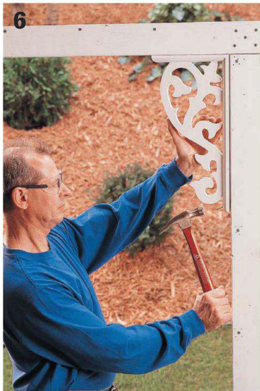
Add millwork brackets at each corner where the tie beams and the trellis frame posts meet. Secure with finish nails.
