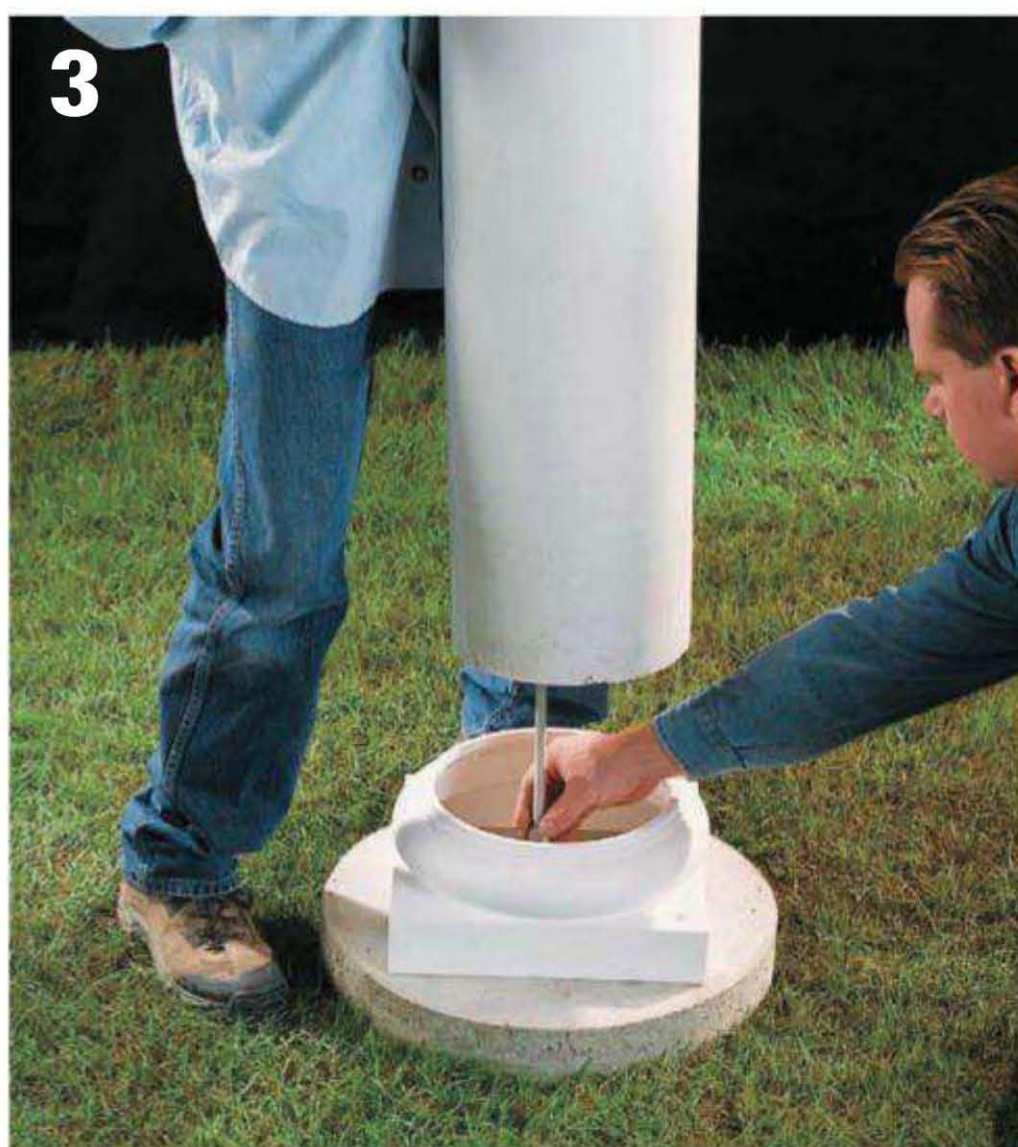
Install the columns. Have one person lift up the column while another tightens the coupler nut to the J-bolt and threaded rod.
