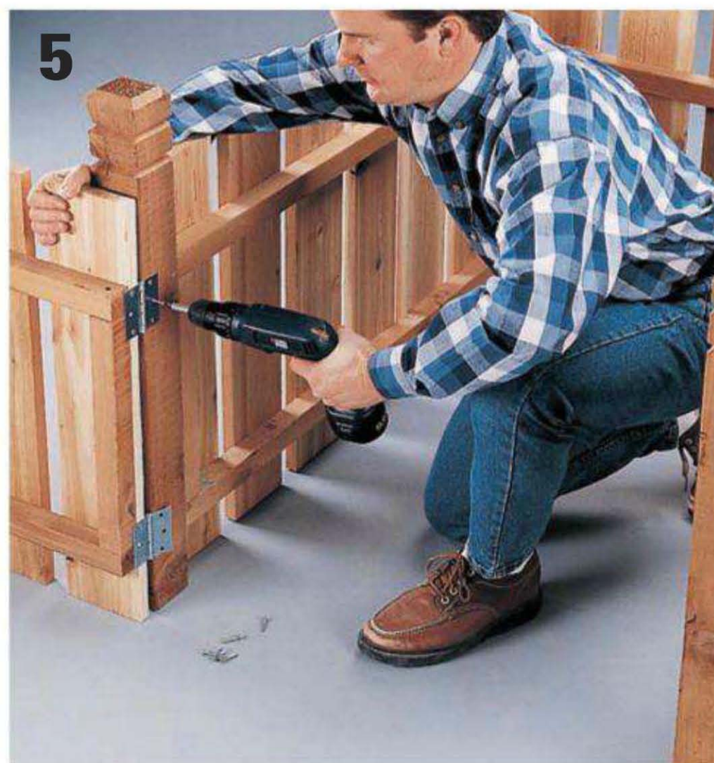
Attach exterior-rated hinges to the end panel frame and then fasten them to the post. Add a latch on the other side of the hinged panel.
