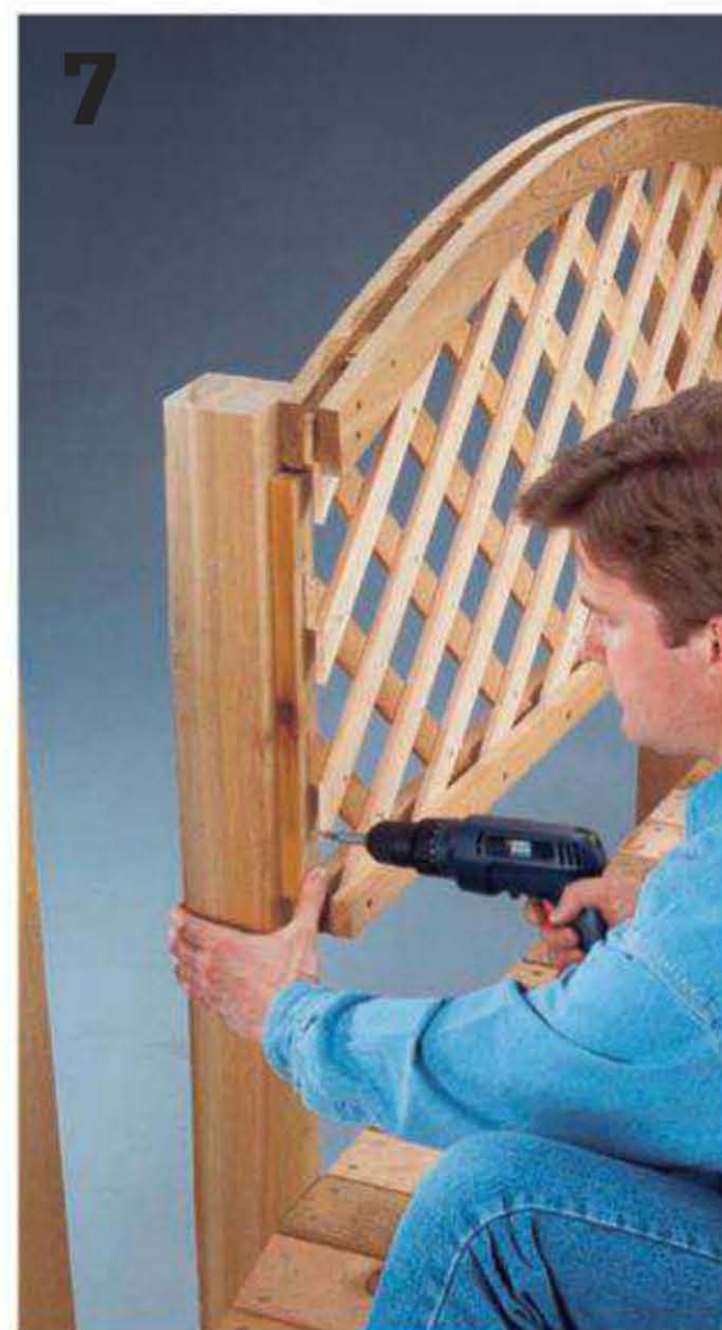
Fasten 1 x 2 filler strips to the posts to close the gaps at the sides of the lattice panels.
