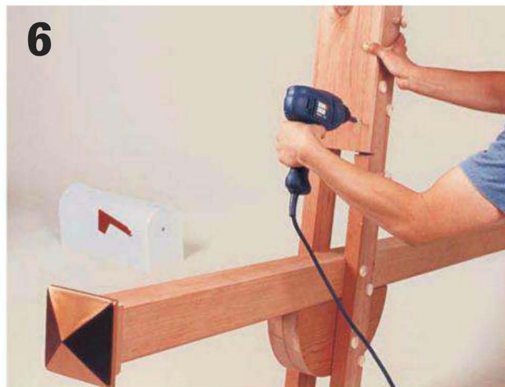
Attach the shelf for the mailbox to the side rails.
