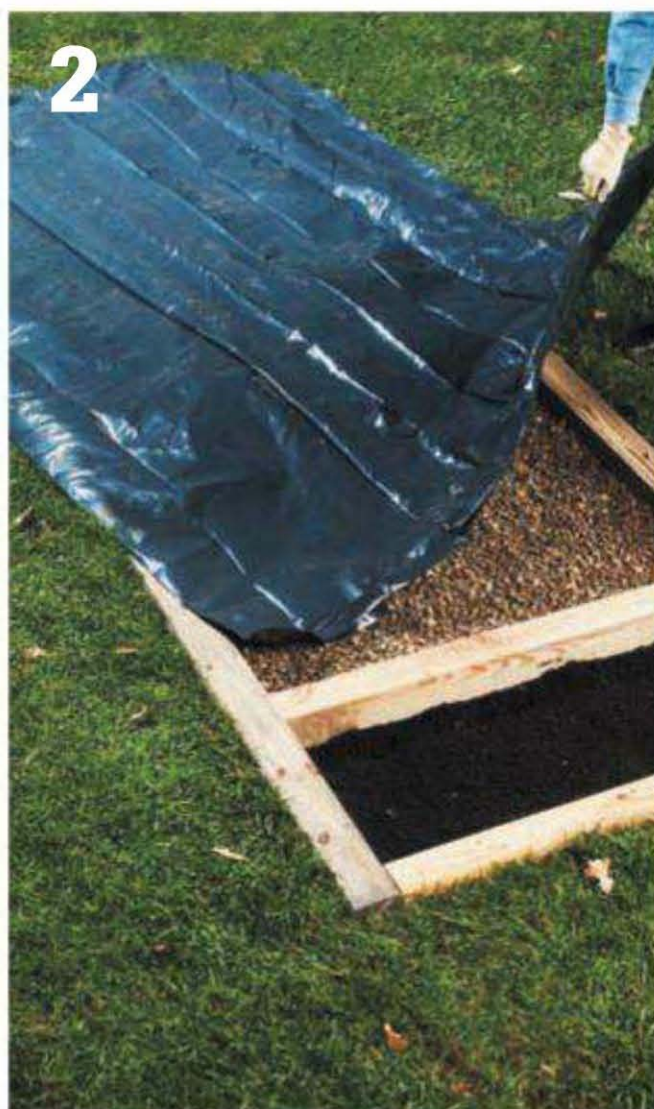
Prepare the base. Lay the first row of timbers, including the wall for the storage box. Fill the sandbox area with a 2" layer of gravel, and cover with plastic sheathing.
