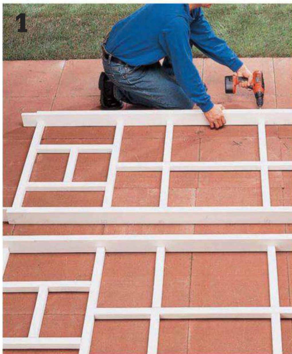
Lay out the pieces for each side of the trellis frame, then secure each joint with 2½" deck screws.
