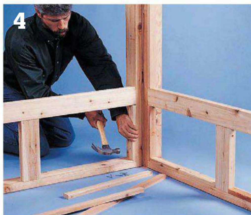
Nail 1 x 2 retaining strips for the lattice panels to the inside faces of the trellis frames.
