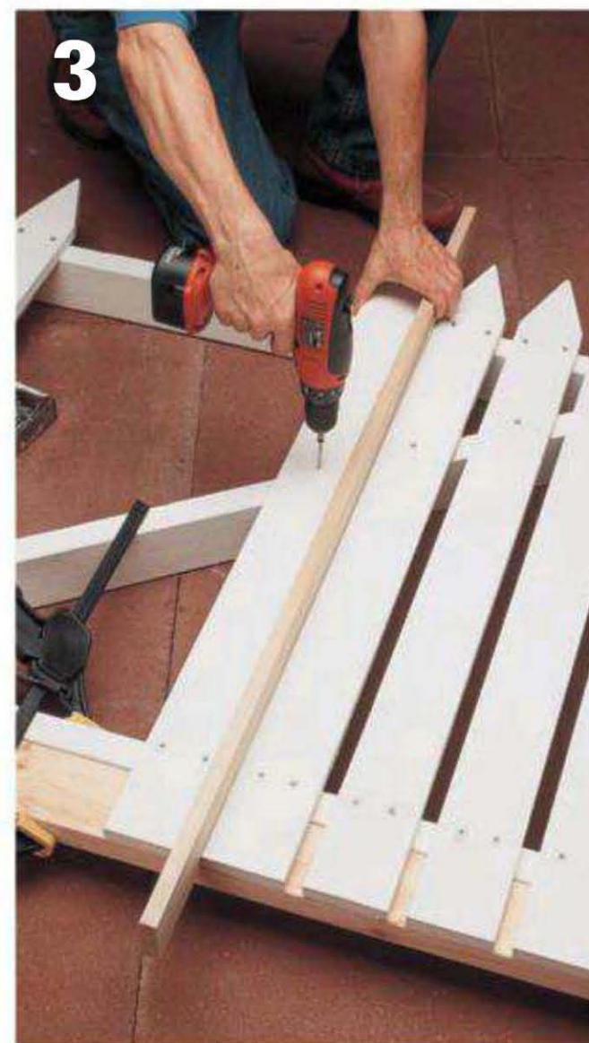
Secure the siding boards to the frame with deck screws using scrap wood as spacers.
