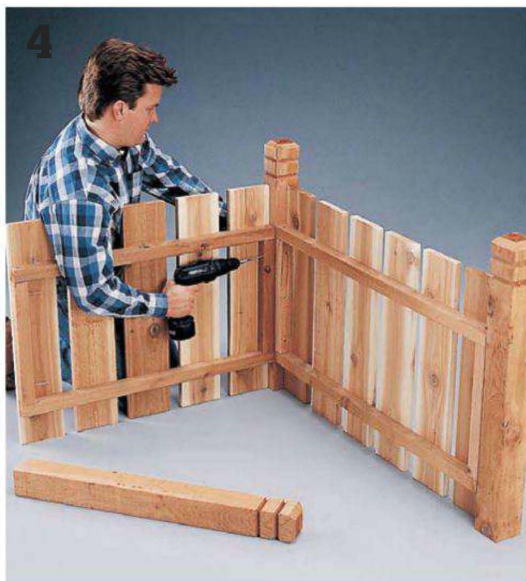
Stand the posts and panels upright, and fasten the panels to the posts by driving screws through the cleats.
