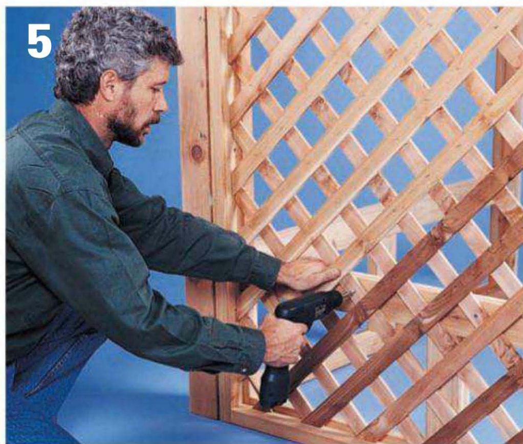
Fasten the lattice panels to the seat supports with 1¼" deck screws, and then attach outer retaining strips.
