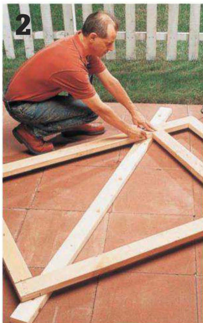
Position a diagonal brace from the bottom of the hinge side to the top of the first horizontal brace of the frame. Mark and cut the brace, then fasten it into the frame..
