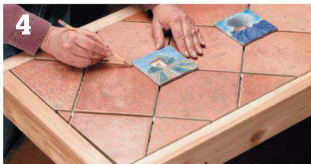
4 Dry-fit the field tiles using tile spacers to set consistent gaps. Set the accent tiles in place and mark the field tiles for cutting.
