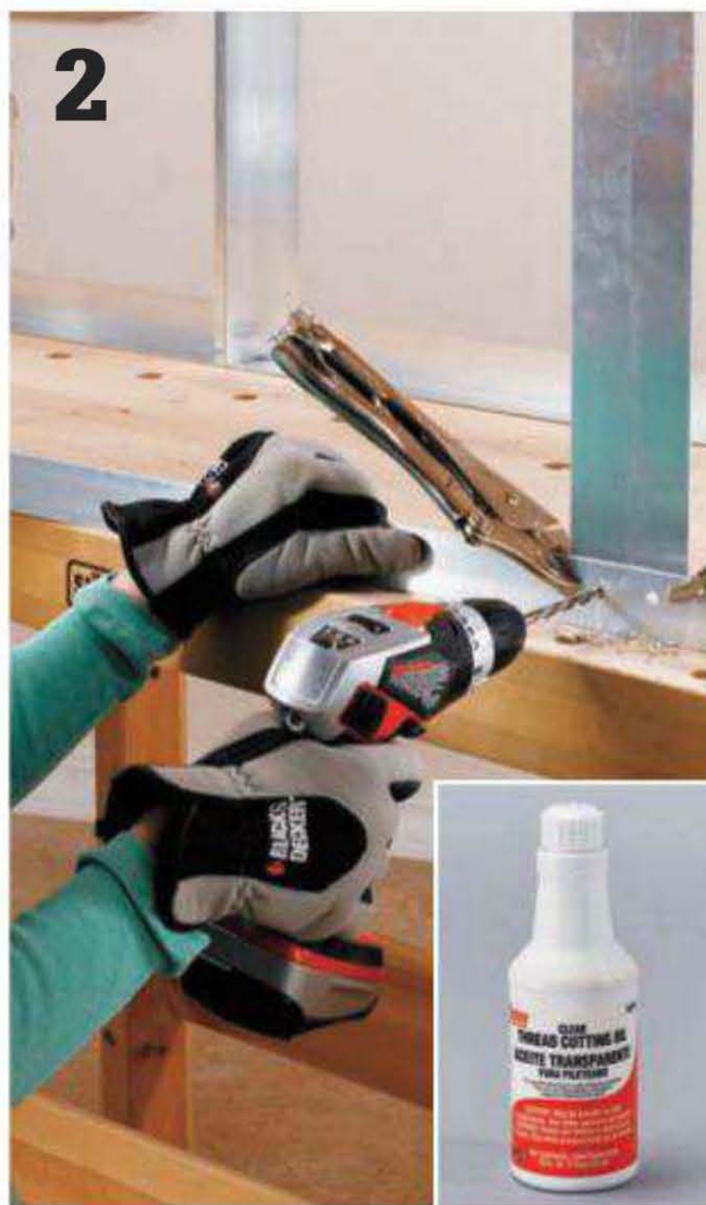
Drill guide holes for bolts. Clamp the part for each joint together with locking pliers and then drill for one \frac{1}{4} " bolt per joint. Apply a drop of cutting oil (inset) to the metal before drilling.
