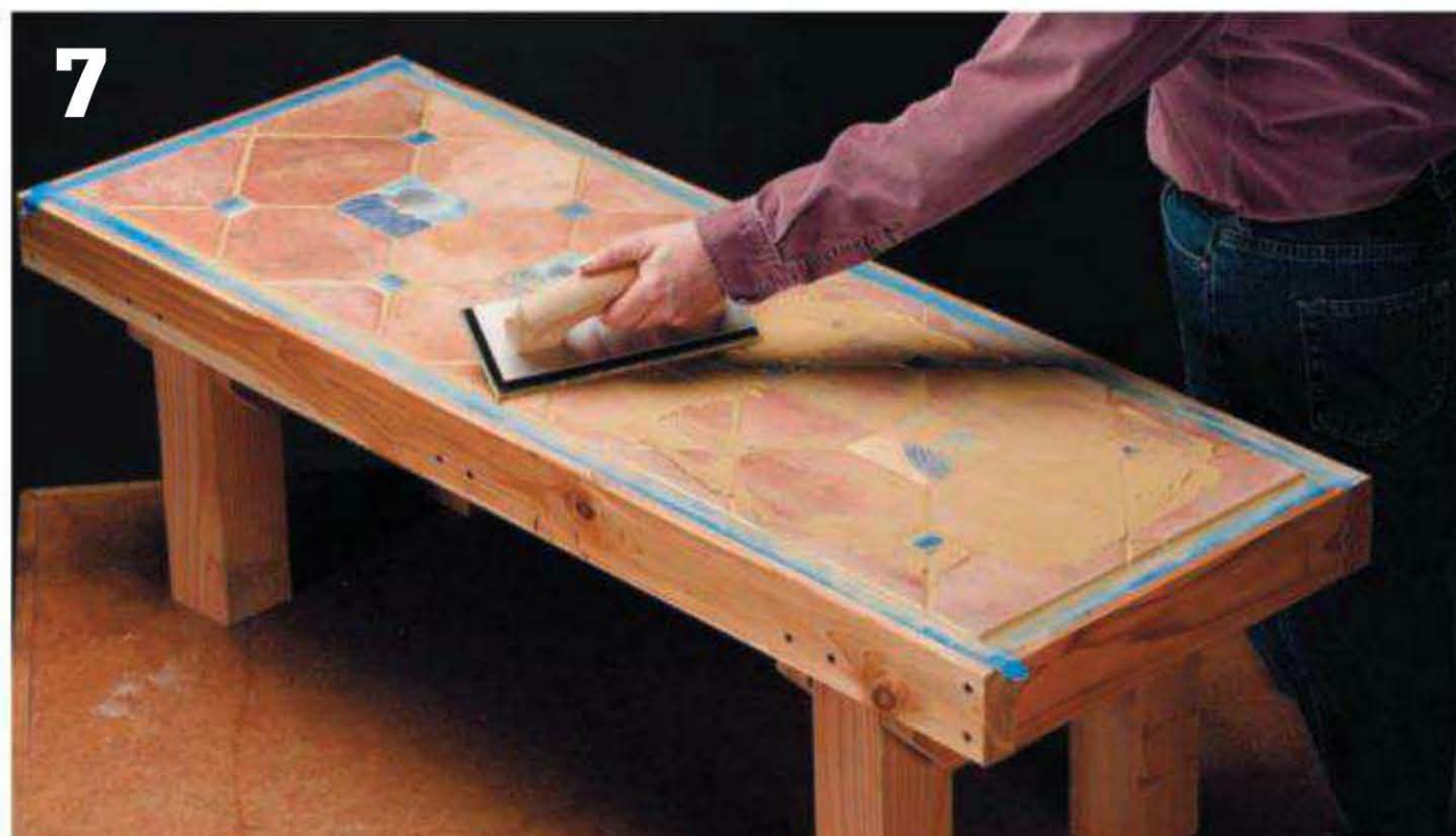
Mix a batch of grout and use a grout float to force it into the joints between tiles. Buff off the excess once the grout sets up.
