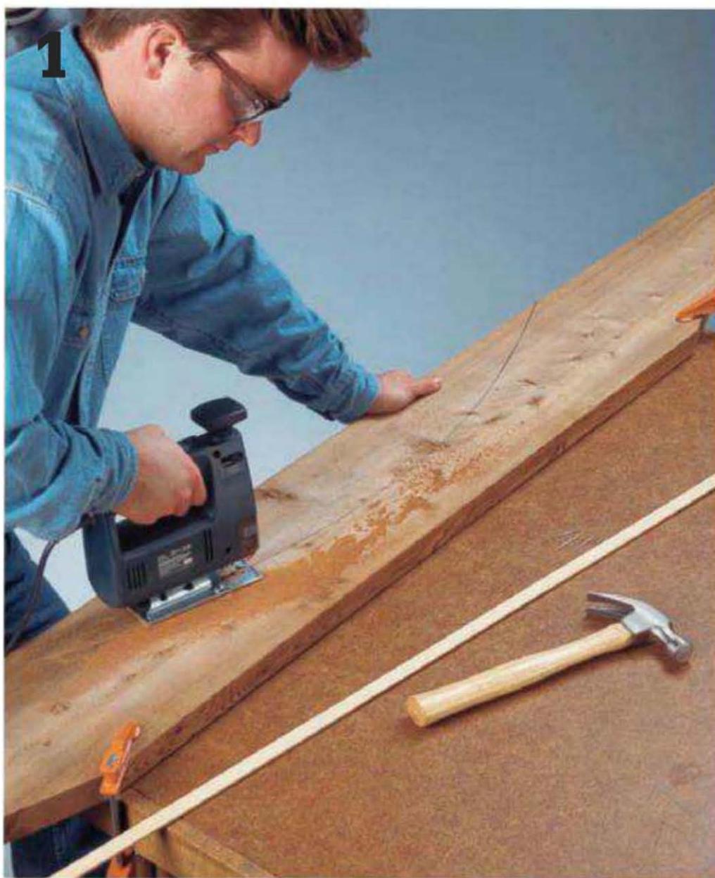
Make the arched cutouts in the bottoms of the 2 x 10 stringers using a jigsaw.
