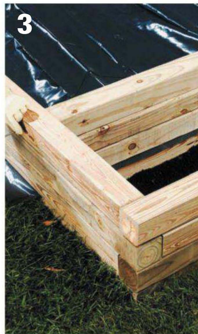
Build the rest of the sandbox frame, staggering the corner joints. Drill holes and drive barn nails through the holes.
