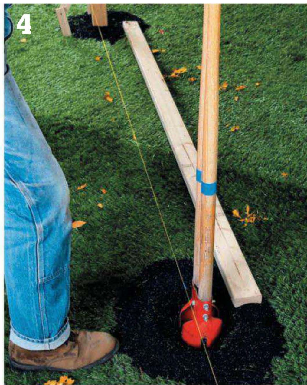
Set, plumb, and brace the first post, then lay a 2 × 4 the same length as the panel width along the fence line as a reference for digging the next posthole.
