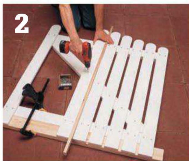
Attach the siding boards. Align the end boards so they are flush with the edges of the frame. Using spacers, attach all siding boards to the frame with deck screws.
