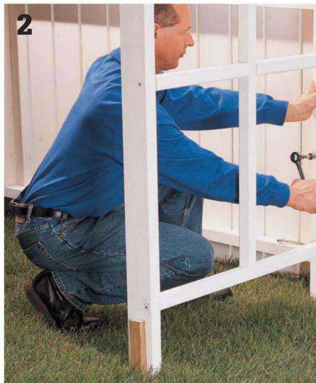
Position the trellis frames , clamping them against the gateposts. Attach the frame to the posts with 3" lag screws.
