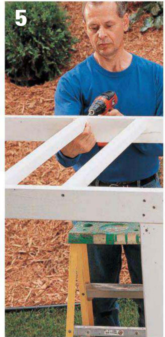
Attach four evenly spaced 2 × 2s between the tie beams for rafters using 2½" deck screws.
