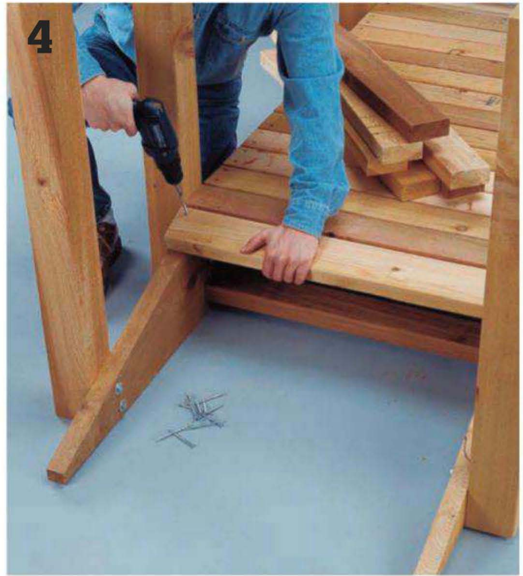
Attach the treads to the stringers with deck screws.
