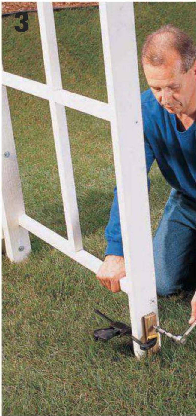
Secure the free end of each frame to stakes using lag screws or deck screws.
