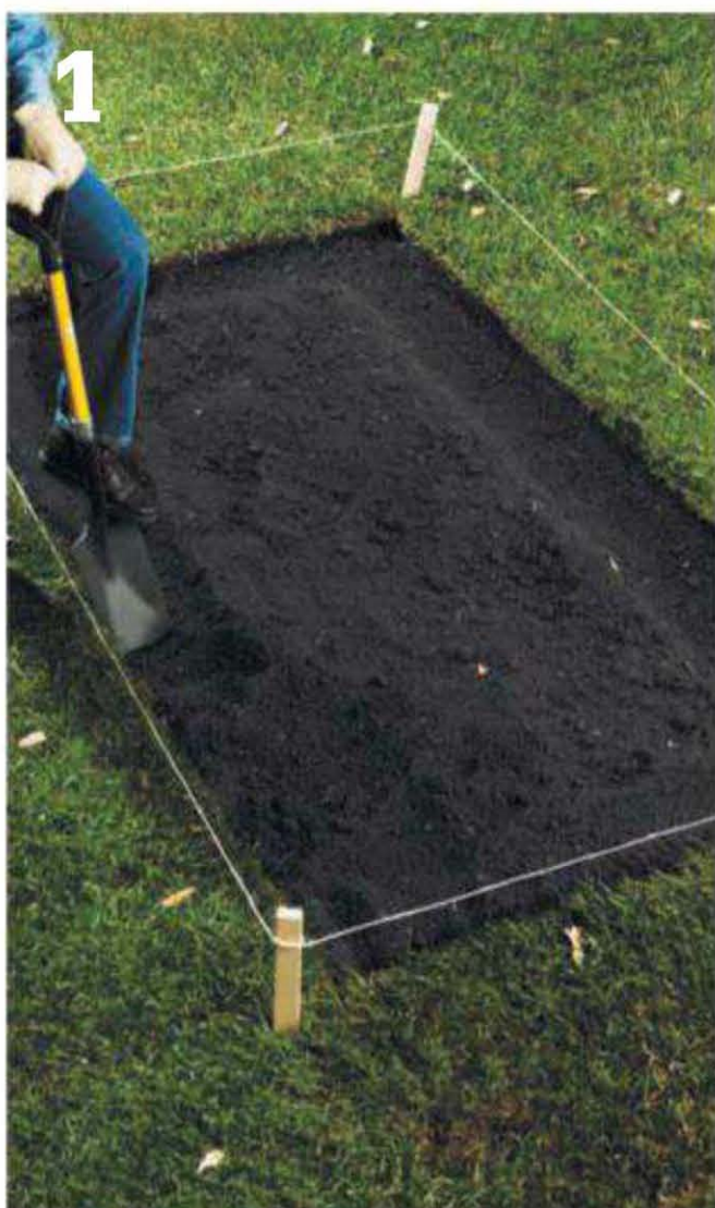
Remove the grass in the sandbox location with a flat-end spade, and then dig a trench for the first row of timbers.
