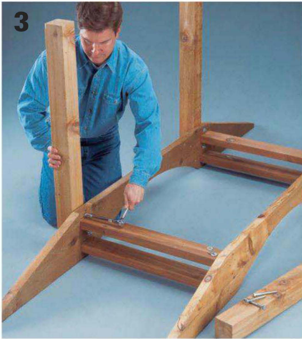
Cut the 4 x 4 posts to their finished height, then use lag screws to attach them to the outsides of the stringers.
