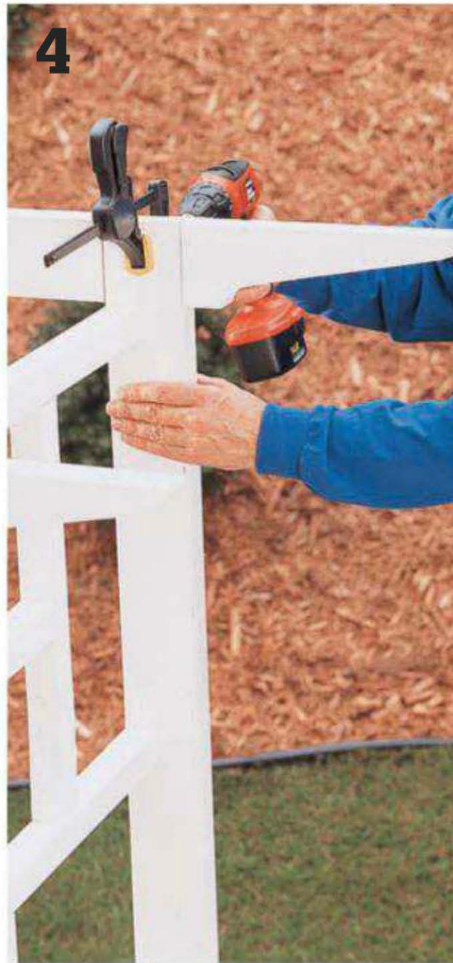
Make the half-lap joints securing the tie beams to the trellis frame post tops and fasten with four 1¼" deck screws at each joint.
