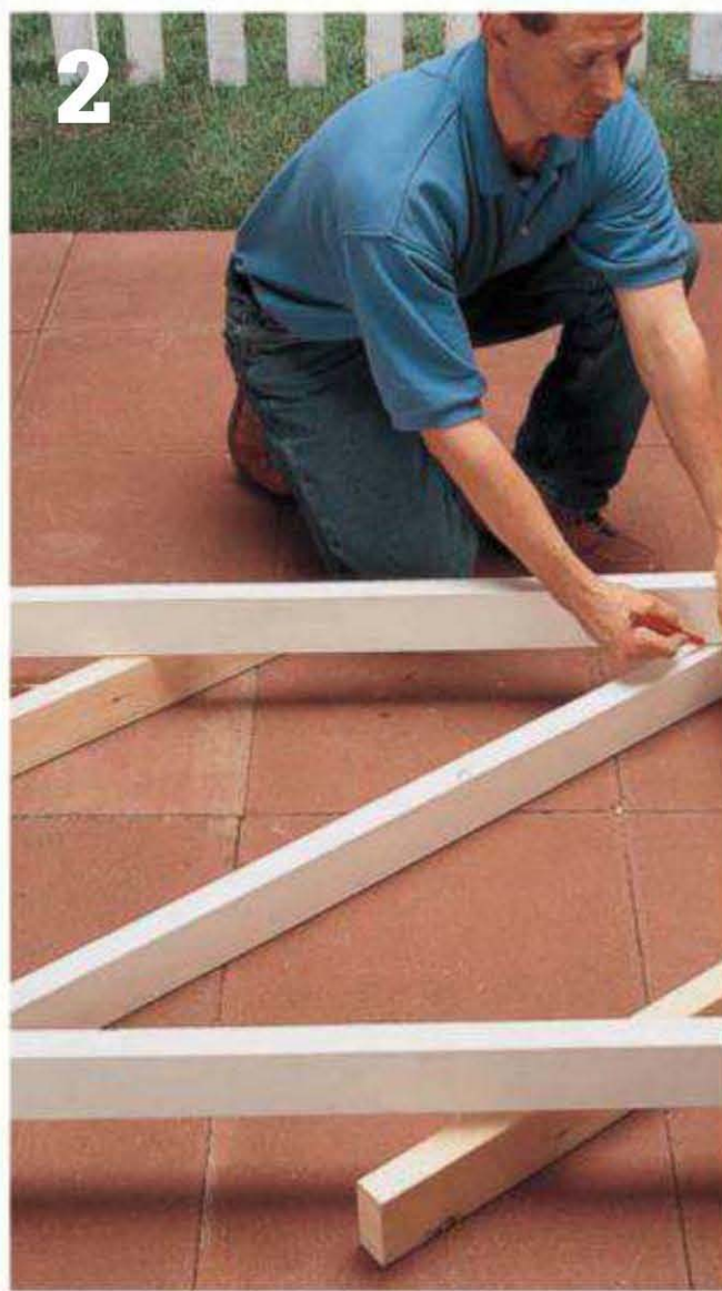
Trace the opposite corners of the frame onto the 2 x 4 diagonal brace to make cutting lines. Cut the brace using a circular saw with the blade adjusted for the appropriate bevel angle.
