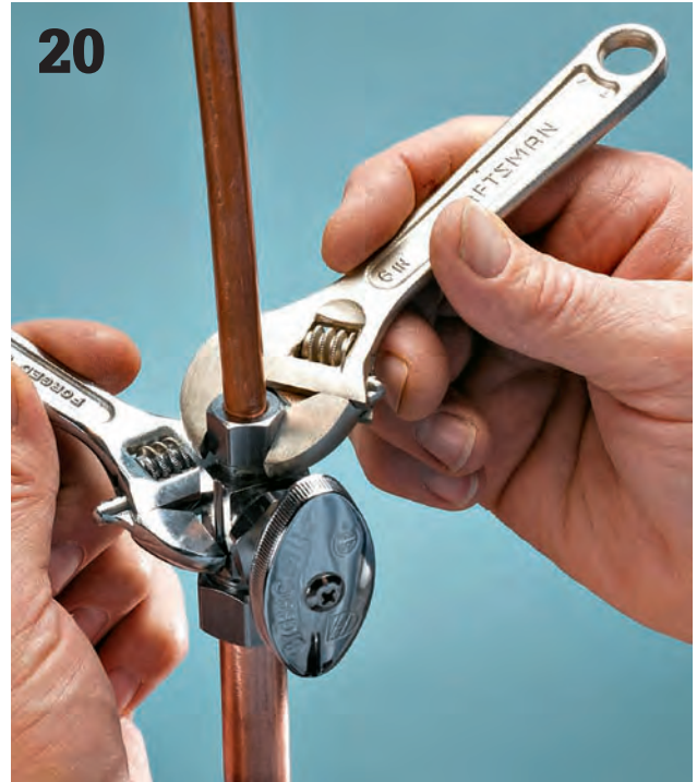
20 Install the spout supply valves and hook them up to the supply risers. Tubs are not predrilled for faucets as sinks are, so you'll need to decide whether to drill holes for the valves in the tub rim using a step bit, or to mount the faucet in the platform or the rim of the support wall.
