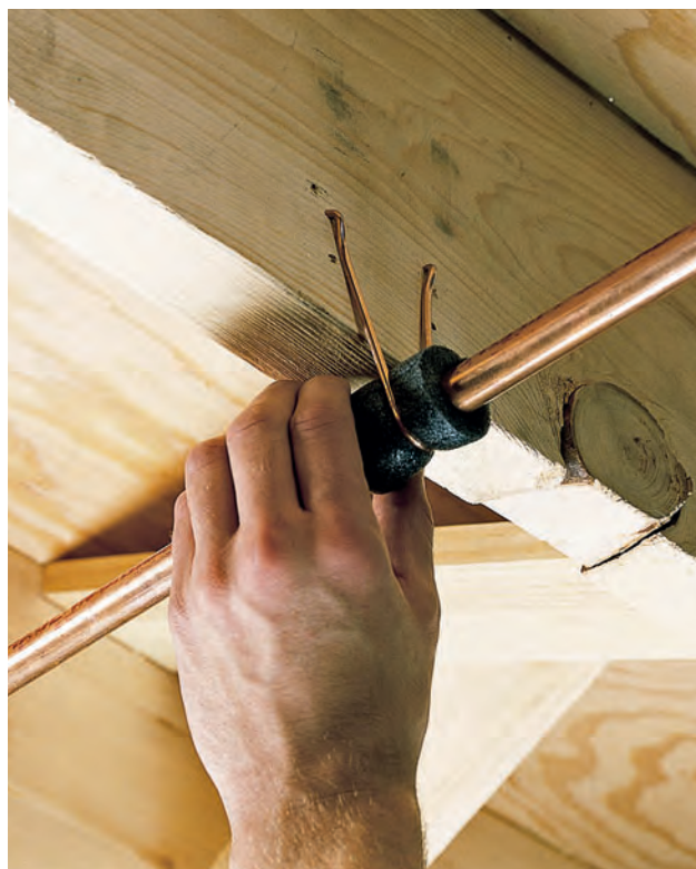
Loose pipes may bang or rub against joist hangers, creating noise. Use pieces of foam rubber pipe insulation to cushion pipes.
