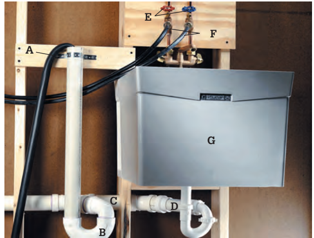
A washing machine with standpipe drain: washing machine drain hose (A), 2" standpipe drain with trap (B), waste line (C), utility sink drain pipe (D), hot and cold supply lines with hose bibs (E), rubber supply hoses to washing machine (F), and utility sink (G).
