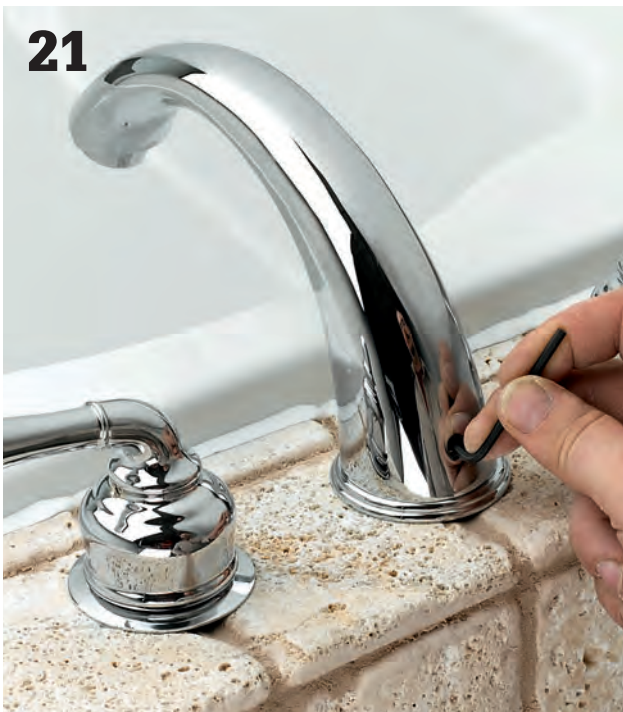
21 Attach the spout and the valve handles and test the supply system. To clear any debris from the lines, remove the spout aerator and run both hot and cold water for a minute or so.
