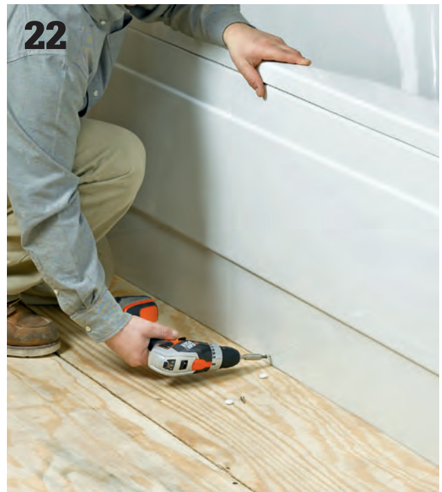
22 Attach the removable front apron or replace the access panel covering. Then, fill the tub and have a nice, long soak.
