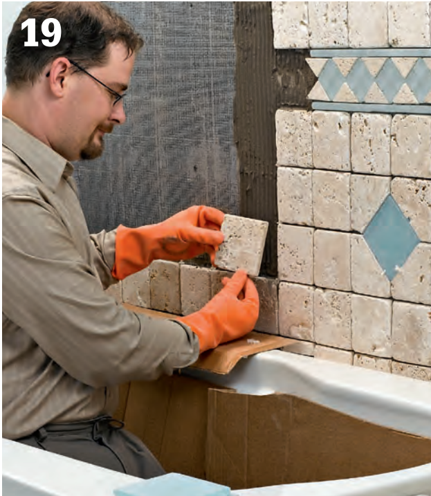
19 Install the wall surface materials , cutting holes for the spout and valves as needed.
