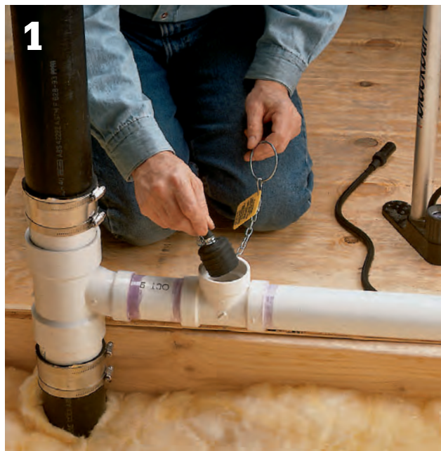
Insert a test balloon into the test T-fittings at the top and bottom of the new DWV line, blocking the pipes entirely. Note: Ordinary T-fittings installed near the bottom of the drain line and near the top of the vent line are generally used for test fittings.
