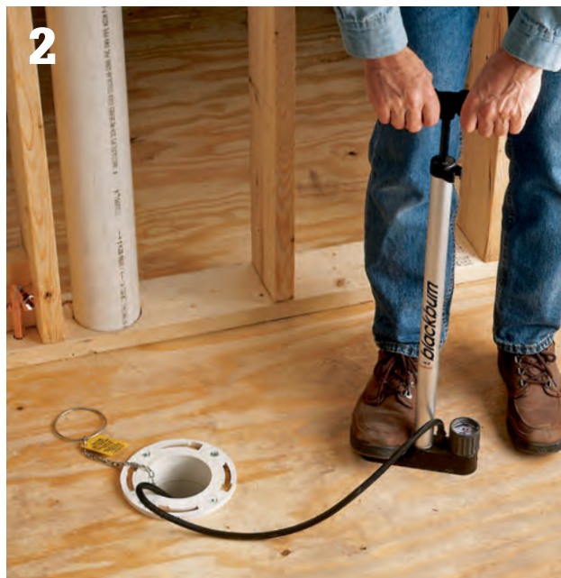
Block toilet drains with a test balloon designed for a closet bend. Large test balloons may have to be inflated with an air pump.
