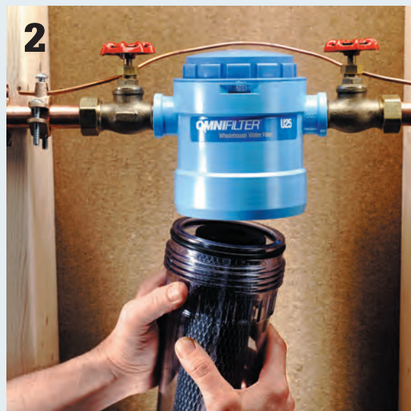
A whole-house water filtration system: (A) intake side, (B) supply pipe from the water meter pipe, (C) outtake side to the house supply pipe, (D) filter, and (E) filtration unit cover.
