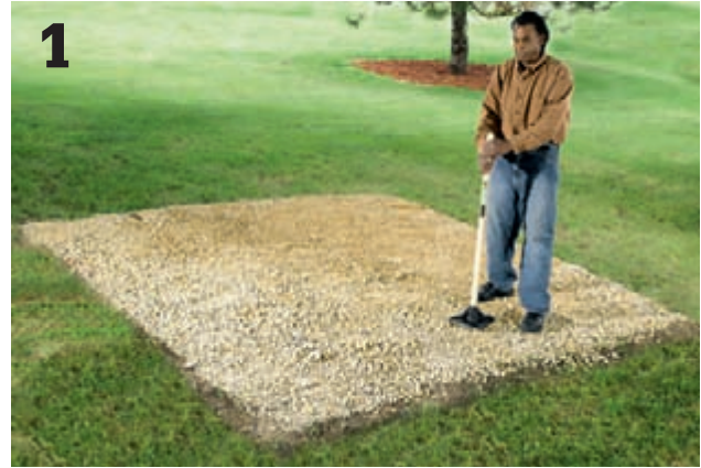
Create a bed of compacted gravel centered at each block location in your layout.
