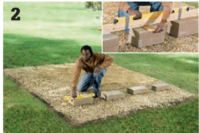
Set a block at the highest point on the site , check it with a level, and adjust as needed. (Inset) Use a level and board spanning across the blocks to establish the height of each stack so all the tops are level.
