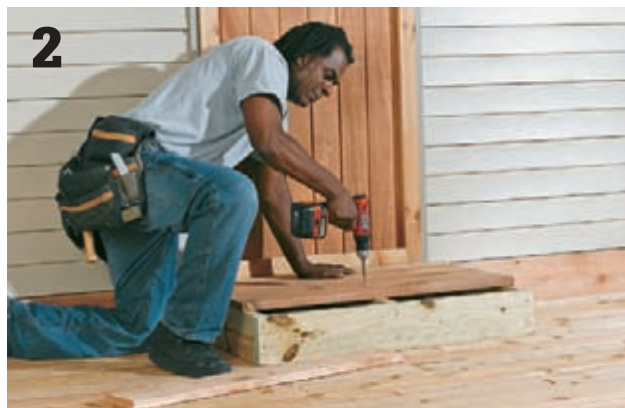
Install the decking with screws , leaving a ¼" gap between boards.
