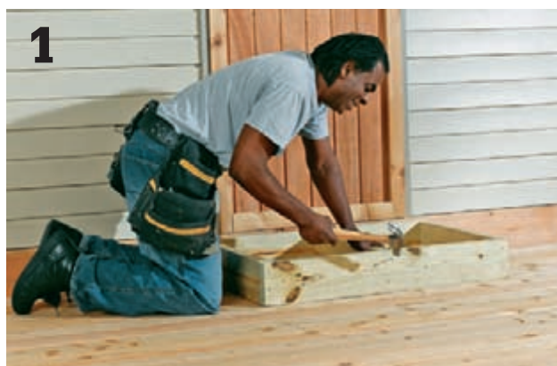
Assemble the frame pieces with pairs of 16d common nails.
