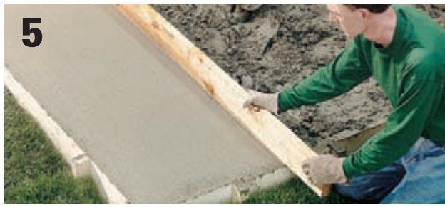
Screed the concrete after filling the form , using two people to screed, while a third fills low spots with a shovel.
