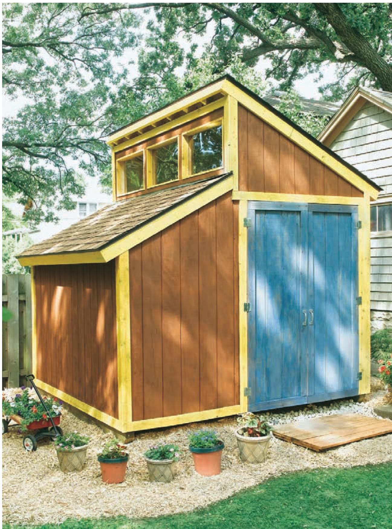
The clerestory windows on this sunlight-filled shed introduce natural light without introducing a security risk.
