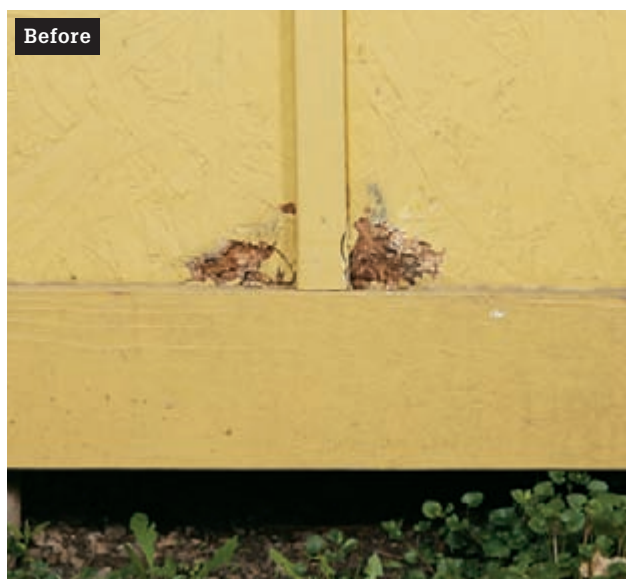
Accumulating rot defaces and devalues your shed; fortunately there's a quick fix.
