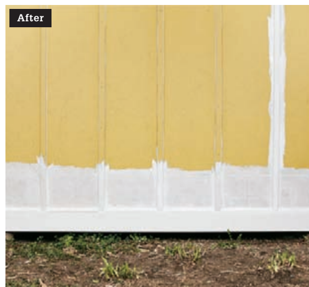
Replacing rotting siding is a common fix for wooden sheds. After painting it will look as good as new.
