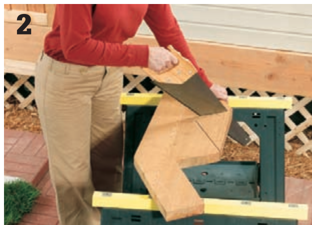
Cut out stringers with a circular saw, and finish the corners of the cuts with a handsaw.
