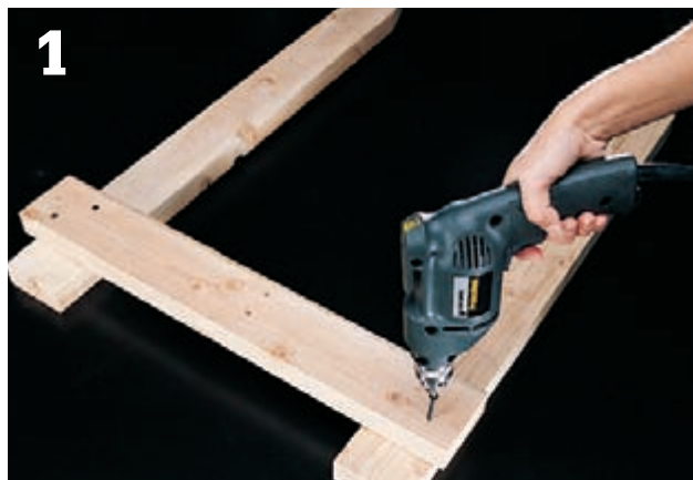
Cut the batter board pieces from 2 × 4 lumber and assemble them with screws.
