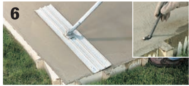
Float the slab with a bull float , then set the J-bolts at the marked locations (inset).
