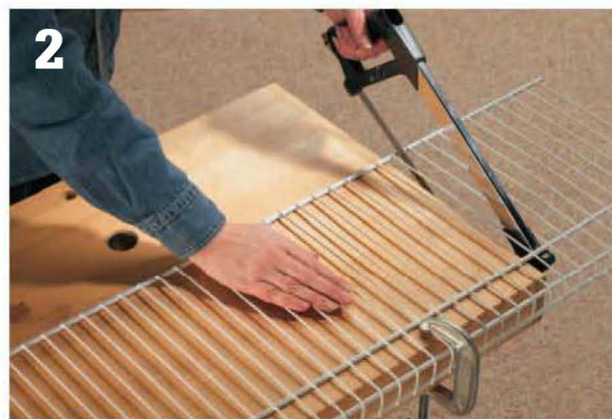
Measure and mark the length of the shelving onto the wire. Cut the wire shelving to length using a hack saw.
