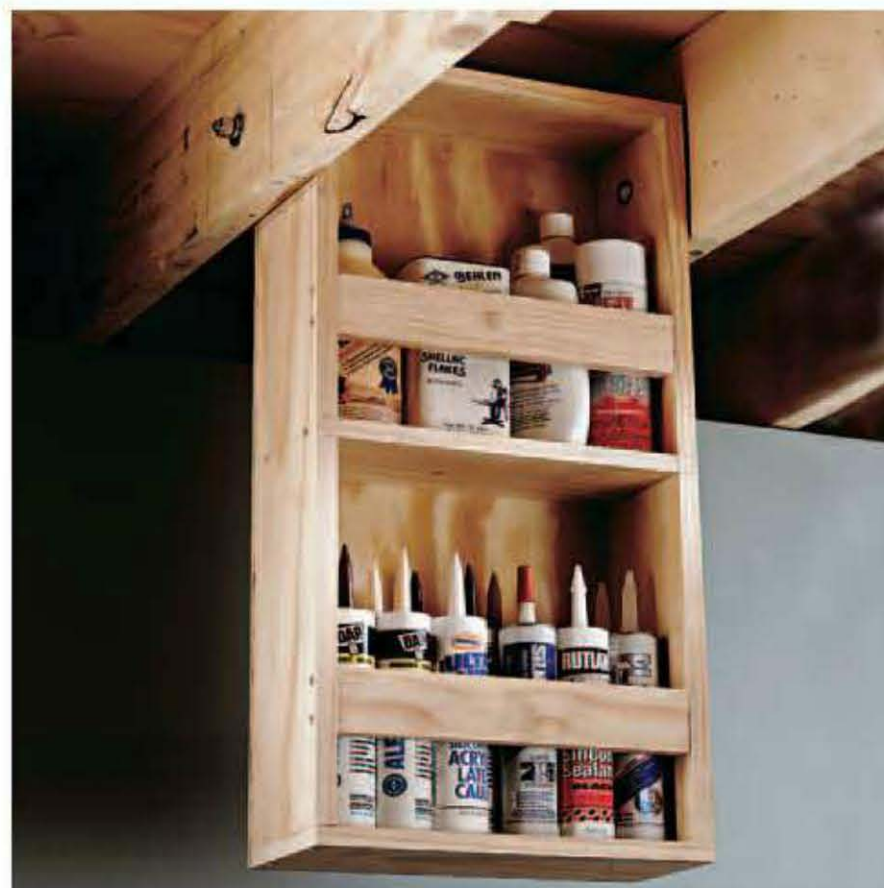
Turn joist cavities into efficient storage cabinets with these inexpensive, easy-to-build folding shelves.
