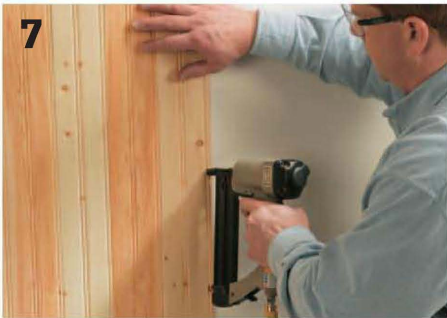
Drive a pneumatic brad through the tongue of one of the far-right boards and into a marked wall stud.
