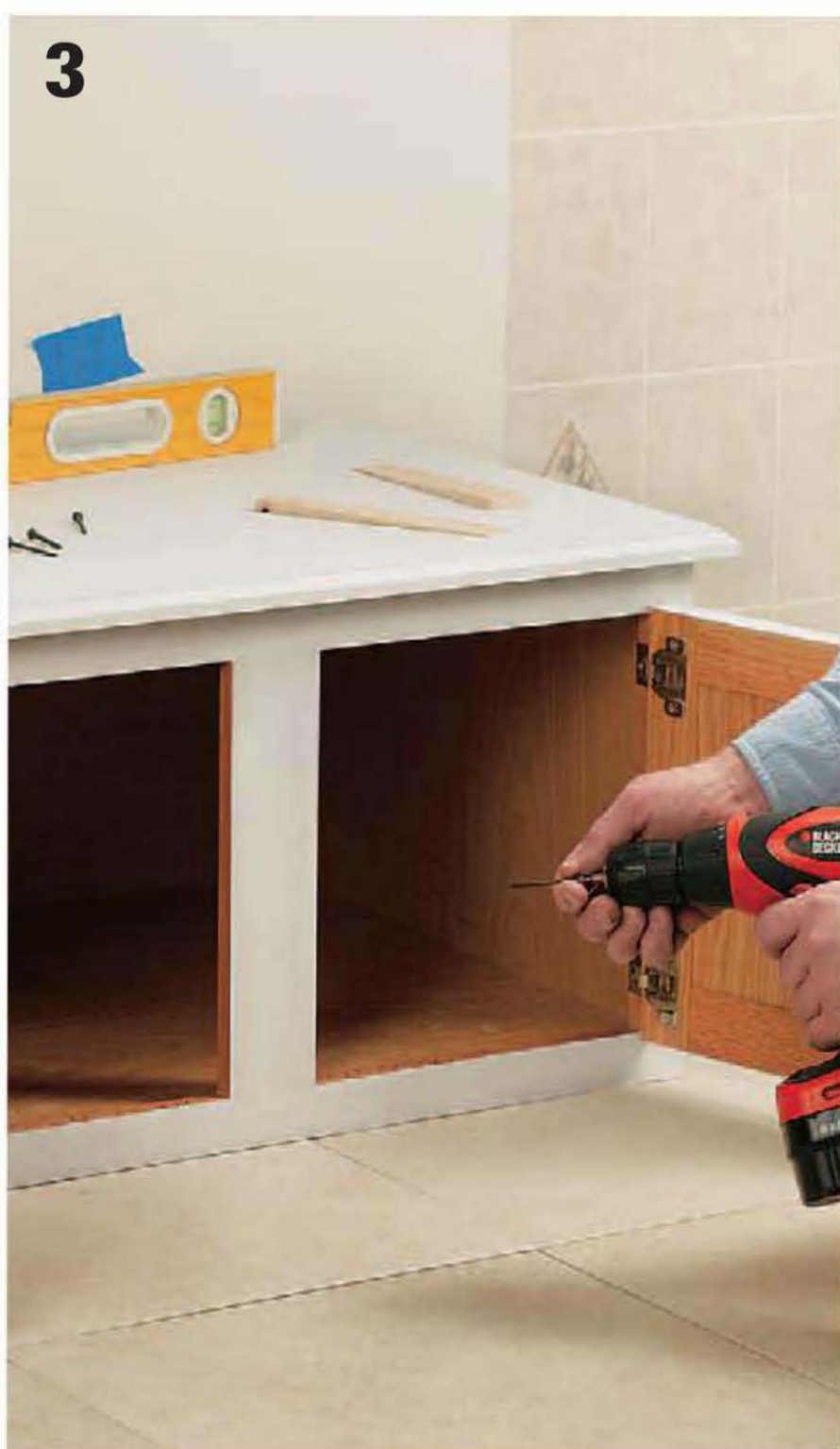
Drive screws through the back of the cabinet at the marked wall stud locations.
