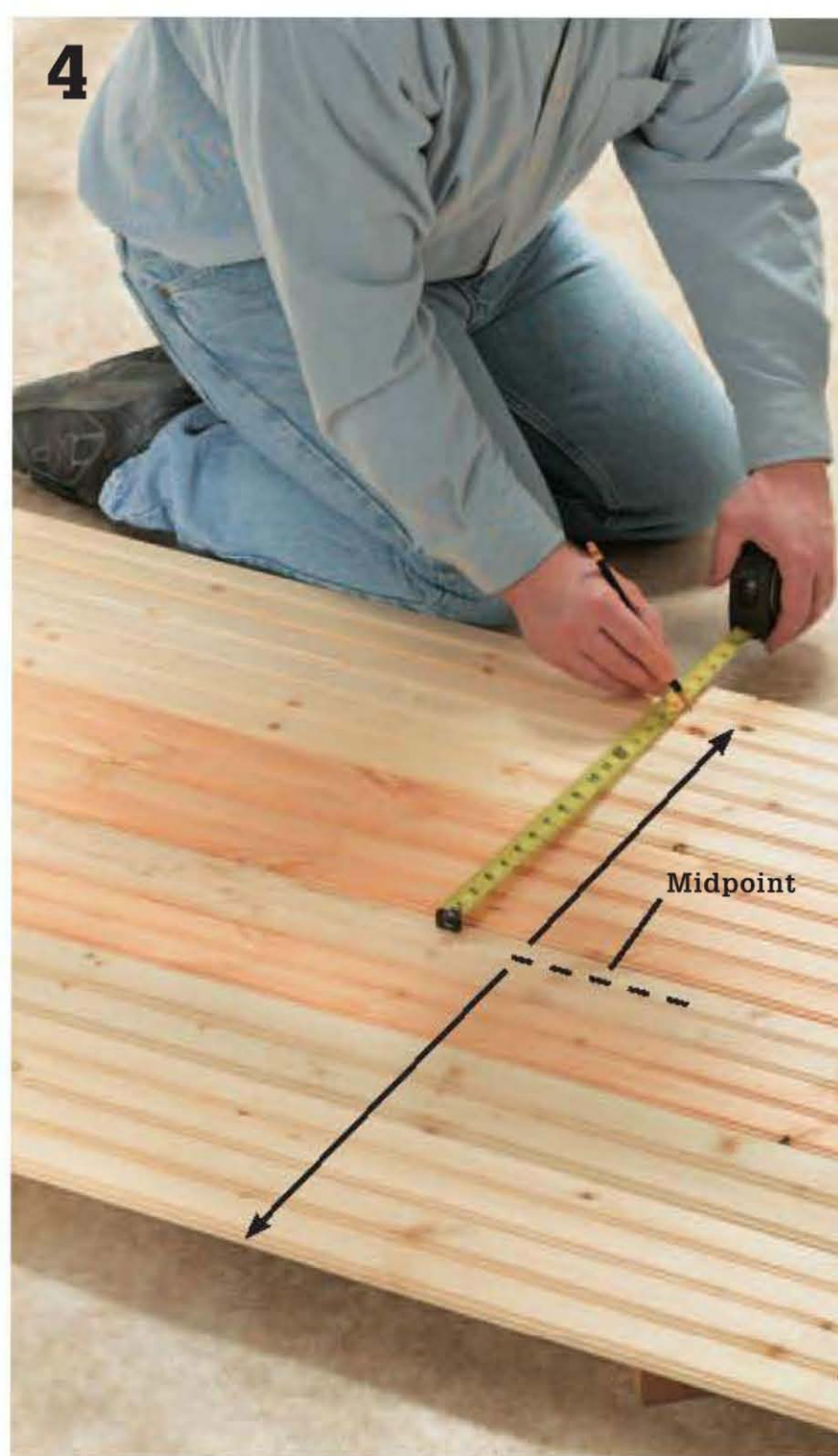
Lay out the tongue-and-groove carsiding boards in a row, with the tongues fitted into grooves. Measure out in one direction (half the width of base cabinets) from a midpoint line in the center board.
