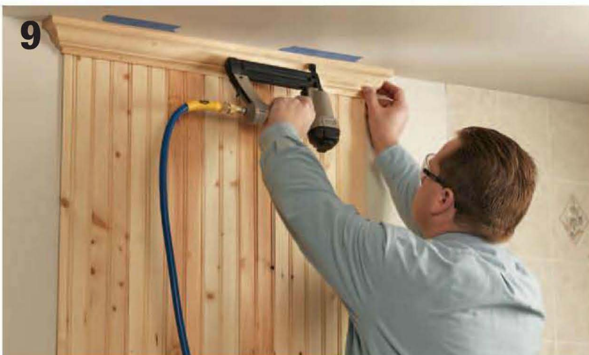
Attach crown molding at the top of the project, creating mitered returns at the ends. Mark the ceiling joists with tape.
