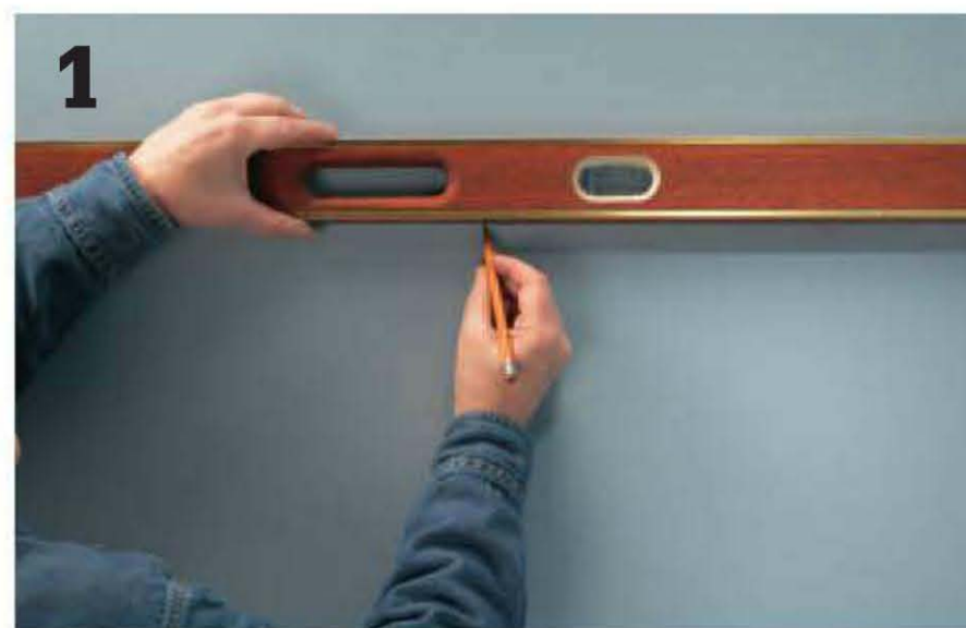
Measure your closet and draw a level line 48" up from the floor.
