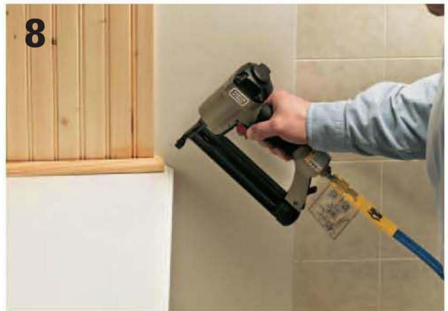
Install quarter-round or base shoe molding at the top edge of the seatboard where it meets the carsiding. Tie the molding back to the wall with mitered returns.
