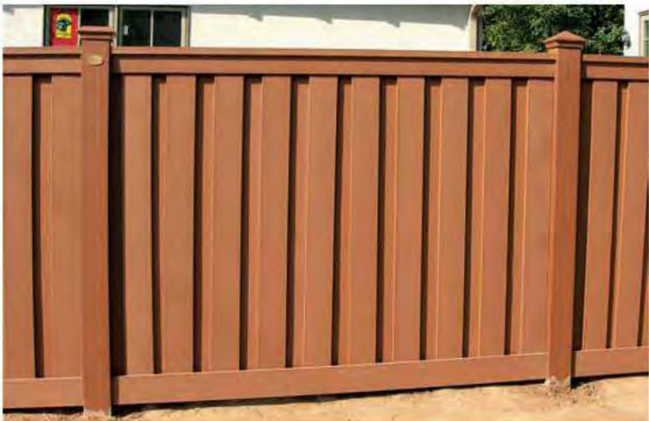
New composite fencing systems offer a broader range of colors and employ installation techniques that are more familiar to DIYers than most vinyl fencing.
