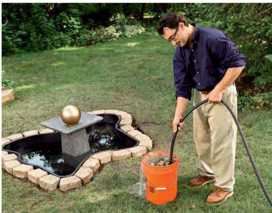
11. Ponds look more natural if you line the bottoms with rock. Small-diameter (2 to 3") river rock is a good choice. Before putting it into the pond, rinse the rock well. One trick is to put the nozzle of a hose in the bottom of a clean 5-gallon bucket and then fill the bucket with dirty rock. Turn on the hose and let the water run for 15 minutes or so. This will cause impurities to float up and out of the bucket.
