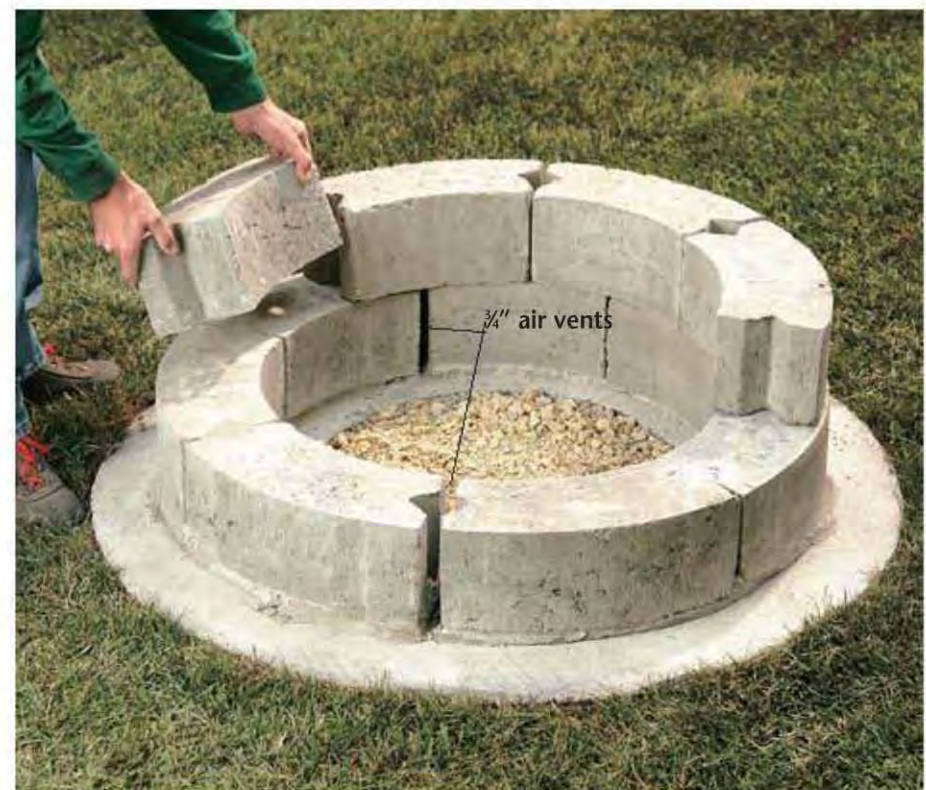
D. Dry-lay the second course of block \frac{3}{8} " from the outside edge of the first course. Fill any block hollows with mortar.
