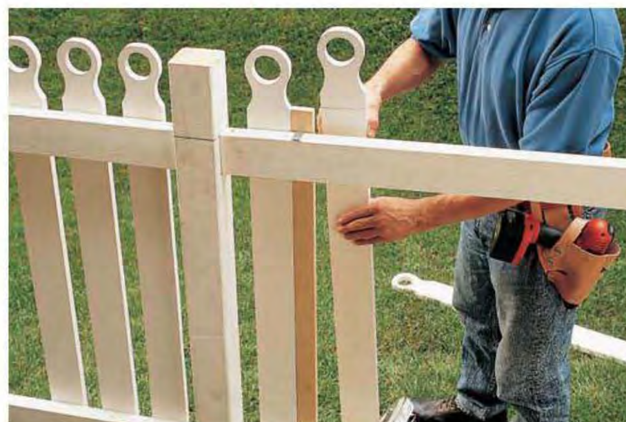
D. Calculate the picket spacing and make a spacing jig. Position the first picket and secure it with 1½" galvanized deck screws. Using the spacing jig, position and install the remaining pickets.
