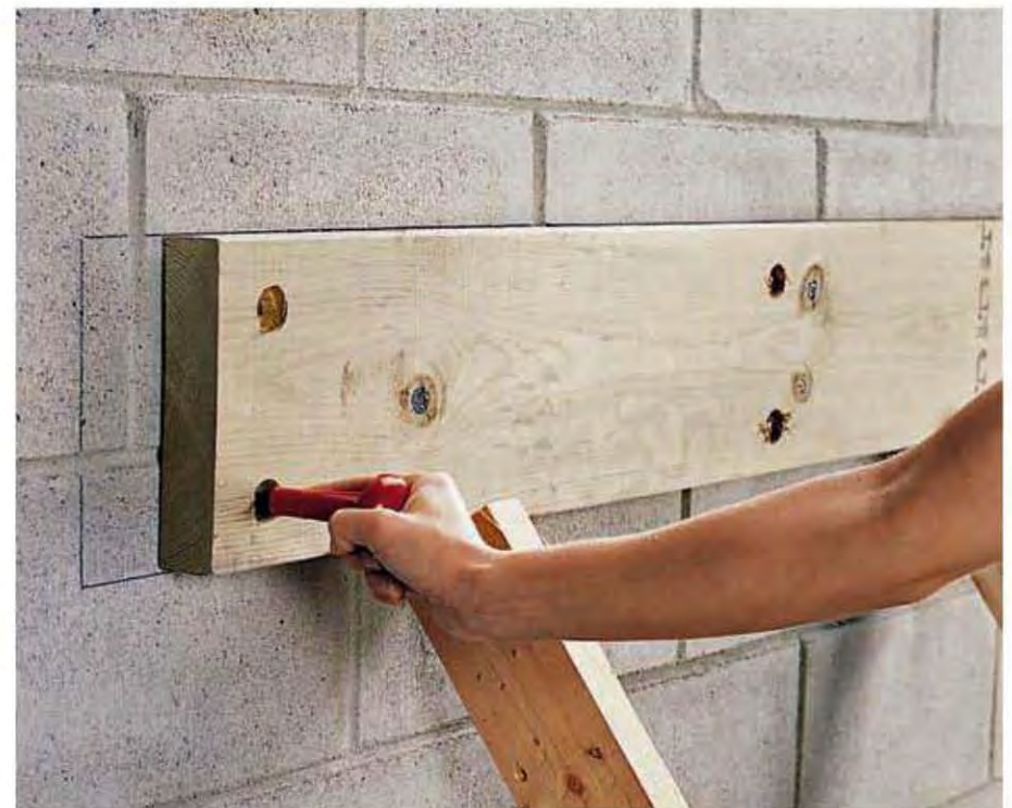
2. Draw an outline of the deck on the wall, using a level as a guide. Center ledger in outline on wall, and brace in position. Mark the pilot hole locations on wall using an awl or nail. Remove ledger.
