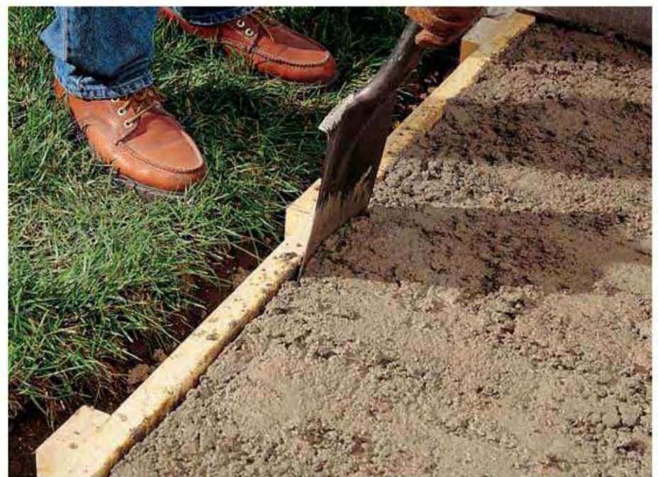
7. After pouring all of the concrete, run a spade along the inside edges of the form, then rap the outside edges of the forms with a hammer to help settle the concrete.
