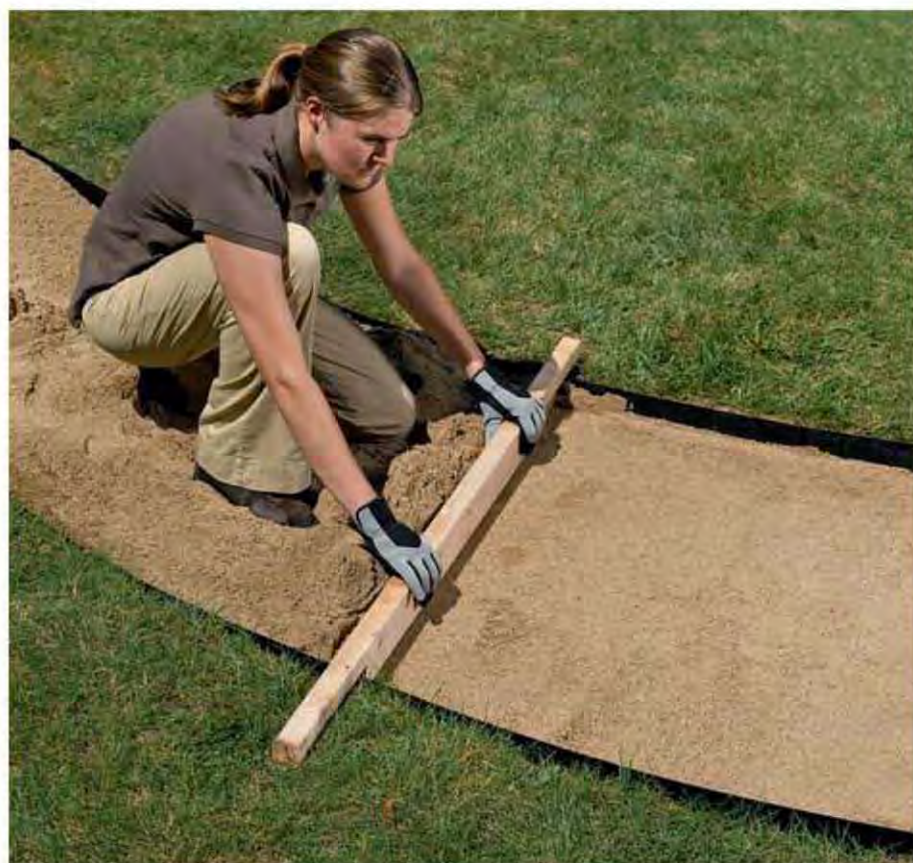
1. Excavate the pathway site and prepare a foundation (as shown on pages 32 to 33). Substitute coarse building sand for compactable gravel. Strike the sand to a consistent depth with a notched 2 × 4.
