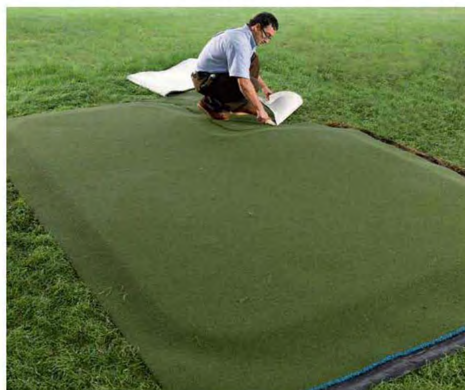
12. Unroll the artificial turf on top of the panels. Pay attention to the nap of the turf to make sure it all runs in the same direction. Use a utility knife to cut it to size, 4" larger than the panel assembly.
