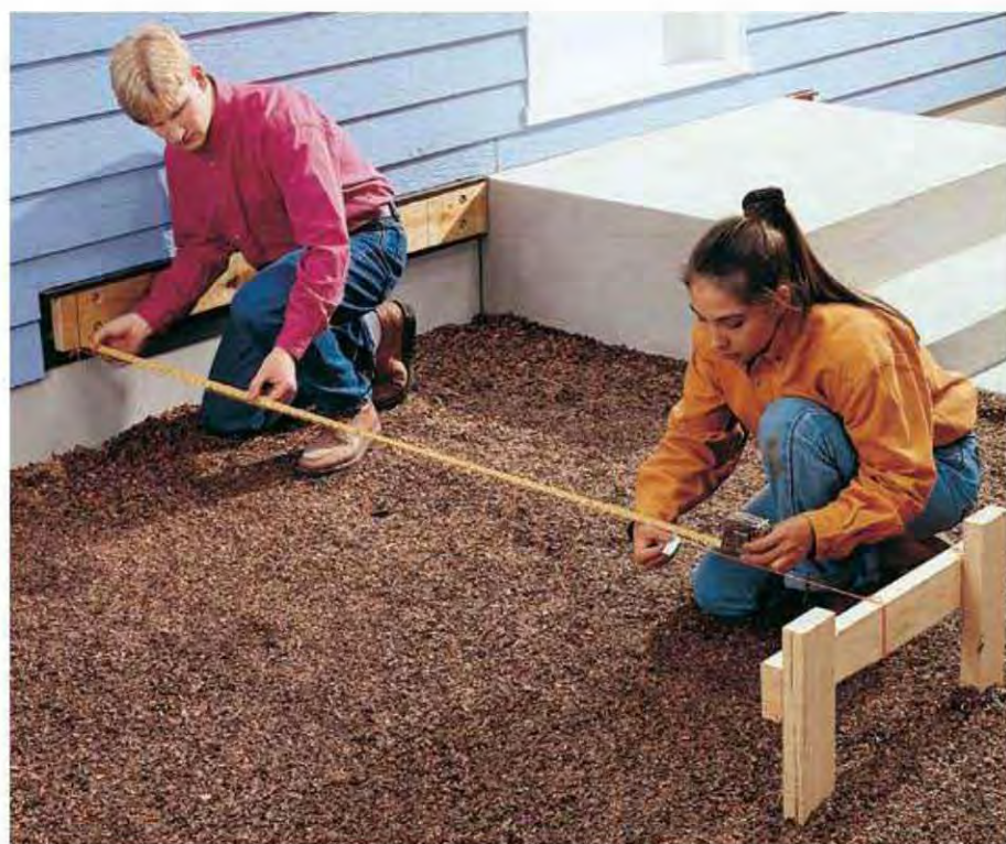
A. Install a ledger to anchor the porch deck to the house, then use it as reference to lay out the footings and posts (pages 316 to 319). If building over old steps, attach a step ledger to the riser of the top step (page 321).
