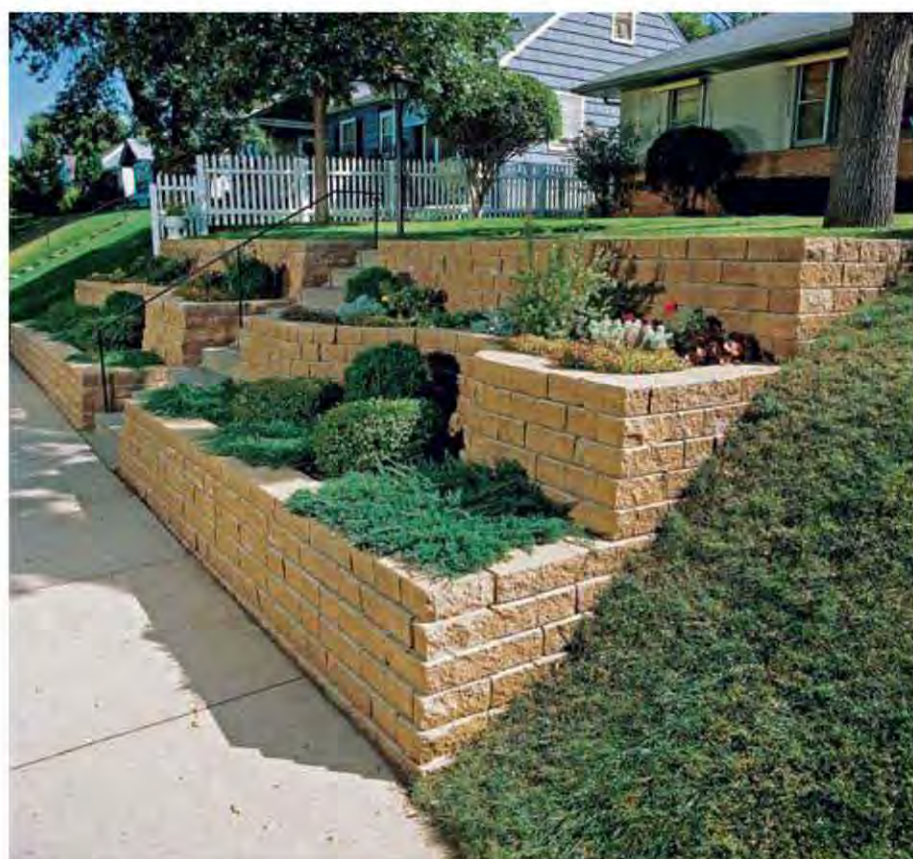
Interlocking block retaining walls are manufactured with the DIYer in mind. They are available as prefabricated designs to eliminate cuts and they come in natural stone looks.
