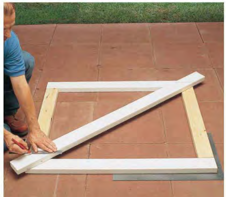
B. Place a 2 × 4 diagonally across the temporary frame, from the lower corner of the hinge side to the upper corner of the latch side, and mark the cutting lines.
