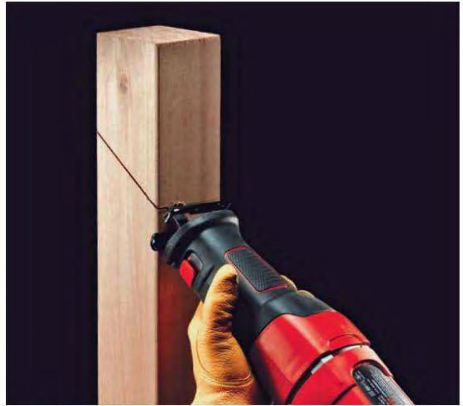
19. Cut off lower stairway post along diagonal cutoff line using a reciprocating saw or circular saw.
