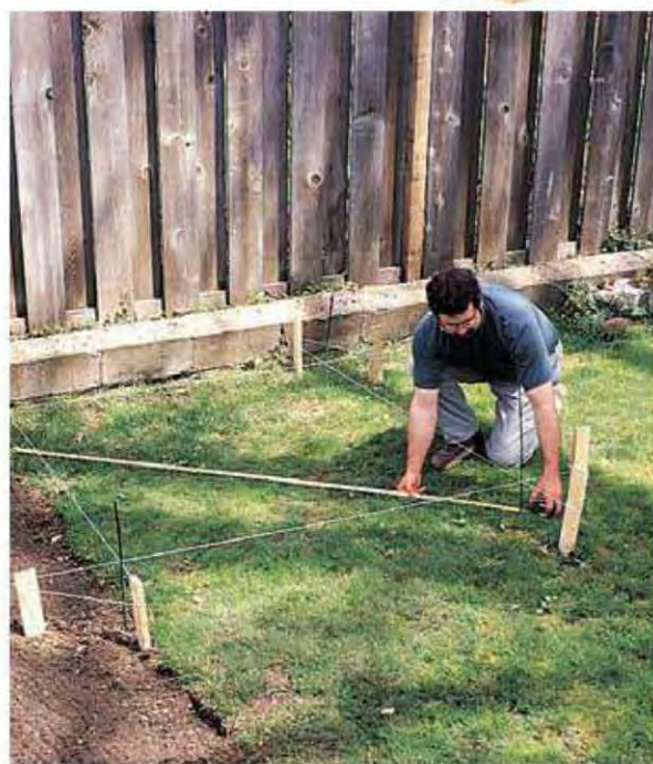
A. Lay out the location of the arbor posts, then measure the diagonals to check for square.
