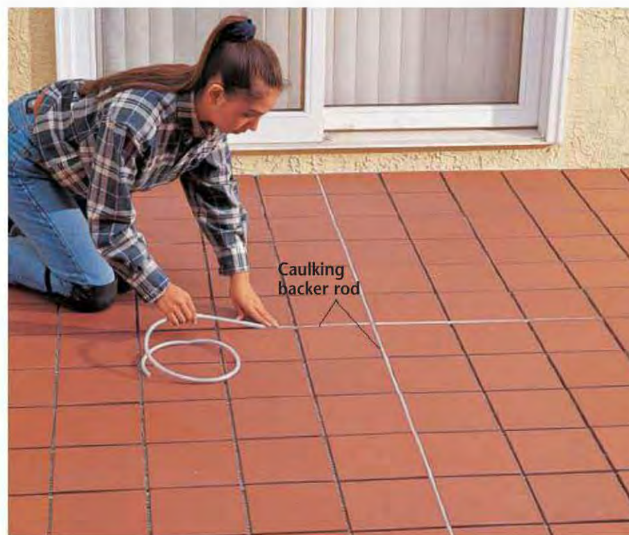
J. After three days, remove plastic sheeting and insert strips of caulking backer rod into the joints between quadrants and control joints.
