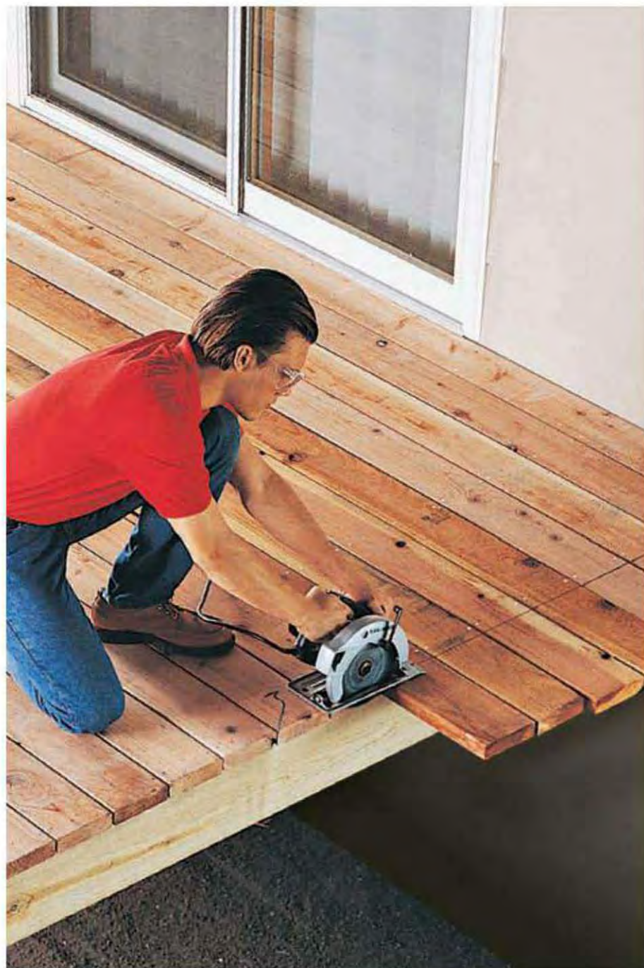
Snap a chalk line flush with the outside edge of the deck, and cut off overhanging deck boards with a circular saw.
