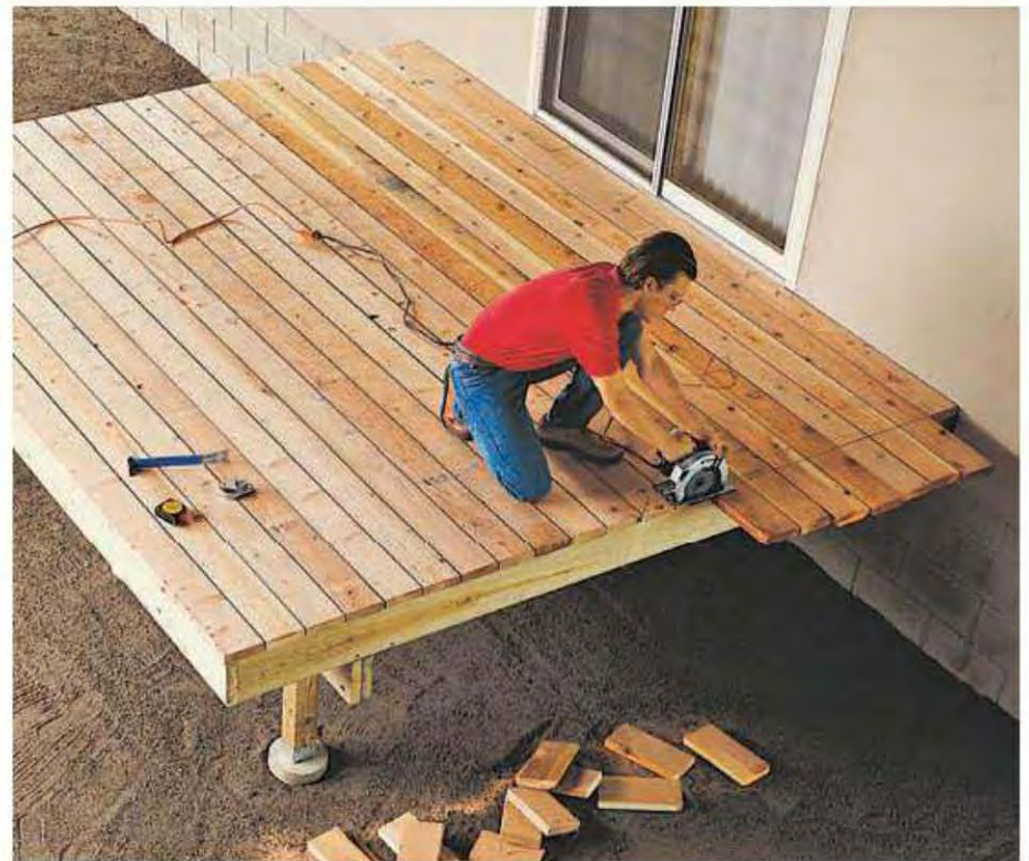
5. Lay decking boards, and trim them with a circular saw. If desired for appearance, cover pressure-treated header and outside joists with redwood or cedar facing boards (page 210).
