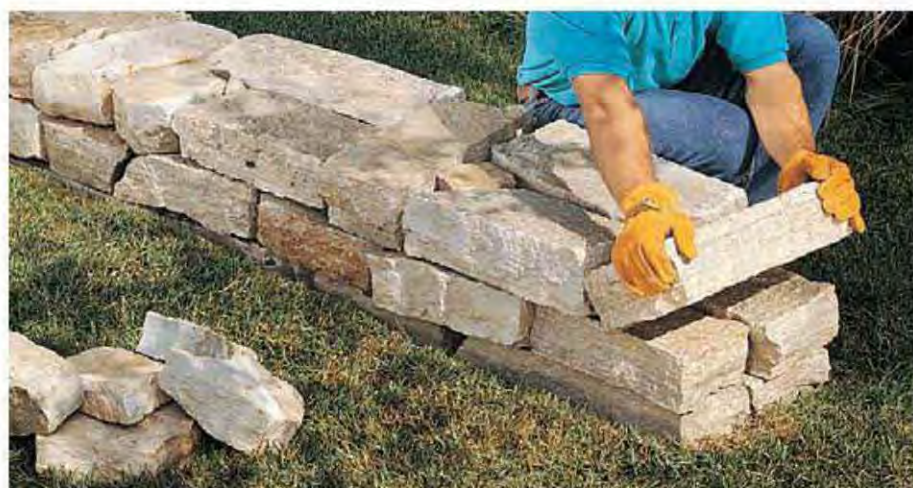
D. Add the third course of stone over the second using tie stones every 36", checking periodically with a level.
