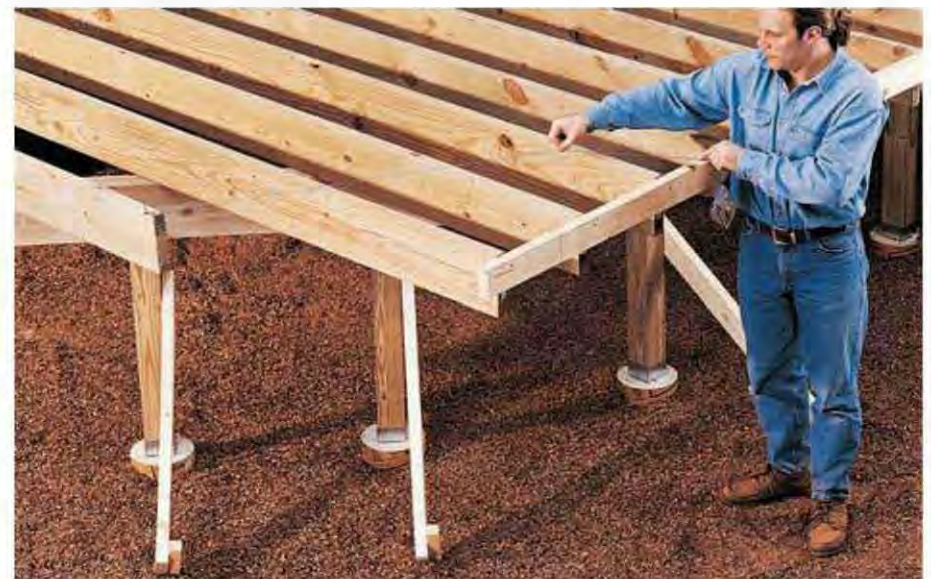
Mark the three remaining inside joists for cutting by snapping a chalk line. Brace and miter-cut the three inside joists.
