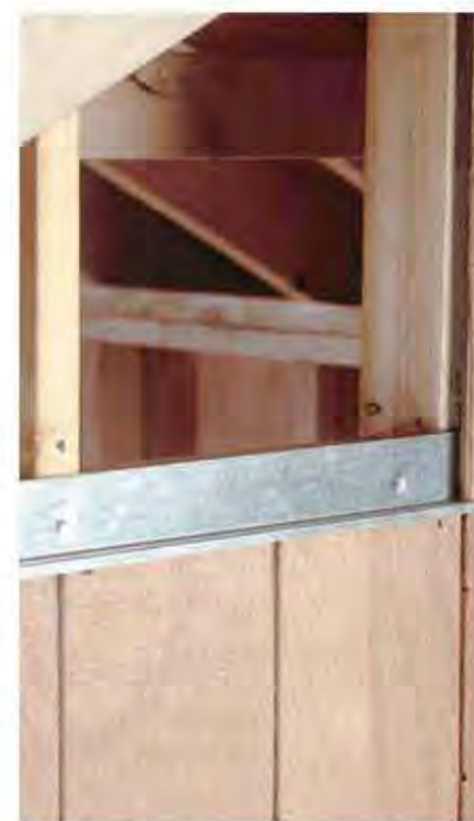
B. Add galvanized metal flashing between rows of siding to prevent water from entering the seam.
