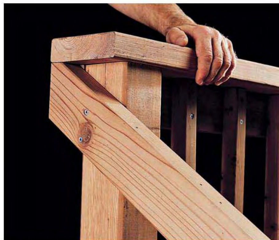
27. At top of stairs, cut cap so that it is flush with stairway rail. Drill \frac{1}{8} " pilot holes and attach cap with 2½" deck screws.
