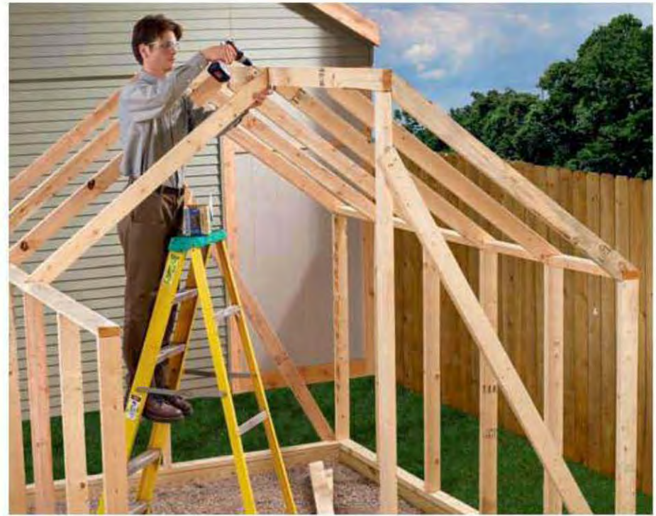
9. Attach the rafters to the ridge pole and the kneewalls with deck screws driven through pilot holes. Try to make the rafters align with the kneewall studs.
