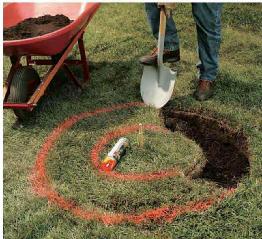
A. Outline the location of the footing using spray paint and a piece of string. Then dig a circular trench 10" deep.
