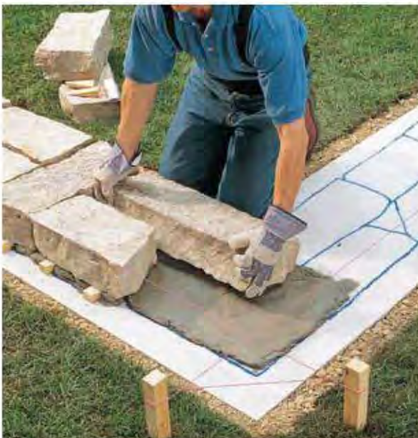
B. Apply mortar to the footing and set the stones in position, according to the layout. If necessary, use wood shims to keep the stones in position.
