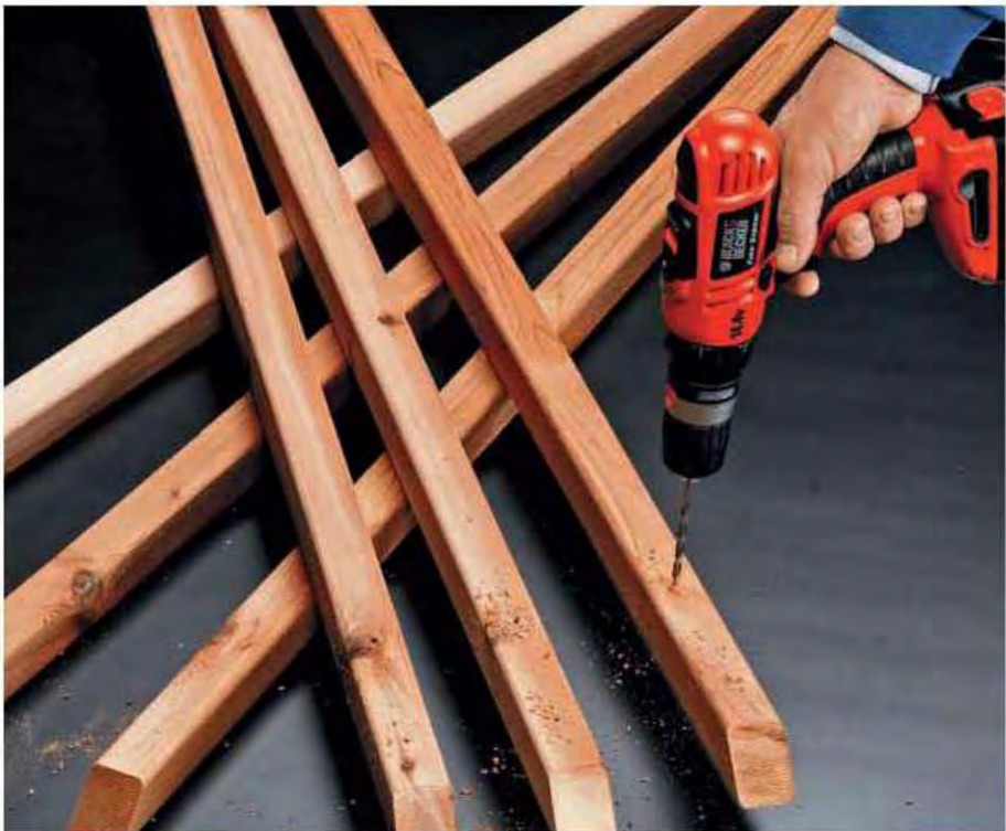
4. Drill two ⅛" pilot holes spaced 4" apart near bottom end of each baluster. Drill two ⅛" pilot holes at top of each baluster, spaced 1½" apart.
