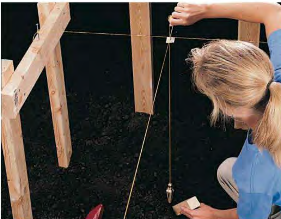
C. Use a plumb bob to mark the pier locations. Drive a stake into the ground directly below the plumb bob pointer.
