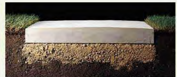
Walkways should crown in the center to provide water runoff.
