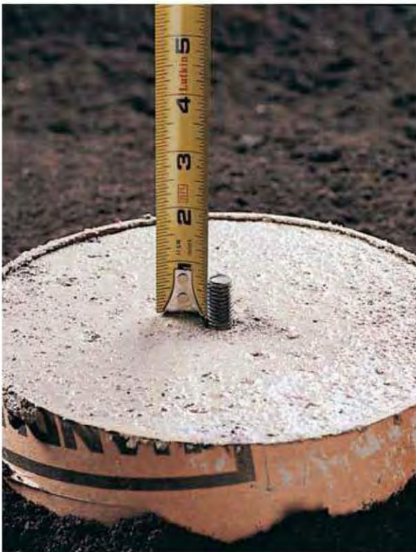
13. Set the J-bolt so \frac{3}{4} " to 1" is exposed above concrete. Brush away any wet concrete on bolt threads with an old toothbrush.
