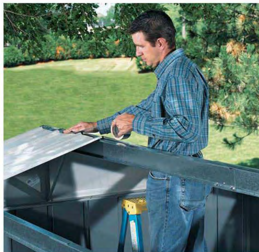
17. Apply weatherstripping tape to the top ends of the roof panels to seal the joints before you attach the overlapping roof panels. If your kit does not include weatherstripping tape, look for adhesive-backed foam tape in the weatherstripping products section of your local building center.
