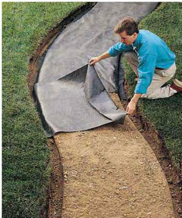
B. Place strips of landscape fabric over the path and into the edging trenches, overlapping sections by 6".
