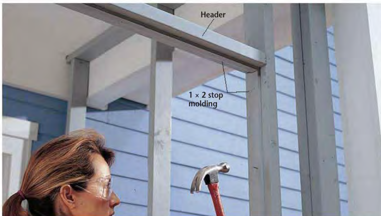
F. Install the door header \frac{3}{4} " higher than the actual height of the door. Attach 1 × 2 stop molding along the inside face of the doorframe so it creates a recess the same thickness as the door.
