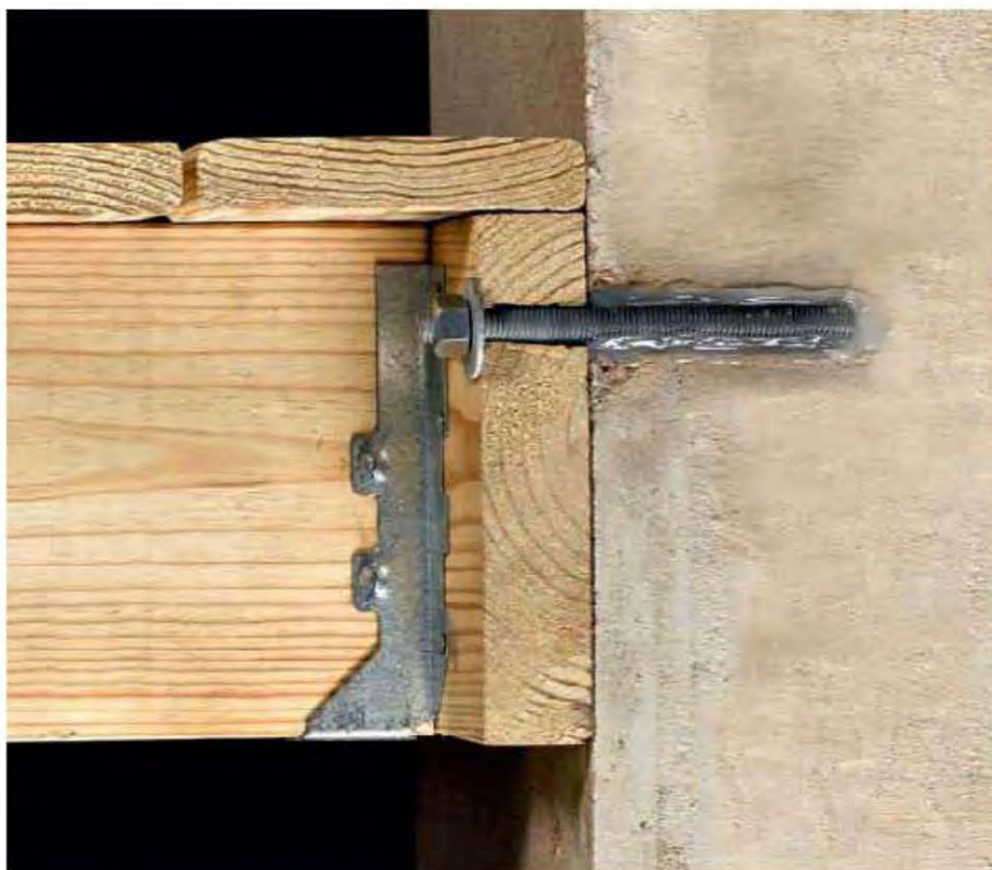
A bolt driven through the foundation from the inside can be fitted with a washer and bolt to secure the ledger.
