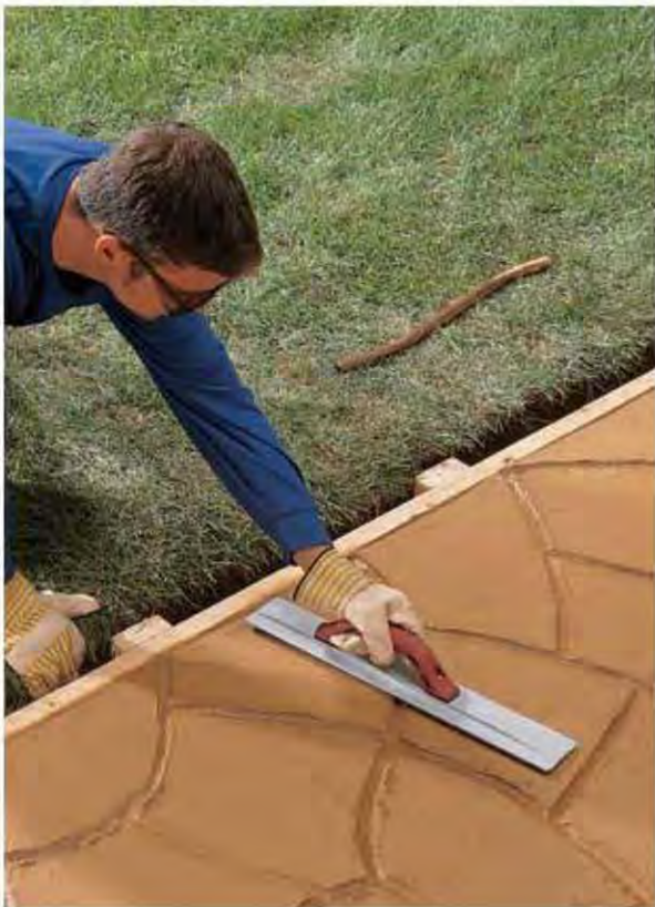
C. Refloat the surface, and remove the forms once the concrete has cured. Protect the surface with a clear concrete sealer.
