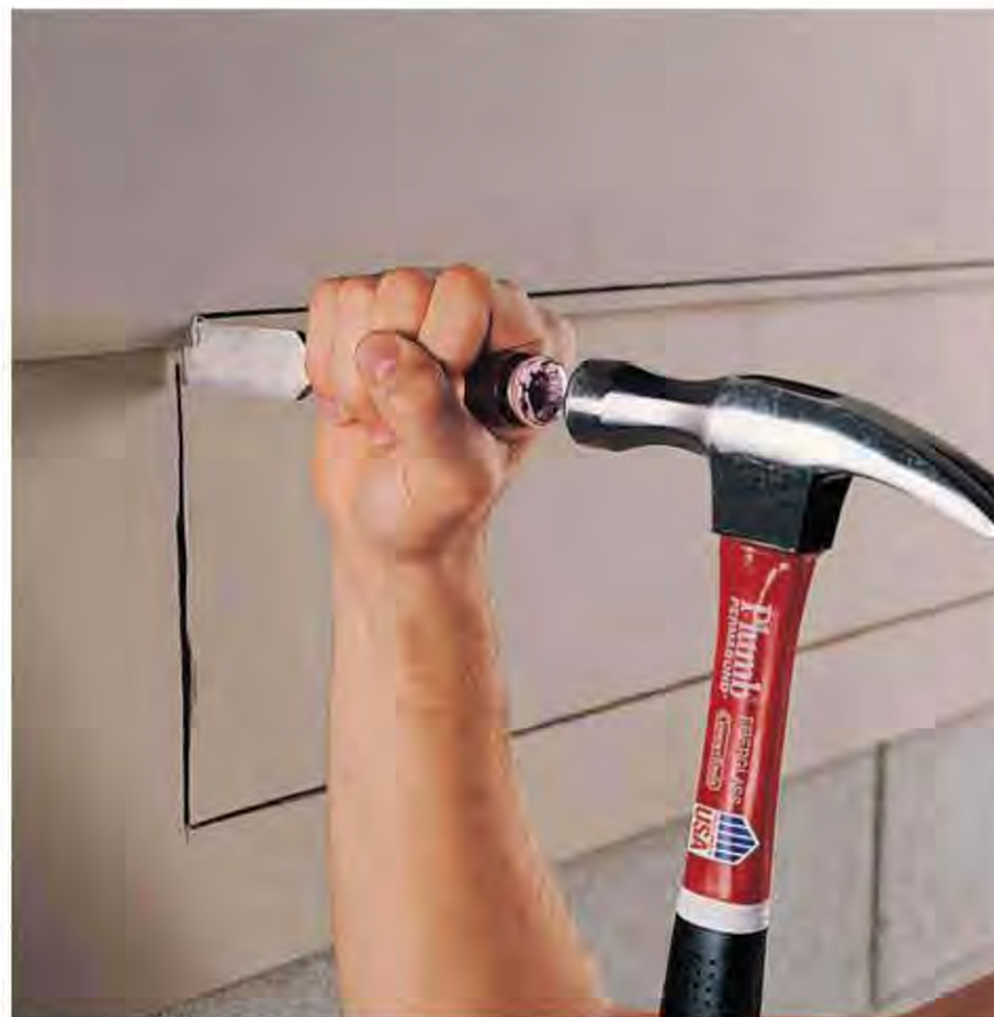
A. After outlining the position of the ledger and cutting the siding with a circular saw, use a chisel to finish the corners of the cutout.
