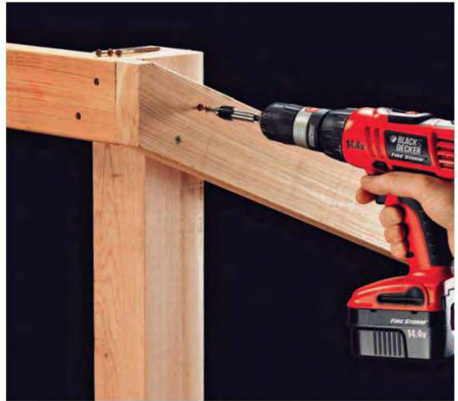
21. Position the stairway rail flush against top edge of posts. Drill \frac{1}{8} " pilot holes, then attach rail to posts with 2\frac{1}{2} " deck screws.
