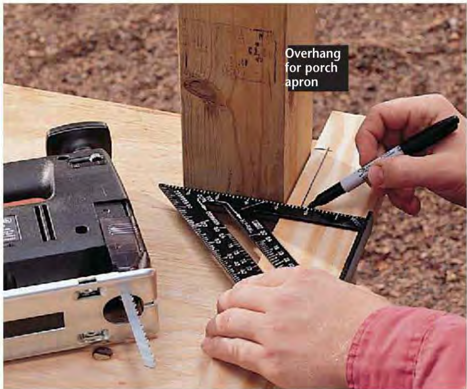
B. Mark the location of the post on the starter board, then notch-out with a jigsaw.
