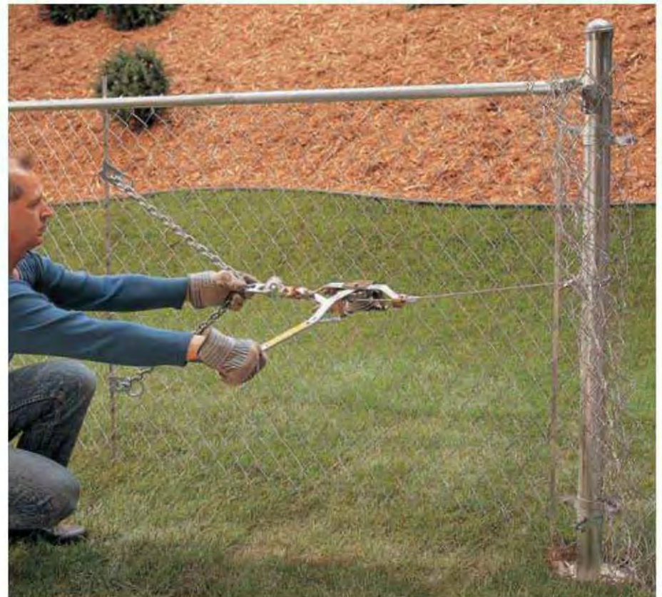
8. Use a come-along to stretch the mesh taut against the fence. The mesh is tight enough when the links are difficult to squeeze together by hand.
