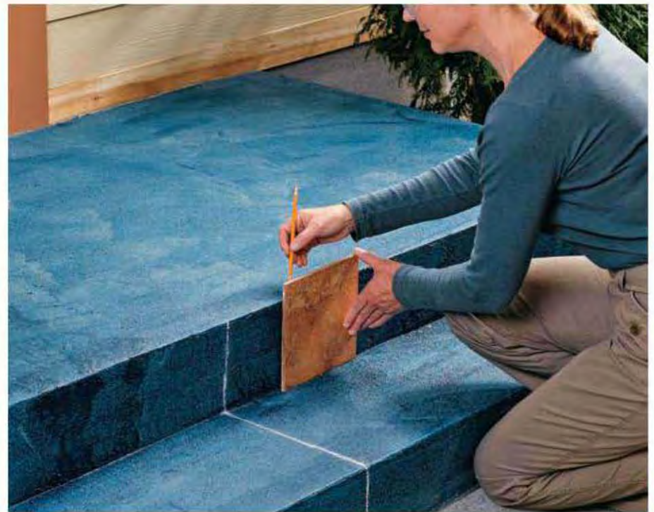
12. Install the tiles on the stair risers. Because the location of the tops of the riser tiles affects the positioning of the tread and landing tiles, you'll get the most accurate layout if the riser tiles are laid first. Start by stacking tiles vertically against the riser. (In some cases, you'll only need one tile to reach from tread to tread.) Add spacers. Trace the location of the tread across the back of the top tile to mark it for cutting.
