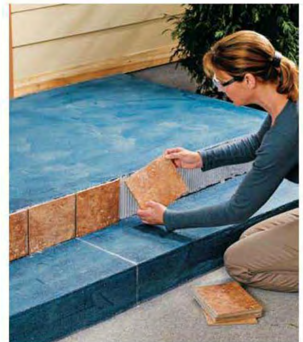
15. Lay tiles on the risers. The bottom tile edges can rest on the tread, and the tops of the top tiles should be flush with or slightly lower than the plane of the tread above.
