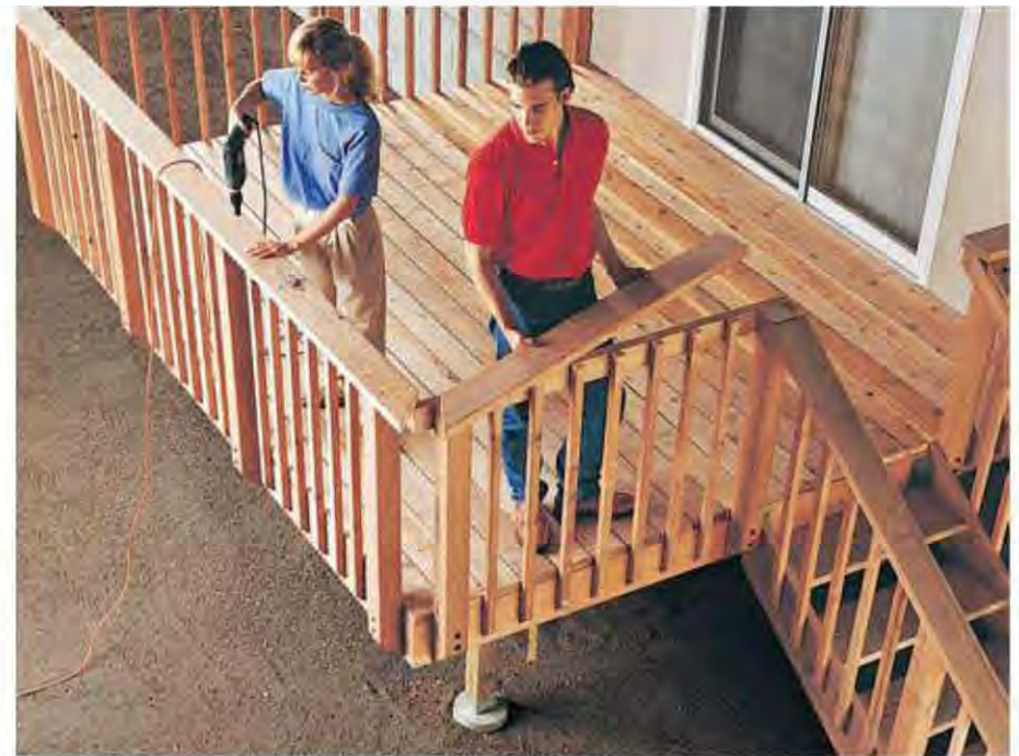
1. Position the rail cap over the posts and balusters. Make sure mitered corners are tight, and attach with deck screws.
