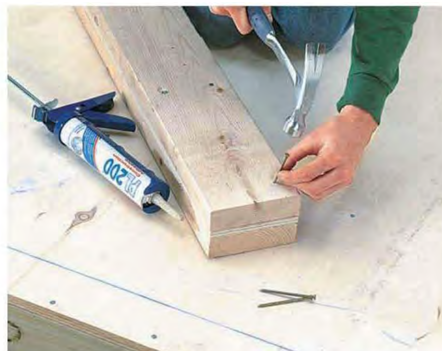
C. Construct the headers from 2× lumber and a \frac{1}{2} " plywood spacer. Assemble the pieces with adhesive and nails.
