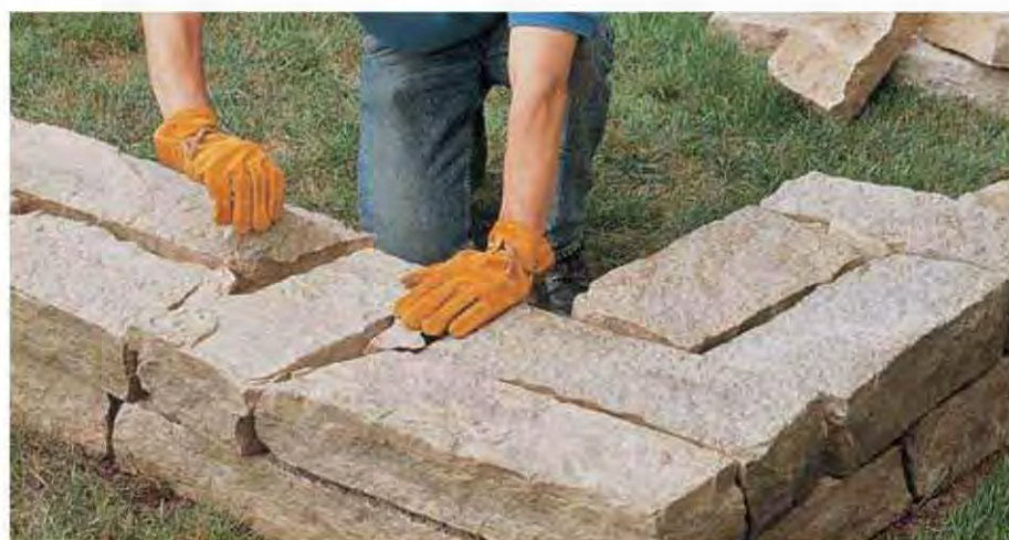
C. Build up the corner two courses high, with tie stones across the width of each just before they meet. Lay the rest of the course, working from the corner to the end of the wall.
