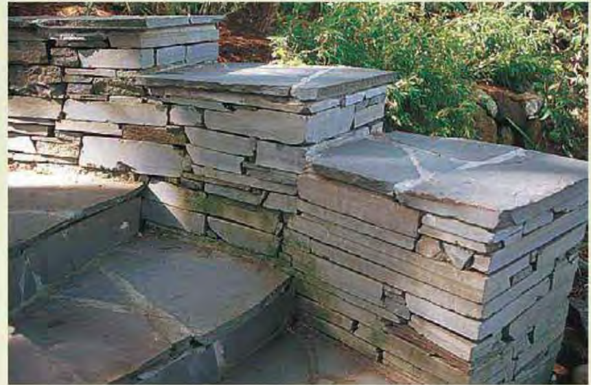
If the wall goes up or downhill, step the trench, the courses, and the top of the wall to keep the stones level.
