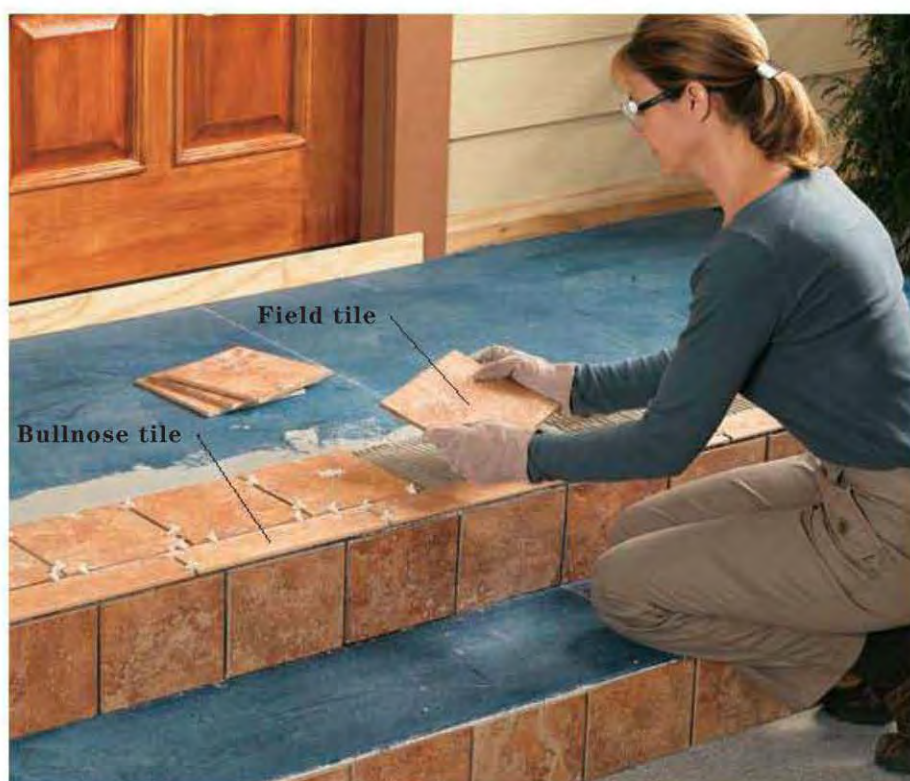
18. Set the first row of field tiles, maintaining an even gap between the field tiles and the bullnose tiles. Set the remaining field tiles.
