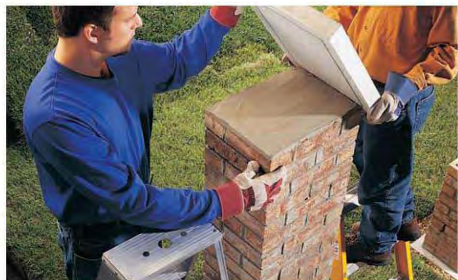
E. Spread a \frac{1}{2} "-thick bed of mortar on top of the pillar, and center the cap, using the reference lines.
