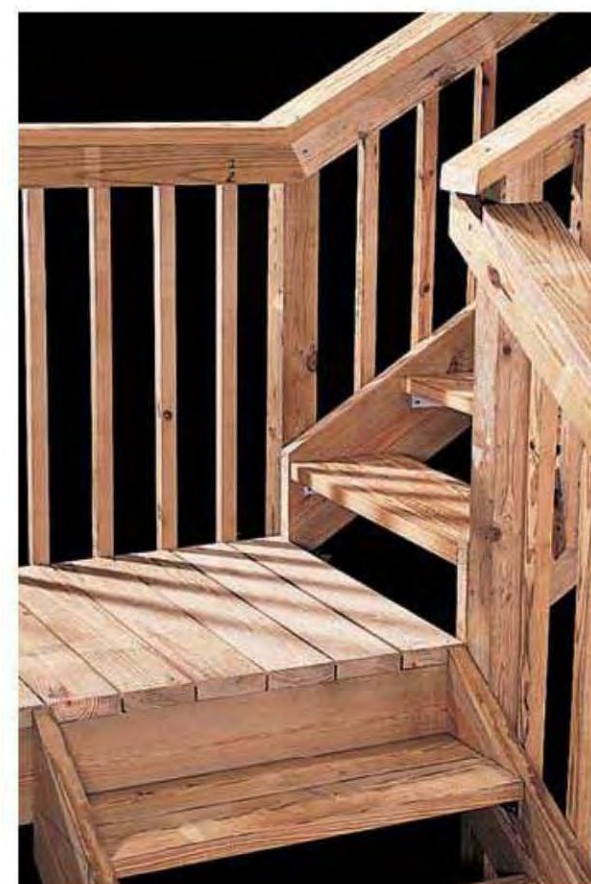
Long stairways sometimes require landings. A landing is a small platform to which both flights of stairs are attached.
