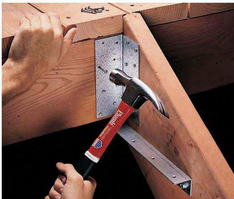
7. Position the stair stringers against side of deck, over the stringer outlines. Align top point of stringer flush with the surface of the deck. Attach stringers by nailing the angle brackets to the deck with 10d joist hanger nails.
