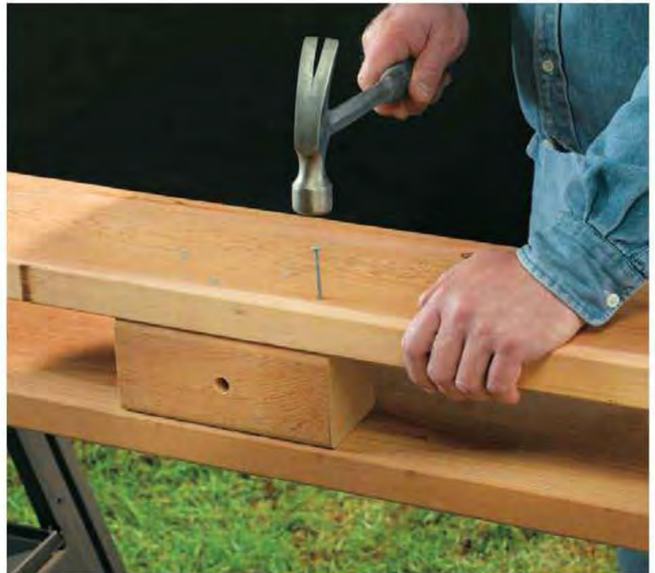
C. Sandwich the blocks between the main beams, and fasten the assemblies with exterior adhesive and 16d nails.
