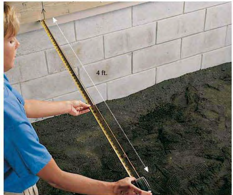
9. Measure mason's string 4 feet from edge of ledger, and mark with masking tape.
