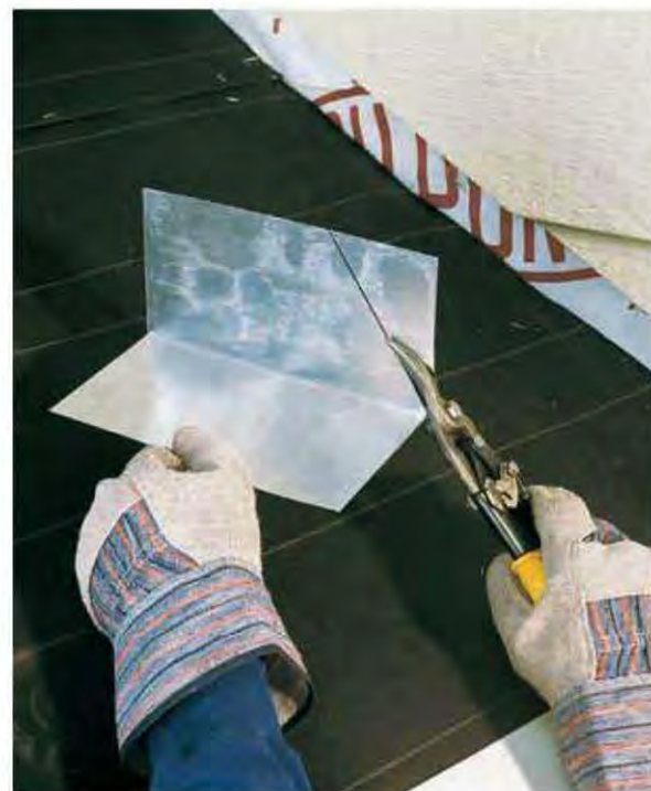
B. Trim the flashing to follow the vertical edge of the roof with aviation snips.
