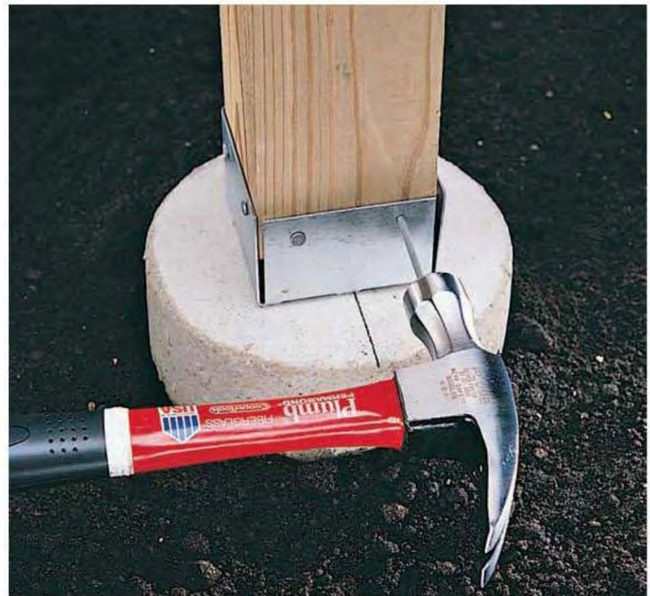
10. Attach the post to the post anchor with 6d galvanized common nails.
