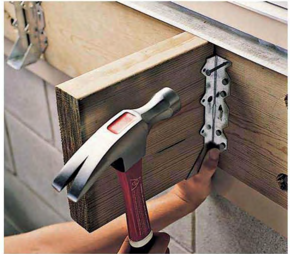
13. Nail the remaining side flange to the framing member with 10d joist hanger nails. Remove spacer.
