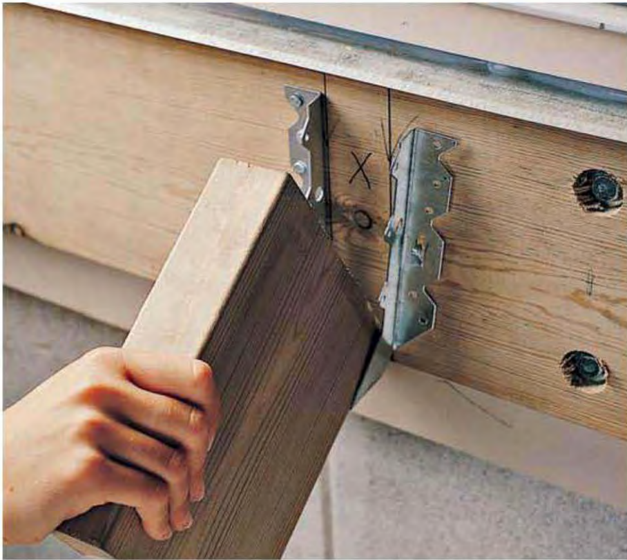
12. Cut a scrap board to use as a spacer. Hold spacer inside each joist hanger, then close the hanger around the spacer.
