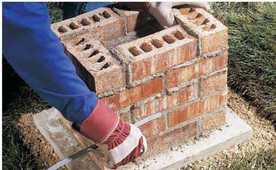
C. Lay each new course so the bricks overlap the joints of the previous course. Use a jointing tool after every five courses to smooth the firm mortar joints.
