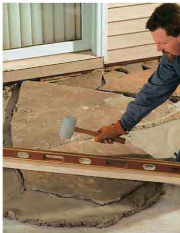
D. Bed the first stone into the mortar, then check it for level.
