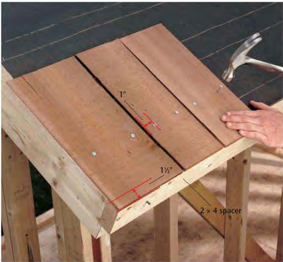
A. Install the starter row of shingles, overhanging the gable end by ⅜" and the eave by 1½".
