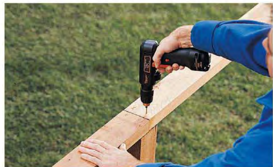
A. Trim the posts and attach the cut stringers on top of the posts with 3" galvanized deck screws.
