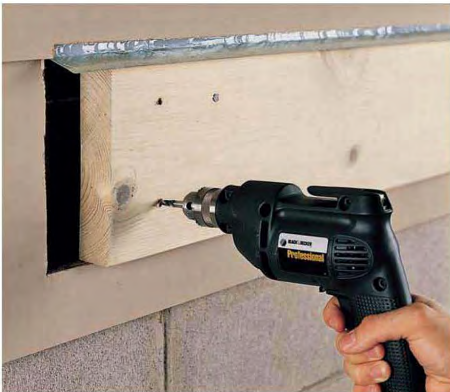
7. Drill pairs of \frac{1}{4} " pilot holes spaced every 2 feet, through the ledger and sheathing and into the header joist.
