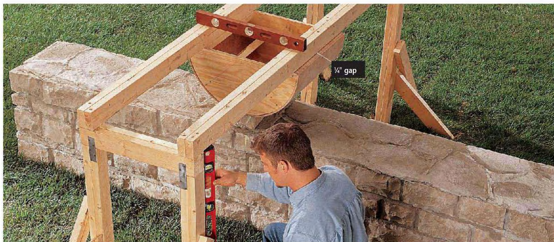
C. Build a 2 × 4 scaffold for the arch form. Position the form on the first stone, level the scaffold, and brace the legs with 2 × 4s.
