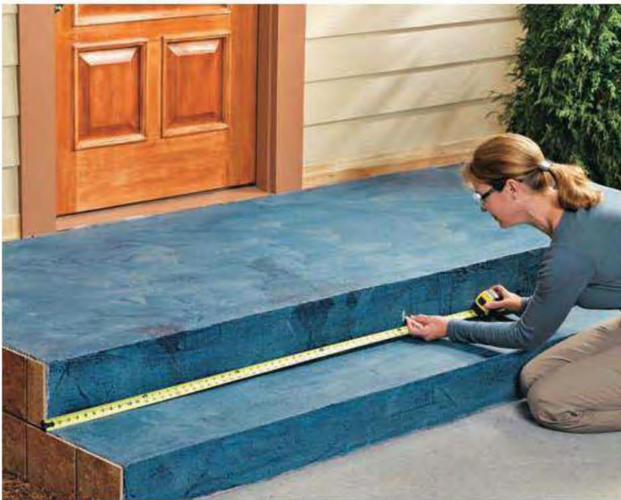
11. Measure the width of a riser, including the thickness of the tiles you've laid on the step sides. Calculate the centerpoint and mark it clearly with chalk or a high visibility marker.
