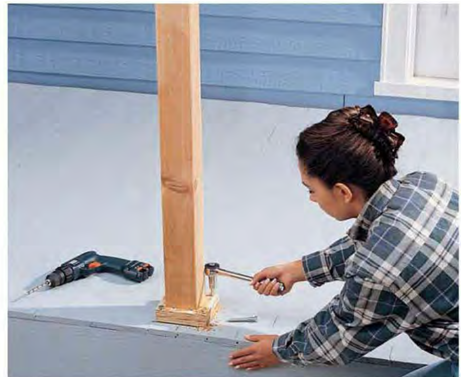
B. Position the post on the porch floor, drill pilot holes at each corner of the base plate, and secure with \frac{3}{8} \times 4 " galvanized lag screws.
