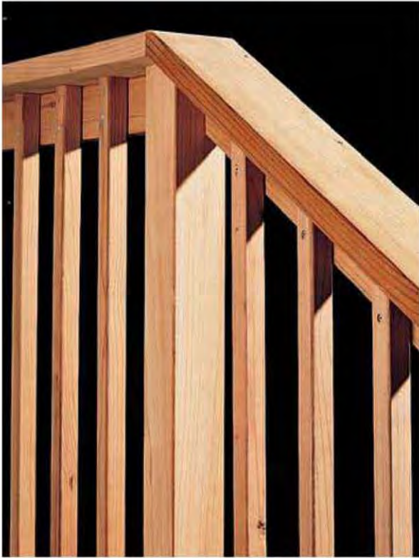
Vertical balusters with posts and rails are a good choice for houses with strong vertical lines. A vertical baluster railing like the one shown above is a good choice where children will be present.
