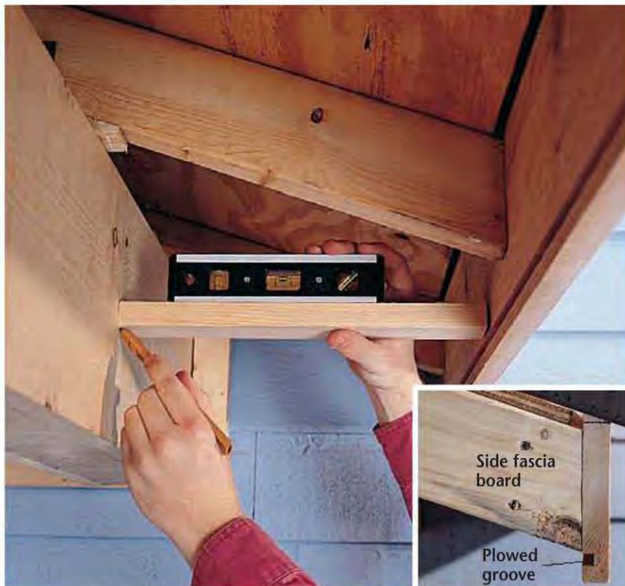
A. Transfer the top height of the plowed groove in the side fascia to the beam and mark a reference for the nailer using a torpedo level. INSET: Plowed groove in side fascia.
