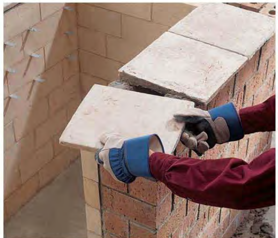
F. Install the capstones in a bed of Type N mortar with a \frac{3}{8} "-thick joint.
