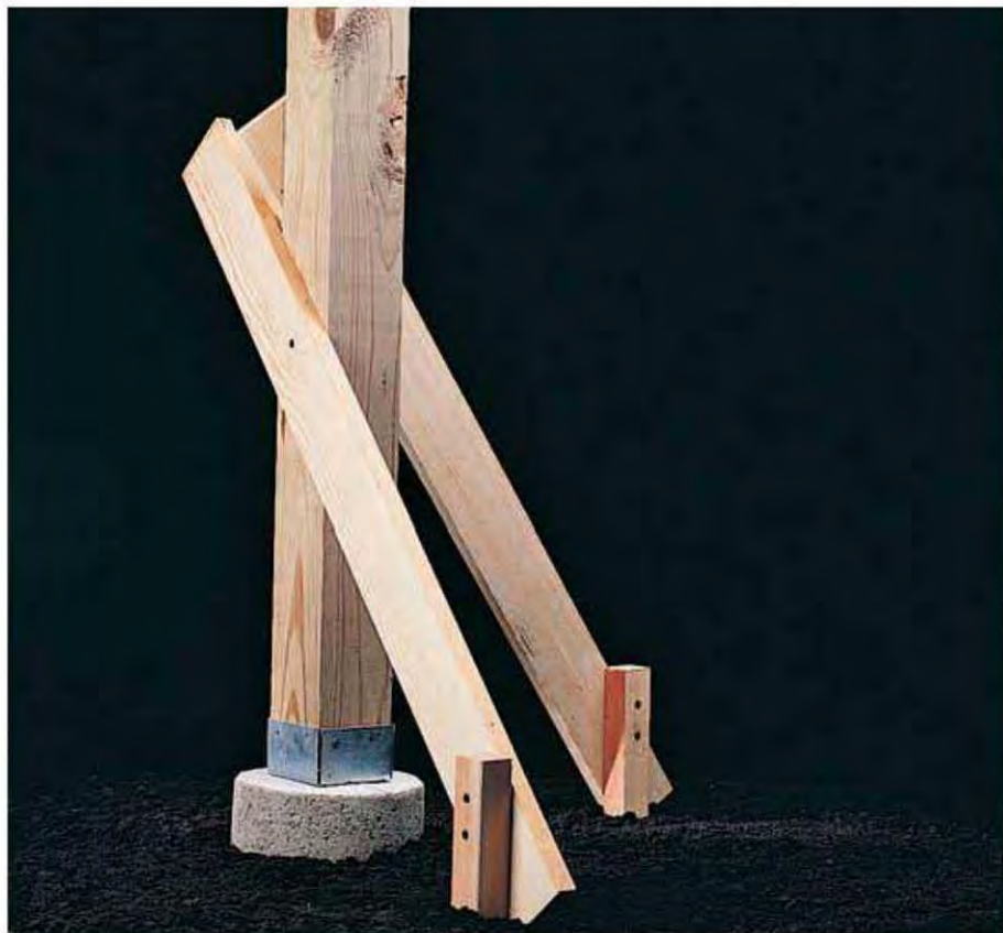
9. Plumb and brace the post on the side perpendicular to the first brace.
