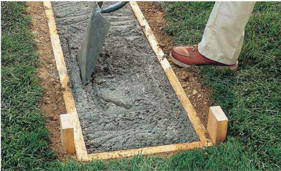
1. Dig trenches and pour footings twice as wide as the proposed wall (reference page 84).
