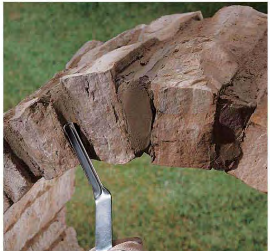
G. Mist the stones lightly and tuck-point each joint with stiff mortar, then tool them, using a jointing tool.
