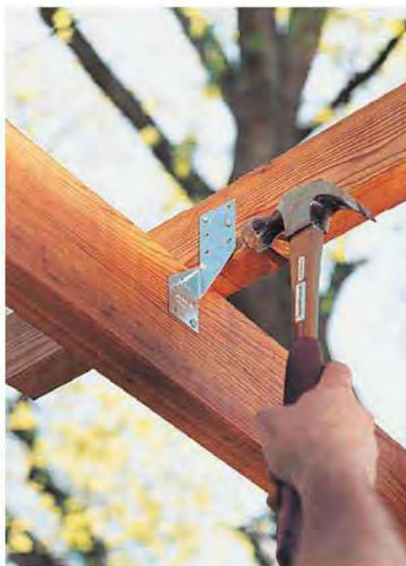
E. Attach the rafters to the tie beams with rafter ties and galvanized nails.
