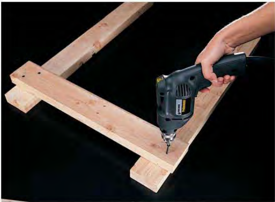
A. Cut the batter board pieces from 2 × 4 lumber and assemble them with screws.
