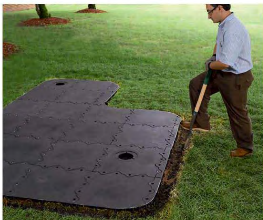
11. Dig a 4"-wide by 4"-deep trench around the perimeter of the green shape, directly next to the edges of the panels.
