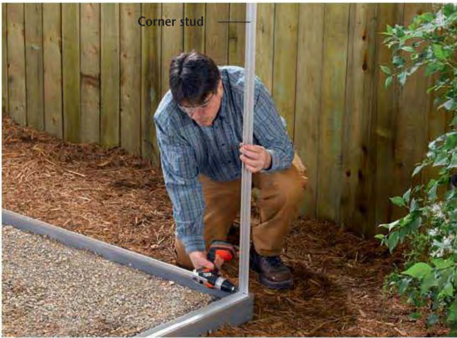
5. Fasten the four corner studs to the bottom wall plates using hold-down connectors and bolts. In this system, each corner stud is secured with two connectors.
