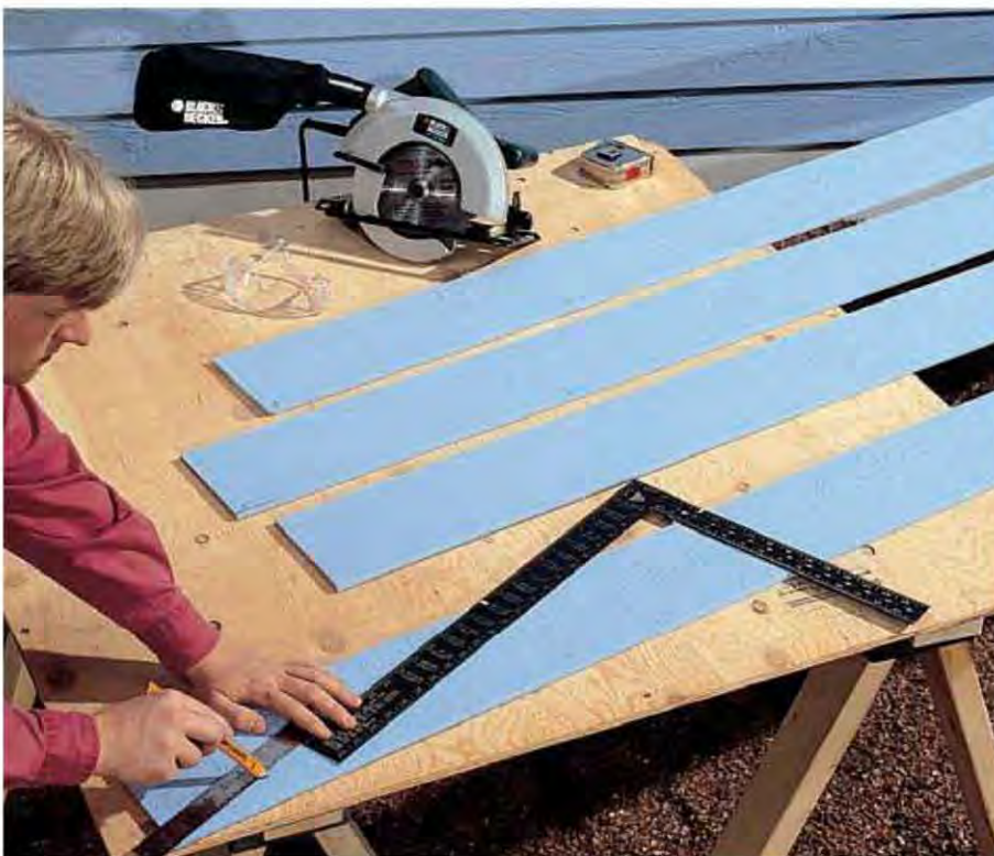
A. Mark cutting lines on the pieces of siding to match the slope of the roof using a framing square or a rafter square and a straightedge.
