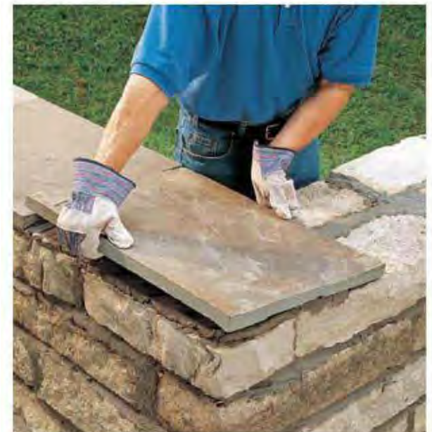
D. Center flat cap stones on top of the wall, setting them in a level bed of mortar.
