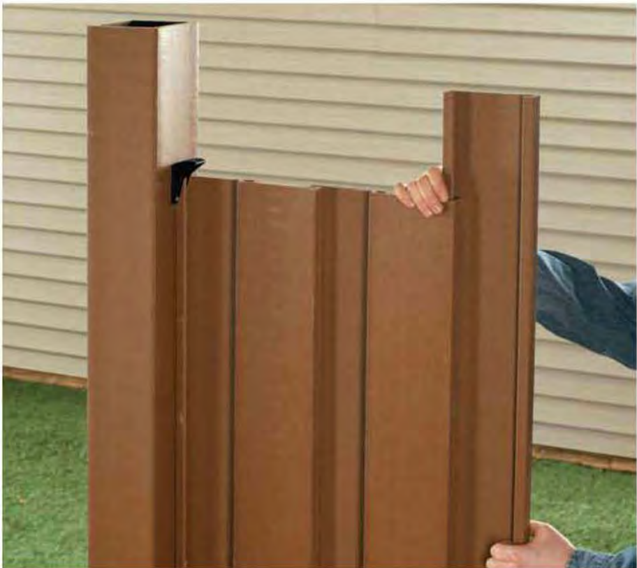
10. Continue filling in with the interlocking siding strips.
