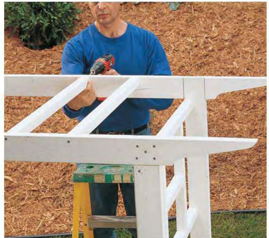
E. Attach four evenly spaced 2 × 2s between the tie beams for rafters using 2 1/2" galvanized deck screws.
