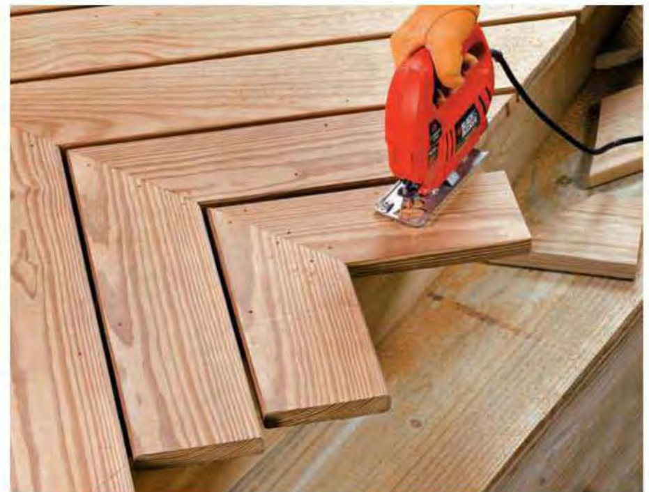
Use a jigsaw to trim the decking boards overhanging the curved rim joist.
