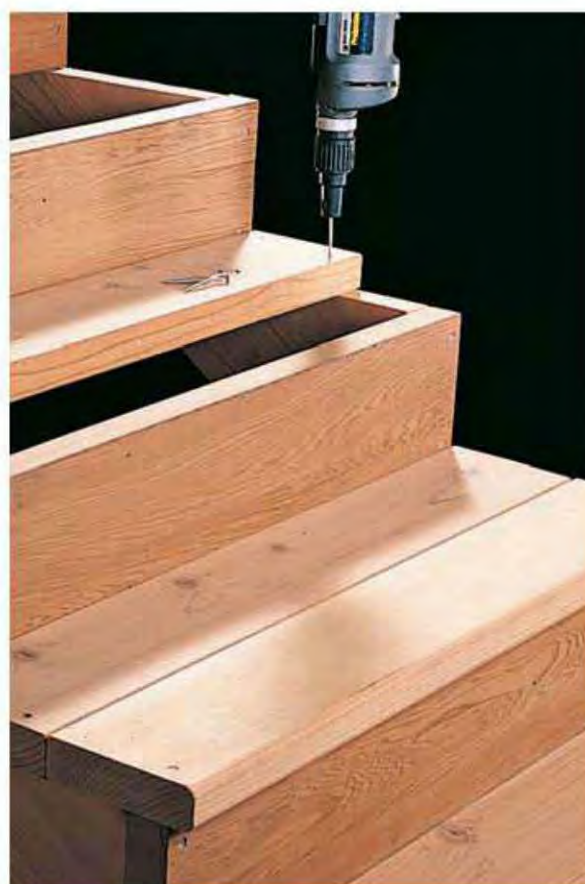
Boxed steps , built with notched stringers and solid risers, give a finished look to a deck stairway. Predrill ends of treads to prevent splitting.
