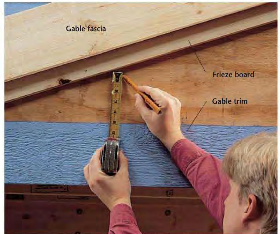
B. Measure from the bottom edge of the frieze boards to find the size of the subsequent pieces of siding. Overlap the siding so the reveal matches the siding on your house.
