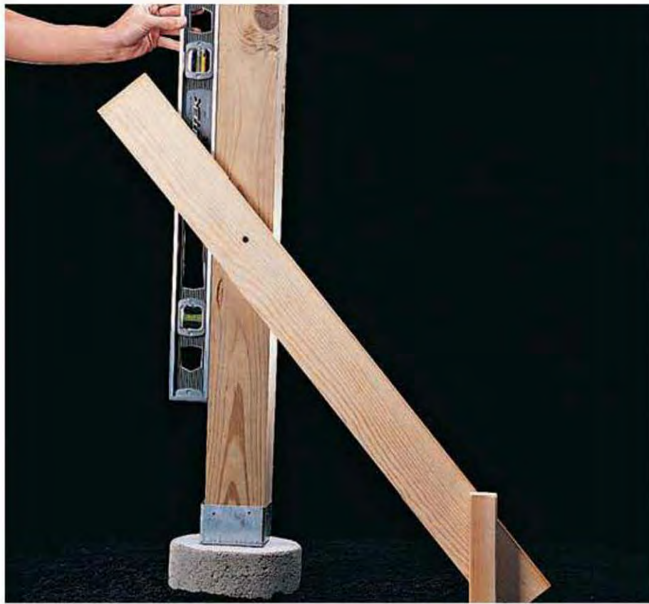
7. Use a level to make sure the post is plumb. Adjust the post, if necessary.
