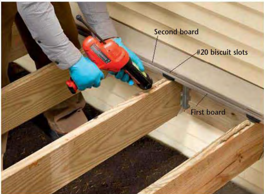
3. Lay a bead of construction adhesive along the edge of the joist to keep it from squeaking later. Cut slots in the adjacent deck board and fit it over the clips of the previous board.
