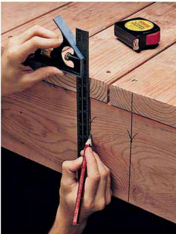
5. Measure and mark position of posts around the outside of the deck using a combination square as a guide. Plan to install a post on outside edge of each stair stringer.
