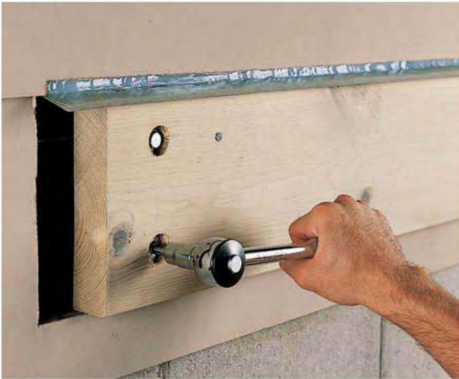
9. Attach ledger to wall with \frac{3}{8} \times 4 " lag screws and washers using a ratchet wrench or impact driver.
