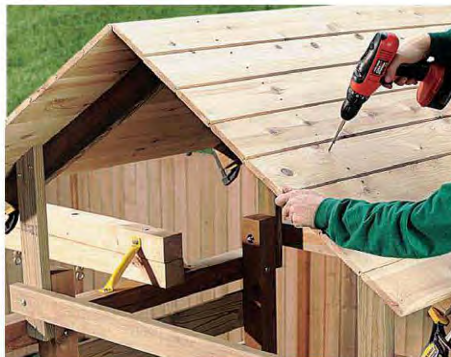
M. Use tongue and groove cedar to cover the roof, fastening it to the rafters with deck screws. Allow the ends to overhang the rafters by 6".
