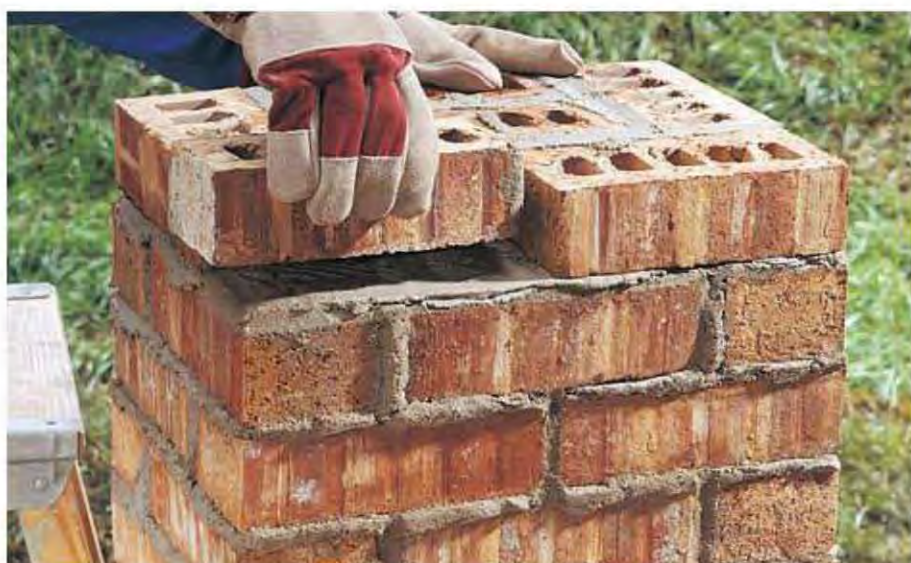
D. Lay the final course over a bed of mortar and wire mesh, with an additional block added to the center. Fill the joints with mortar, and work them with a jointing tool as soon as they become firm.
