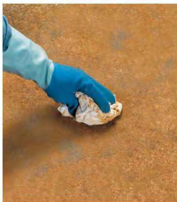
2. Once stain has absorbed, remove residual stain with rags.
