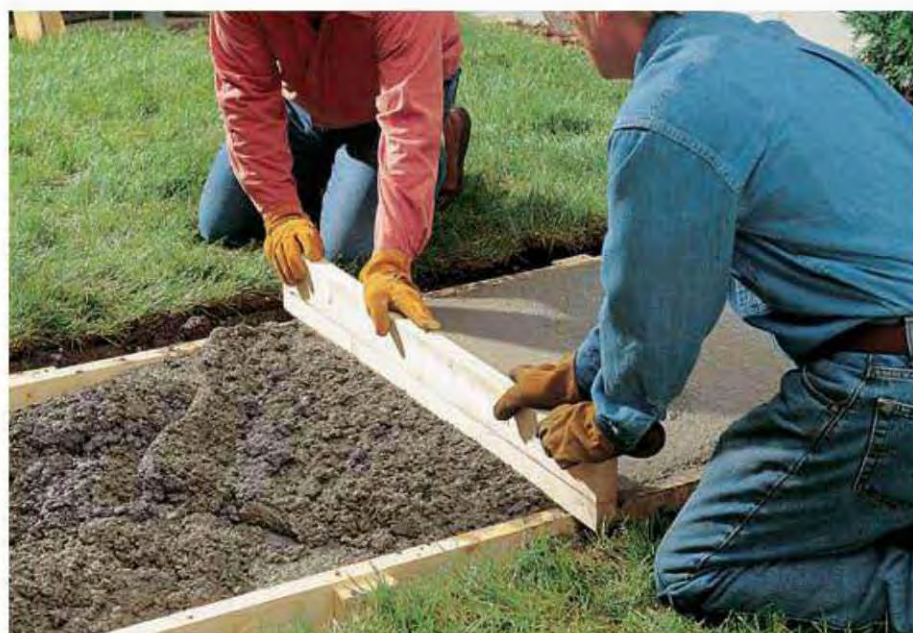
8. Build a curved screed board and use it to form a crown when you smooth out the concrete. NOTE: A helper makes this easier.
