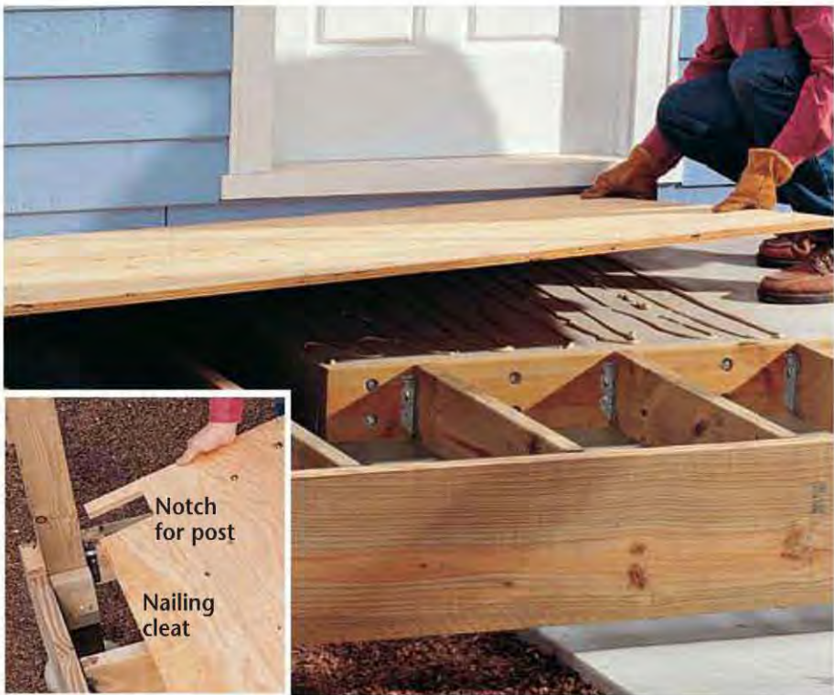
A. Cut pieces of plywood subfloor to size and install with deck screws. INSET: Notch plywood pieces to fit around posts, and fasten to nailing cleats attached to posts.
