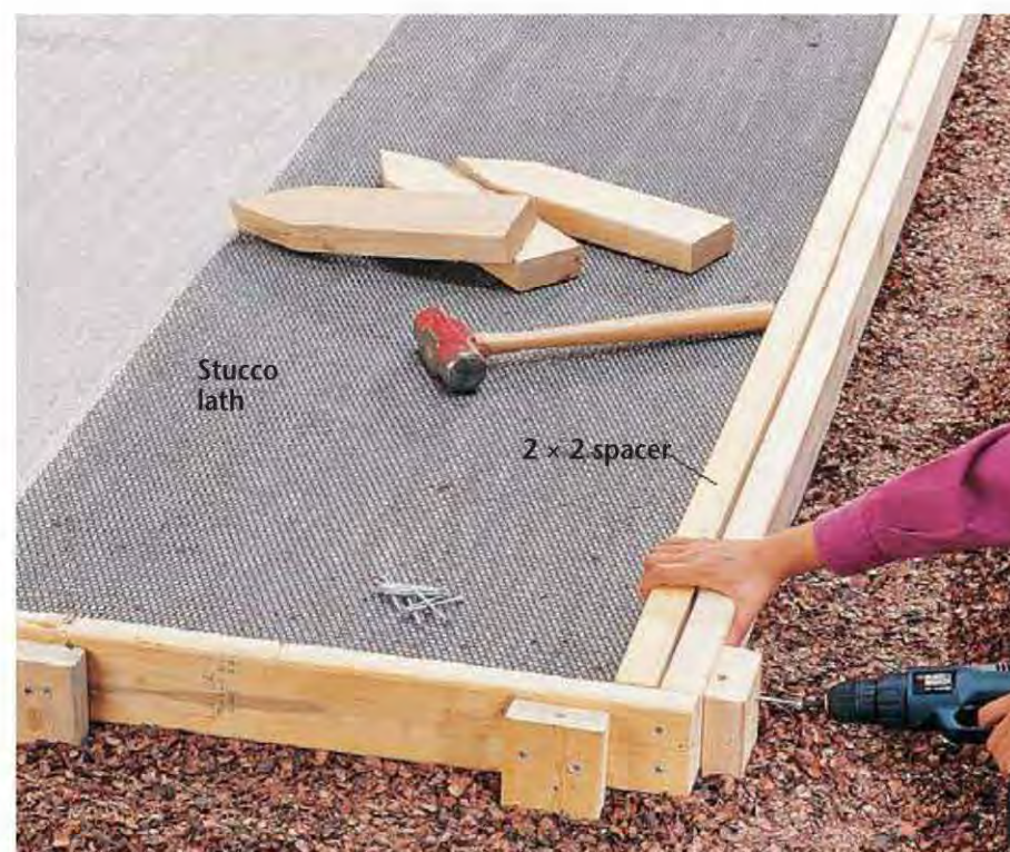
A. Adjust the form height by setting stucco lath on the surface, then place a 2 × 2 spacer on top of the lath (their combined thickness should equal the thickness of the subbase).
