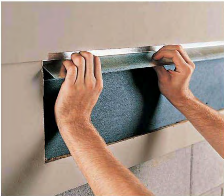
5. Cut galvanized flashing to length of cutout using metal snips. Slide flashing up under siding. Do not nail the metal flashing in place.
