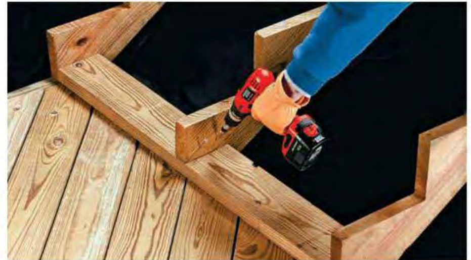
Attach the center stair stringer to the kick plate using deck screws driven at an angle.
