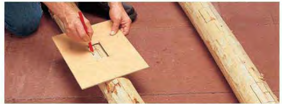
A. Outline the mortise on the first fence post according to the dimensions in the illustration above. Use a cardboard template to lay out the mortise shape.
