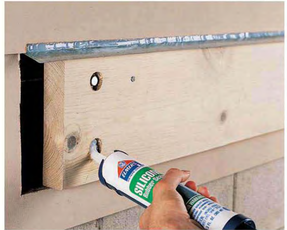
10. Seal lag screw heads with silicone caulk. Seal the crack between the wall and the sides and bottom of the ledger.
