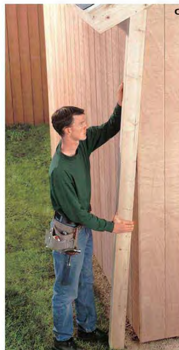
Install corner trim by nailing the two pieces together then attaching the assembly to the building.
