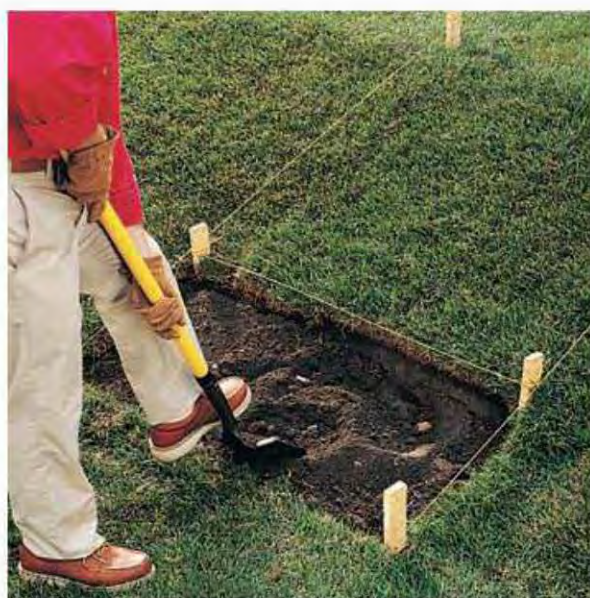
C. Excavate the area for the first step, and install the first step frame. Create a flat bed with a very slight forward slope, dropping about \frac{1}{8} " from back to front. Tamp the soil down firmly using a hand tamp. Set the timber frame into the excavation area and check for level. Using a spade bit, drill two 1" guide holes in the front timber and the back timber, 1 ft. from the ends. Anchor the steps to the ground by driving a 2½-ft. length of \frac{3}{4} " pipe through each guide hole until the pipe is flush with the timber.
