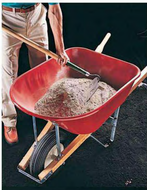
6. Mix dry ingredients for concrete in a wheelbarrow using a hoe.
