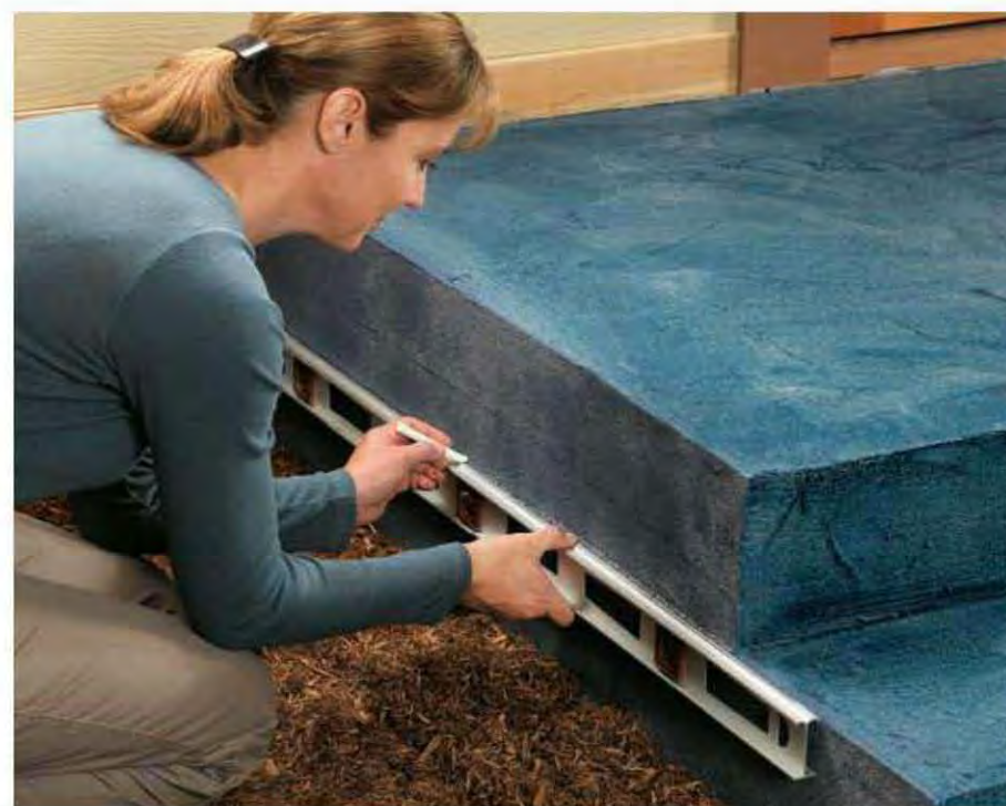
7. The sequence is important when tiling a stairway with landing. The primary objective is to install the tile in such a way that the fewest possible cut edges are visible from the main viewing position. If you are tiling the sides of concrete steps, start laying tile there first. Begin by extending horizontal lines from the tops of the stair treads back to the house on the sides of the steps. Use a 4-foot level.
