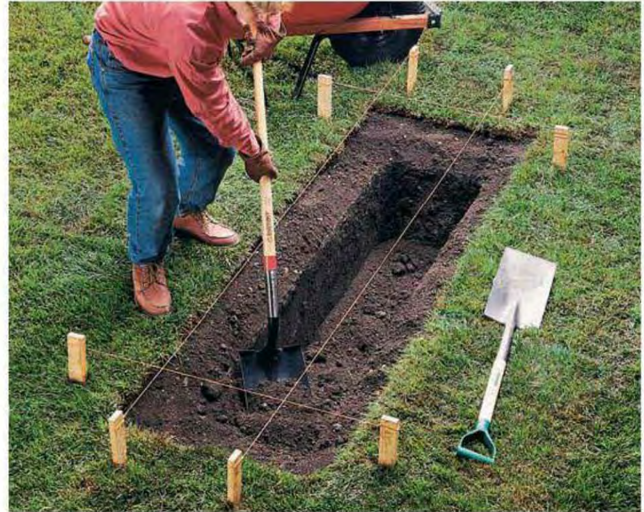
2. Strip away sod 6" outside the project area on all sides, then excavate the trench for the footing to a depth 12" below the frost line.
