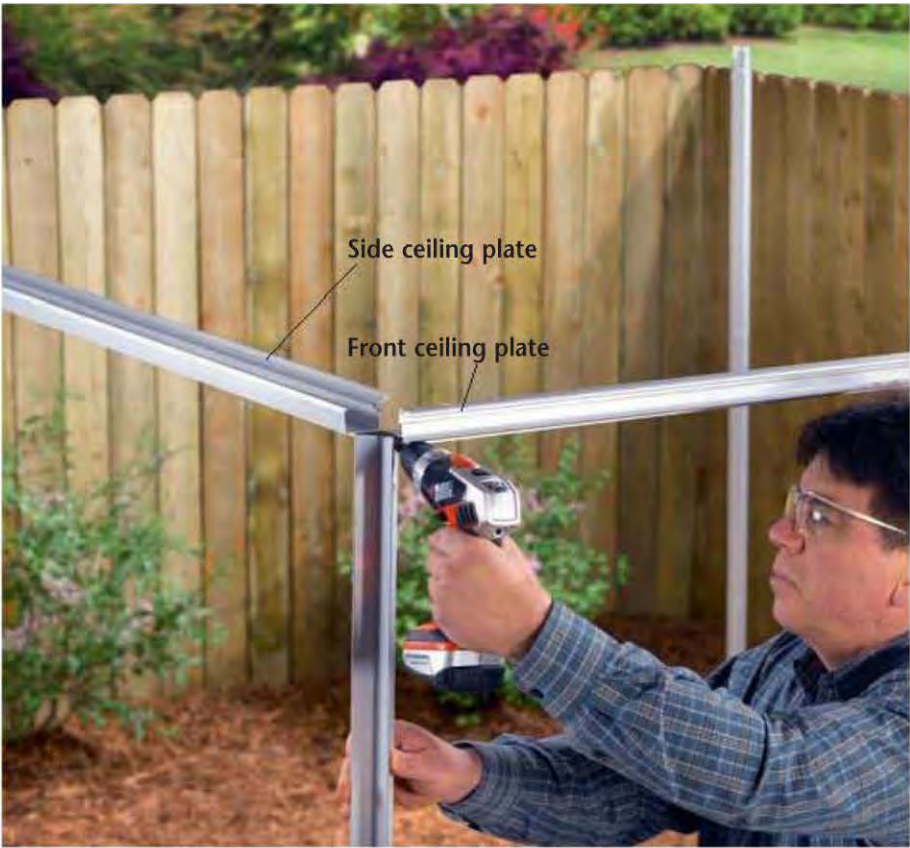
6. Assemble the pieces for each side ceiling plate, then attach one assembled side plate against the inside of the two corner studs, making sure the gutter is positioned correctly. Now attach the front ceiling plate to the outside of the two corner studs that are over the front floor plate.
