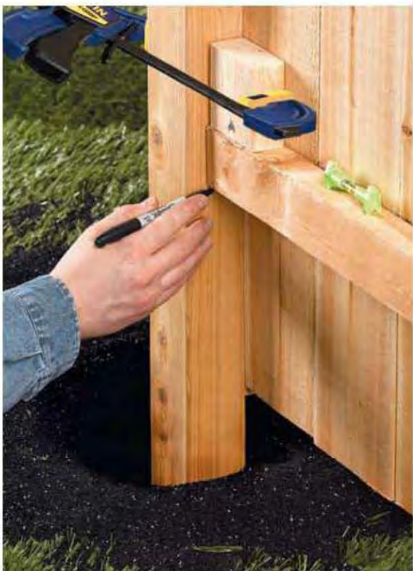
7. Position a post in the next post hole and clamp the unattached end of the fence panel to the post (you may need to tack a clamping block to the post rail first). Mark the positions of the rails onto the post. Unclamp the fence panel and remove the post from the hole.
