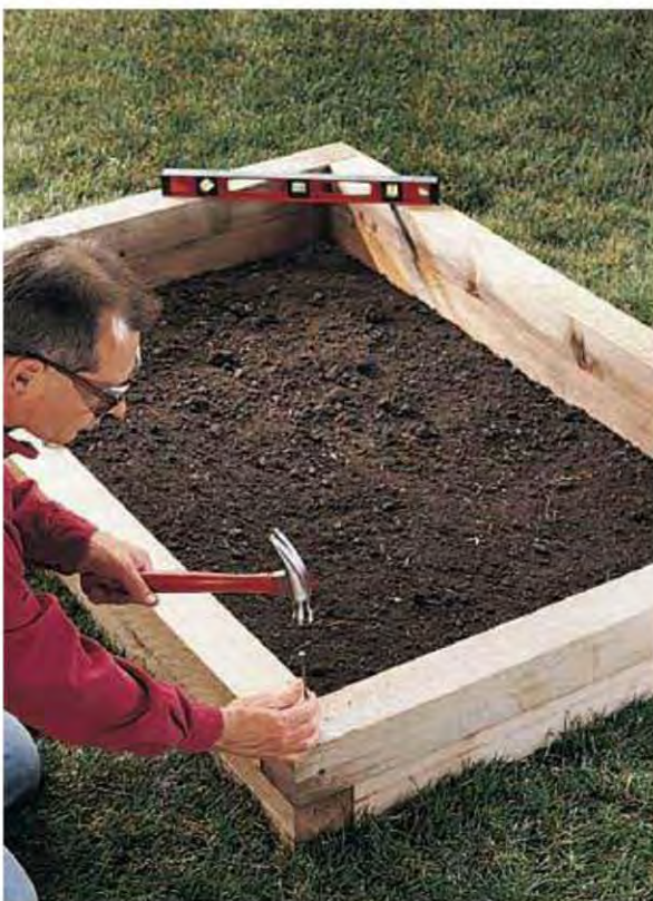
B. Level timbers in the trench, then lay the next layer, staggering the joints. Drill holes and drive nails through them.
