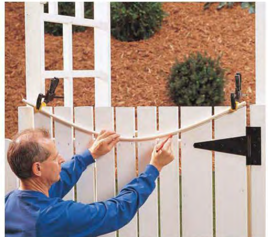
J. Clamp the ends of a length of PVC pipe at each end of the gate top. Deflect the pipe down to create the curve and trace. Cut to shape using a jigsaw.
