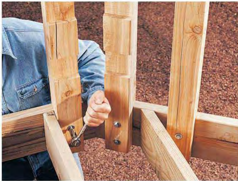
Drill pilot holes through the posts and into the rim joists, and attach the posts with lag screws. Note the unnotched stairway post.
