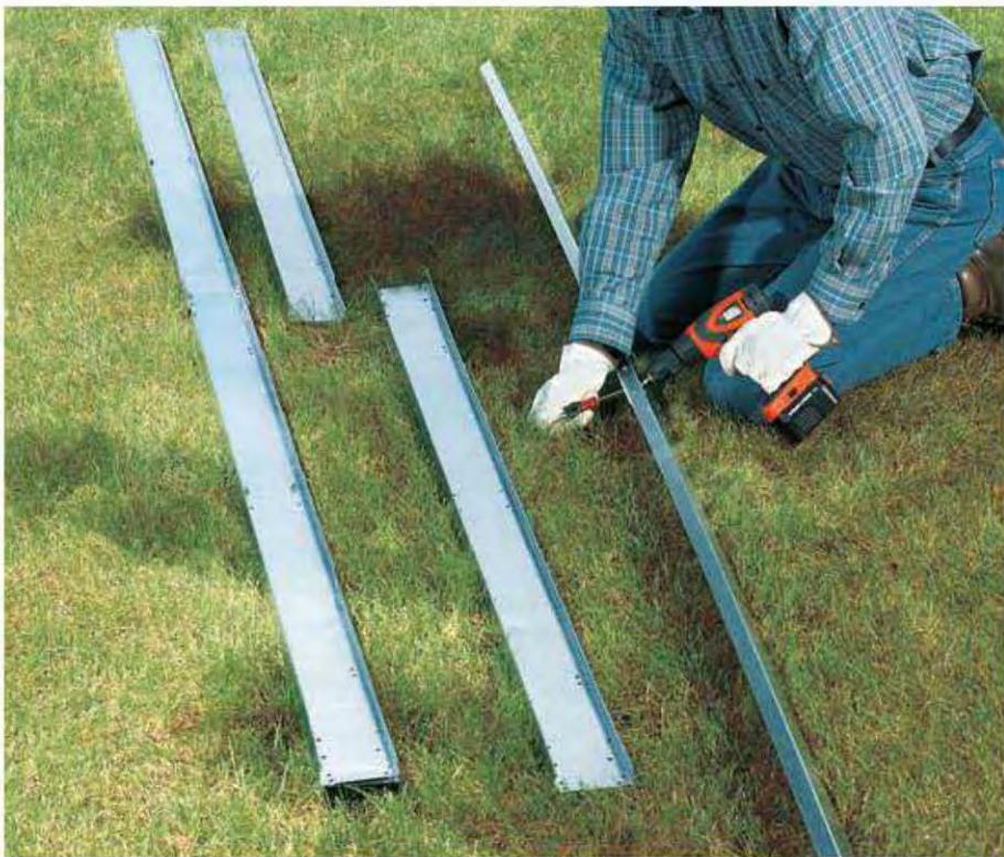
8. Lay out the parts for assembling the roof beams and the upper side frames and confirm that they fit together properly. Then, join the assemblies with the fasteners provided.
