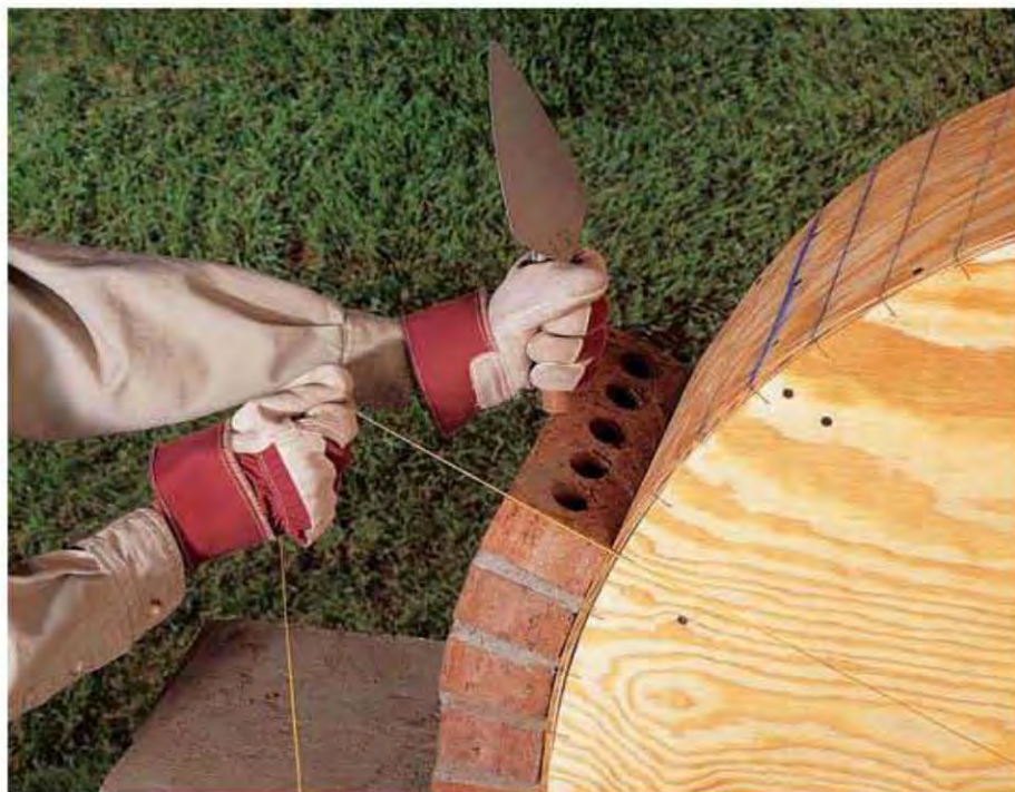
C. Place five bricks, then tack a string to the center point of the form on each side, and use the strings to check each brick's alignment.
