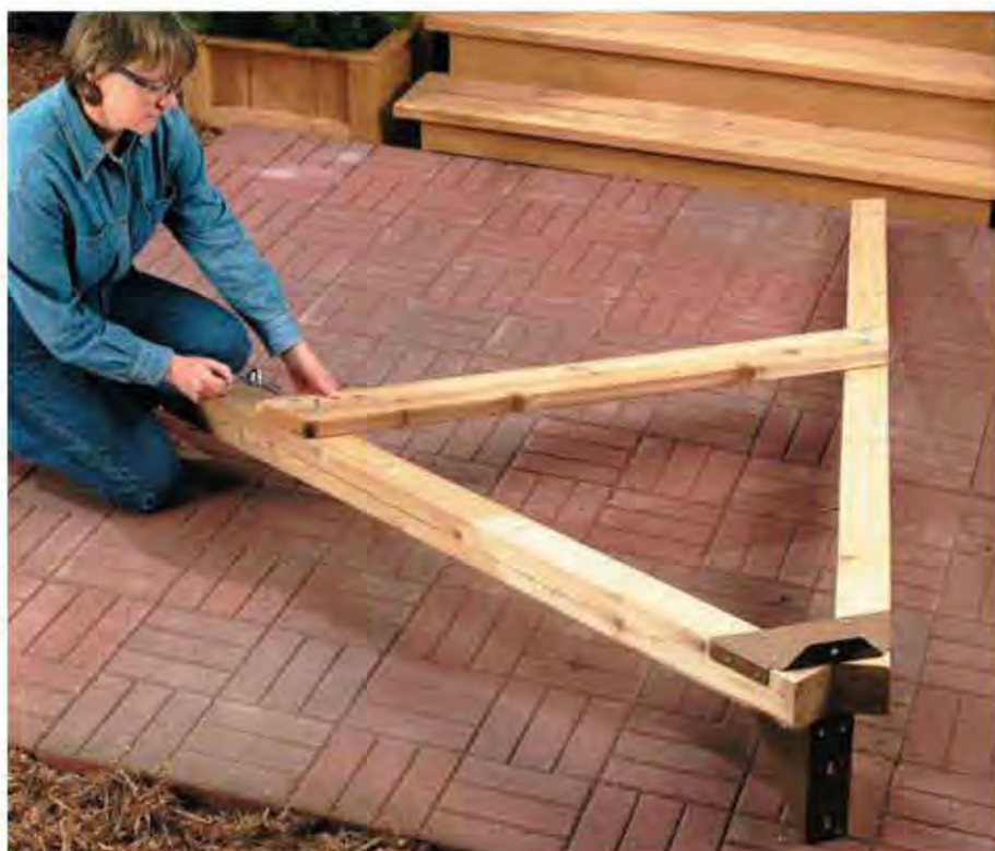
A. Insert carriage bolts through the brace and legs. Fasten a washer and nut in the recesses, then tighten the nut.
