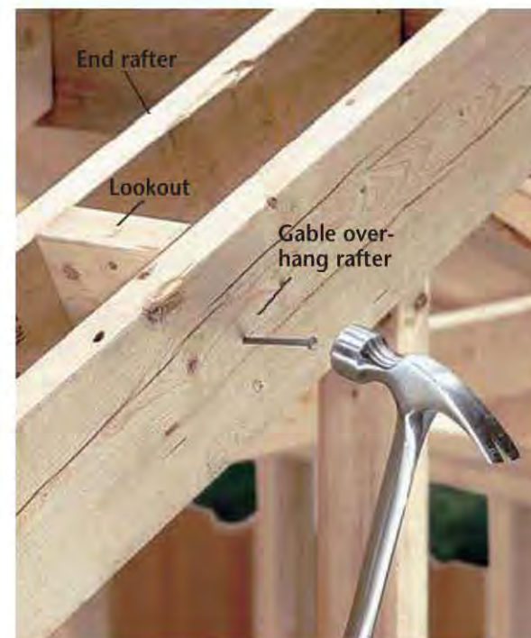
I. Nail the outer gable overhang rafters to the lookouts, making sure the top edges of the rafters are flush.
