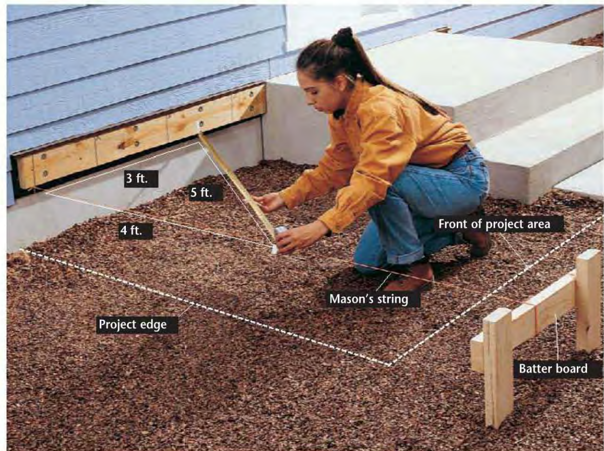
E. Establish square lines for the sides of the porch by using the 3-4-5 carpenter's triangle, then measure for the location of the posts and drop a plumb bob to transfer the center point of the post to the ground.
