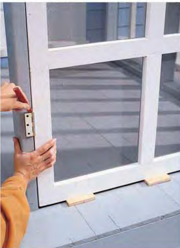
G. Mark the hinge locations onto the doorframe, then chisel mortises deep enough so the hinge plate will be flush with the surface of the frame.
