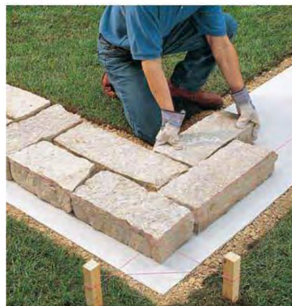
A. Pour footings and let them cure. Dry-fit stones to follow the mason's string guides, staggering the joints (see page 84).
