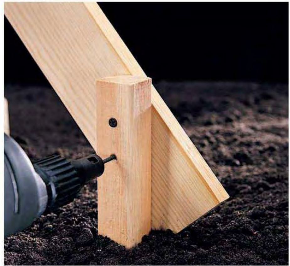
8. Attach the brace to the stake with two 2" wallboard screws.
