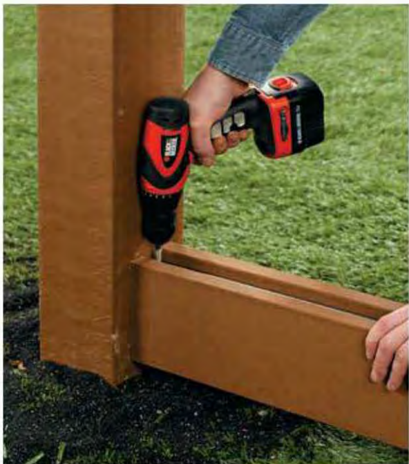
7. Attach each side of the rail insert to its bracket with a screw provided for the purpose.
