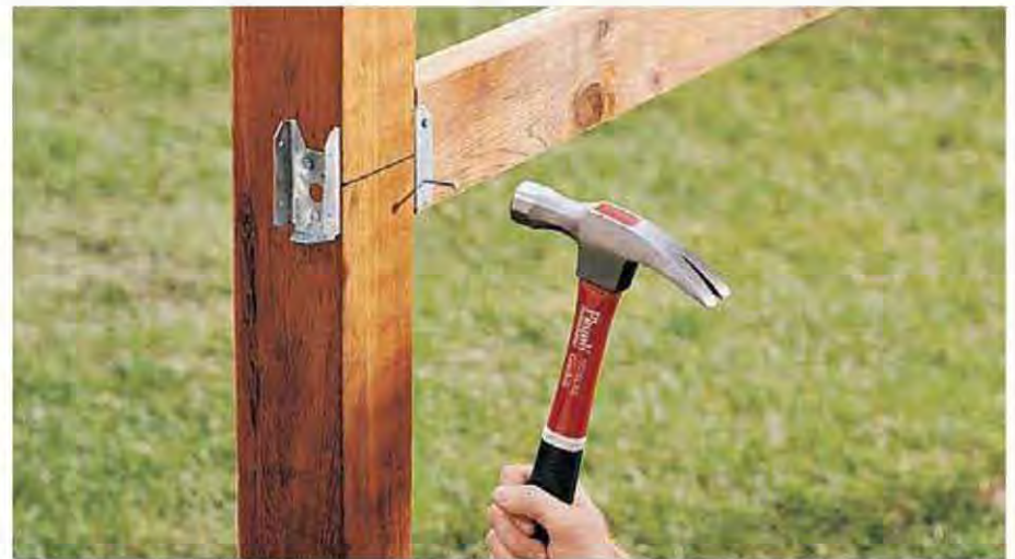
B. Attach the fence brackets to the inside faces of the posts. Position the stringers in the brackets, then nail them in place.
