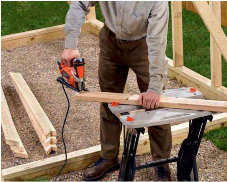
8. Mark cutting lines for the rafters using the templates and cut them all. You'll need to use a jigsaw or handsaw to make the bird's-mouth cuts on the rafter ends that rest on the kneewall.
