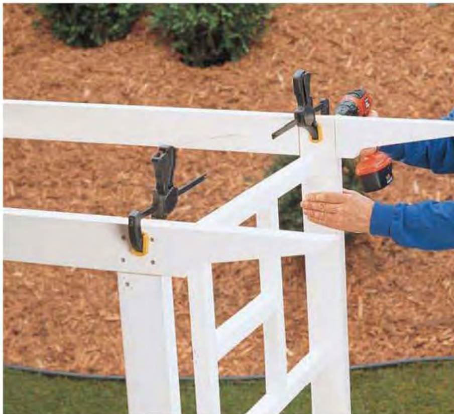
D. Cut 2 × 4s using the grid pattern for tie beams. Dado each to accommodate the trellis frame post tops, then clamp into position and attach with five 1 1/2" galvanized deck screws at each joint.
