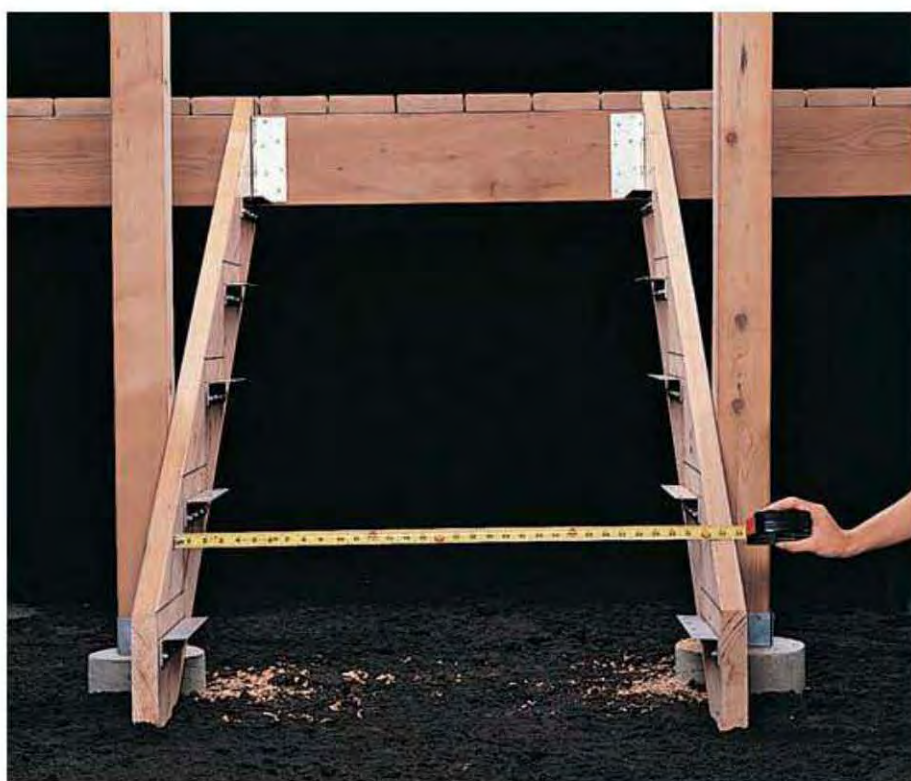
9. Measure width of stair treads. Cut two 2 x 6s for each tread using a circular saw.
