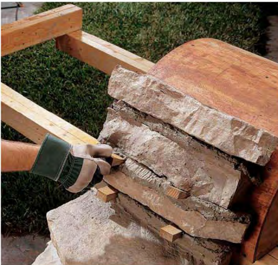
F. Lay the stones around the circle, working from the bottom up, so the keystone is laid last. If necessary, use wood shims to prevent mortar from seeping out of the joints.
