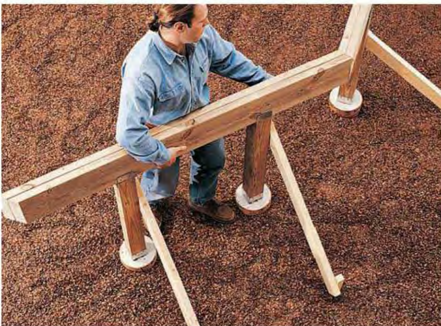
Fit beam C-4 tightly against beam C-3 and attach the two beams to each other with deck screws.
