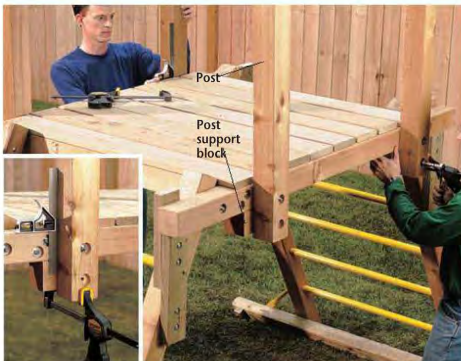
F. Clamp the posts in place, make sure they are properly aligned, and plumb (INSET), then attach to the lower beams and support blocks with lag screws.
