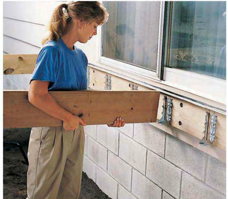
15. Seal cut ends with clear sealer-preservative. Place joists in hangers with crowned edge up.
