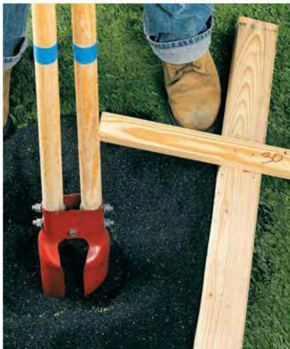
2. Dig a post hole at a corner or an end post location. A clam-shell type post-hole digger is a good choice for holes up to 30" deep. Make a depth gauge from scrap wood to measure the hole depth as you dig.
