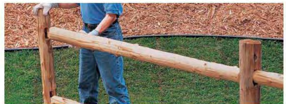
D. Assemble the entire fence with the posts loose set in the post holes. Once all the rails are in place, square and plumb each section and then pack the posts in more tightly or set in concrete.
