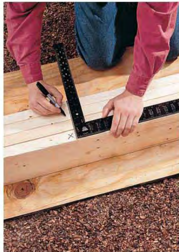
D. Nail the beam members together in pairs, then lay out the truss locations 24" on center across the tops using a framing square.
