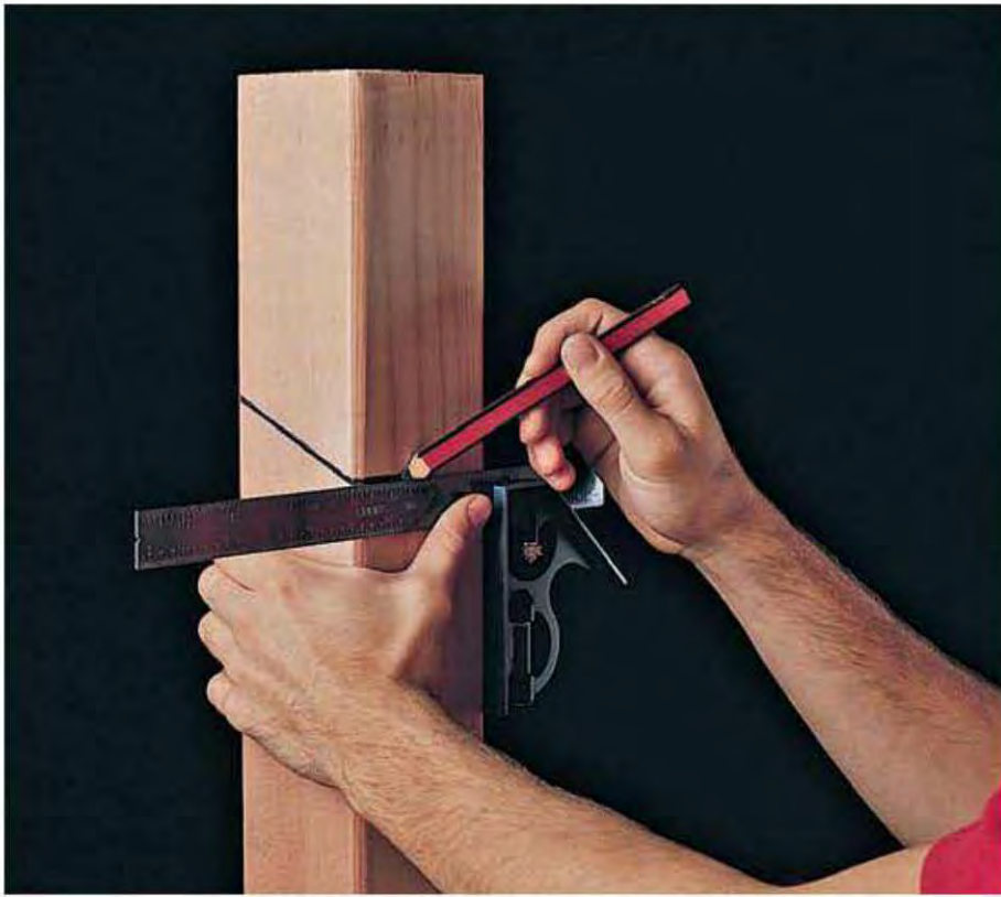
18. Extend the pencil lines across both sides of the stairway post using a combination square as a guide.
