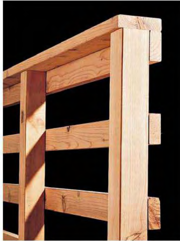
Horizontal railings are often used on low, ranch-style homes. Horizontal railings are made of vertical posts, two or more wide horizontal rails, and a railing cap.
