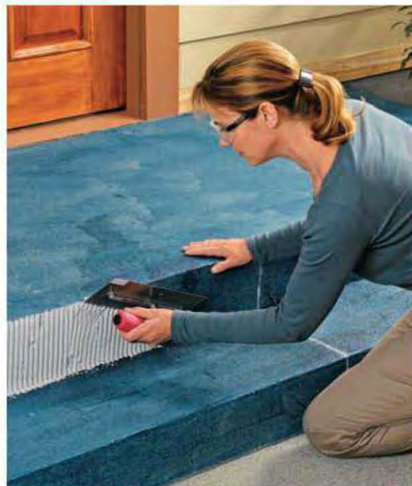
14. Trowel thinset mortar mixed with bonding adhesive onto the faces of the risers. In most cases, you should be able to tile each riser all at once.
