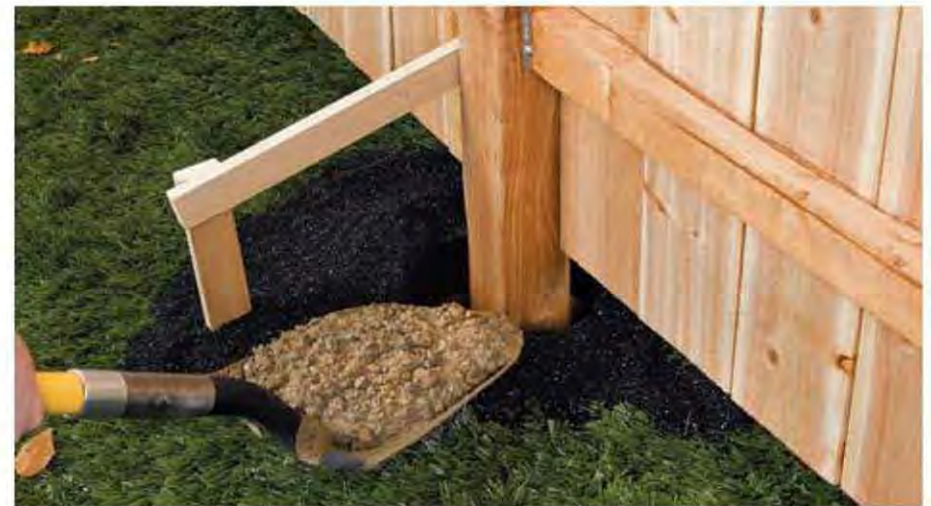
10. Finish installing the posts and panels. You can continue to fill the holes with concrete one at a time, or wait and fill them all once the posts are all positioned and braced.
