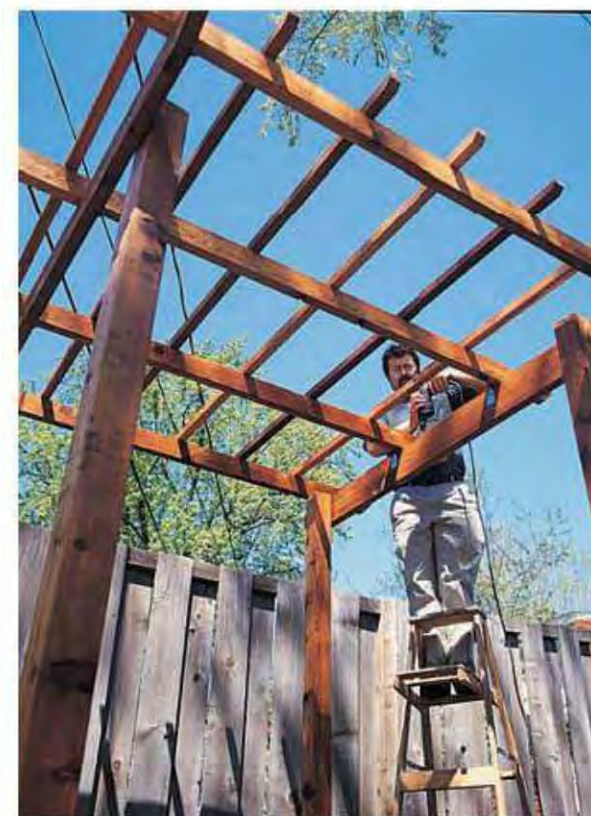
F. Space the cross strips 1 ft. apart and attach them to the rafters.
