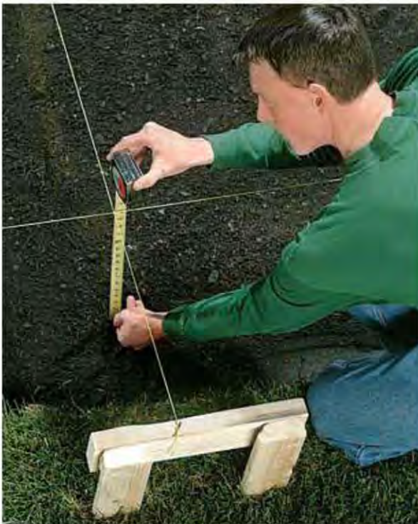
A. Measure down from the temporary cross strings to check the depth of the excavation.
