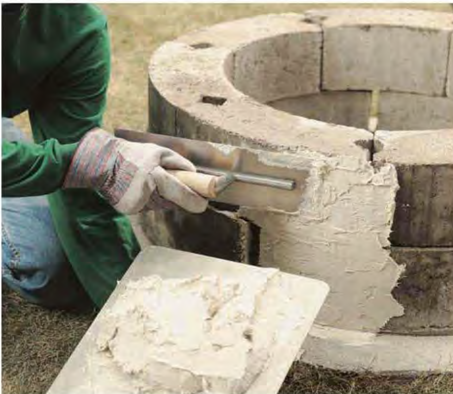
E. Mist the surface of the walls and apply surface-bonding cement with a square-end trowel. Use more surface-bonding cement on the second course to even out the gap between the courses.
