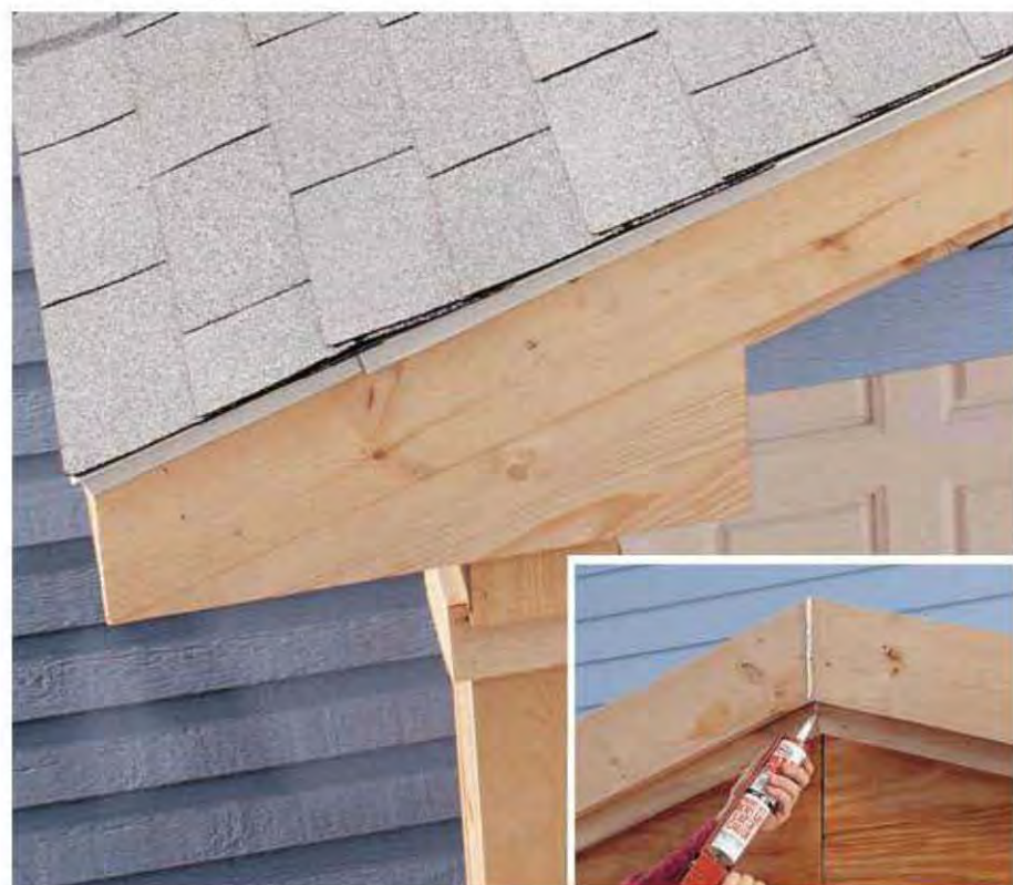
Caulk all seams between the fascia boards and cornice and at the peak of the gable (INSET).
