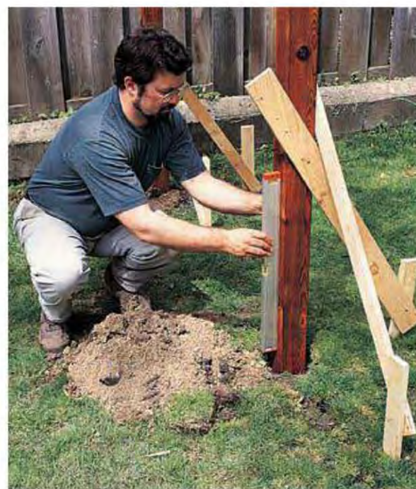
B. Brace the posts into place, then use a level to make sure they are plumb.
