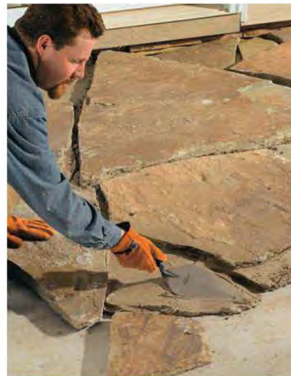
E. Add mortar and stones to complete the surface, checking for level as you go.
