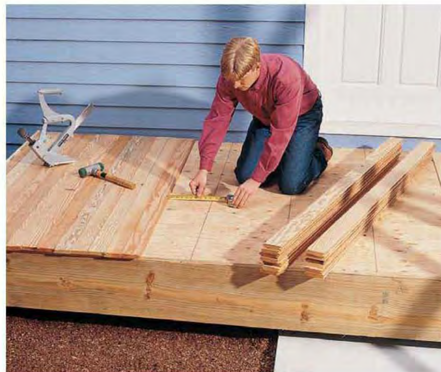
C. Install a plywood subfloor over the joists, then tongue-and-groove porch boards (pages 322 to 323). The porch boards, usually made of fir, are nailed to the subfloor with a floor nailer tool (shown).
