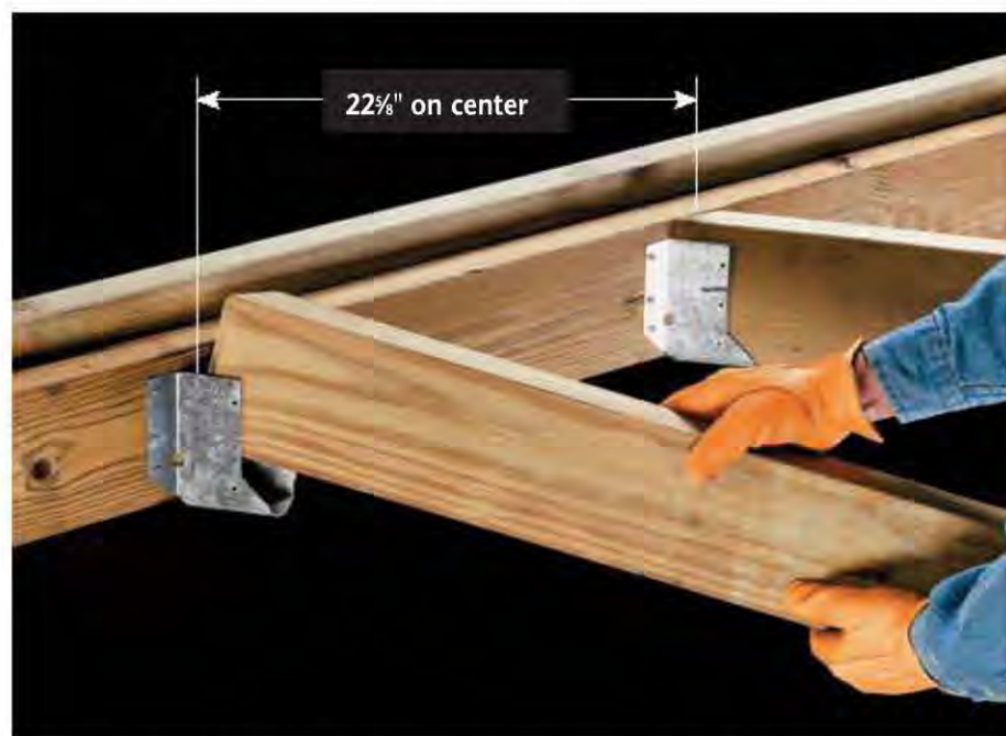
Use 45°-angled joist hangers where joists meet the angled rim joists. Space joists 22 \frac{5}{8} " on center.
