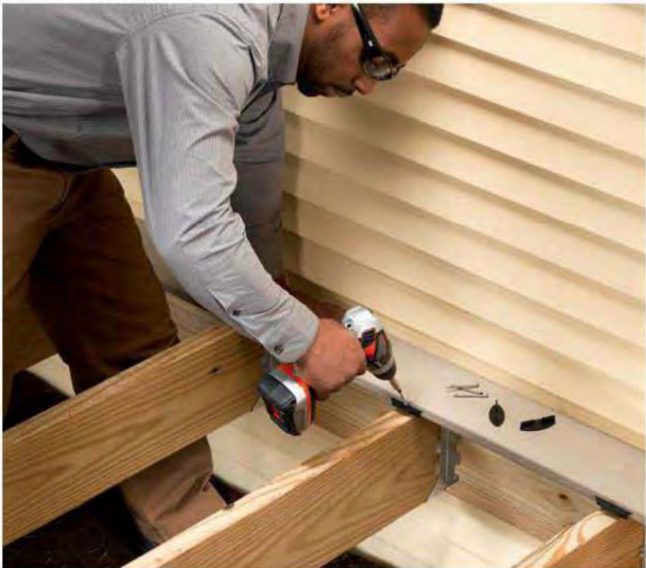
2. Insert the biscuit clip into the slot. Drive a deck screw through the hole in the clip and down at an angle through the deck board and into the joist. One screw secures two deck boards at this joist location.
