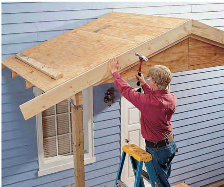
C. Cut fascia boards long enough to extend several inches past the ends of the rafter tails and attach using 8d galvanized finish nails.
