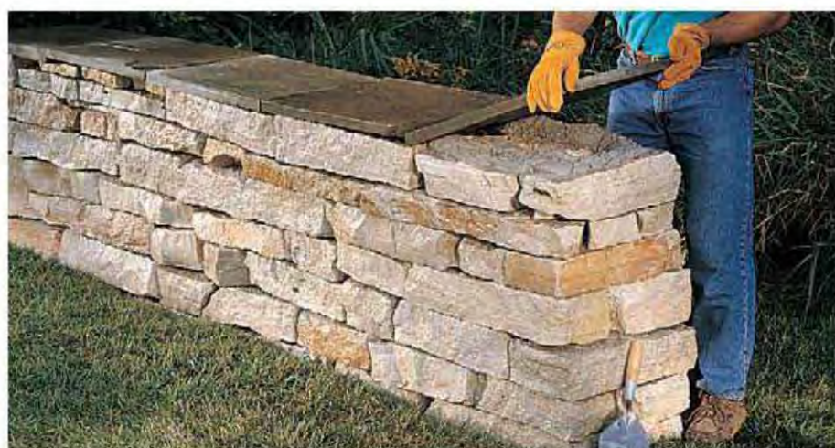
E. Once all the courses are in place, mortar the capstones to the top course of stone, then seal all the gaps between them.
