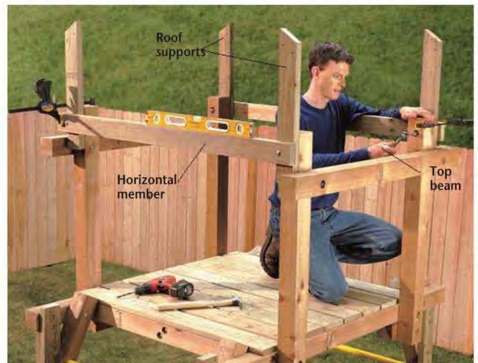
G. Attach the top beams to the posts with 7" carriage bolts. Also attach the horizontal members and roof supports in place using 6\frac{1}{2} " carriage bolts.
