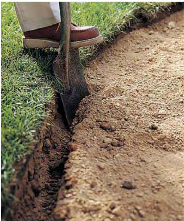
A. Dig narrow trenches for the edging on both sides of the excavated path site. Check the depth with a brick paver.
