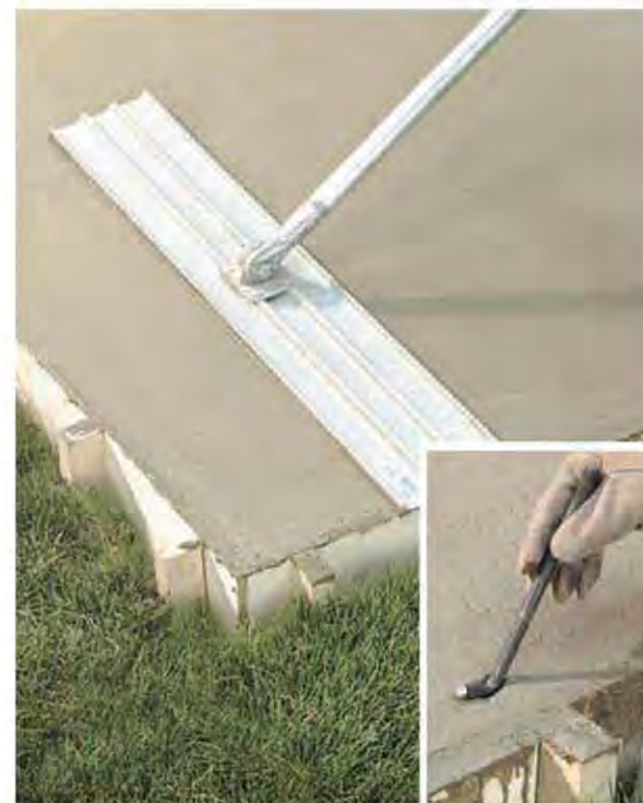
F. Float the slab with a bull float, then set the J-bolts at the marked locations (INSET).
