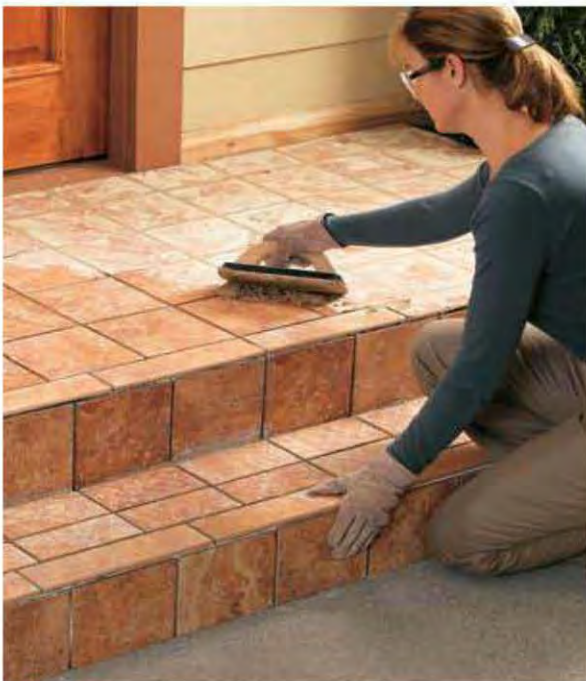
22. Apply grout in the gaps between tiles using a grout float. Wipe away the grout after it clouds over. Cover with plastic in the event of rain.
