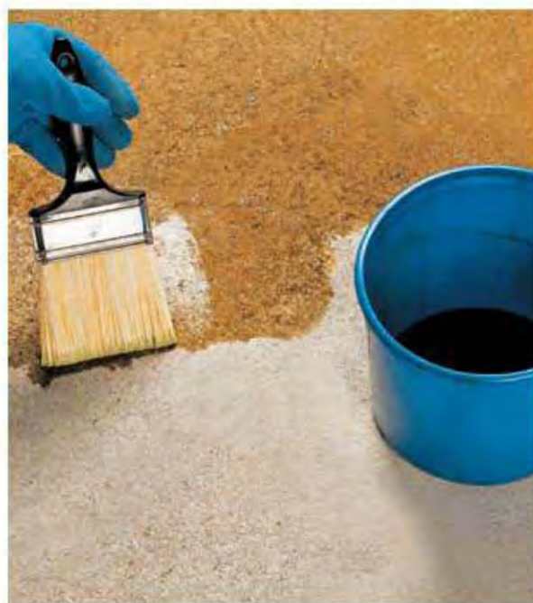
1. Use a paintbrush to apply stain using long, even strokes. Minimize brush strokes.
