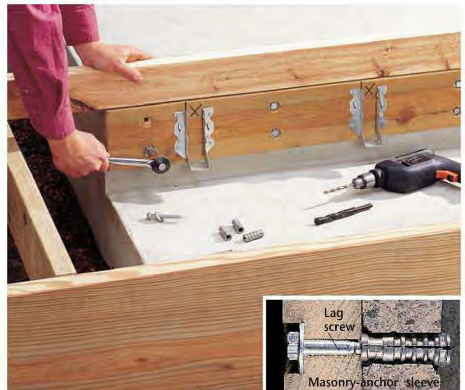
E. To install the step ledger, drill \frac{3}{8} "-dia. holes into the top riser of the steps and install masonry-anchor sleeves (INSET). Fasten the ledger to the riser with \frac{3}{8} \times 4 " lag screws.
