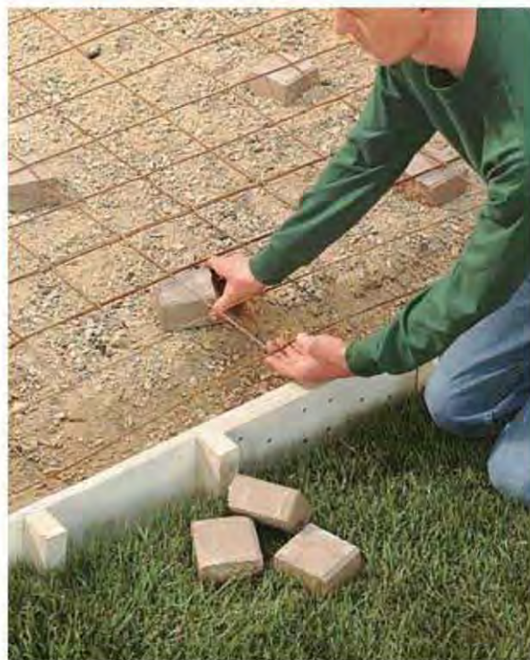
D. Lay out rows of wire mesh, tie the rows together, then prop up the mesh with brick pavers or metal bolsters.
