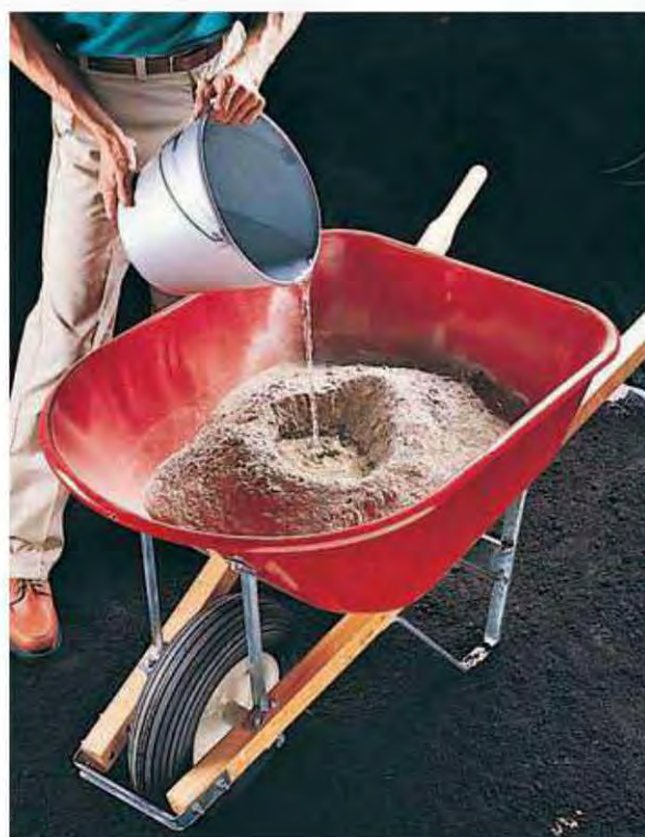
7. Form a hollow in center of dry concrete mixture. Slowly pour a small amount of water into hollow, and blend in dry mixture with a hoe.
