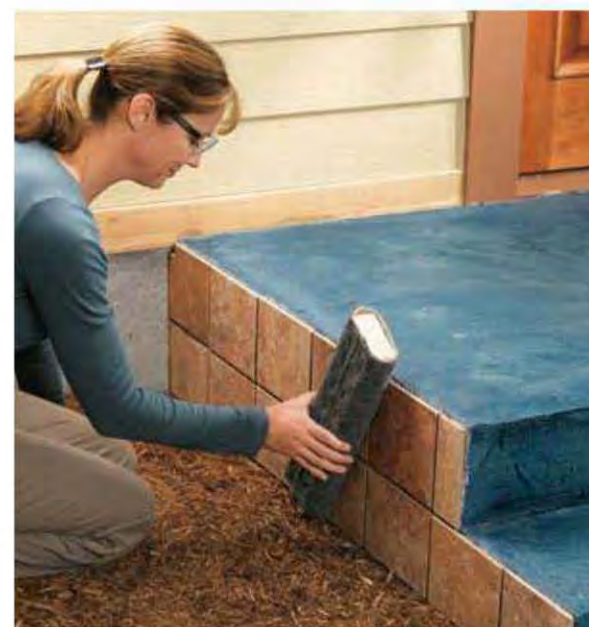
10. Wrap a 2 × 4 in old carpet and drag it back and forth across the tile surfaces to set them evenly. Don't get too aggressive here—you don't want to dislodge all of the thinset mortar.
