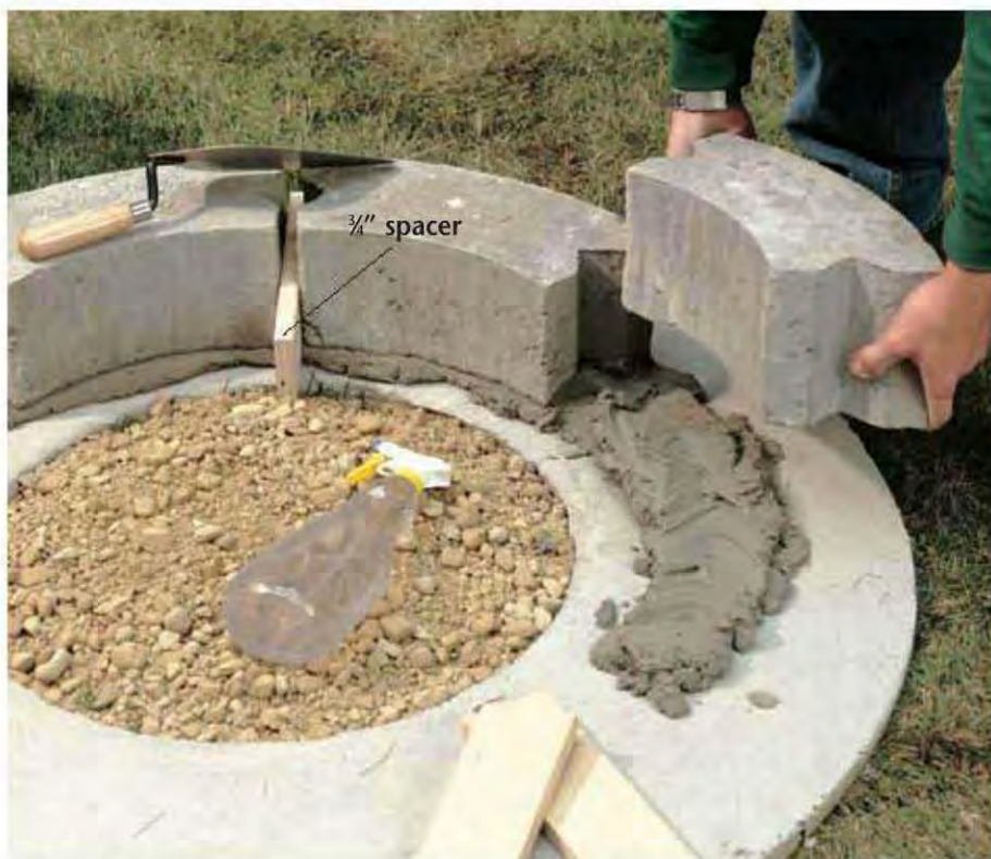
C. Mist the footing with water and spread a bed of mortar inside the reference lines. Place the blocks of the first course in position, with three \frac{3}{4} " spacers in the course to create air vents.
