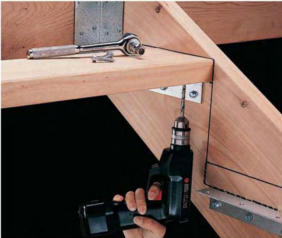
11. Drill \frac{1}{8} " pilot holes, then attach the front 2 \times 6 to the cleats with \frac{1}{4} \times 1\frac{1}{4} " lag screws.
