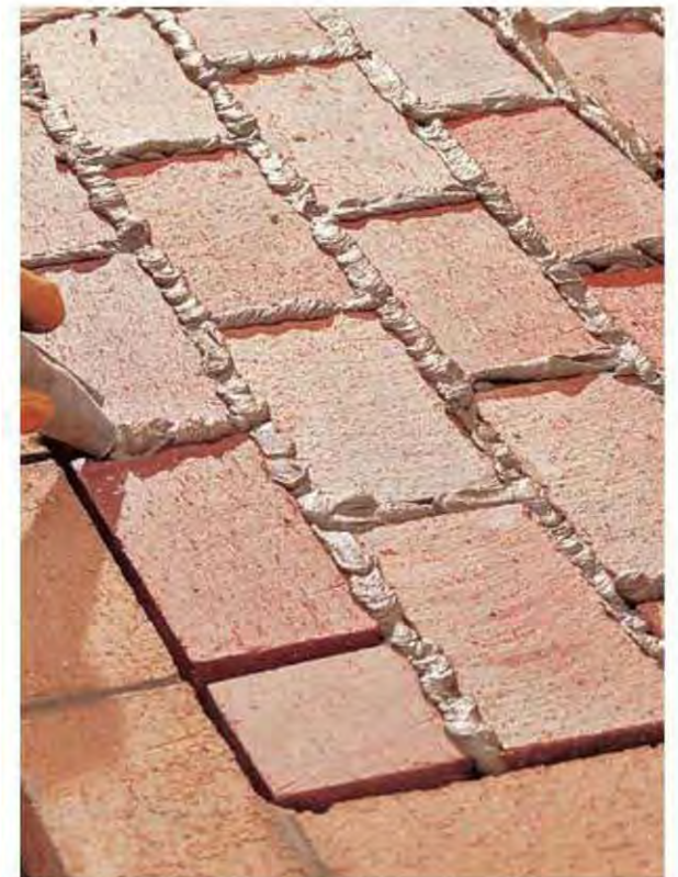
D. Use a mortar bag to fill mortar joints between pavers. Smooth with a jointing tool, making sure the joints are even with the tops of the pavers.
