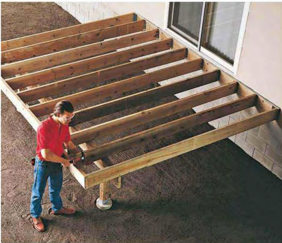
4. Install metal joist hangers on the ledger and header joist, then hang the remaining joists (page 204). Most decking patterns require joists that are spaced 16" on center.
