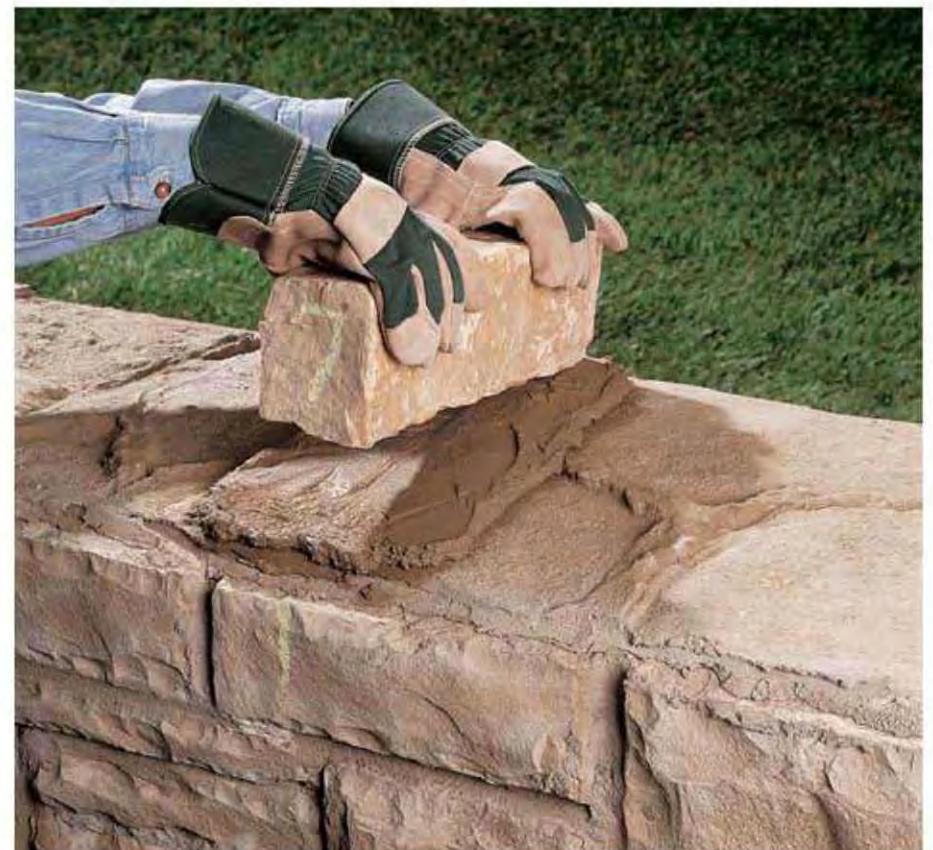
B. Set the first stone in a \frac{1}{2} "-thick mortar bed at the base of the window circle.
