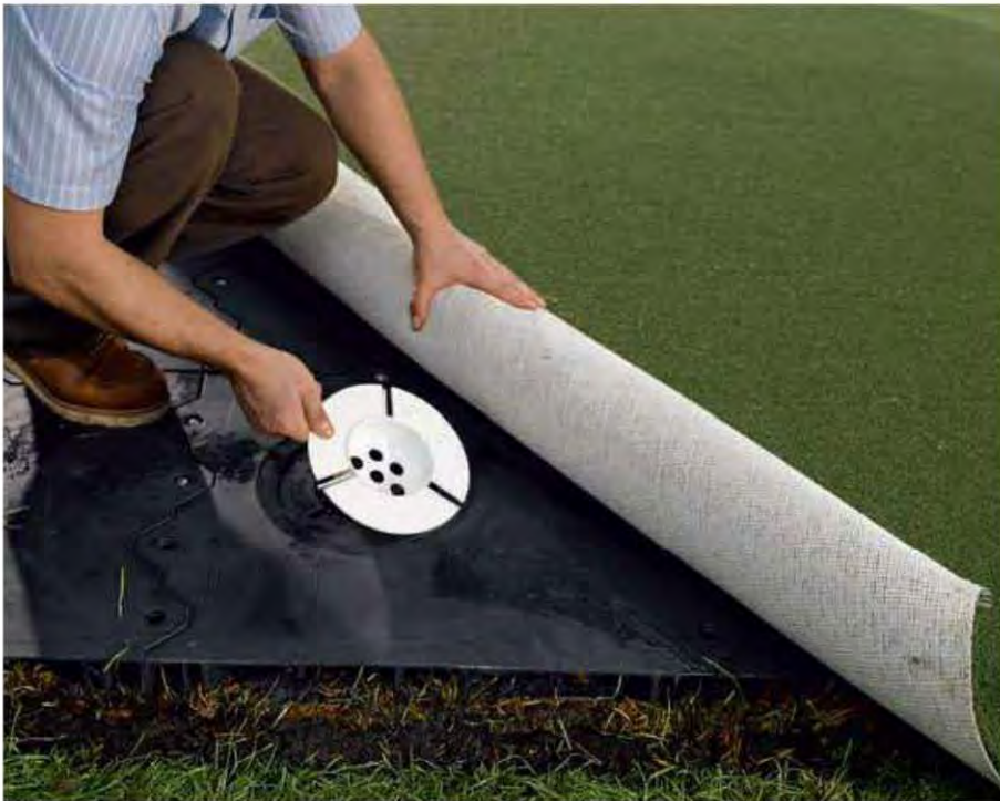
13. Install the cups into the panels containing the cup bodies, and then cut holes in the turf with a utility knife.
