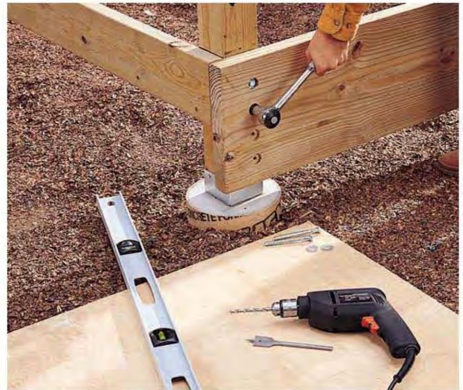
D. Tack the rim joist in position, drill four counterbored pilot holes, and fasten to the post with \frac{3}{8} \times 4 " lag screws with washers.
