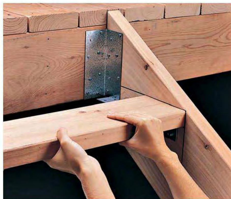
10. For each step, position the front 2 x 6 on the tread cleat, so that the front edge is flush with the tread outline on the stringers.
