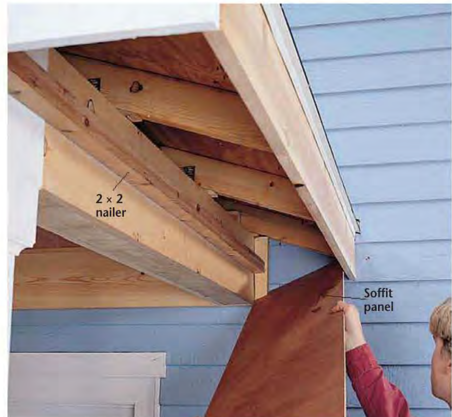
B. Insert one edge of the soffit panel in the plowed groove and place the other end against the nailer. Fasten with 4d galvanized box nails.
