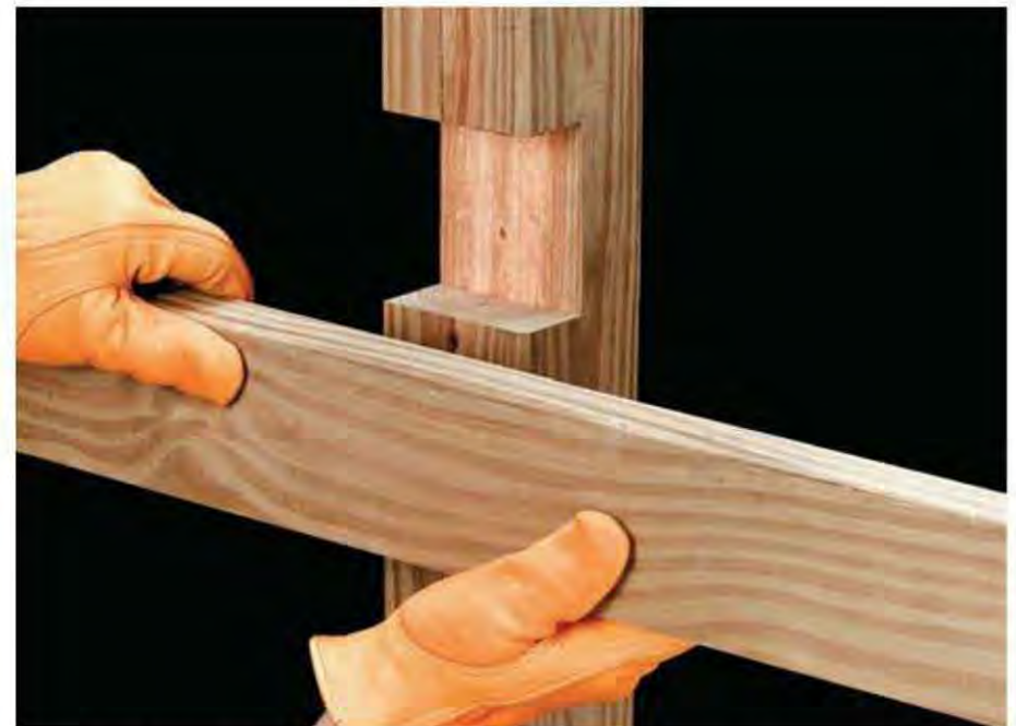
Cut and install railings into notches cut into the inner faces of the railing posts.
