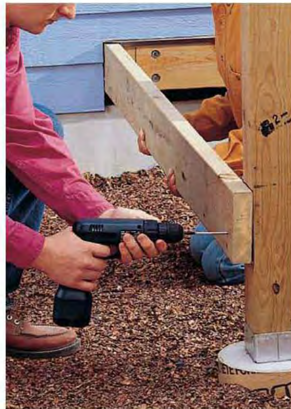
B. Cut the outer joists to size, drill pilot holes, and fasten to the post with 3" galvanized deck screws.
