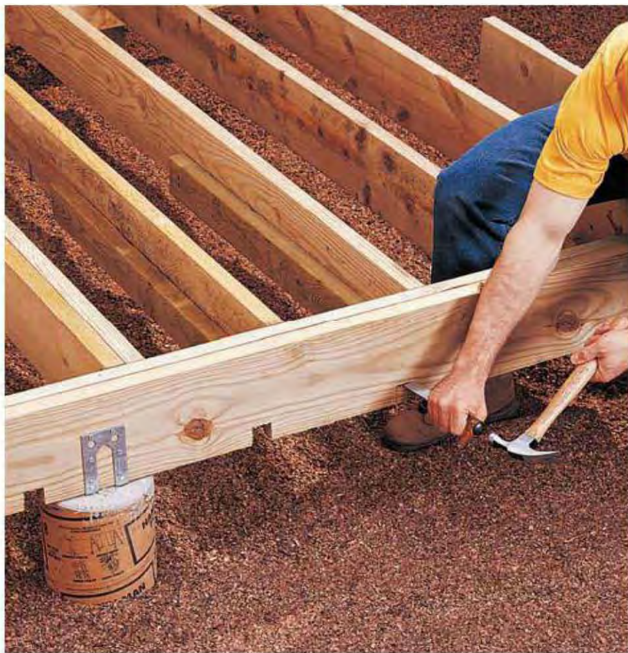
E. Cut notches for the step supports in the outer beam with a reciprocating saw or handsaw. Finish the notches with a hammer and chisel.
