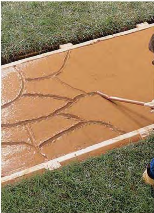
B. Cut shallow lines in the concrete, using a jointing tool or a curved copper pipe.
