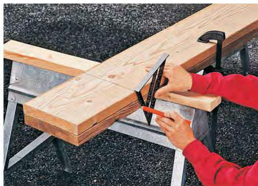
Use a speed square to mark a 22\frac{1}{2}^\circ miter cut where the ends of beams C-3 and C-4 fit together.
