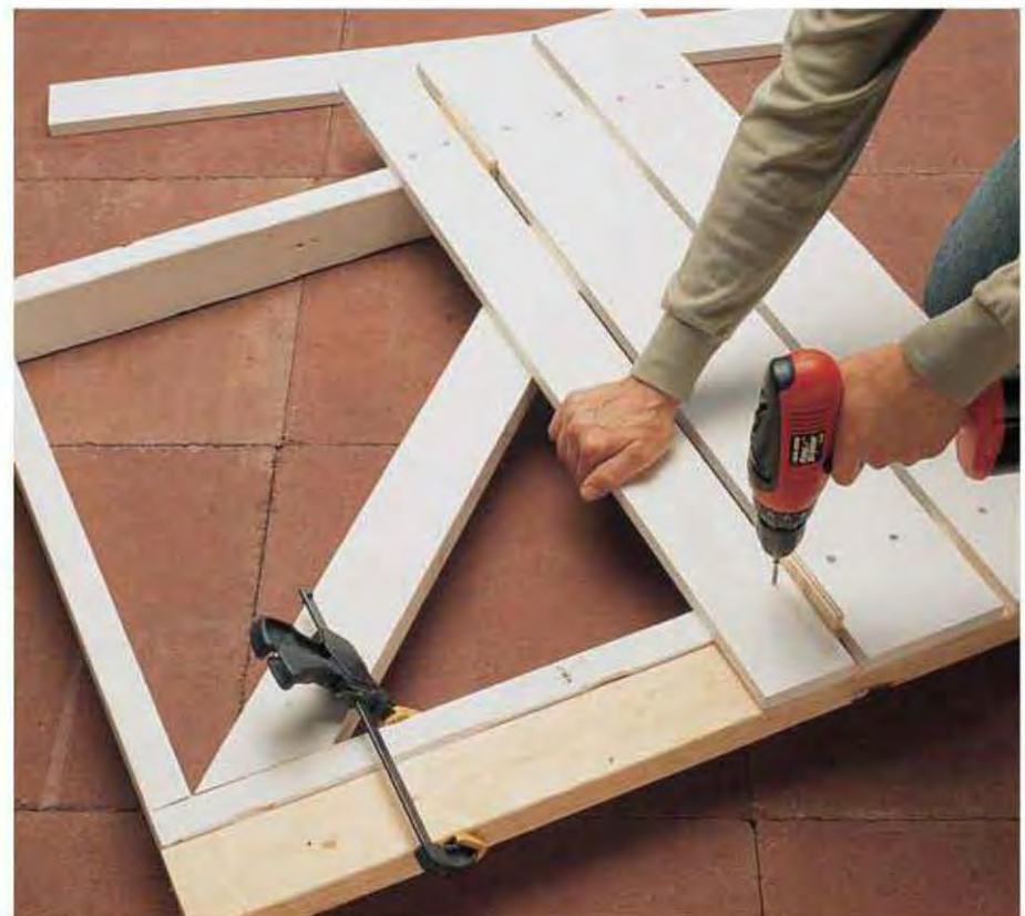
H. Clamp a 2 × 4 across the bottom of the gate frame as a guide, then attach the siding. Begin with two 1 × 6s on the hinge side, then finish with 1 × 4s. Use scraps of ⅝" plywood as spacers.
