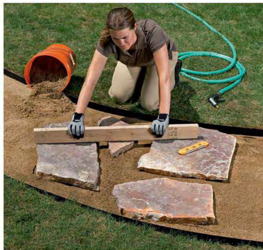
2. Level the stones by adding and removing sand until they are solidly seated. On flat runs, you should be able to rest a flat 2 × 4 on three stones at once, making solid contact with each. It is much easier to pack sand under stones if you moisten the sand first. Also moisten the sand bed to prevent sand from drifting.
