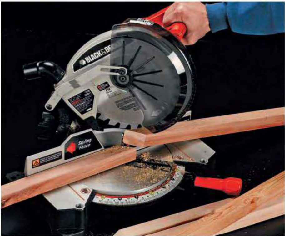
2. Measure and cut balusters for main deck using a power miter saw or circular saw. Cut off tops of the balusters square and cut bottoms at 45° angle. Seal cut ends of lumber with clear sealer-preservative.
