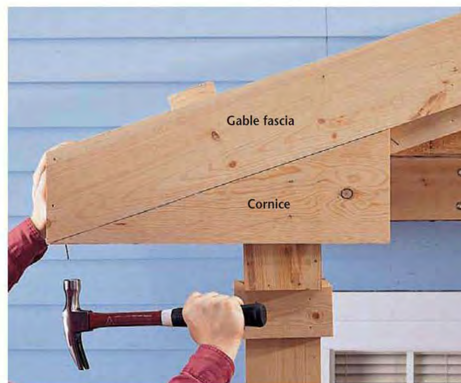
B. Attach the cornice pieces to the ends of the wrapped beams with 8d finish nails and to the bottom edge of the fascia with 4d finish nails.
