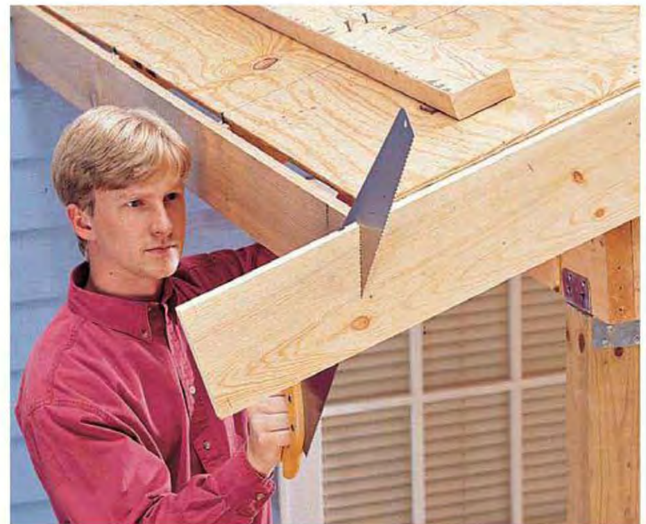
D. Cut side fascia boards to fit between the house and the back faces of the gable-end fascia, then trim off the gable-end fascia boards with a handsaw.
