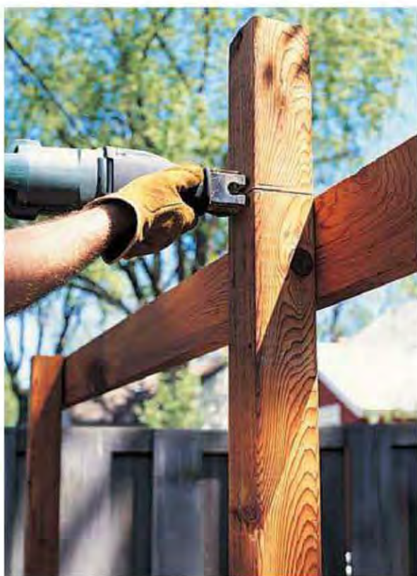
D. Attach the other tie beam and trim the tops of the posts flush with the tie beams.
