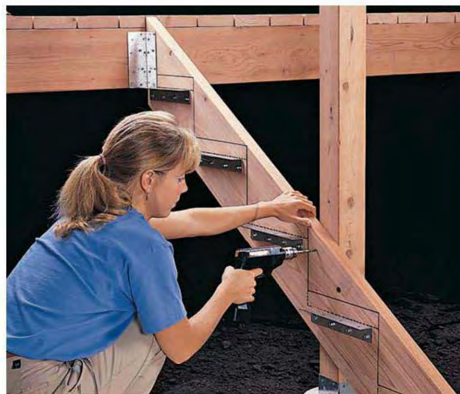
8. Drill two \frac{1}{4} " pilot holes through each stringer and into each adjacent post. Counterbore each hole to depth of \frac{1}{2} " using a 1" spade bit. Attach stringers to posts with \frac{3}{8} x 4" lag screws and washers using a ratchet wrench or impact driver. Seal screw heads with silicone caulk.
