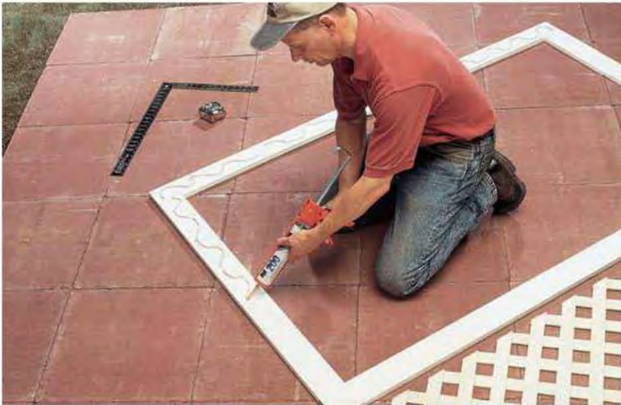
D. Set up the pieces of the back frame, butting the joints. Square the frame, then apply a bead of construction adhesive along the center of the frame. Carefully set the lattice panel in place.
