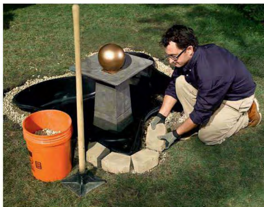
10. Set interlocking pavers in place around lip of liner. Adjust compactable gravel as necessary to make the pavers level.
