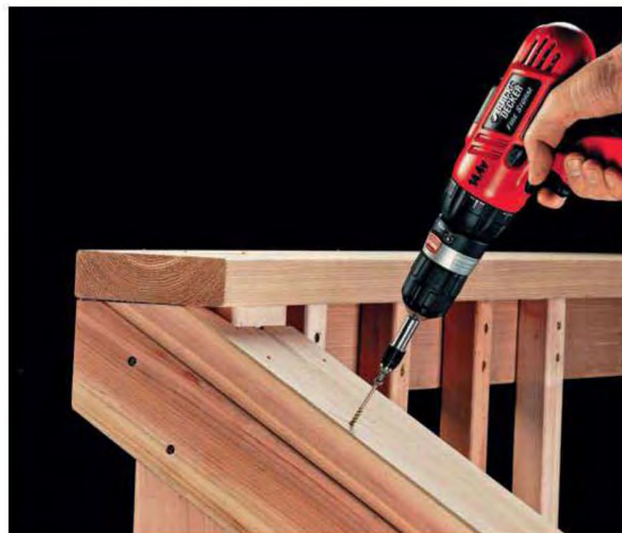
29. Position cap over the stairway rail and balusters so that edge of cap is flush with inside edge of rail. Drill \frac{1}{8} " pilot holes and attach cap to rail with 2½" deck screws driven every 12". Also drive screws through cap into stair post and into every third baluster.
