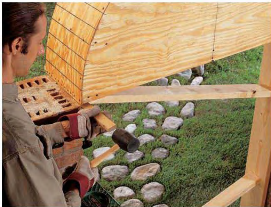
B. Cut two 2 × 8 braces, ½" shorter than pillar height, and prop one against each pillar with 2 × 4 cross braces.
