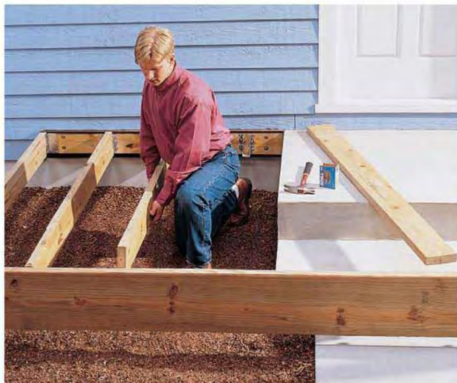
B. Build the porch deck frame, then install metal joist hangers on the ledger and rim joist, and install the remaining joists (pages 320 to 321).
