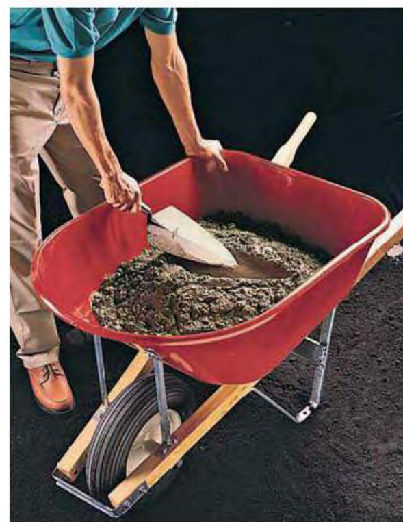
8. Add more water gradually, mixing thoroughly until concrete is firm enough to hold its shape when sliced with a trowel.
