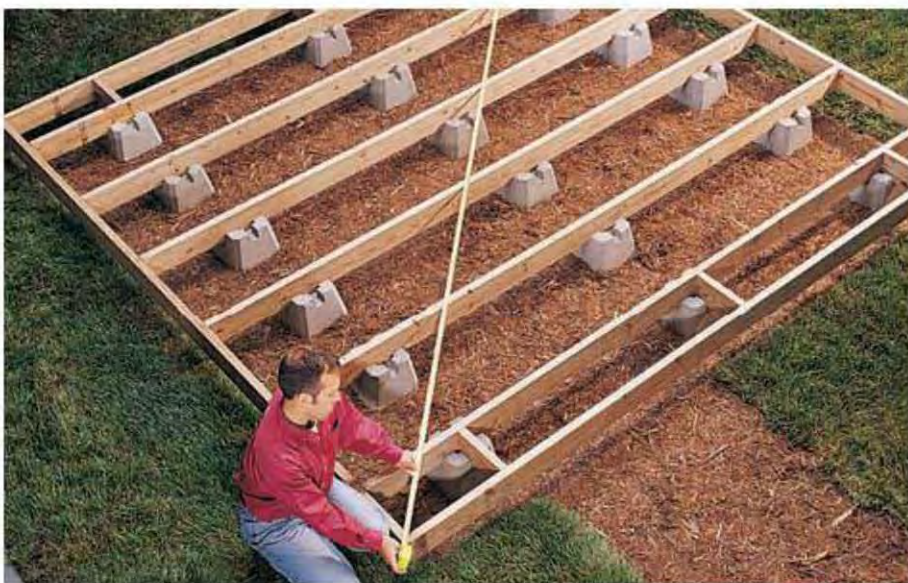
After the framing is completed, measure the diagonals and adjust the frame until it's square.
