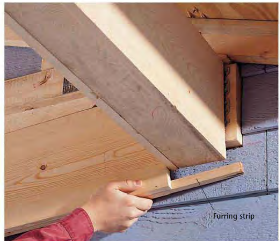
E. Cover the ledger with a 1 × 10 using furring strips to fill the gap between the bottom of the ledger and the wrapped beam.
