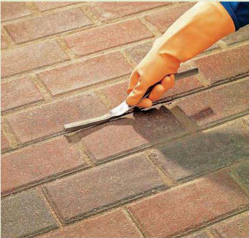
After the mortar has been packed into the joints and wetted, finish the joints with a jointing tool.
