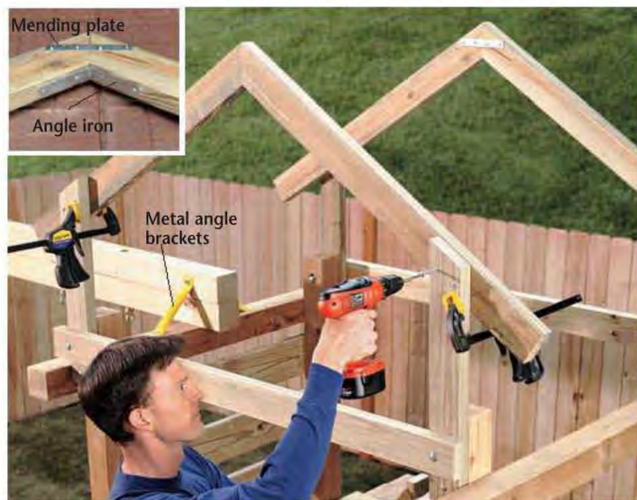
L. Cut the ends of the rafters at 45° angles, butt the ends together, and secure the joint with an angle iron and a mending plate (INSET). Align the rafter assembly with the roof supports, and secure with deck screws.
