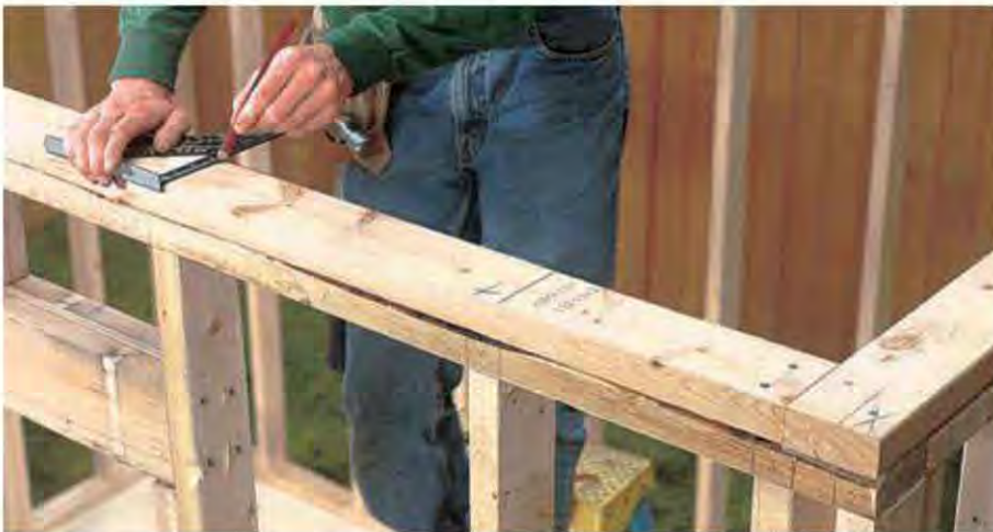
E. Mark the rafter layout onto the wall plates and the ridge board, starting from the same end of the building for each.
