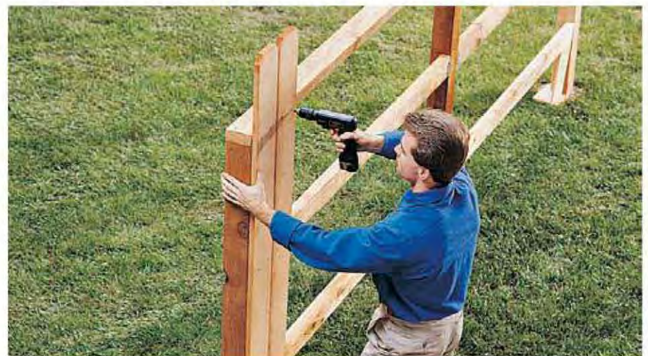
C. Measure and cut the siding to size. Attach the siding to the framework, spacing them at least 1/8" apart.
