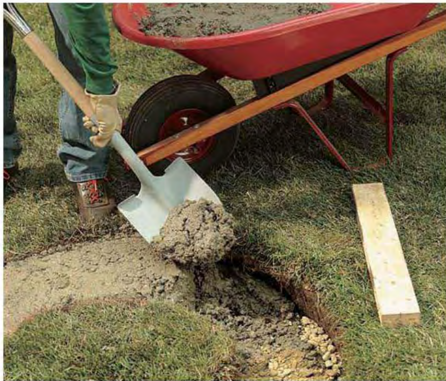
B. After tamping a 2" layer of compactable gravel in the bottom of the trench, fill with concrete and screed it with a scrap of 2 × 4. Float the surface with a trowel.
