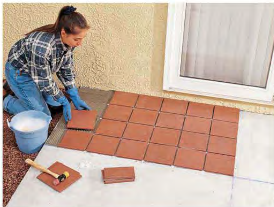
H. Set tiles into the field area of the first quadrant, saving any cut tiles for last. Cut tile using a wet saw or a tile cutter. For curved cuts, use tile nippers.
