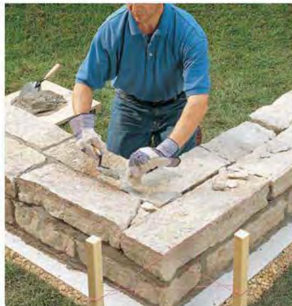
C. Add courses, staggering the vertical joint. Fill between the two sides of the courses with smaller stones and mortar.
