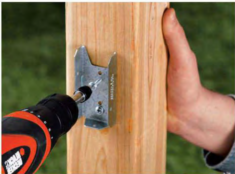
5. Attach three evenly spaced and centered fence brackets to the first post and trim fence post to desired height.
