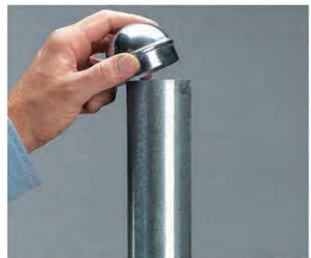
4. Top each terminal post with a post cap and each line post with a loop cap. Make sure the loop cap openings are perpendicular to the fence line, with the offset side facing the outside of the fence line.
