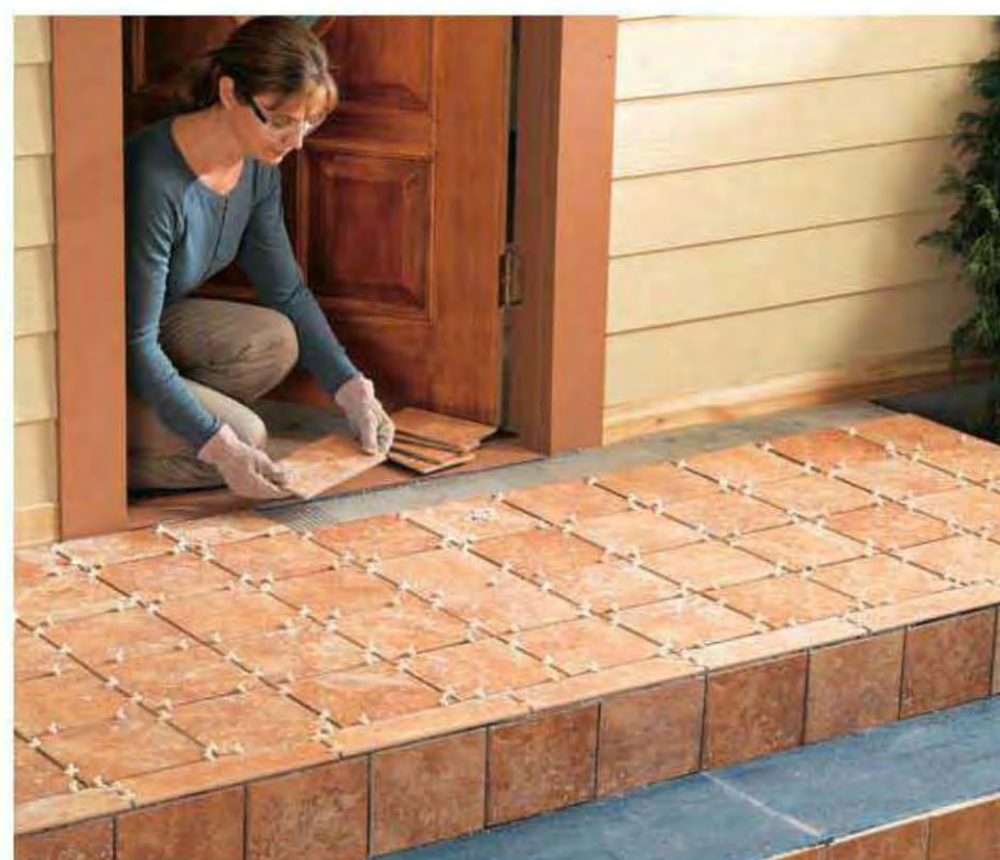
19. Add the last row of tiles next to the house and threshold, cutting them as needed so they are between \frac{1}{4} and \frac{1}{2} " away from the house.
