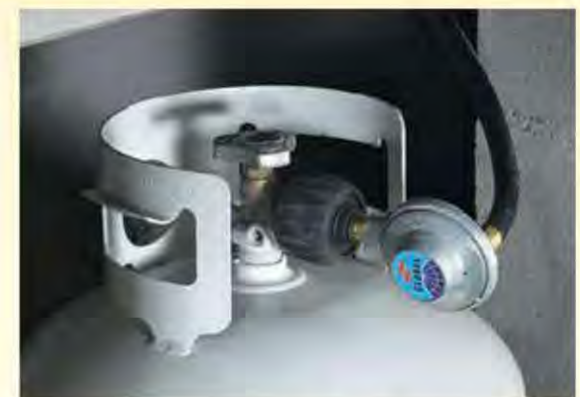
A grill gas line typically extends up into the cabinet space under the grill and is fitted with a shutoff valve.
