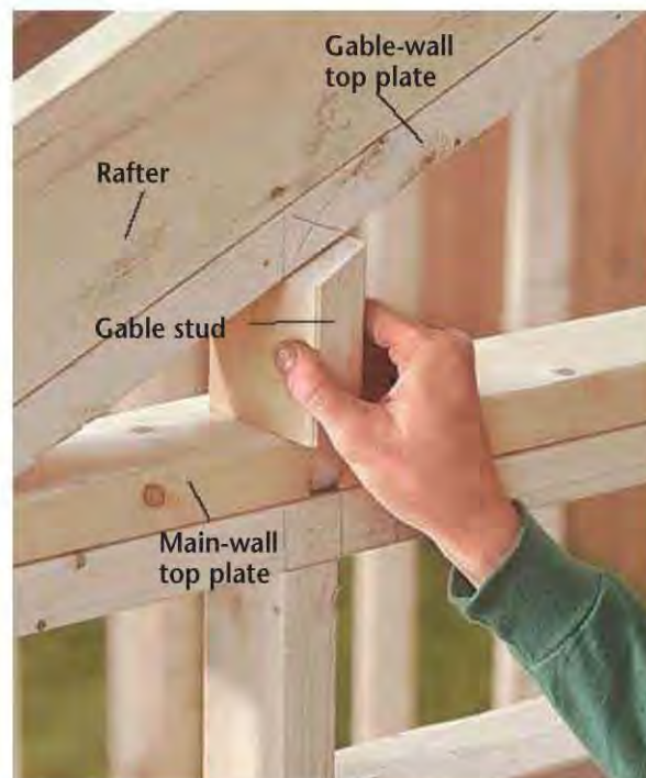
H. Mark the gable stud layout onto the main-wall top plate and gable-wall top plate, then install the gable studs.
