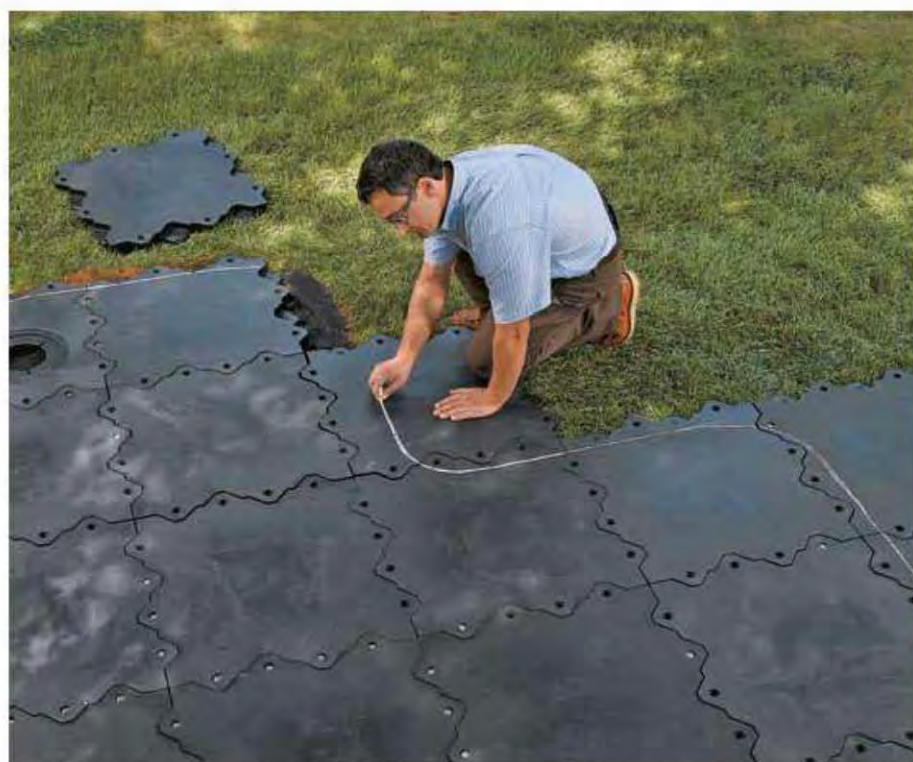
9. Where panels go beyond the outline, use a light-colored crayon or chalk to mark a cutting line. Avoid cutting extremely close to panel edges.
