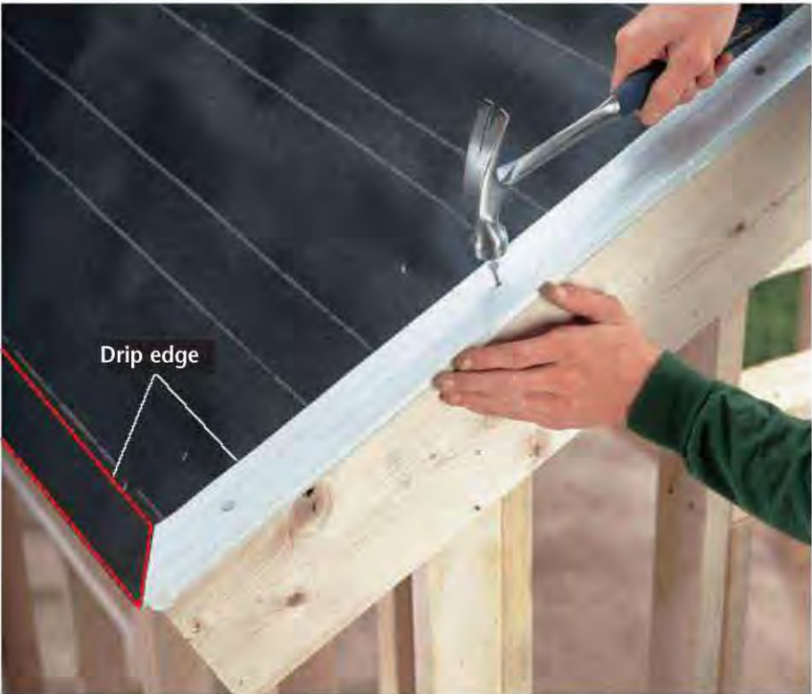
A. Install drip edge along the eaves over the sheathing. Add the building paper, then install drip edge along the gable ends.
