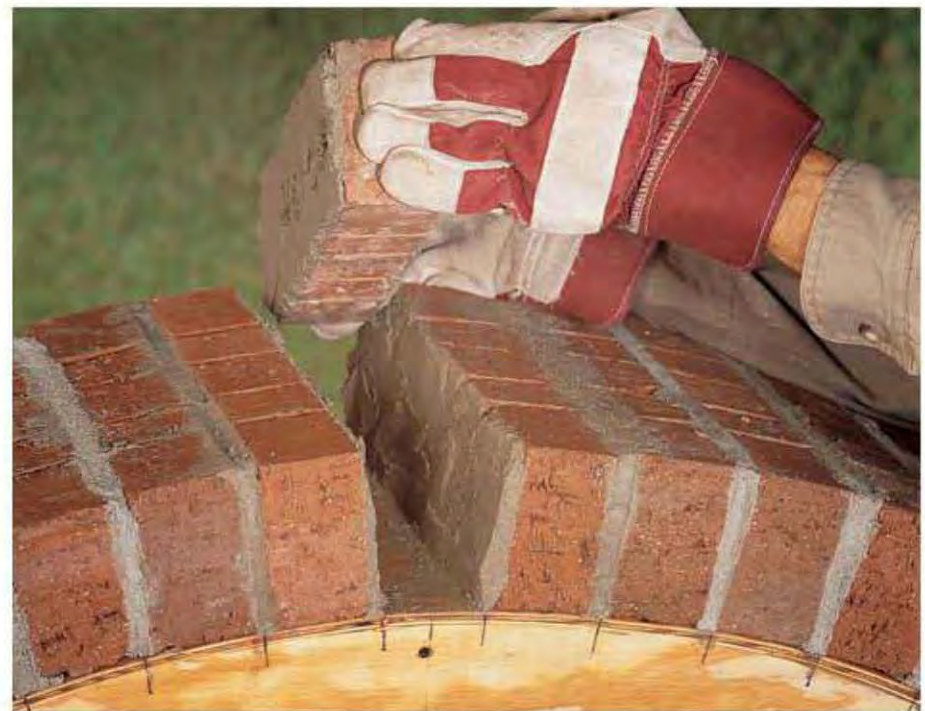
D. Butter the center, or keystone, brick as accurately as possible and ease it into place. Smooth the remaining joints with a jointing tool.
