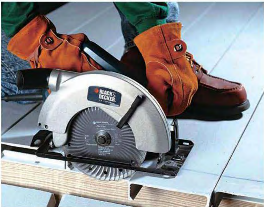
3. Cut the overhanging ends of the decking boards flush with the outside joists using a circular saw with a fresh carbide-tipped blade or a masonry cut-off disc.
