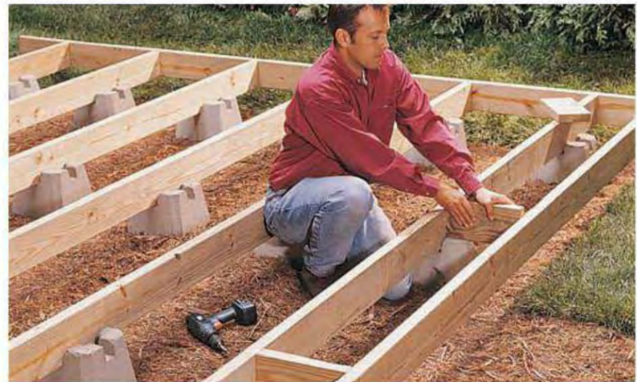
Position the sleepers in the slots of the footings, then attach them to both joists with pairs of deck screws.
