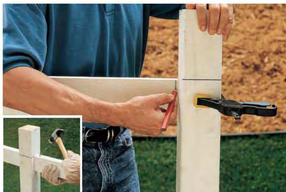
C. Mark the stringer position on the posts, then scribe and cut the stringer to size. Toenail the stringer in place (INSET).
