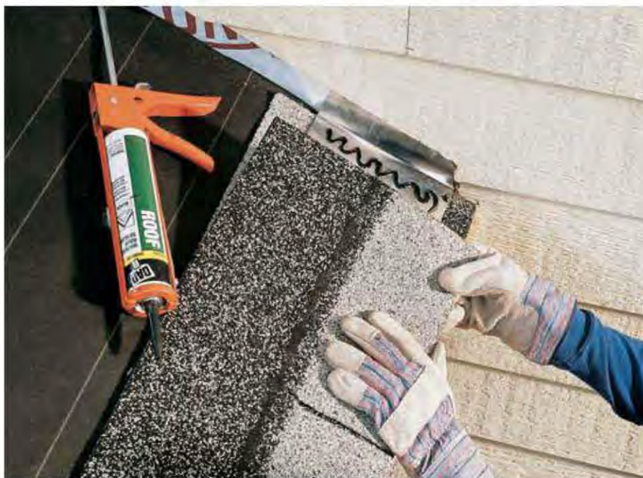
D. Apply roofing cement to the flashing, then press the shingle into it. Do not nail through the flashing when attaching the shingle.
