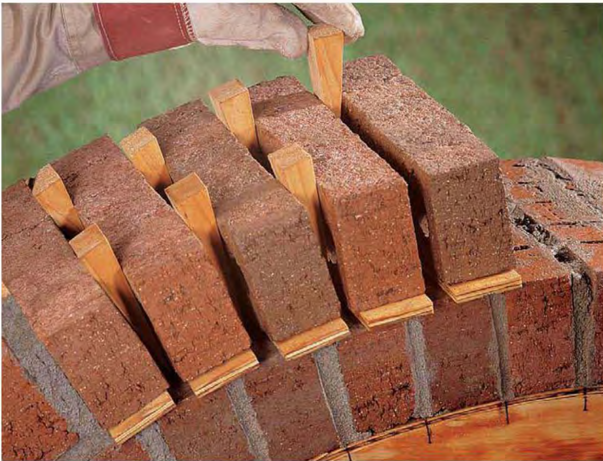
E. Lay the second course halfway up each side of the area. Dry-lay several more bricks on one side—using shims as substitutes for mortar joints—to check the amount of space remaining. Remove the shims and lay the final bricks.
