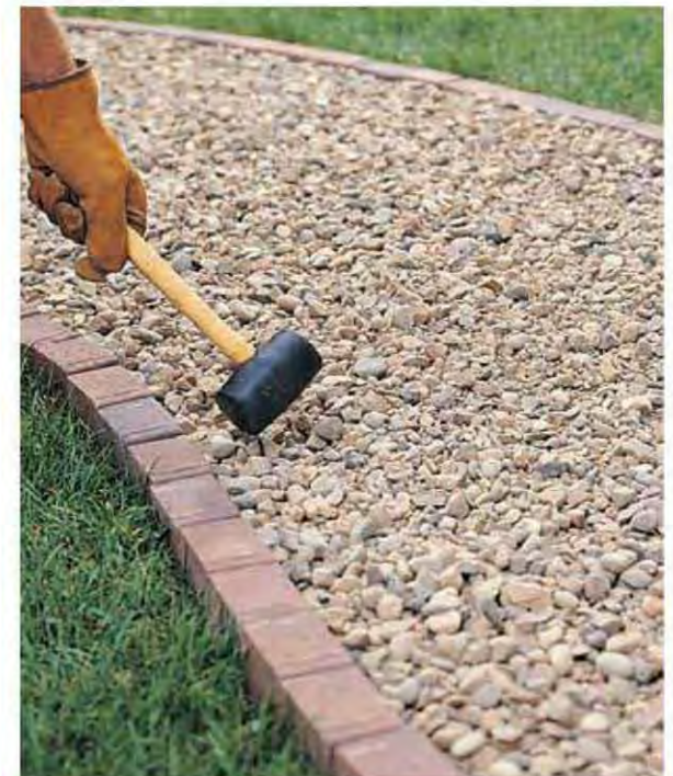
D. Fill the pathways with loose-fill material. Tap the inside face of each brick paver with a mallet to help set them permanently in the ground.
