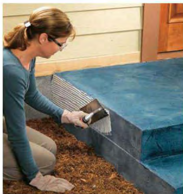
8. Mix a batch of thinset mortar with latex bonding adhesive and trowel it onto the sides of the steps, trying to retain visibility of the layout lines. Because the top steps are likely more visible than the bottom steps, start on top and work your way down.
