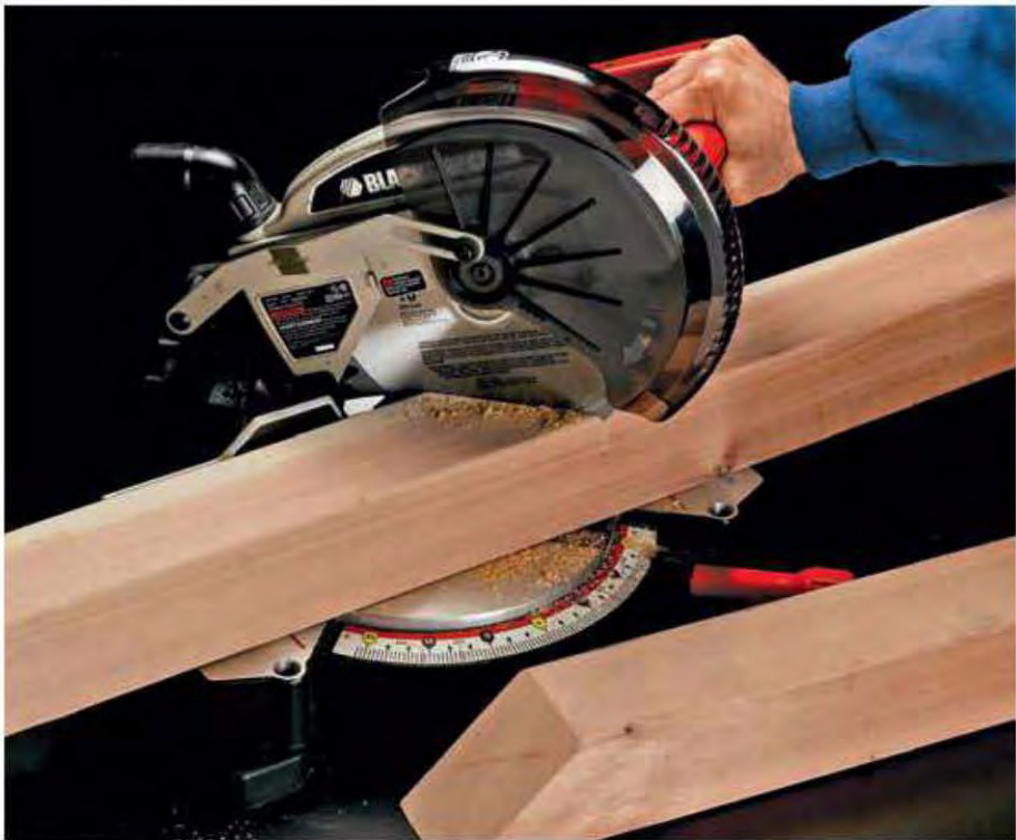
1. Measure and cut 4 × 4 posts using a power miter saw or circular saw. Cut off tops of the posts square and cut the bottoms at 45° angle. Seal cut ends of lumber with clear sealer-preservative.
