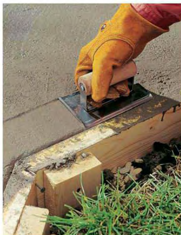
10. Shape the edges of the concrete by running an edger along the forms. Smooth out any marks created by the edger using a float. Lift the leading edge of the edger and float slightly as you work.
