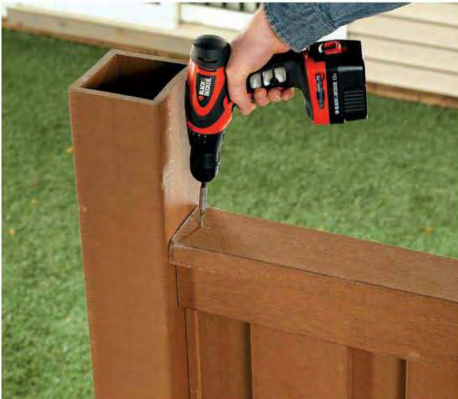
13. From above, screw the top rail to each bracket with a rail-to-bracket screw.
