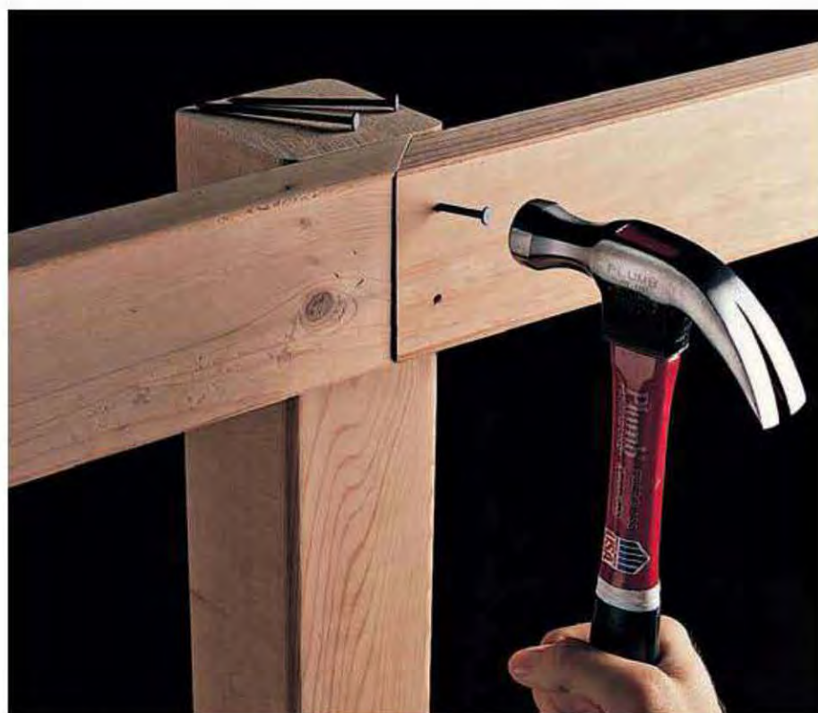
10. Join 2 × 4s for long rails by cutting ends at 45° angles. Drill 1/16" pilot holes to prevent nails from splitting end grain and attach rails with 10d galvanized nails. (Screws may split mitered ends.)
