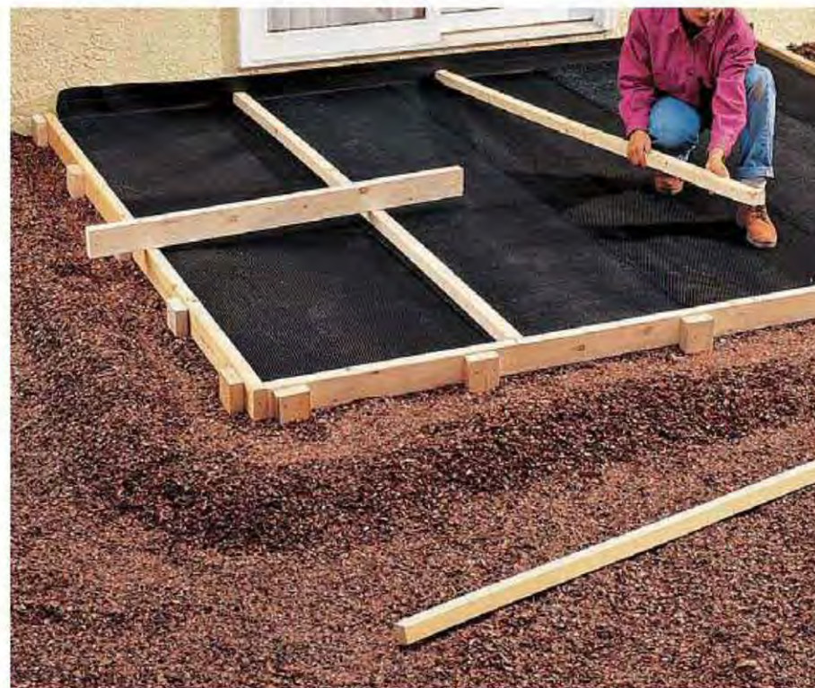
B. Build temporary 2 × 2 forms to divide the project into working sections. The forms also provide rests for the screed board used to level and smooth the fresh concrete.
