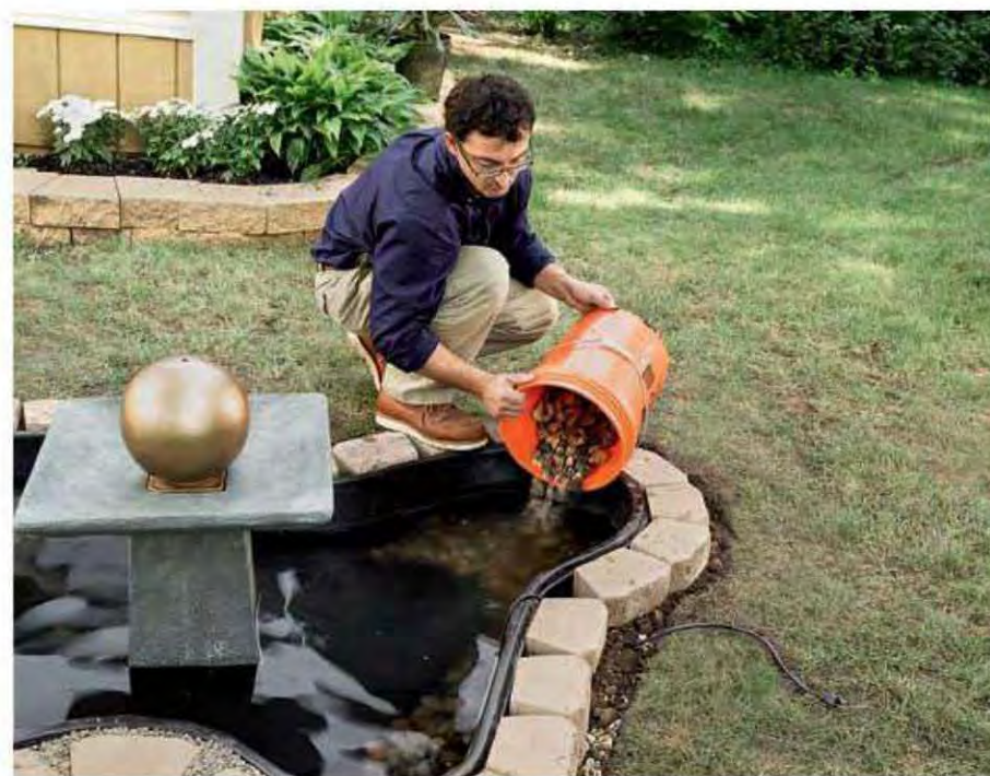
12. Remove the tarp from the pond and cover the bottom of the liner with washed river rock. Place the fountain onto the pedestal and submerge the cord, running it out of the pond in an inconspicuous spot, such as between two pavers.
