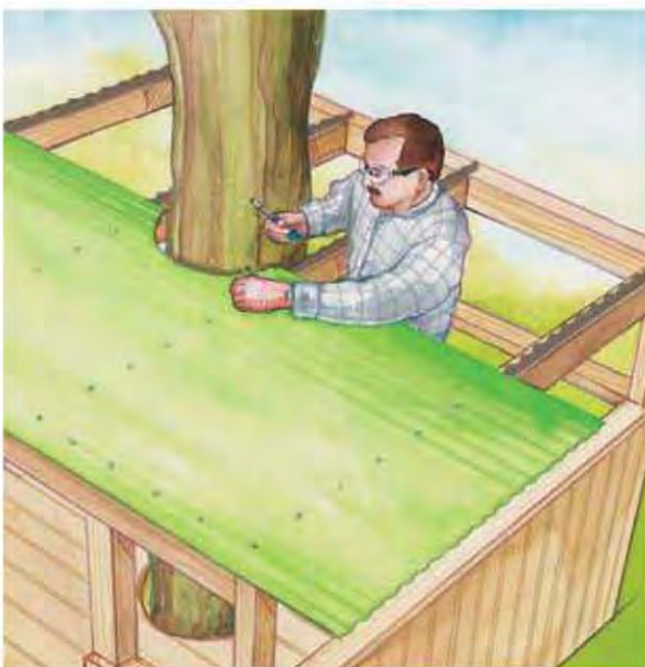
J. Cut the roof panel to fit around the tree, then set the panel in place over the first panel, drill pilot holes, and fasten the panel to the beams and rafters.
