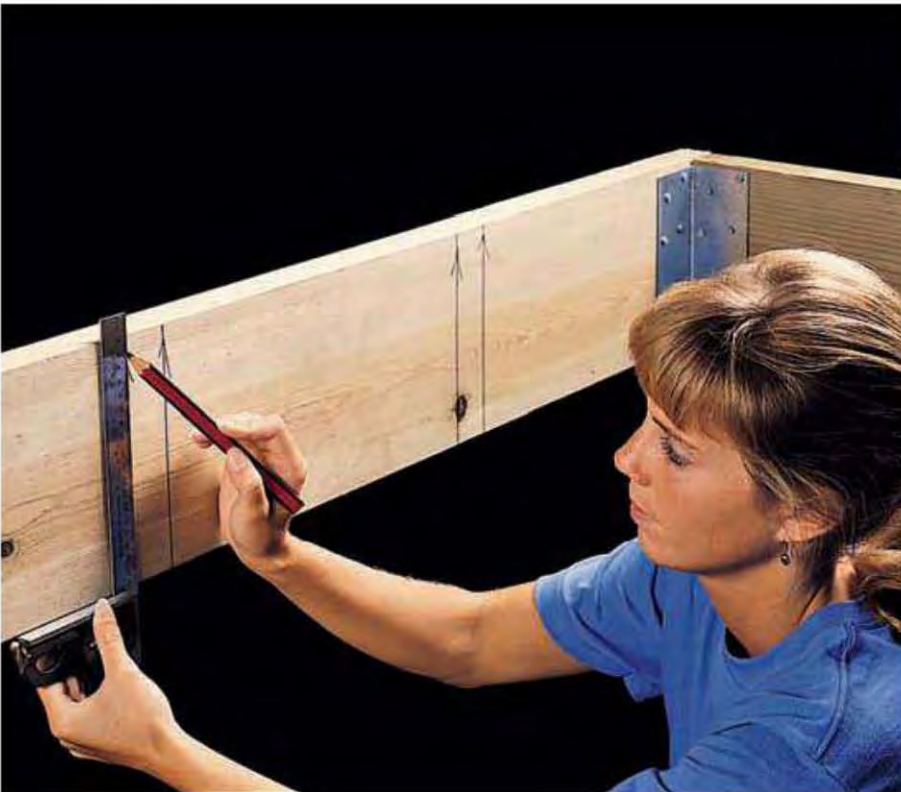
10. Measure along the header joist from the outside joist, and mark where joists will be attached to header joist. Draw the outlines on the inside of the header using a combination square as a guide.
