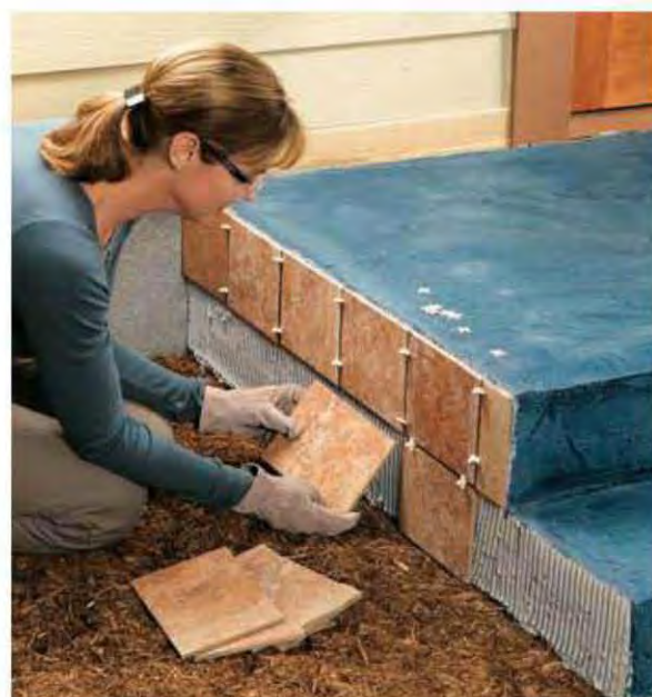
9. Begin setting tiles into the thinset mortar on the sides of the steps. Start at the top and work your way downward. Try to lay out tile so the vertical gaps between tiles align. Use spacers if you need to.
