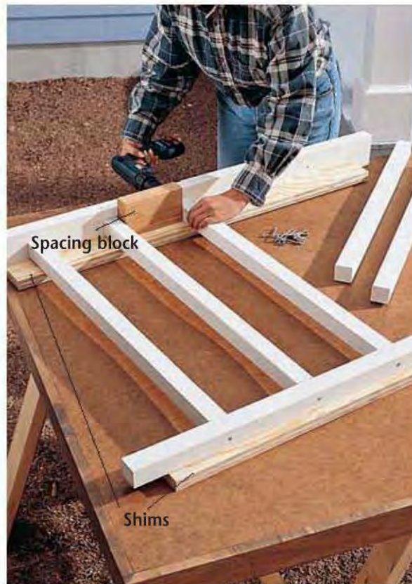
D. Support the balusters and top rail with shims. Use a spacer block to align the balusters with the pilot holes, and fasten with 2½" deck screws.
