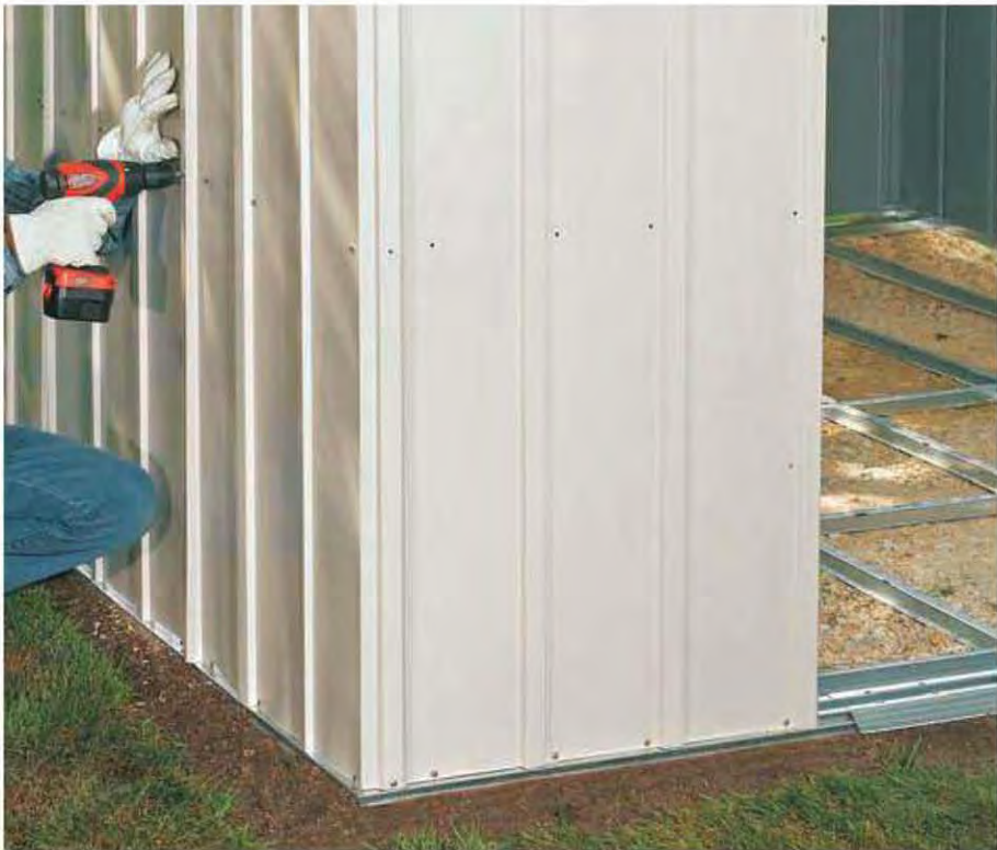
11. Fill in the wall panels between the completed corners, attaching them to the frames with the provided fasteners. Take care not to overdrive the fasteners.
