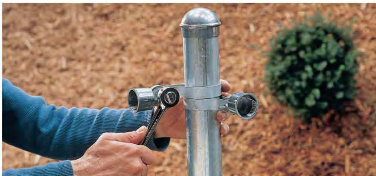
3. For a corner, place two brace bands 3" from the top of the post. Attach stringer ends with the angle side up to the upper brace band and the angle side down to the lower band.
