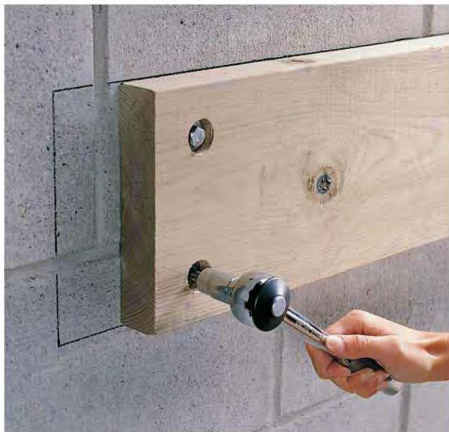
A. Attach the ledger to the wall with lag screws and washers using a ratchet wrench.
