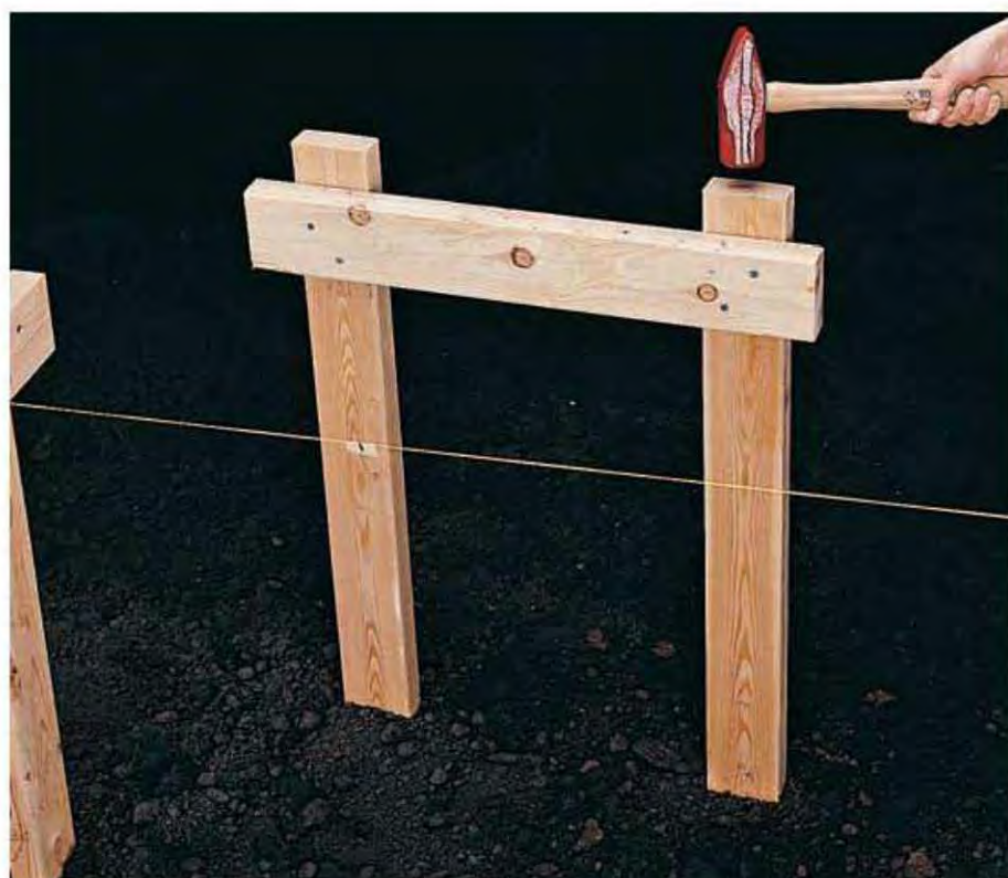
14. Drive additional batter boards into ground, about 2 feet outside mason's strings and lined up with post centerpoint marks (step 13).
