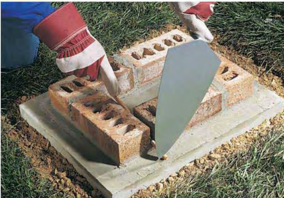
B. Trowel a bed of mortar inside the reference lines and lay the first course. Create a weep hole in the mortar with a dowel to ensure the drainage of any moisture that seeps into the pillar.
