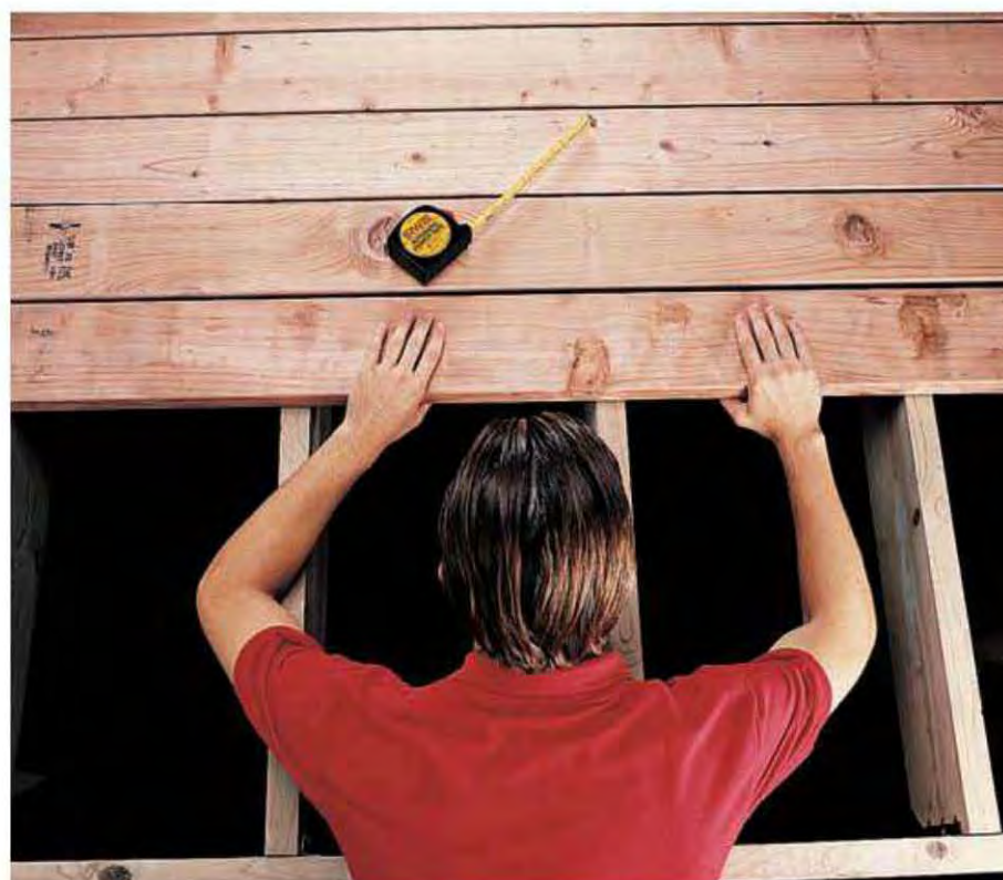
6. Adjust board spacing by changing the gaps between boards by a small amount over three or four rows of boards. Very small spacing changes will not be obvious to the eye.
