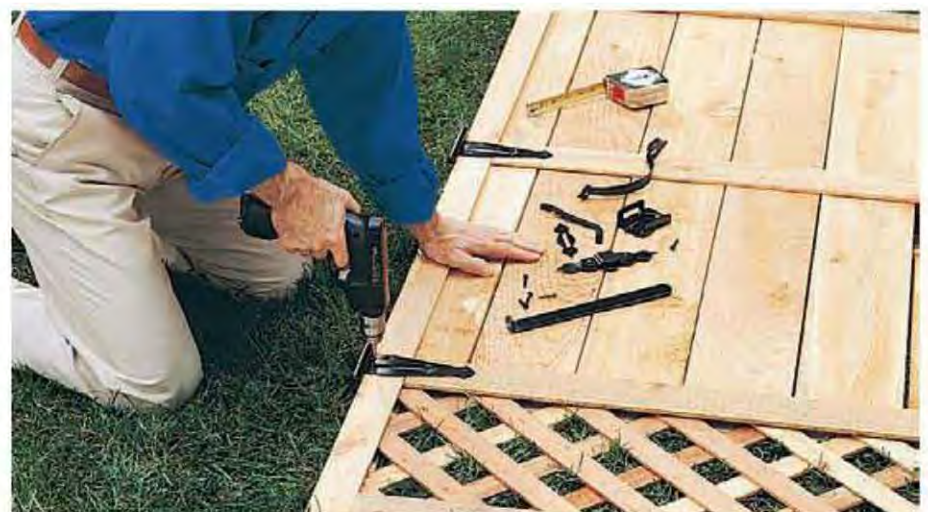
D. Attach the hinges according to the manufacturer's directions, then hang the gate and install the latch hardware.
