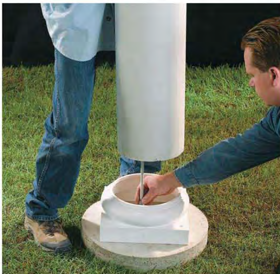
D. Install the columns. Have one person lift up the column while another tightens the coupler nut to the J-bolt and threaded rod.
