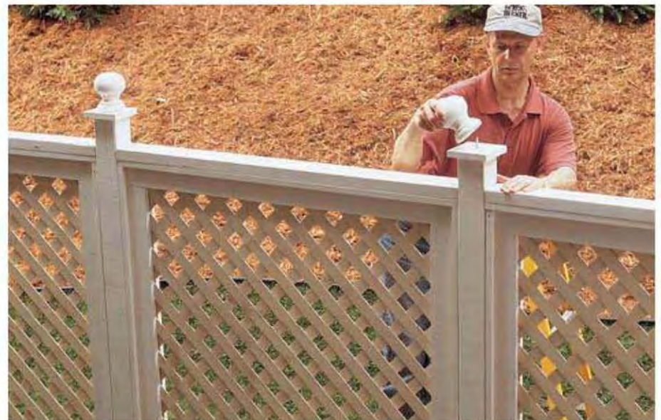
G. Install the remaining panels and add post caps to the posts. Add a deck finial to each post.
