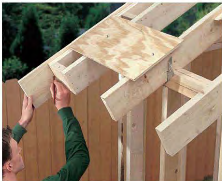
A. Mark the bottom end of the gable fascia by tracing along the end of the rafter (or the subfascia). If the fascia will be installed flush with the sheathing, use a spacer for positioning.
