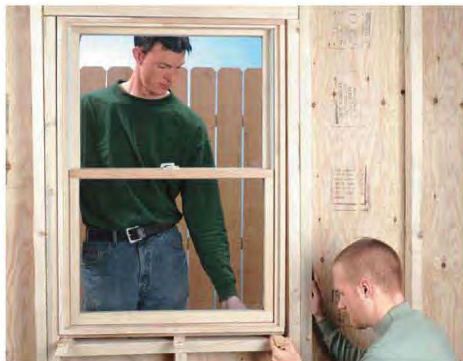
A. Add pairs of tapered shims under the side window jambs and under the center of the sill.
