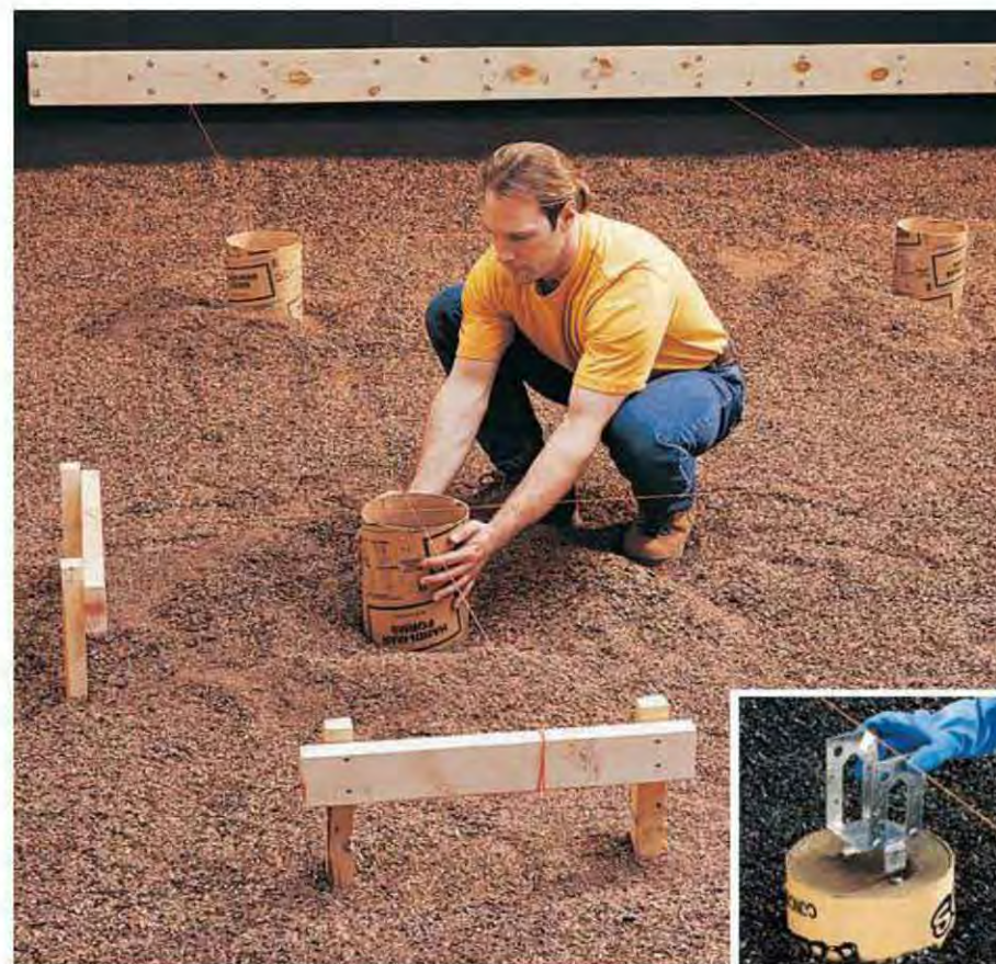
B. Level the footing forms against the mason's strings, pour the concrete, and set the direct-bearing hardware into the wet concrete using the layout strings to ensure accurate alignment (INSET).
