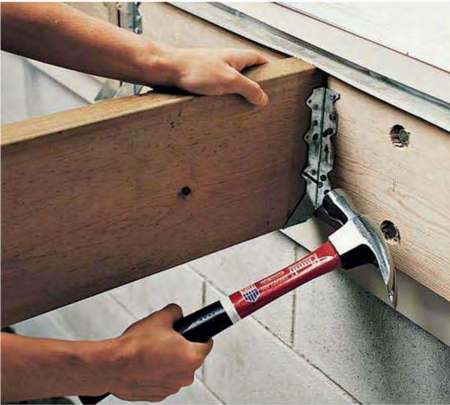
16. Attach the ledger joist hangers to the joists with joist hanger nails. Drive nails into both sides of each joist.
