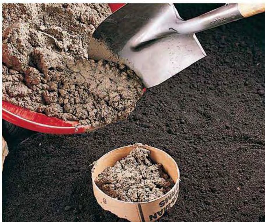
9. Pour concrete slowly into the tube form, guiding concrete from the wheelbarrow with a shovel. Fill about half of the form, using a long stick to tamp the concrete, filling any air gaps in the footing. Then finish pouring and tamping concrete into the form.
