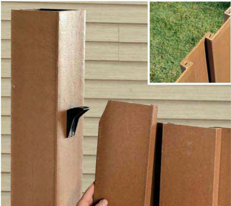
9. Begin installing the interlocking (INSET photo) siding strips. Trim off the corner of the first infill picket in each section in order to avoid upper bracket assembly. Set the siding into the lower stringer channel and secure the first strip to its post with screws provided by the manufacturer.
