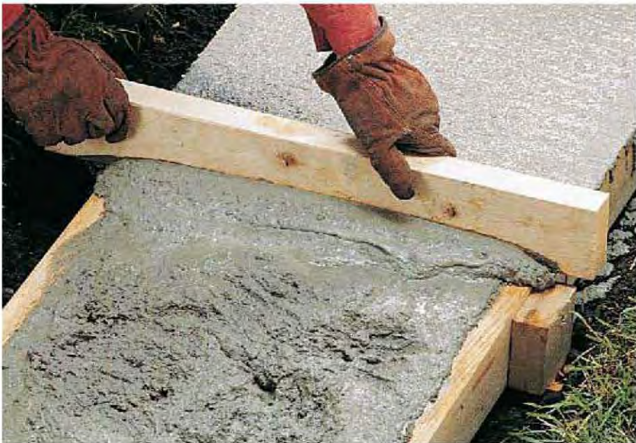
A. Pour footings that are 4" longer and wider than the pillars on each side. This project calls for 16 × 20" footings (see page 84).
