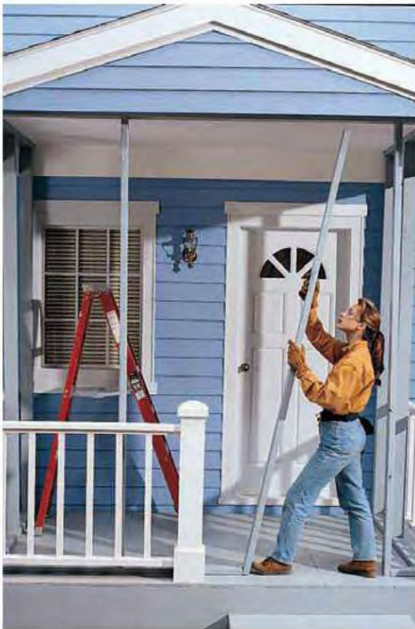
D. Install studs and posts at reference marks on the top and sole plates. Toenail in place with 16d casing nails.
