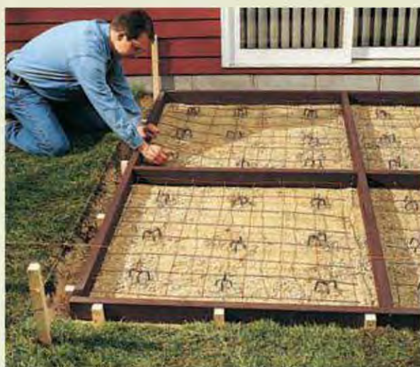
Concrete patios require reinforcement with steel mesh or rebar.
