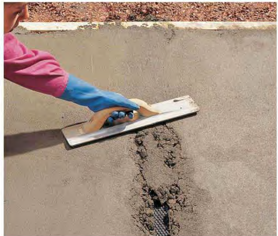
D. Pour and smooth out the next working section. After floating this section, remove the 2 × 2 temporary form between the two sections and fill with fresh concrete.
