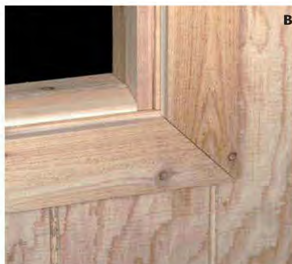
Window trim with miter joints. Cut all miters at 45° and test-fit the joints before nailing the pieces.
