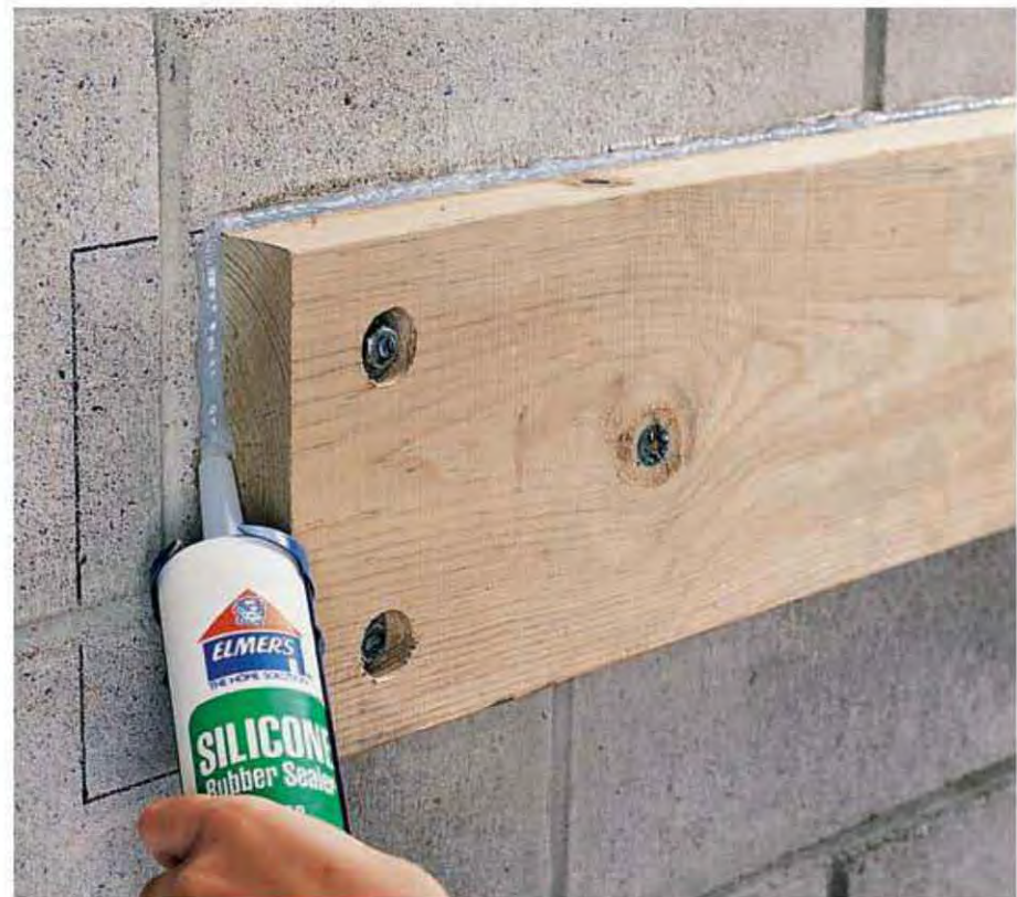
6. Seal the cracks between the wall and ledger with silicone caulk. Also seal the lag screw heads.
