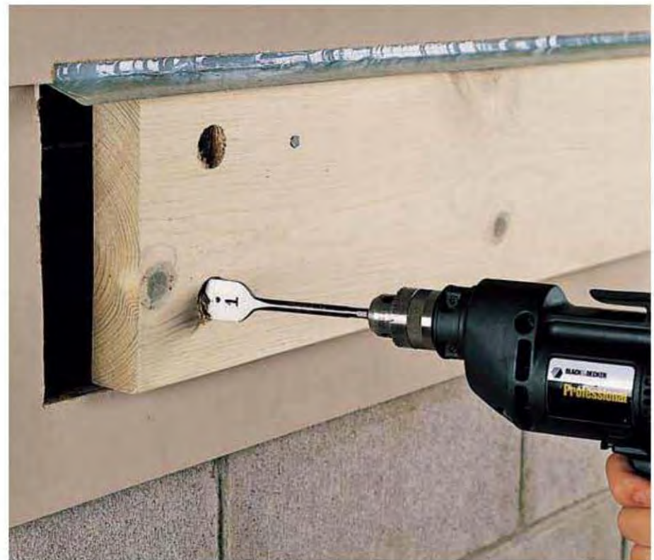
8. Counterbore each pilot hole to \frac{1}{2} " depth, using a 1" spade bit.
