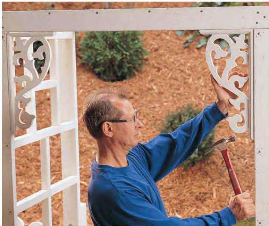
F. Add millwork brackets at each corner where the tie beams and the trellis frame posts meet. Secure with finish nails.
