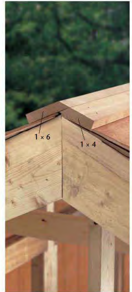
D. Use a T-bevel and scrap boards to find the ridge angles, then cut the 1×4 and 1×6 for the ridge cap.
