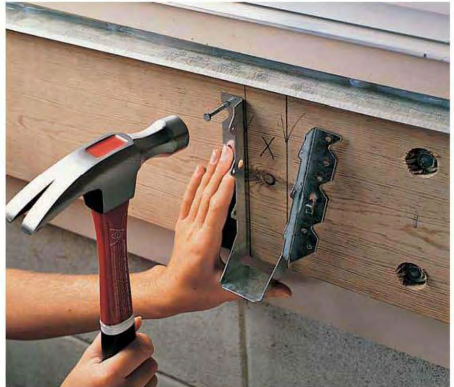
11. Attach joist hangers to the ledger and to the header joist. Position each hanger so that one of the flanges is against the joist outline. Nail one flange to framing members with 10d galvanized common nails.
