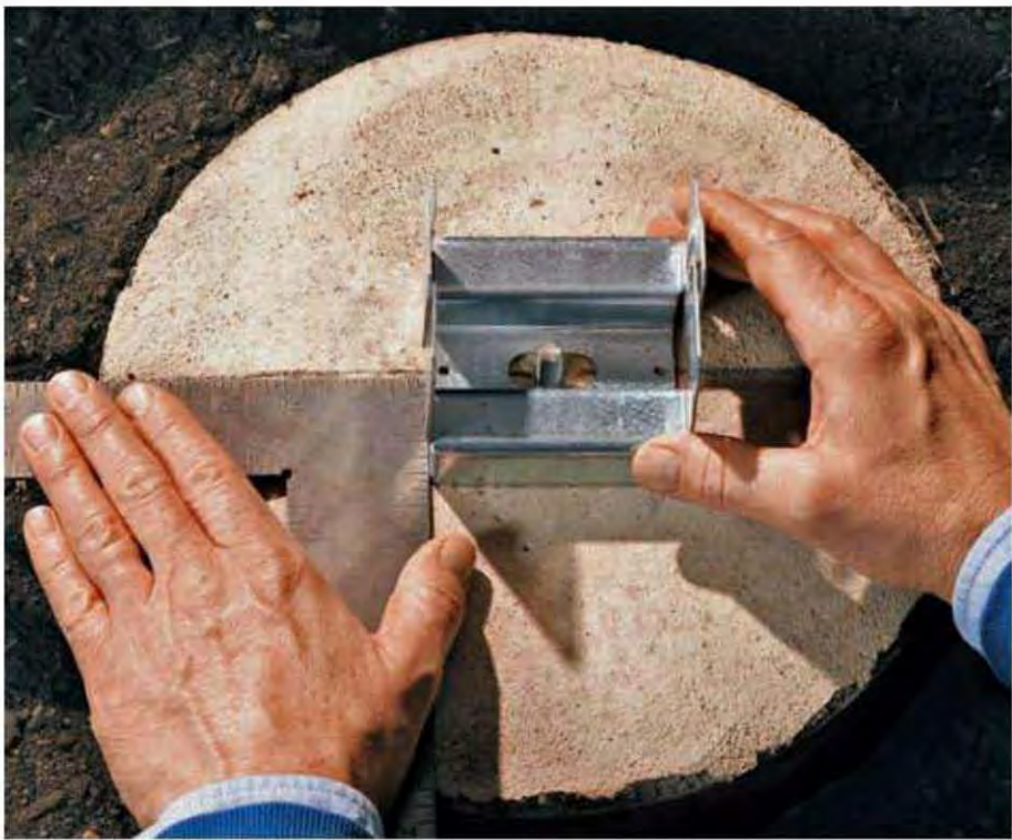
4. Use a framing square to make sure the post anchor is positioned square to the reference line drawn on the footing.
