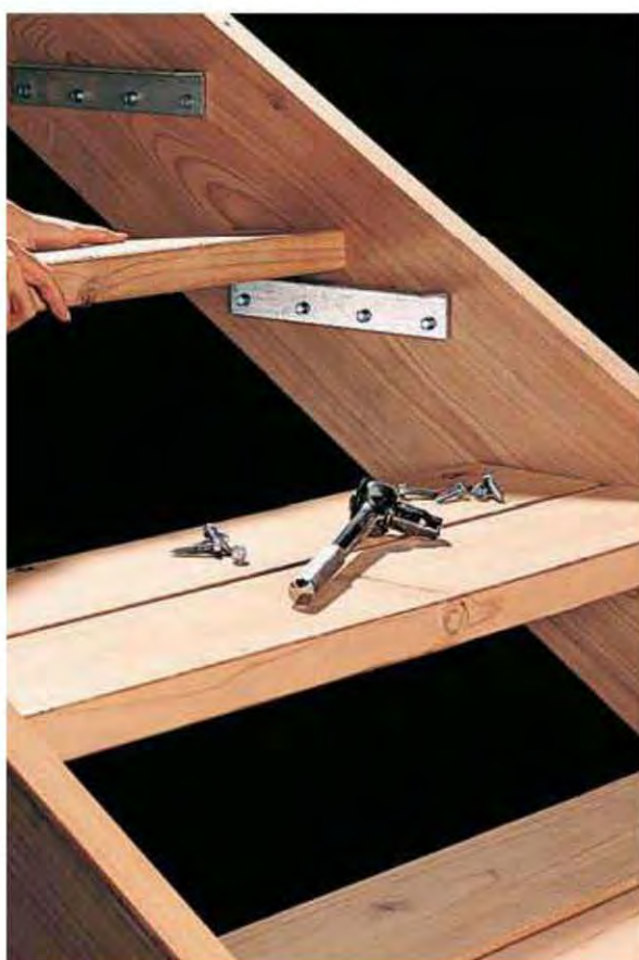
Open steps have metal cleats that hold the treads between the stringers. The treads on this stairway are built with 2 × 6s to match the surface decking.
