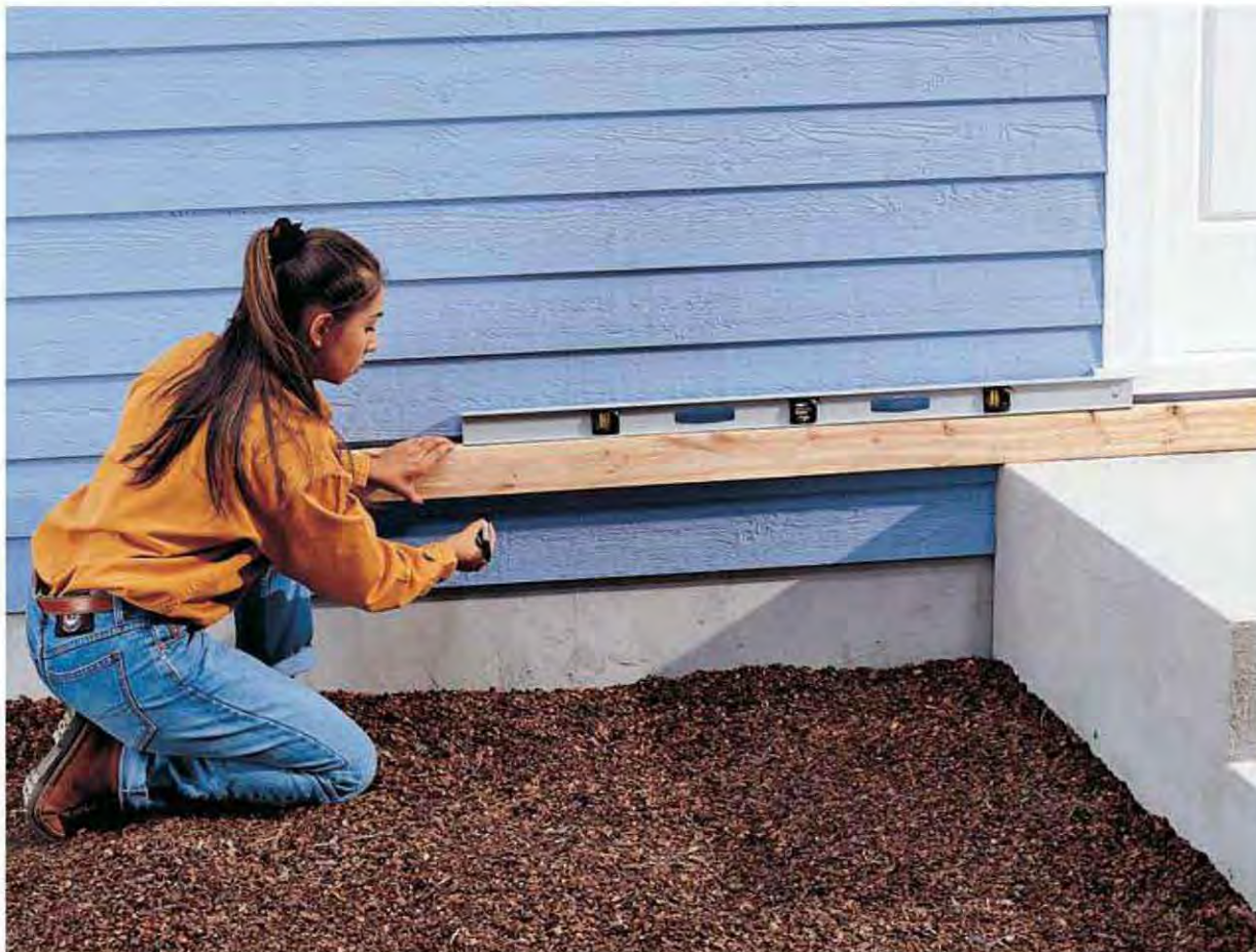
A. Mark the center and endpoint of the ledger location, then mark the ledger height. Use a straight, scrap 2 × 4 and a level to ensure the ledger is at the same height as the steps.
