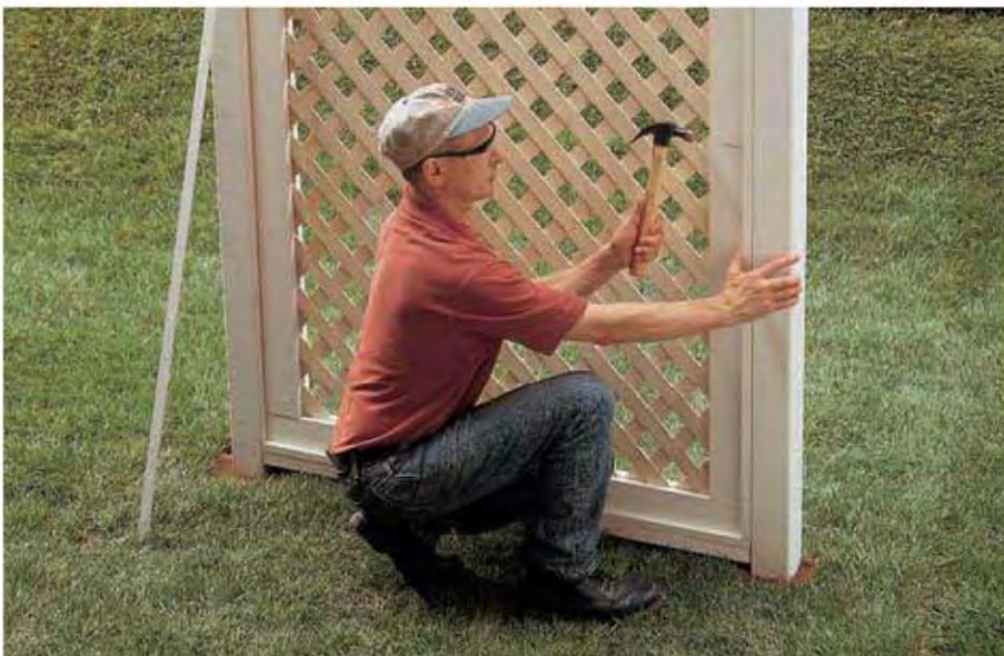
F. Set the panel in place between the center pair of posts. Add stops on the front side, then drill pilot holes and nail the stops in place, using 6d galvanized nails.
