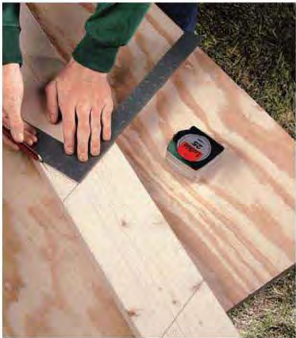
B. Mark the bird's mouth level cut by squaring off of the bird's mouth plumb cut.
