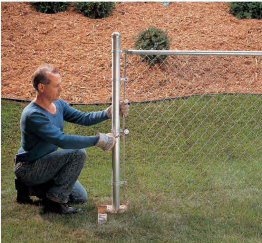
7. Weave a tension bar through the chain link mesh and attach it to the tension braces with bolts.
