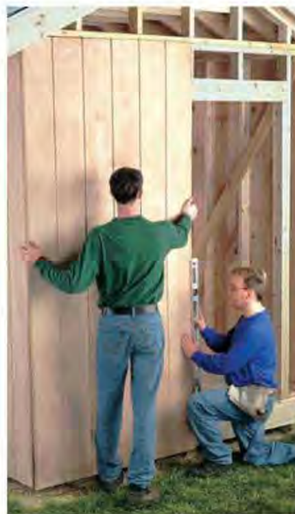
A. Install the plywood siding vertically. Plumb each sheet and fasten it to the framing with 8d galvanized finish nails.
