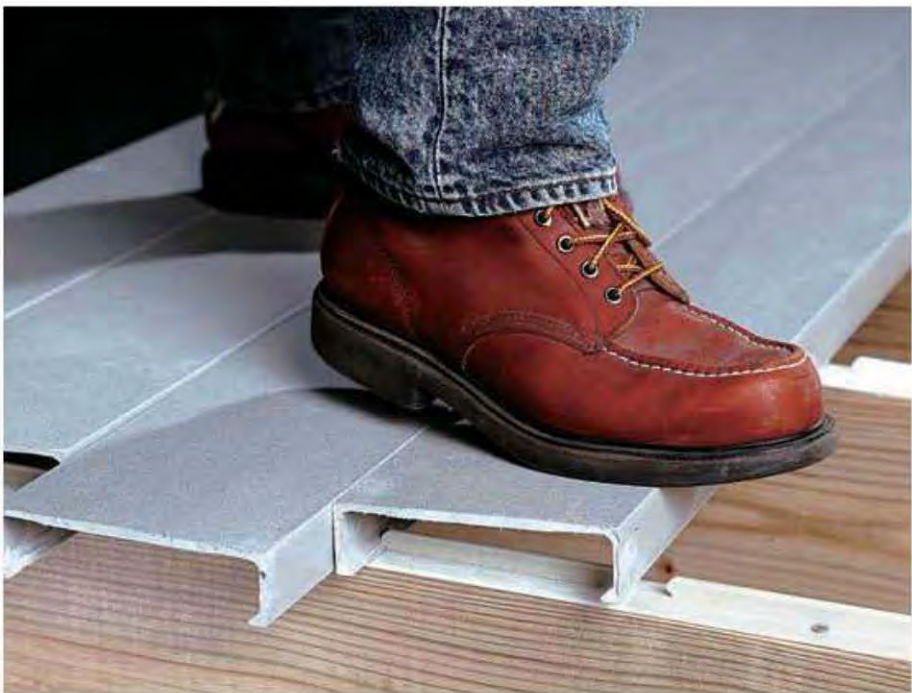
2. Place the open face of a decking board perpendicular to the joists, resting on top of a row of clips. Apply firm pressure to the top of the deck board until the decking snaps into place over the retaining clips. Work along the row, snapping the deck board in place. Attach the remaining deck boards in place, snapping each onto a row of retaining clips.
