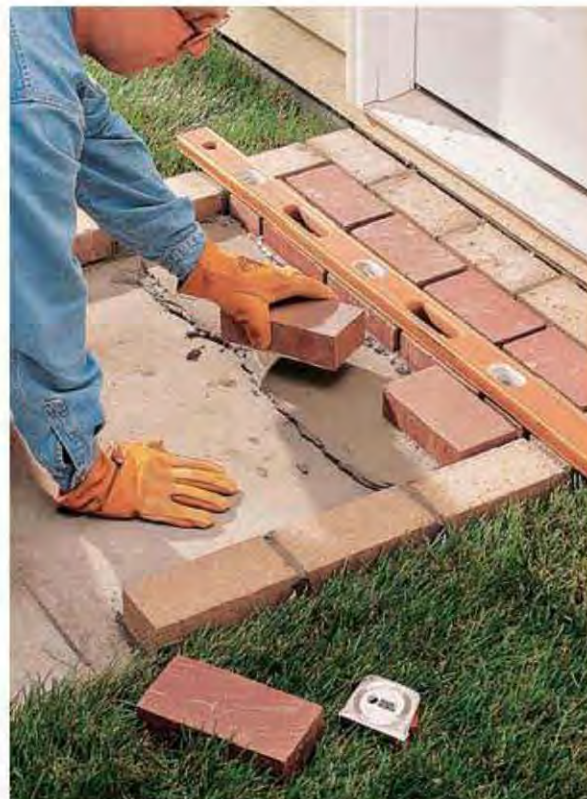
C. Set the pavers in the field area, without buttering the edges. Apply mortar beds in small sections—no more than 4 sq. ft.
