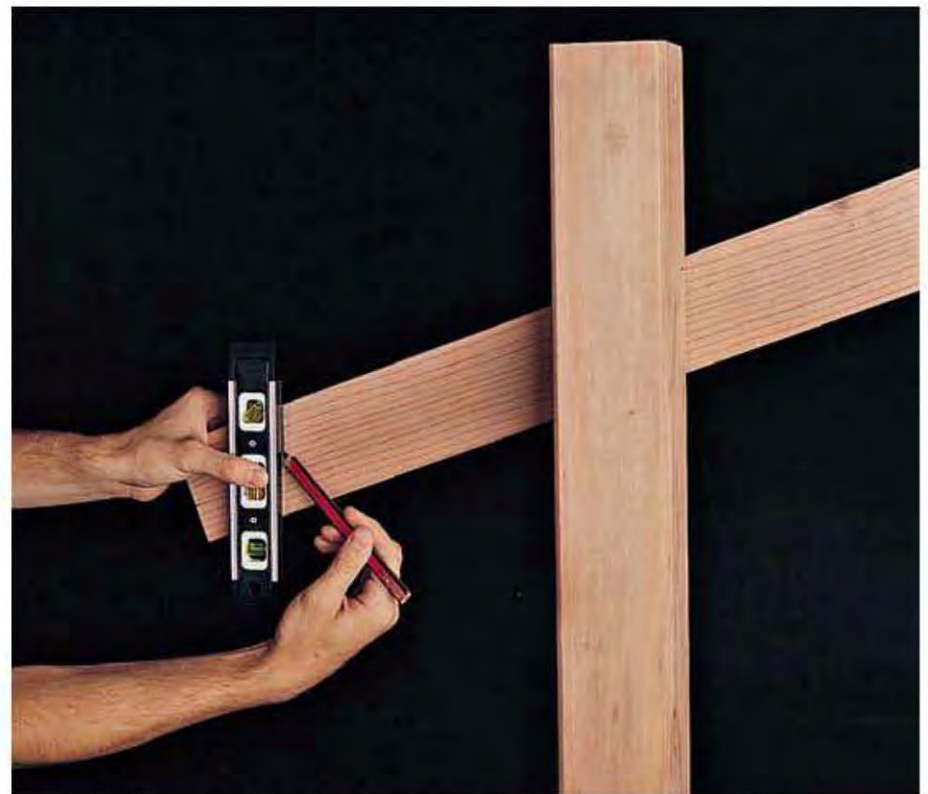
17. Use a level to mark a plumb cutoff line at the bottom end of the stairway rail. Remove the rail.
