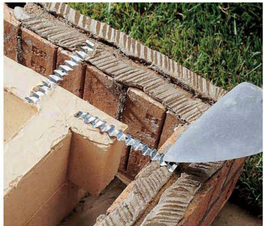
D. Place metal ties between the corners of the inner and outer walls at the second, third, fifth, and seventh courses.
