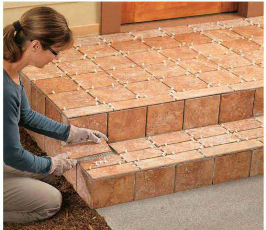
21. Fill in the field tiles on the stair treads, being sure to leave a gap between the back tiles and the riser tiles that's the same thickness as the other tile gaps. Allow thinset mortar to cure for a few days.
