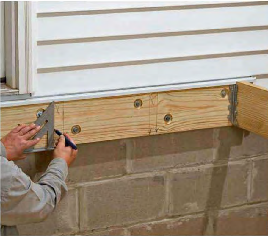
8. Draw the outline of each joist on the ledger using a combination square as a guide.
