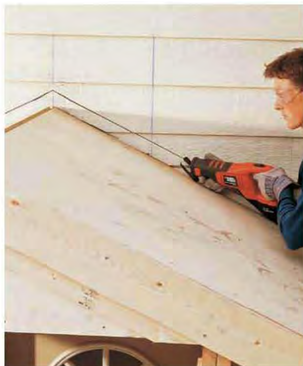
A. Cut away 2" of siding above the roof sheathing.
