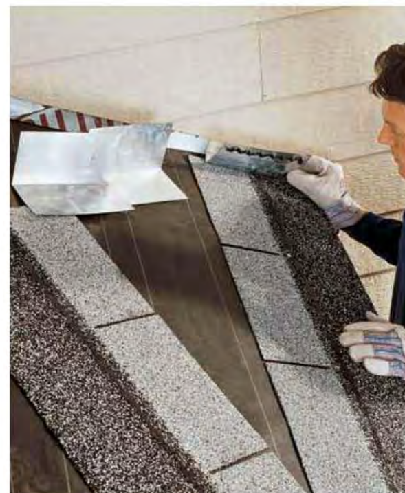
C. Apply roofing cement to the base of the flashing, then tuck the flashing under the siding and secure it to the roof.
