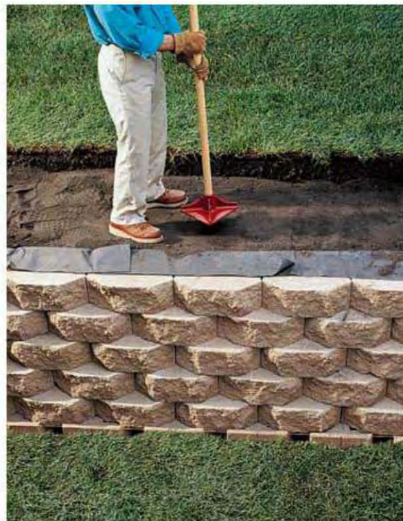
8. Fold the landscape fabric back against the drainage rock and then backfill over the fabric with black dirt.
