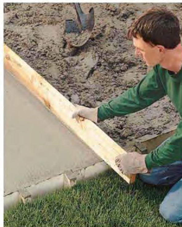
E. Screed the concrete after filling the form, using two people to screed, while a third fills low spots with a shovel.
