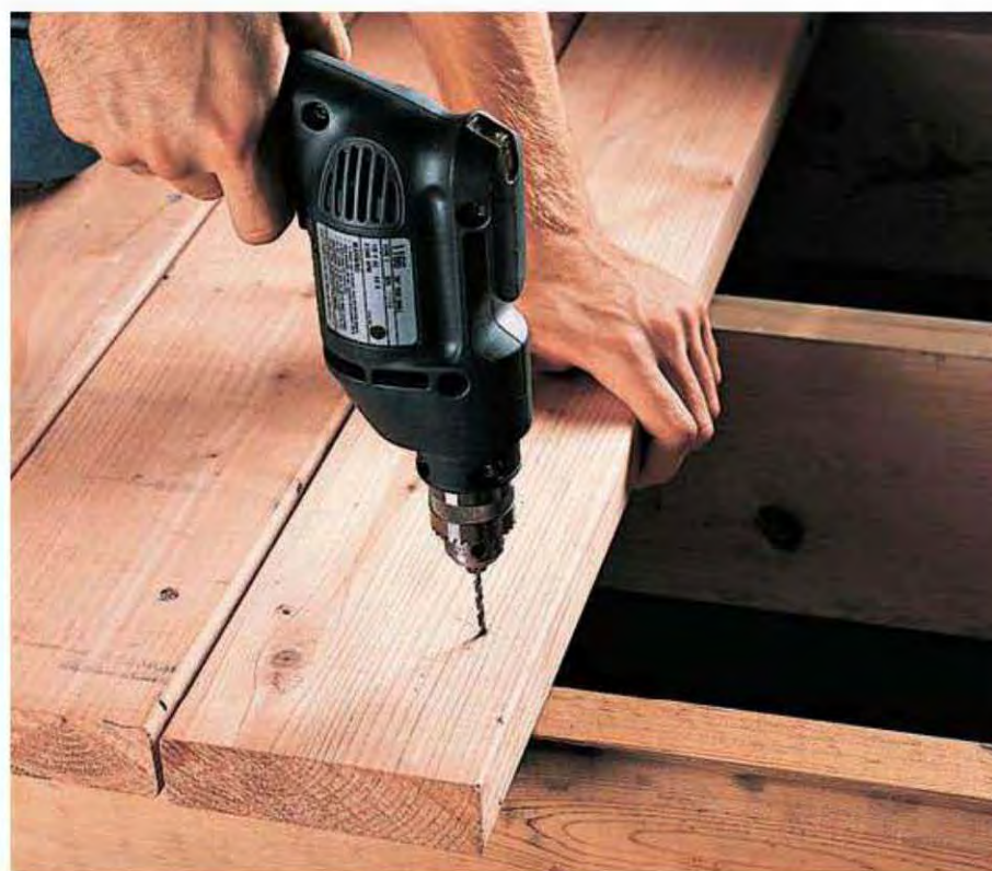
4. Drill \frac{1}{8} " pilot holes in ends of boards before attaching them to outside joists. Pilot holes prevent screws from splitting decking boards at ends.
