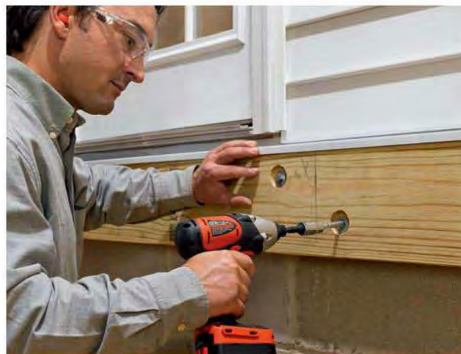
Galvanized or stainless steel lag bolts and washers are the correct fasteners for installing ledgers to the band joist of a house. You can also use them for making other wood-to-wood connections.
