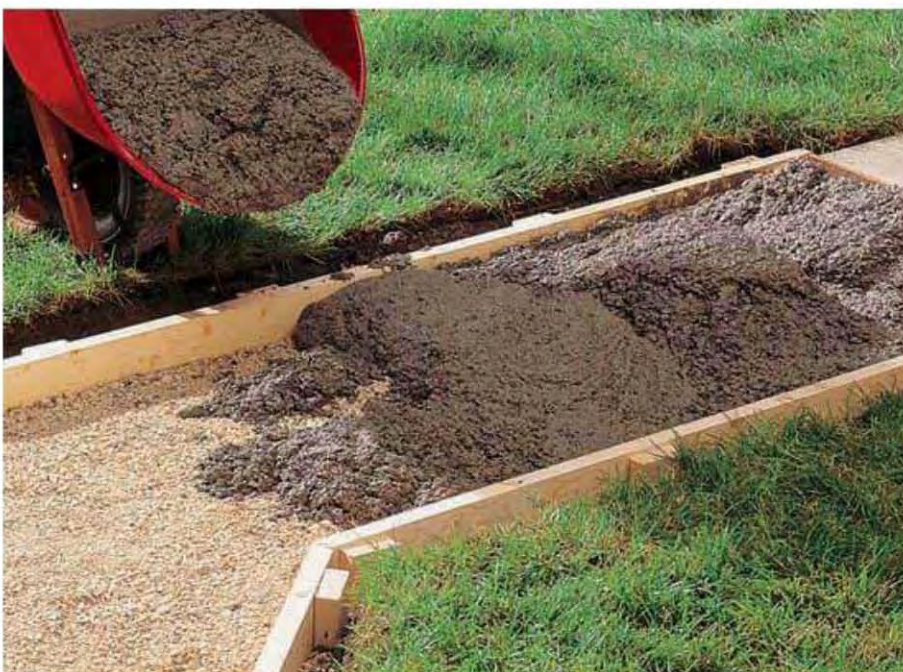
6. Mix, then pour concrete into the project area. Use a masonry hoe to spread it evenly within the forms.
