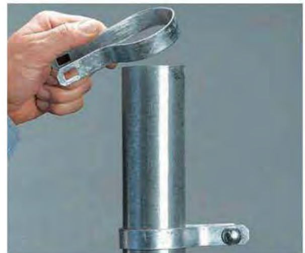
2. Place three tension bands on every gate and end post. Place the first band 8" from the top, the second 24" from the top, and the third 8" off the ground. Make sure the flat side of each tension band faces the outside of the fence and points into the fence bay.
