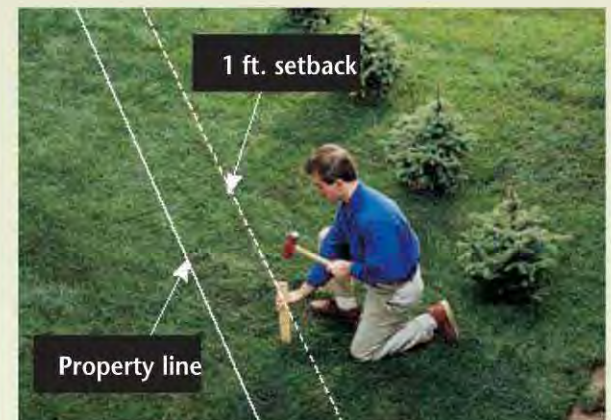
Fences should be set back at least 1 ft. from the formal property lines.
