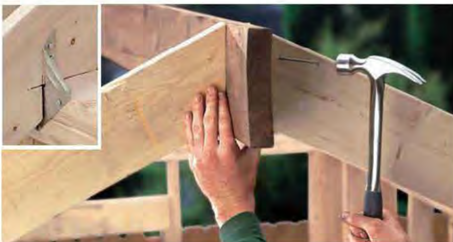
F. Endnail the first rafter to the ridge, then toenail the second. Reinforce the bottom connection with a metal anchor (INSET).
