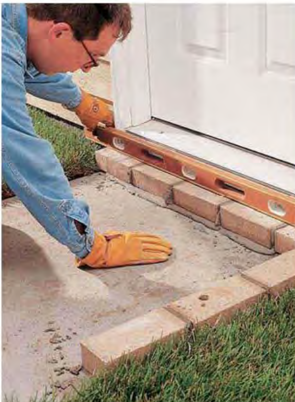
B. Lay the border pavers, buttering an end of each paver with mortar. Use a level to make sure the pavers are even across the tops.
