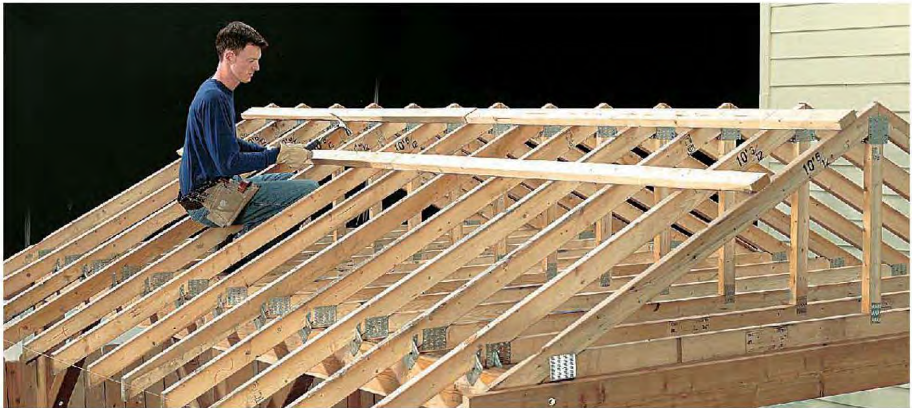
A. Install the purlins across the rafters, then add blocking at the gable ends.
