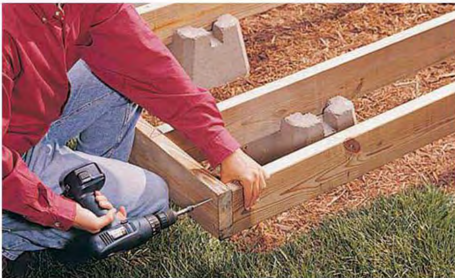
Install the front and back rim joists between the ends of the side joists, securing them with pairs of deck screws.
