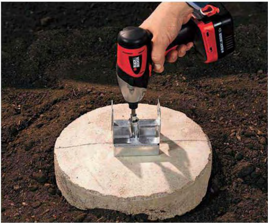
5. Thread a nut over each J-bolt, and tighten it securely with a ratchet wrench or impact driver.
