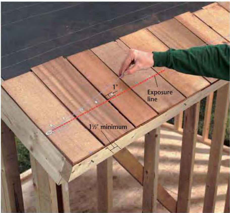
C. Install the first course of shingles on top of the starter course, offsetting the shingle gaps 1½" between the courses.
