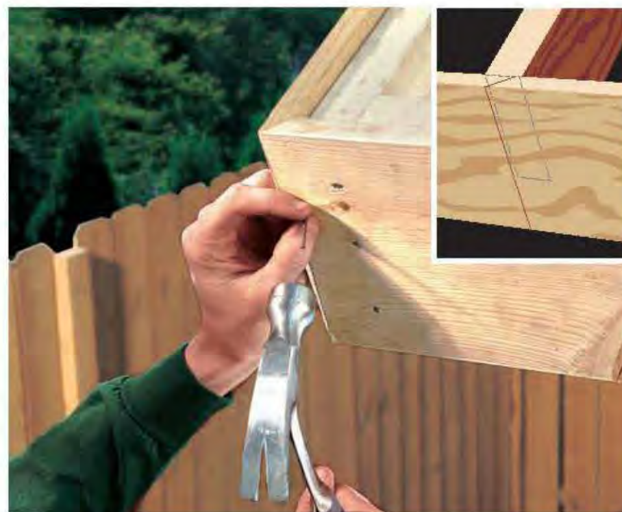
B. Fasten the fascia to the rafters (or subfascia) with 8d finish nails, then lock-nail the corner joints with 6d nails. Use scarf joints to join boards in long runs (INSET).
