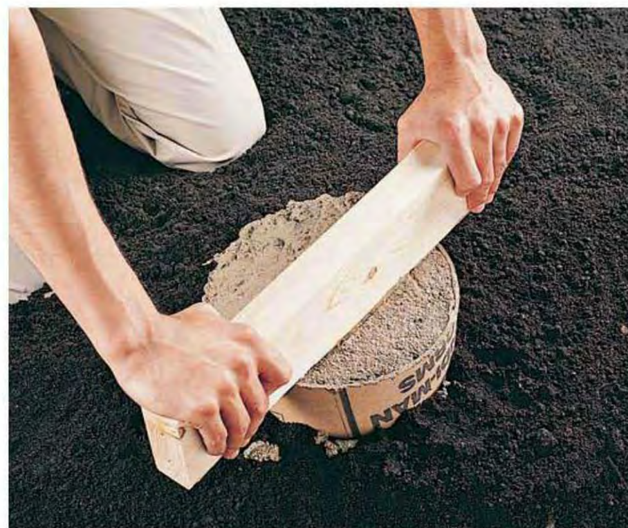
10. Level the concrete by pulling a 2 × 4 across the top of the tube form, using a sawing motion. Add concrete to any low spots. Retie the mason's strings on the batter boards and recheck measurements.
