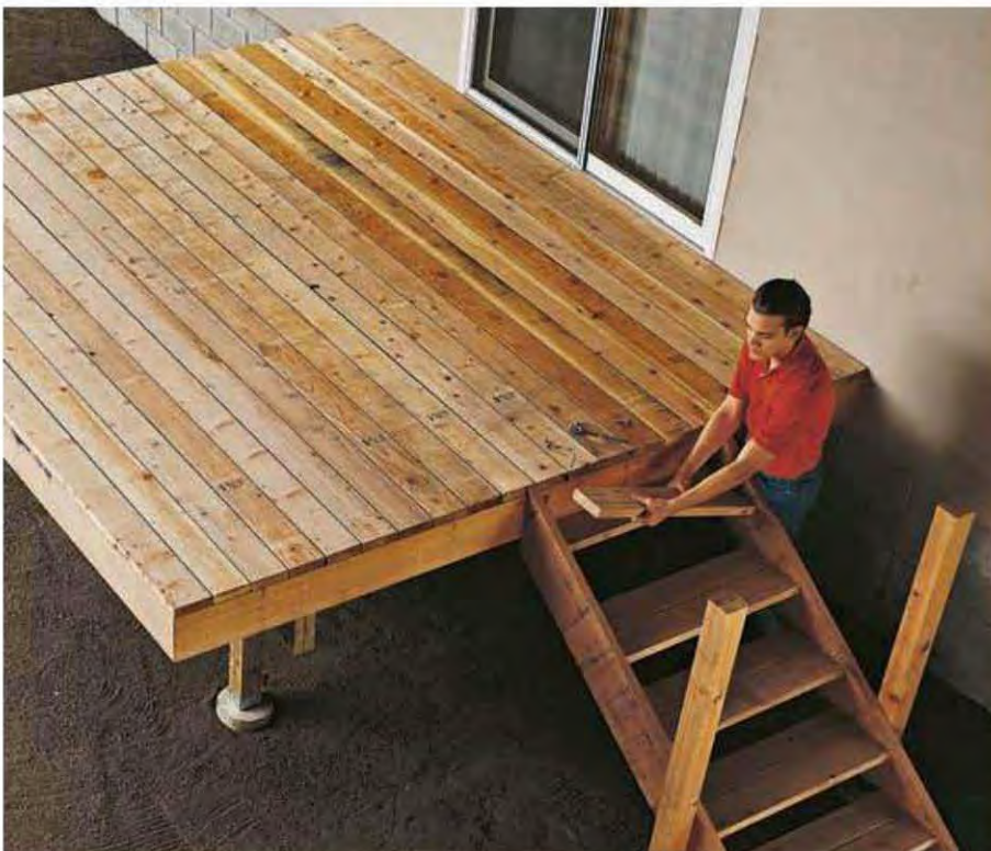
6. Build deck stairs (page 222). Stairs provide access to the deck and establish traffic patterns.
