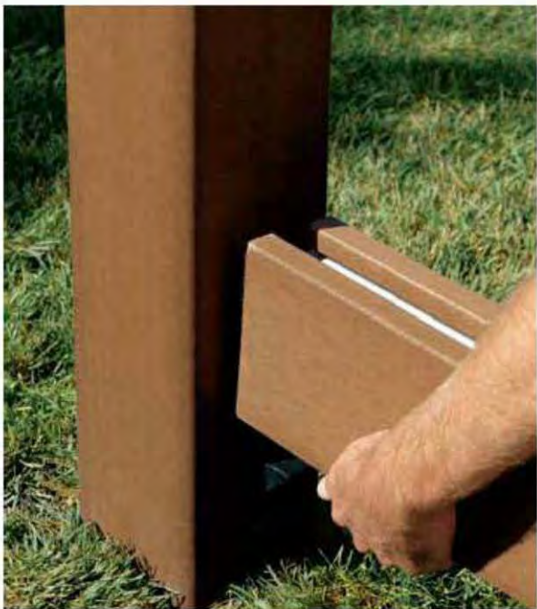
6. Rest the clad rail stringers onto the post brackets and check with a level. If necessary, remove the stringer and adjust the bracket height.
