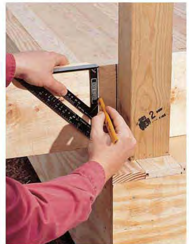
B. Place the roof ledger on the deck, flush against the posts. Mark the edges of the deck and the posts, then cut the ledger to size.
