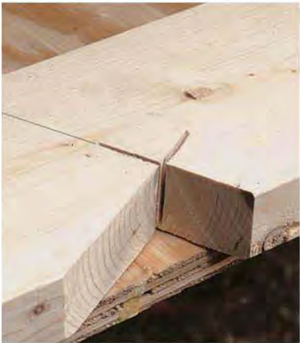
C. Cut the bird's mouth by overcutting the lines just until the blade cuts entirely through the thickness of the board.
