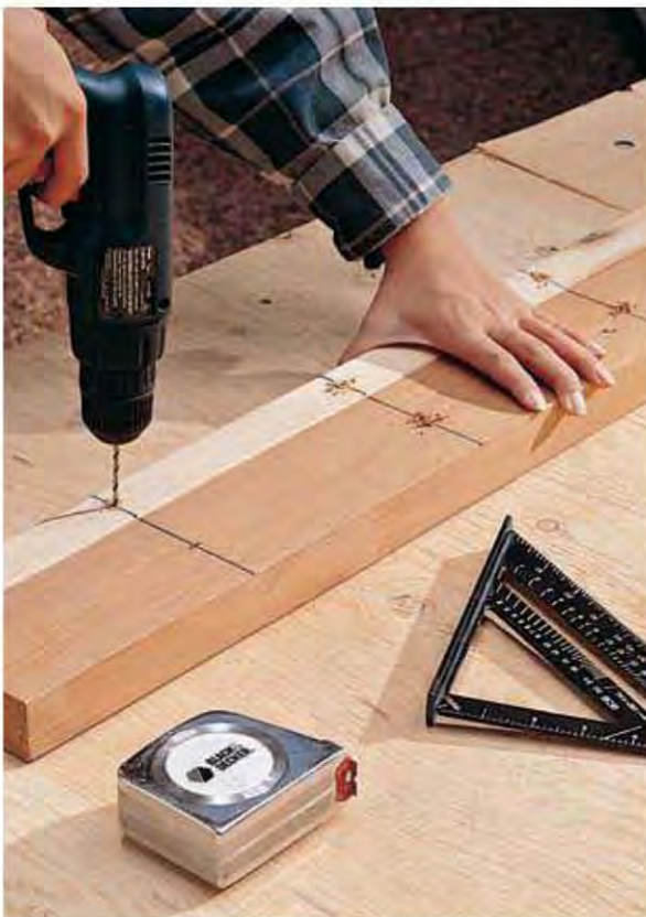
C. Drill ⅛" pilot holes through the top and bottom rails, centered side-to-side at each baluster layout mark.
