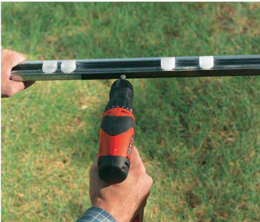
9. Attach the moving and nonmoving parts for the upper door track to the side frames if your shed has sliding doors.
