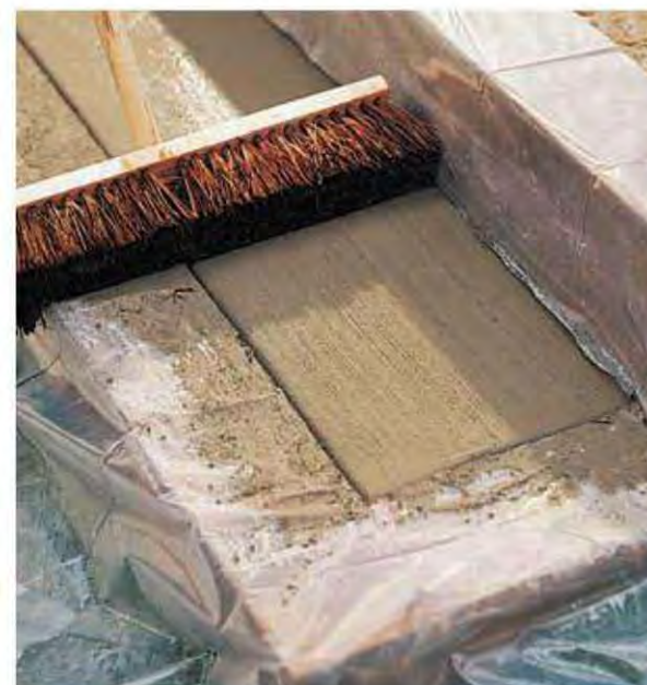
G. Texture the surface of the concrete by drawing a stiff-bristled broom across it in one sweeping motion while the concrete is still wet. Brush only once to avoid overlap. Remove plastic. When hardened, mist with water and then cover with plastic. Allow to cure for one week.
