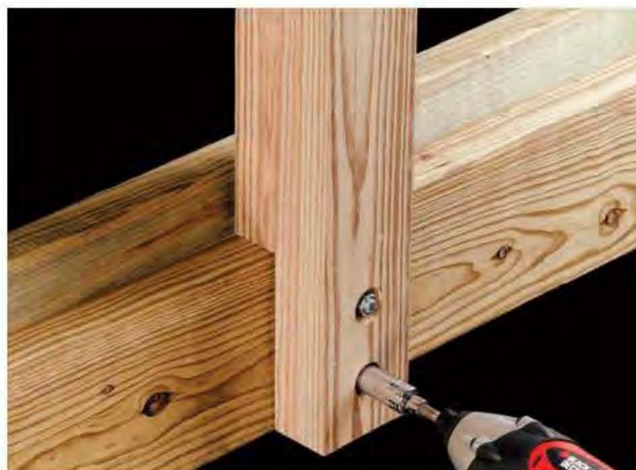
Attach the railing posts to the upper deck rim joists with carriage bolts, washers, and nuts.
