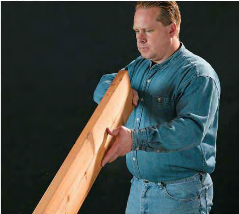
B. Sight along both narrow edges of the beams. If a beam is arched, mark the beam on the convex side of the arch.
