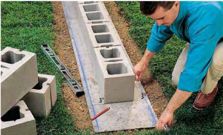
2. Dry-lay the first course, leaving a 3/8" gap between blocks. Draw reference lines on the concrete base to mark the ends of the row, extending the lines well past the edges of the block. Use a chalk line to snap reference lines on each side of the base 3" from the blocks. These reference lines will serve as a guide when setting the blocks into mortar.
