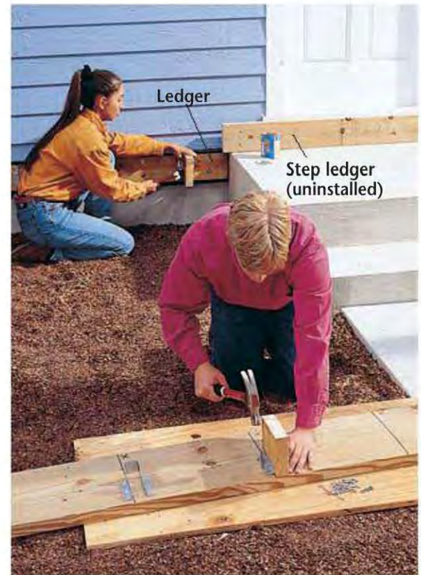
C. Attach joist hangers to the ledger and rim joist at each marked location using 10d joist hanger nails.
