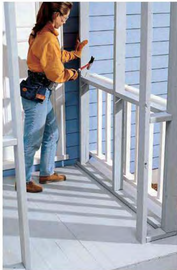
E. Measure and cut 2 × 4 spreaders to size, and fasten between studs at the height of the railings.
