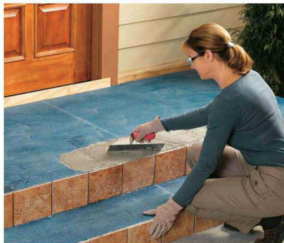
17. Cut tiles as indicated by your dry run, and then begin installing them by troweling thinset adhesive for the bullnose tiles at the front edge of the landing. The tiles should overlap the top edges of the riser tiles, but not extend past their faces.
