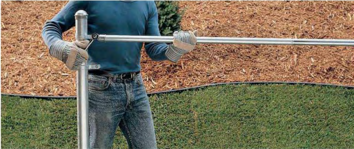
5. Cut the last piece of top stringer in a section to size. Adjust the brace band and stringer end to fit it in place.
