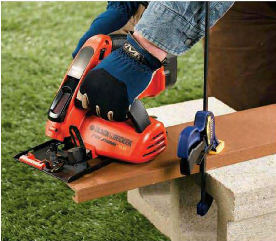
11. Trim the upper corner of the last picket to clear the bracket. Secure last picket to the post like the first, with three evenly spaced screws into the post.
