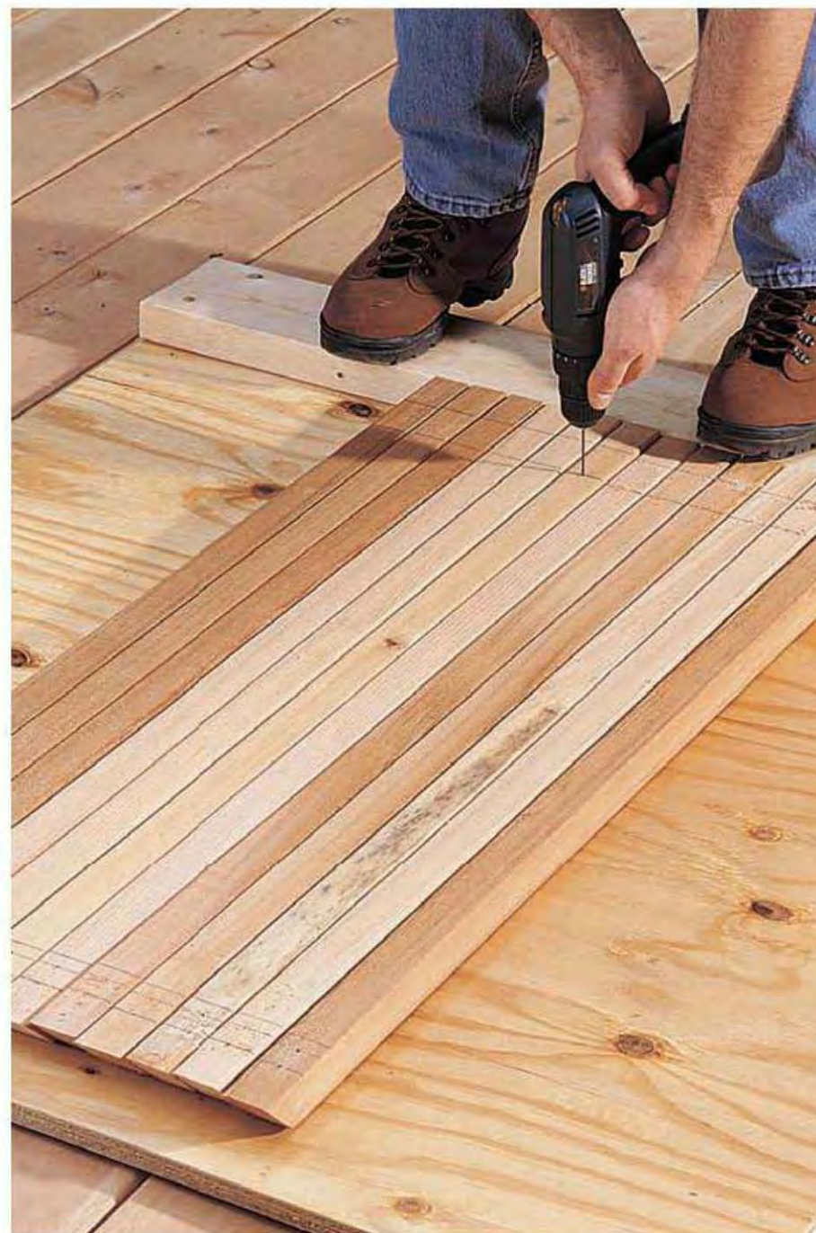
After cutting balusters to length , gang them up and drill \frac{1}{8} " pilot holes through the top and bottom.
