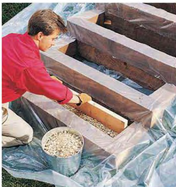
E. Cover the completed framework with plastic. Pour and smooth a 2" layer of compactable gravel in each frame.
