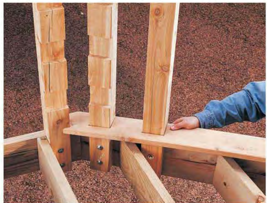
Cut the notches for the first decking board and position it above the stairway.
