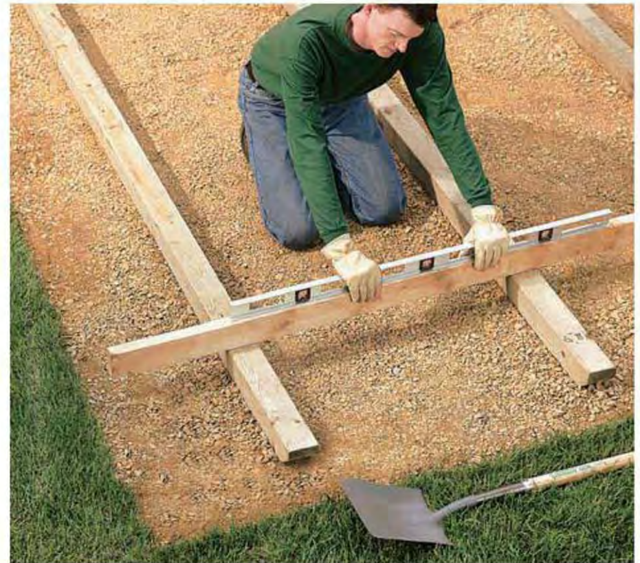
C. Using a board and a level, make sure each skid is level along its length and width and is level with the other skids.
