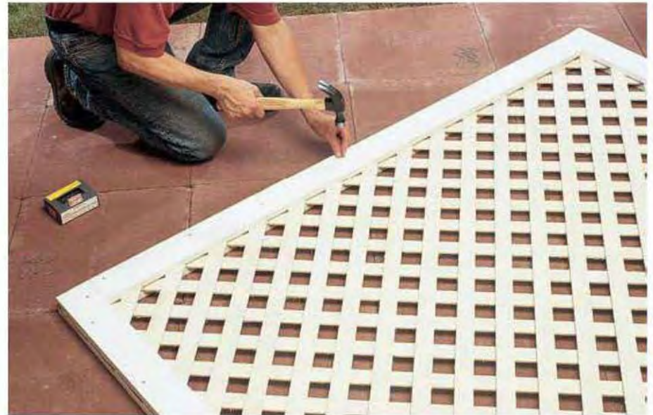
E. Set the front frame in place, butting the pieces in the opposite direction of the back frame. Drive 4d galvanized finish nails every 6" to secure the front frame to the lattice panel and back frame.
