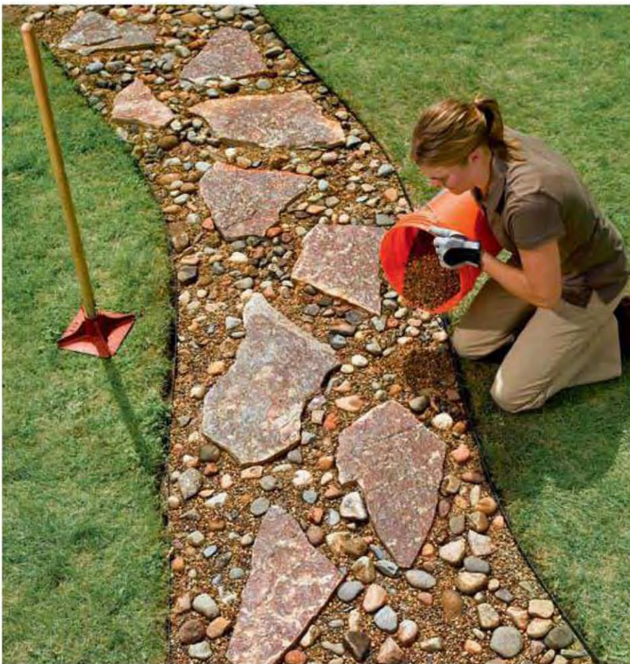
4. Add the smallest size infill stones last, spreading them evenly so you do not have to rake them much.
