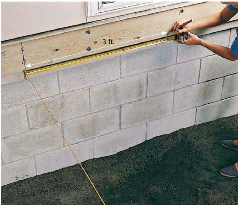
8. Check the mason's string for square using "3-4-5 carpenter's triangle." First, measure along the ledger 3 feet from the mason's string and mark a point, using a felt-tipped pen.
