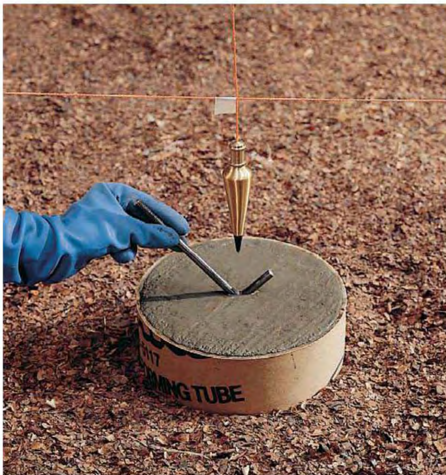
F. Drop a plumb bob to determine the exact center of the footing, and then install a J-bolt at the point to attach the post anchor.
