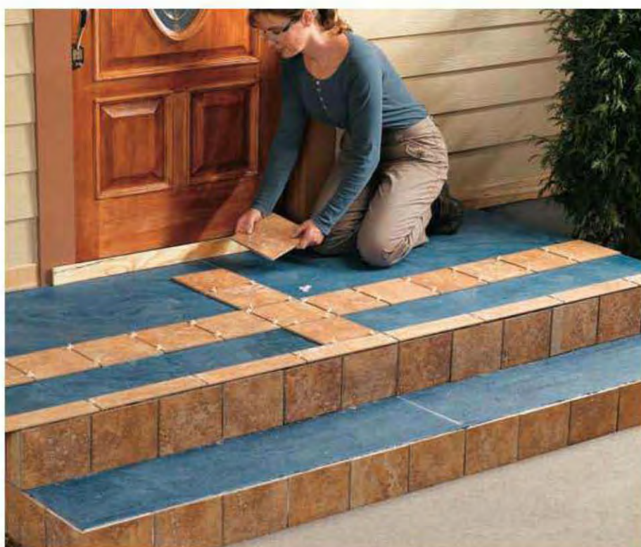
16. Dry-lay tile in both directions on the stair landing. You'll want to maintain the same grout lines that are established by the riser tiles, but you'll want to evaluate the front-to-back layout to make sure you don't end up with a row of tiles that is less than 2" or so in thickness.
