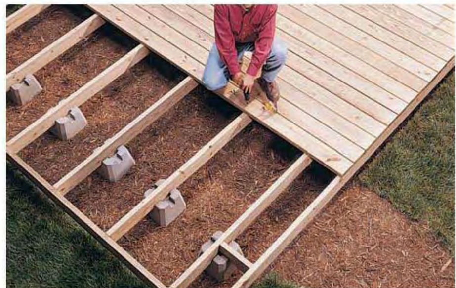
Install the decking by driving a pair of screws into each joist. Use a framing square to leave a 1/8" space between boards.
