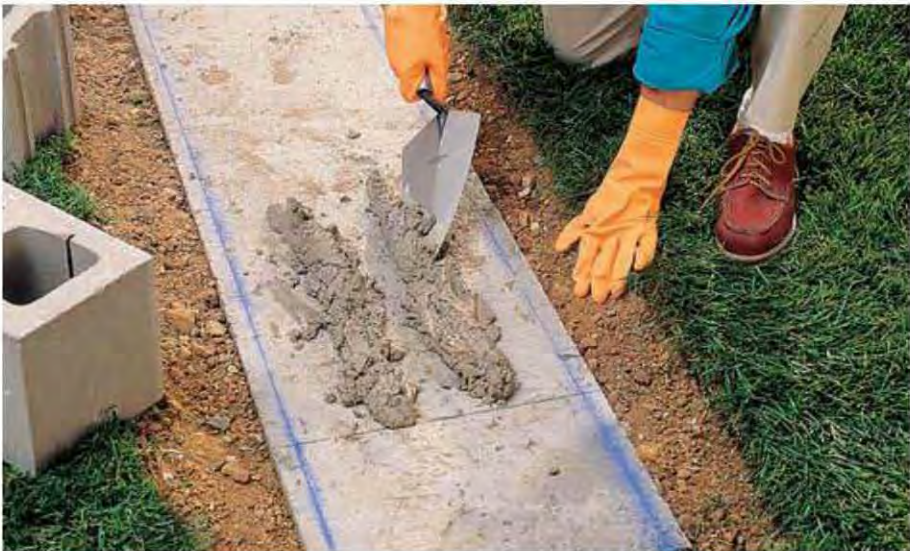
3. Dampen the concrete slab or footing with water, and dampen the blocks if necessary. Mix mortar and place a layer of mortar on to the footing for the first two blocks at one end of the layout. The mortar should be firm enough to support the weight of the first block course.
