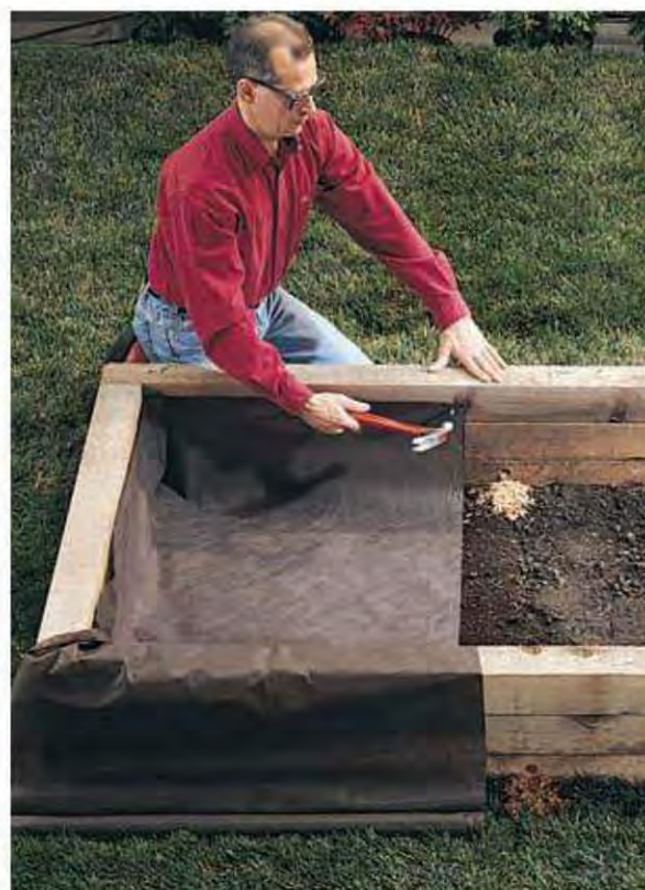
C. Place the third layer of landscape timbers over the second, staggering the joints. Secure the timbers in place with nails. Drill 1" drainage holes through the bottom row of the timbers. Line the bed with landscape fabric.
