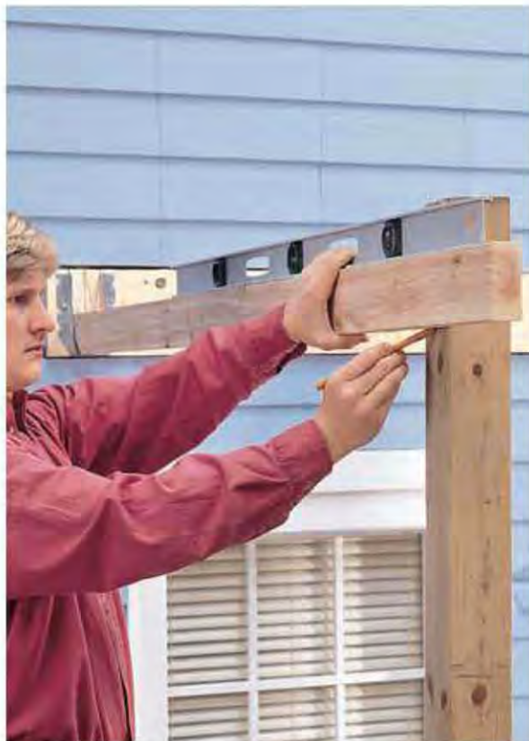
C. Hold a straight 2 \times 4 in the double-joist hanger and against the post, level, and mark a cutting line on the post.
