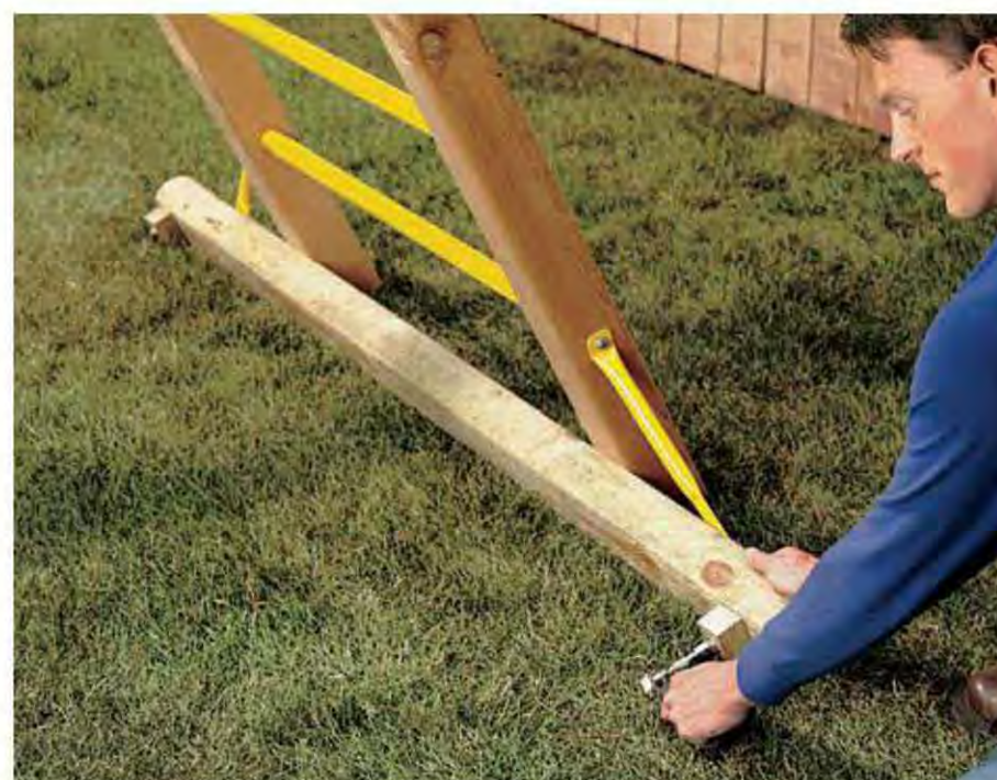
E. With the lower structure on level ground and the ladder support bases attached to the bottom of the ladders, drive anchor stakes into the ground at each end of the base, then attach the stakes to the bases with lag screws.
