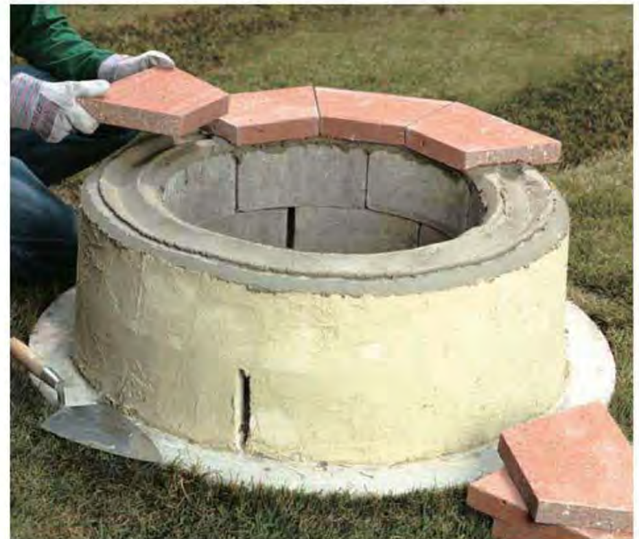
F. Lay a bed of mortar on top of the second course and set the cap stones into place, maintaining a uniform overhang.
