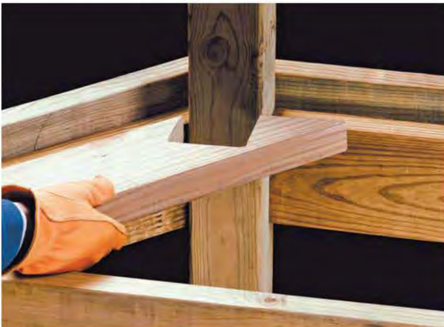
Cut notches in the decking boards that meet the railing posts. Test fit the board: The leading edge should be flush with the face boards.
