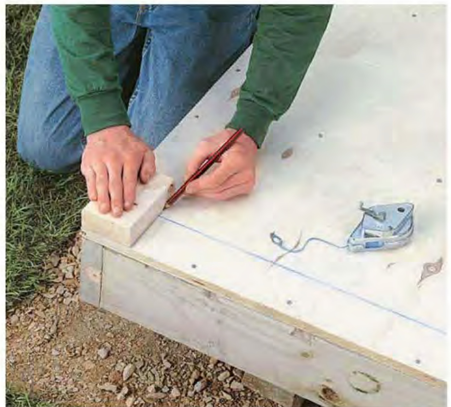
A. Use a block cut from plate material to lay out the bottom plates. Mark at the ends of each wall then snap a chalk line.
