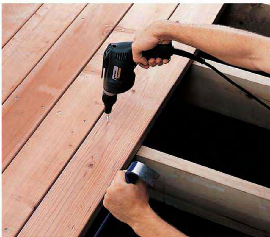
3. If boards are bowed, use a pry bar to maneuver them into position while fastening.
