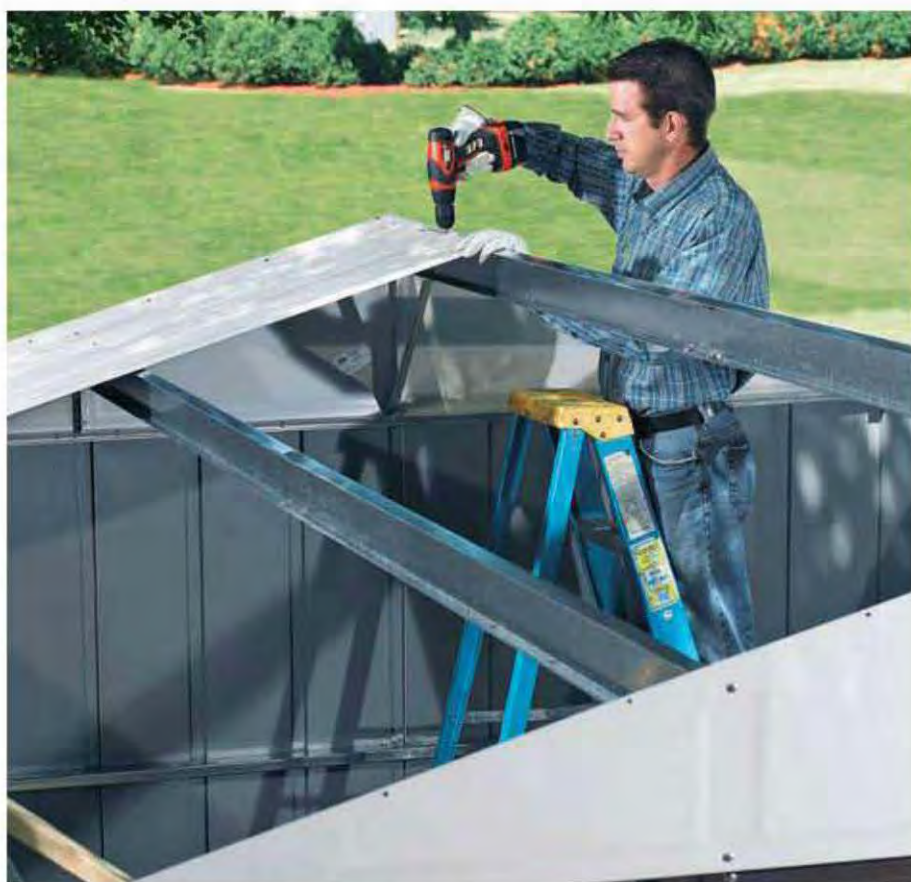
16. Begin installing the roof panels at one end, fastening them to the roof beam and to the top flanges of the side frames.
