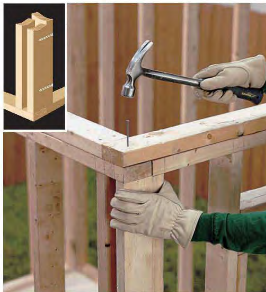
G. Nail together the corner studs of intersecting walls (INSET). Add the double top plates, overlapping the wall corners.
