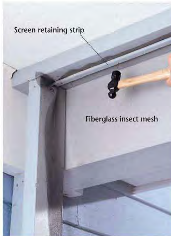
H. Mark center reference lines on the inside faces of all studs and posts. Align mesh and retaining strips with the lines, then fasten with brass brads.
