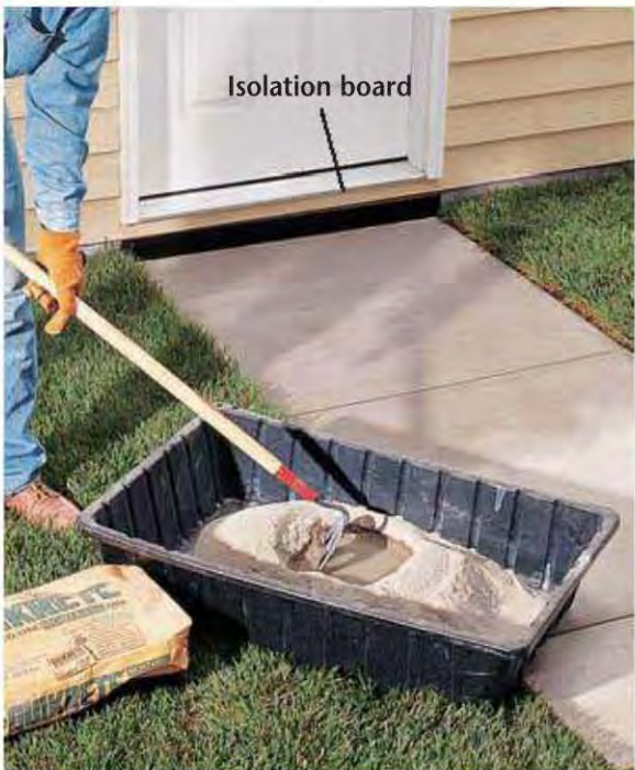
A. Mix a batch of mortar and dampen the concrete slightly. If the landing will abut an adjoining structure, secure an isolation board in place.
