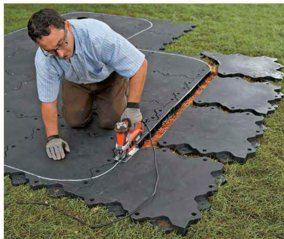
10. One panel at a time, cut panels to shape, using a jigsaw with a blade that's slightly longer than the panel thickness. Use panel scraps to fill in open areas in the layout wherever you can, and then mark and cut the scraps to fit.
