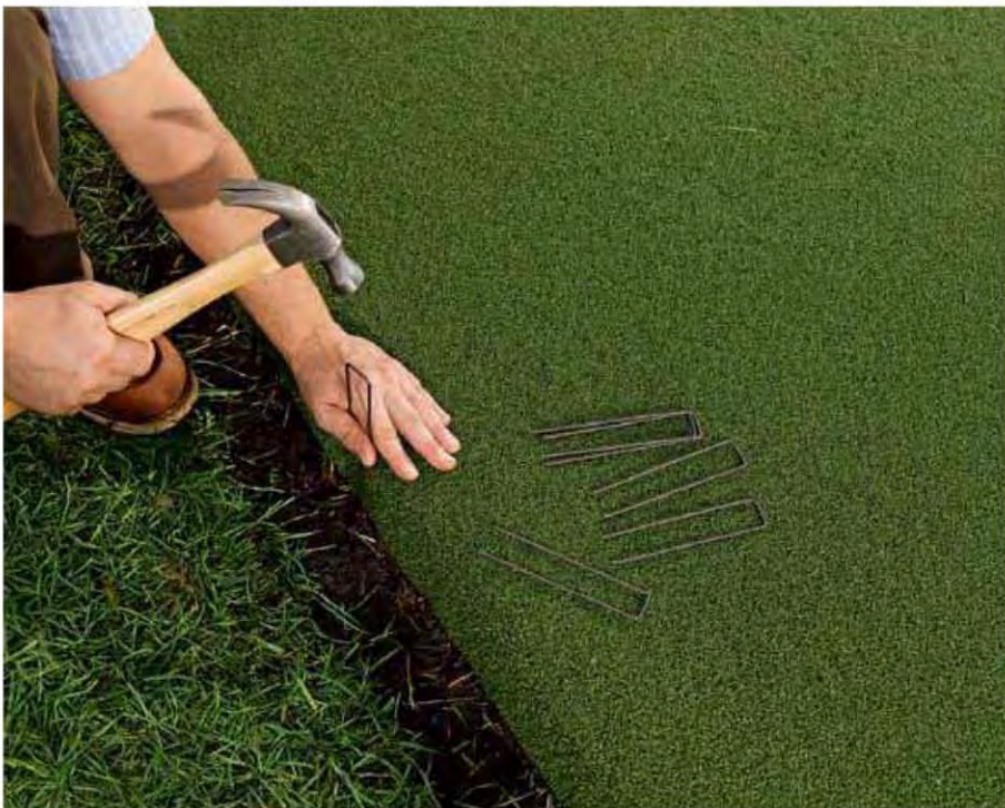
15. Drive carpet spikes or fabric spikes (provided by the kit manufacturer) through the edges of the turf and into the trench to secure the turf.
