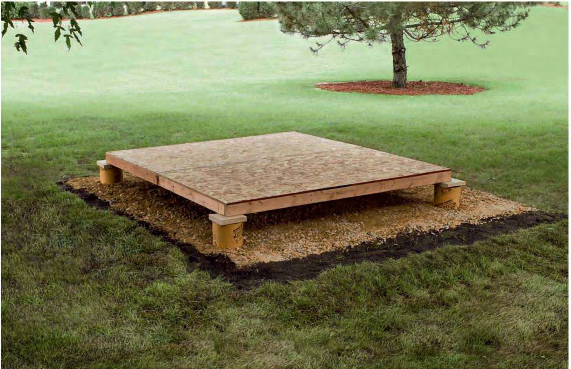
A concrete pier foundation is a stable structure base that combines the permanence of post footings with the potential mobility of a wood-framed floor.
