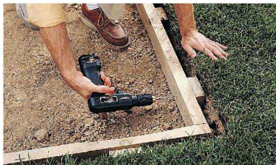
A. Drive 12" stakes outside the 2 × 6 pressure-treated edging, then attach them together with galvanized screws.
