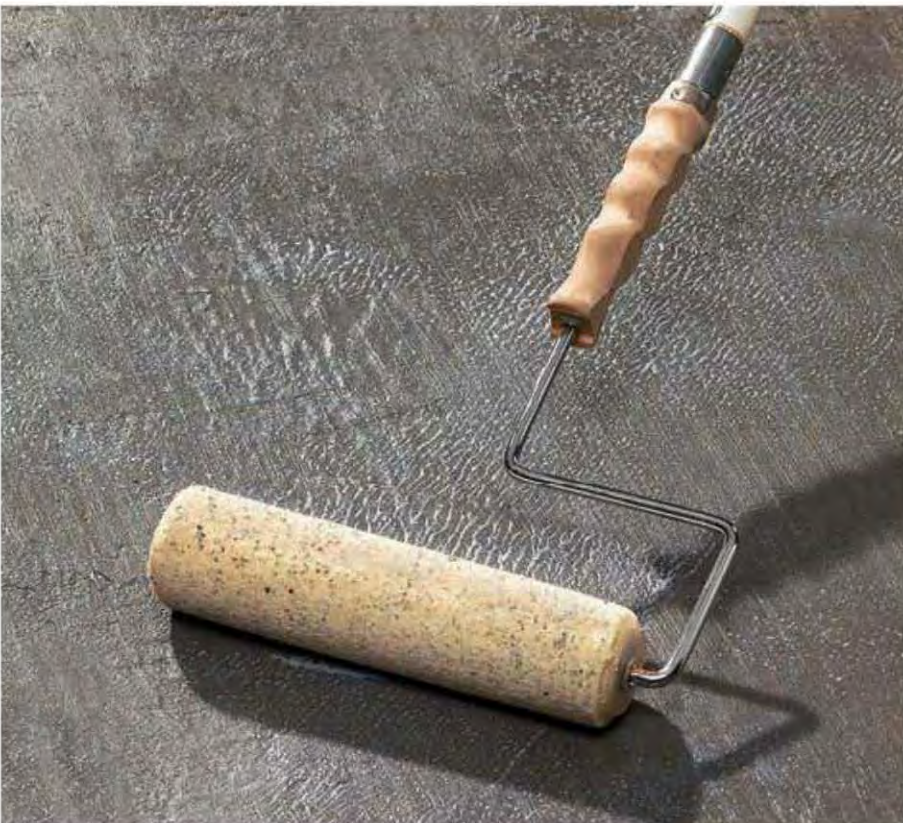
OPTION: Apply acrylic cure and seal with a garden sprayer or roller to eliminate the need for water curing and to seal the concrete for a more durable surface.
