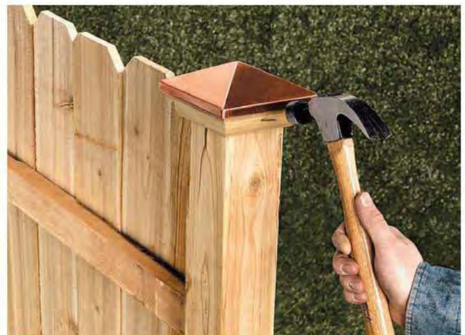
11. Attach post caps or finials and seal, stain or paint your new fence.
