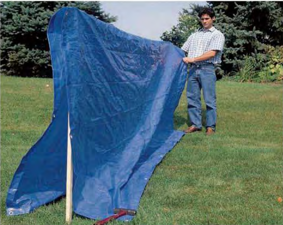
Hang tarps or landscape fabric over a stake-and-string frame to get a sense of the size of the structure and its impact on the landscape.
