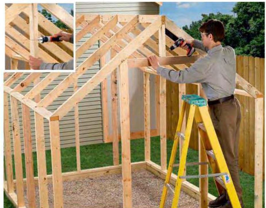
11. Measure up 78" (or less if you want a shorter door) from the sole plate in the door opening and mark a cutting line on the temporary ridge post. Make a square cut along the line with a circular saw or cordless trim saw (INSET). Then cut the door header to fit between the vertical doorframe members. Screw the header to the cut end of the ridge post and drive screws through the frame members and into the header.
