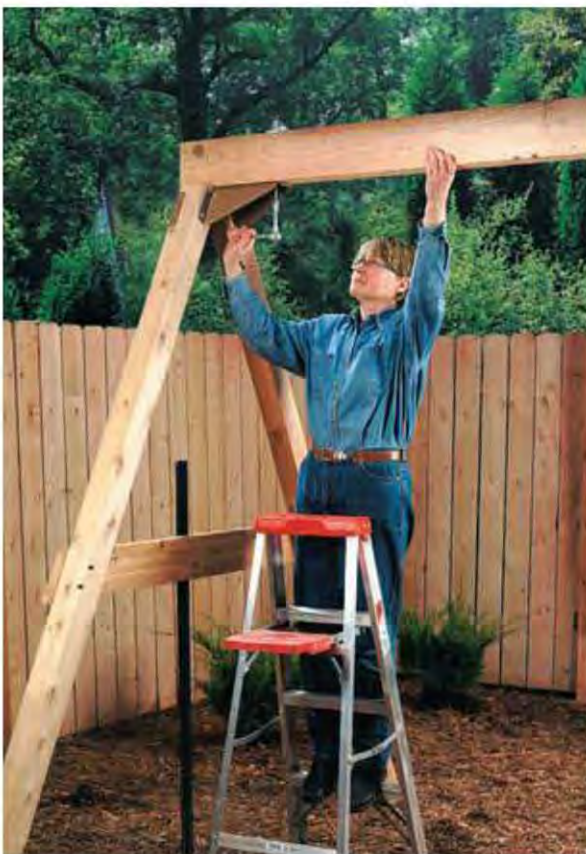
C. Tie the leg assemblies to fence stakes, then center the beam on the brackets and fasten it in place.
