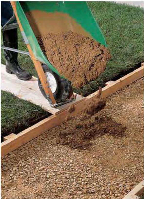
A. Pour concrete into forms, and smooth the surface with a screed board and magnesium float.
