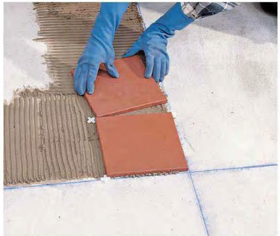
G. Set the first tile in the corner of the quadrant where the lines intersect, adjusting until it is exactly aligned with both reference lines. Position the next tile along one arm of the quadrant, fitting it neatly against the spacer.
