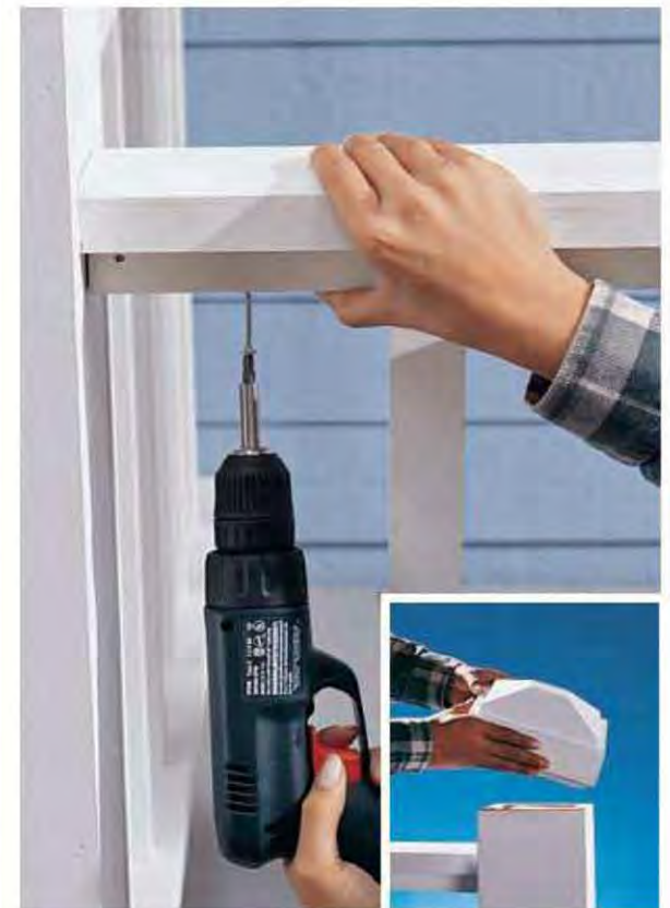
E. Position the cap rail on the top rail, and attach with 2½" deck screws every 18". NOTE: Attach post caps to posts using finish nails.
