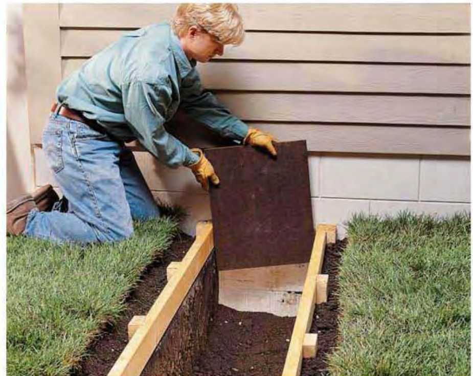
VARIATION: If your project abuts another structure, such as a house foundation, slip a piece of asphalt-impregnated fiber board into the trench to create an isolation joint between the footing and the structure. Use a few dabs of construction adhesive to hold it in place.
