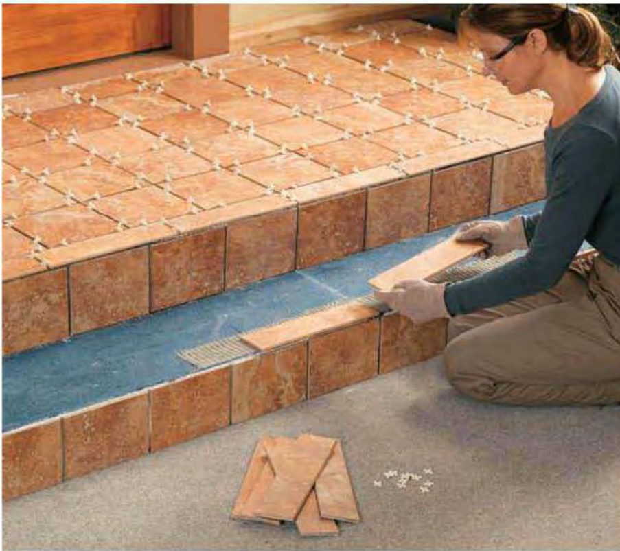
20. Install tiles on the stair treads, starting at the top tread and working your way downward. Set a bullnose tile on each side of the centerline and work your way toward the sides, making sure to conceal the step side tiles with the tread tiles.
