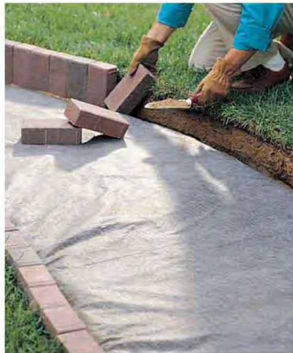
C. Install bricks end to end and flush against each other in the trenches, then pack soil behind and beneath each brick.
