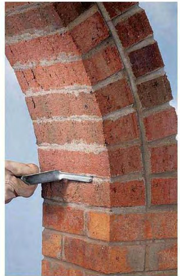
F. Leave the form in place for a week, misting occasionally. Remove the braces and form, then tuck-point the joints on the underside of the arch.
