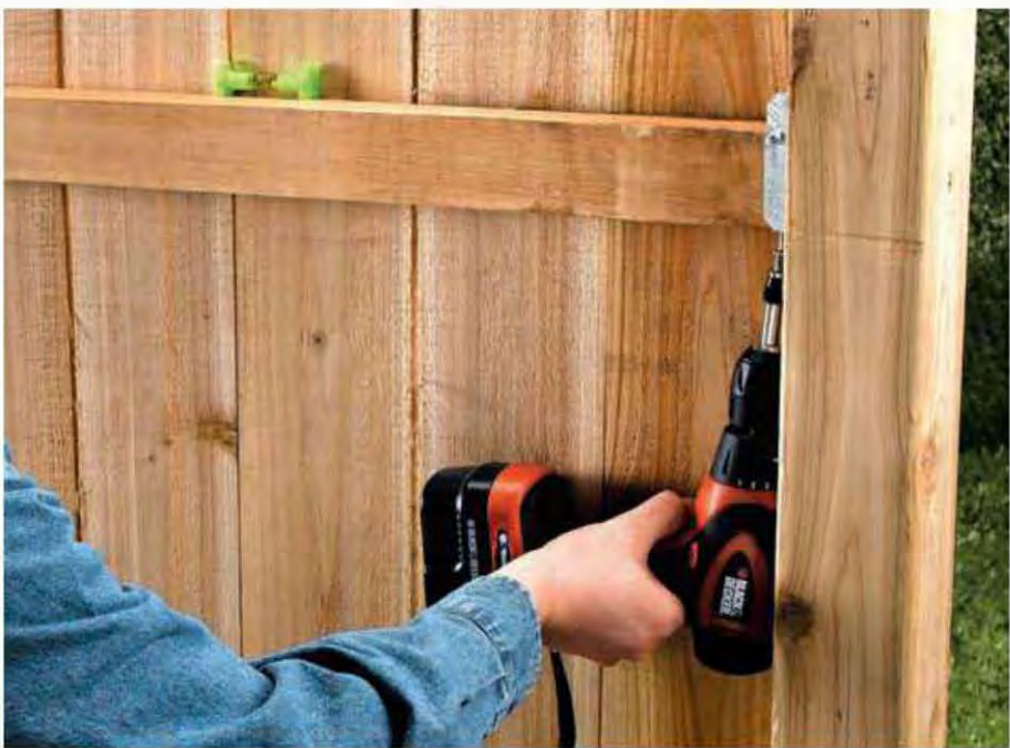
6. Set the first fence panel into the brackets, level it, and attach the end to the brackets with deck screws or joist hanger nails.
