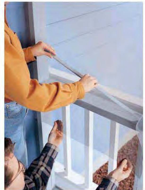
I. Secure the screen at the stretcher with retaining strips and brads. At the sides, pull the screen taut and staple in place, then cover with retaining strips and fasten with brads.
