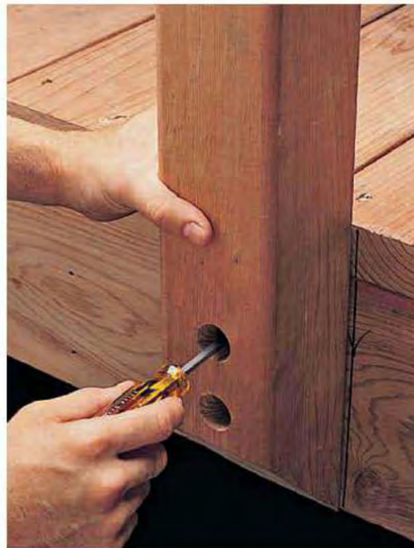
6. Position each post with beveled end flush with bottom of deck. Plumb post with a level. Insert a screwdriver or nail into pilot holes and mark side of deck.
