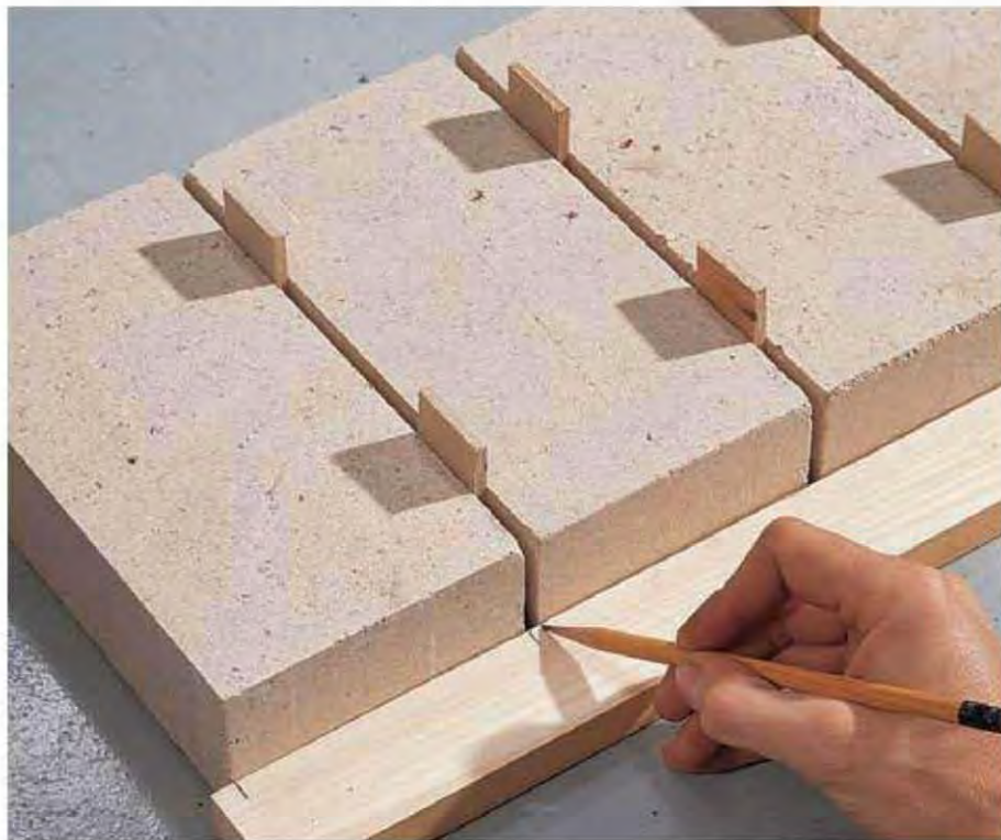
B. To make a story pole, mark one side of a straight board for eight courses of fire brick, leaving a \frac{3}{8} " gap for the bottom mortar joint and \frac{1}{8} " gaps for the remaining joints.
