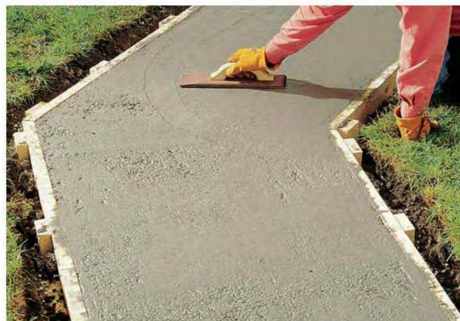
9. Smooth the concrete surface with a wood float. The goal is to smooth it, not to level it. (You should maintain the slight crown created by the curved screed board.)
