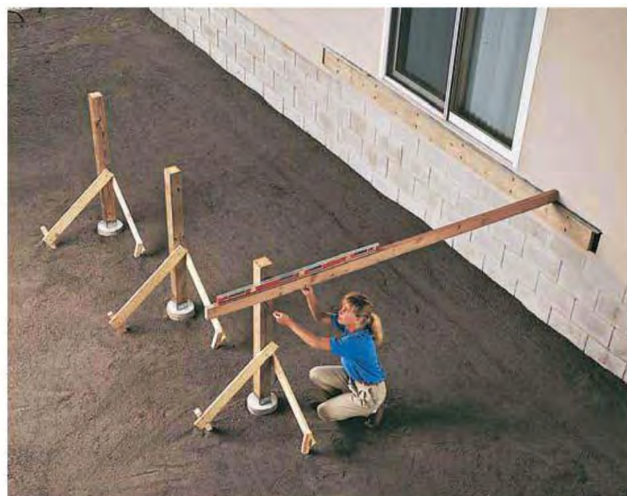
2. Pour concrete post footings (page 190), and install metal post anchors. Set and brace the posts, attach them to the post anchors, and mark posts to show where beam will be attached.
