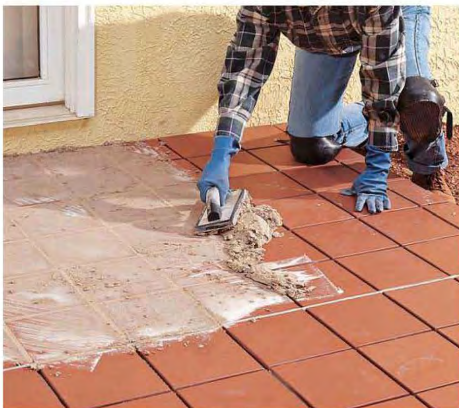
K. Mix a batch of tile grout to the recommended consistency and use a grout float to pack it into tile joints.
