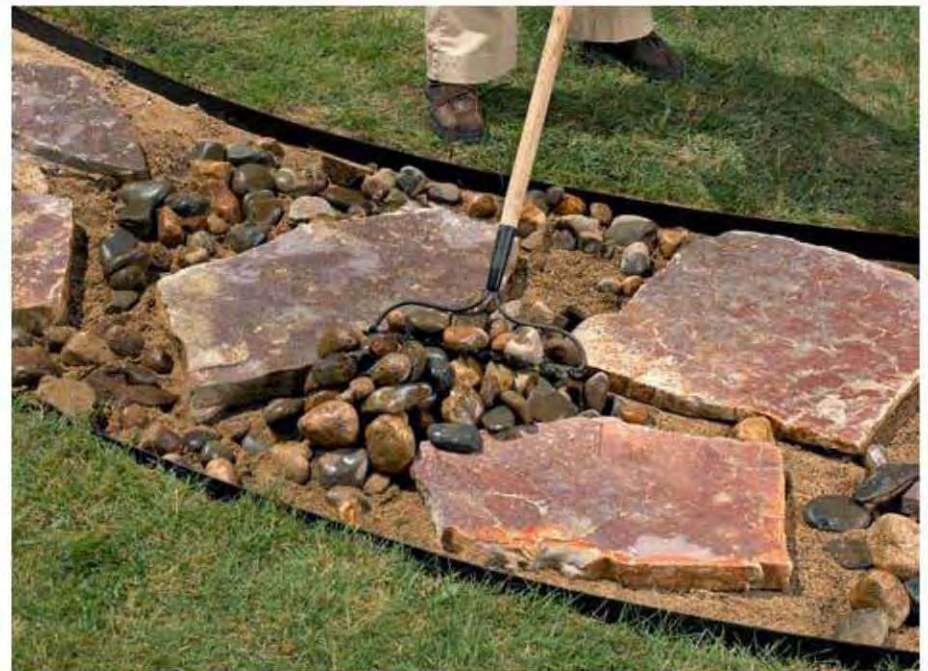
3. If you're using two or more sizes of infill, start by spreading out a layer of the largest diameter rock.
