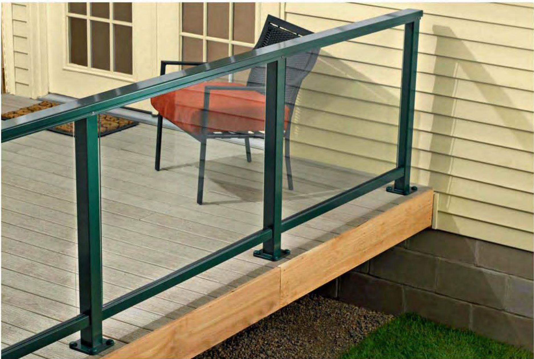
Tempered glass panels are both DIY friendly and code approved, provided you install them according to the manufacturer's guidelines.
