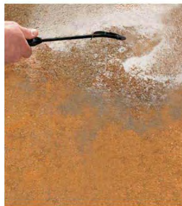
3. Apply a sealer using a hand-pump sprayer.
