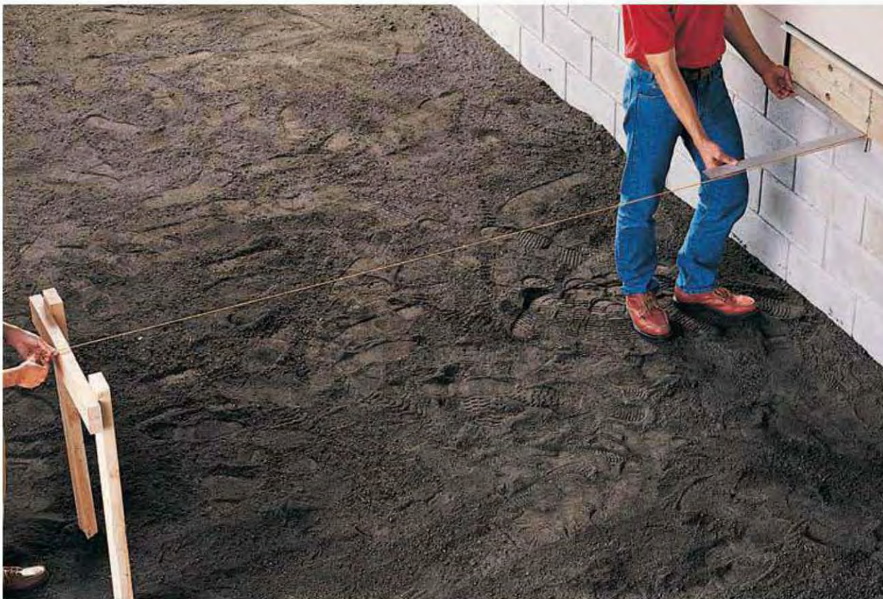
7. Extend the mason's string so that it is taut and perpendicular to the ledger. Use a framing square as a guide. Secure the string temporarily by wrapping it several times around the batter board.
