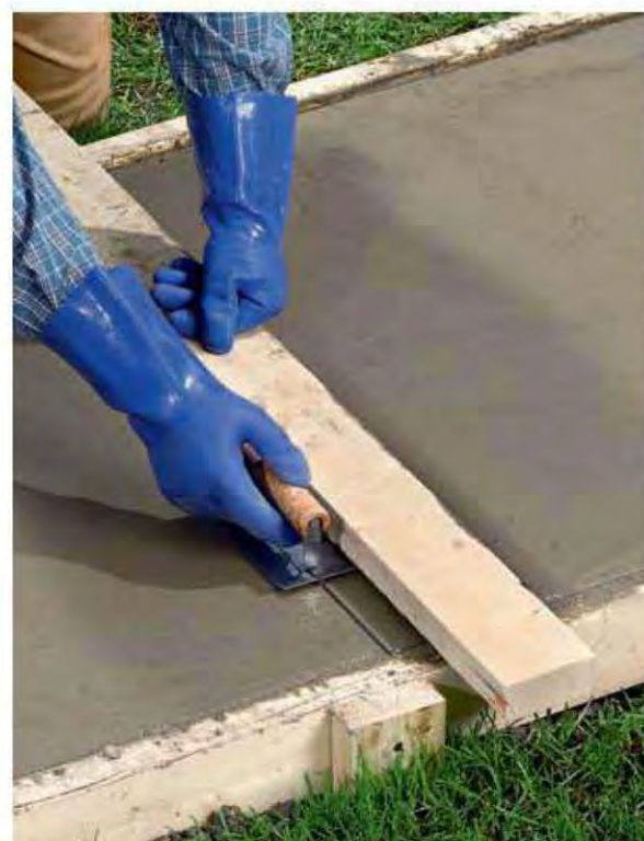
11. Cut control joints in the concrete after the concrete sets up, but before it hardens.
