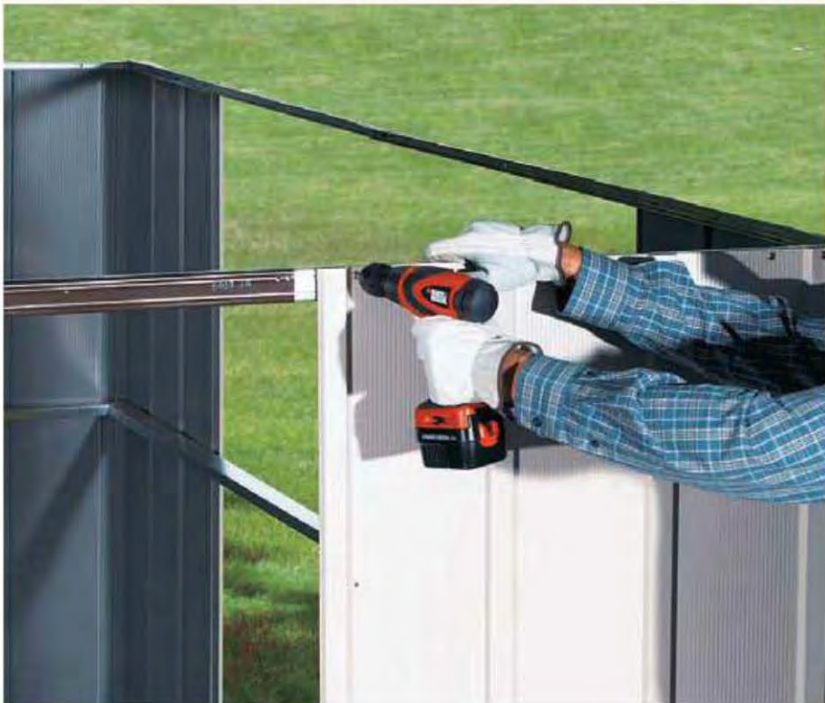
10. Fasten the shed panels to the top frames, making sure that any fasteners holes are aligned and that crimped tabs are snapped together correctly.
