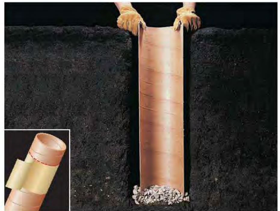
D. Wrap paper around the form to mark a straight cutting line (INSET). Set the forms in the holes on top of a 4" gravel layer.
