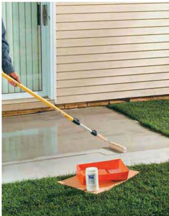
A. Thoroughly clean the concrete slab, then apply a concrete bonding agent.
