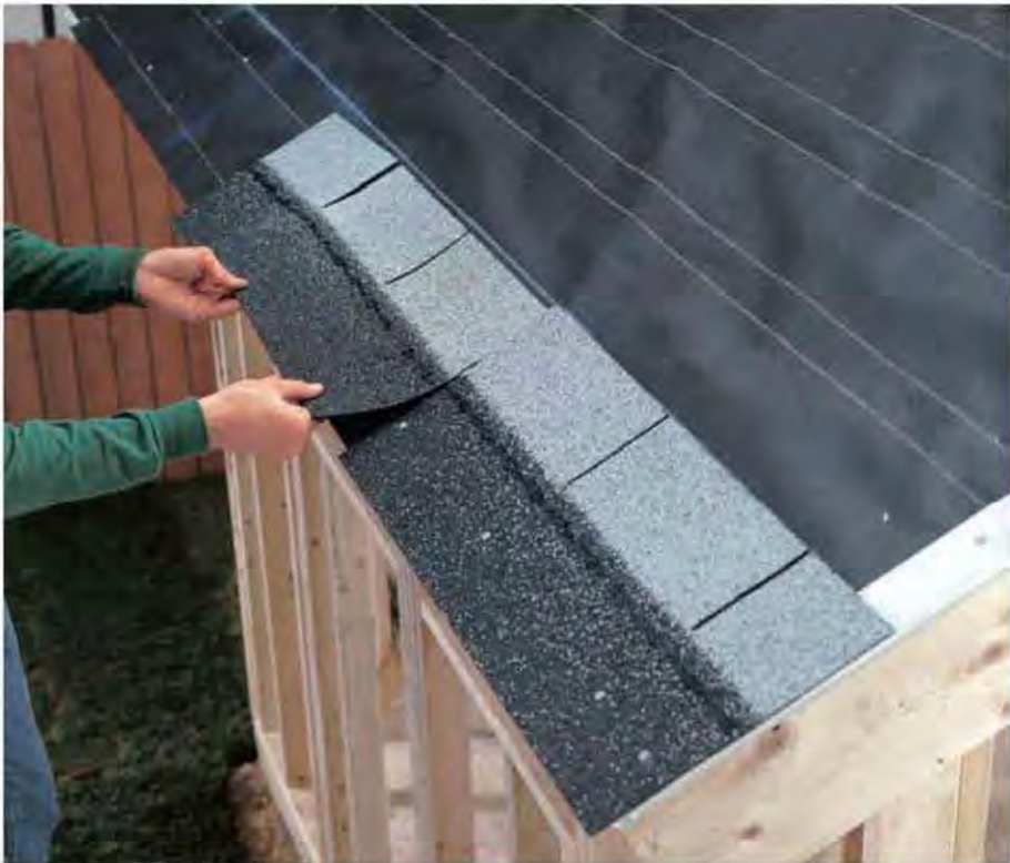
B. Trim 6" from the end tab to begin the starter row. Position the starter row shingles upside-down so the tabs point up.
