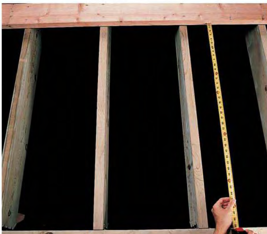
5. After every few rows of decking are installed, measure from edge of the decking board to edge of header joist. If measurements show that the last board will not fit flush against the edge of the deck, adjust board spacing.
