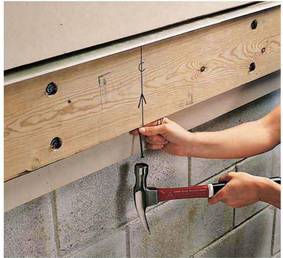
6. Drive a 10d nail into bottom of ledger at reference point (step 4). Attach a mason's string to nail.
