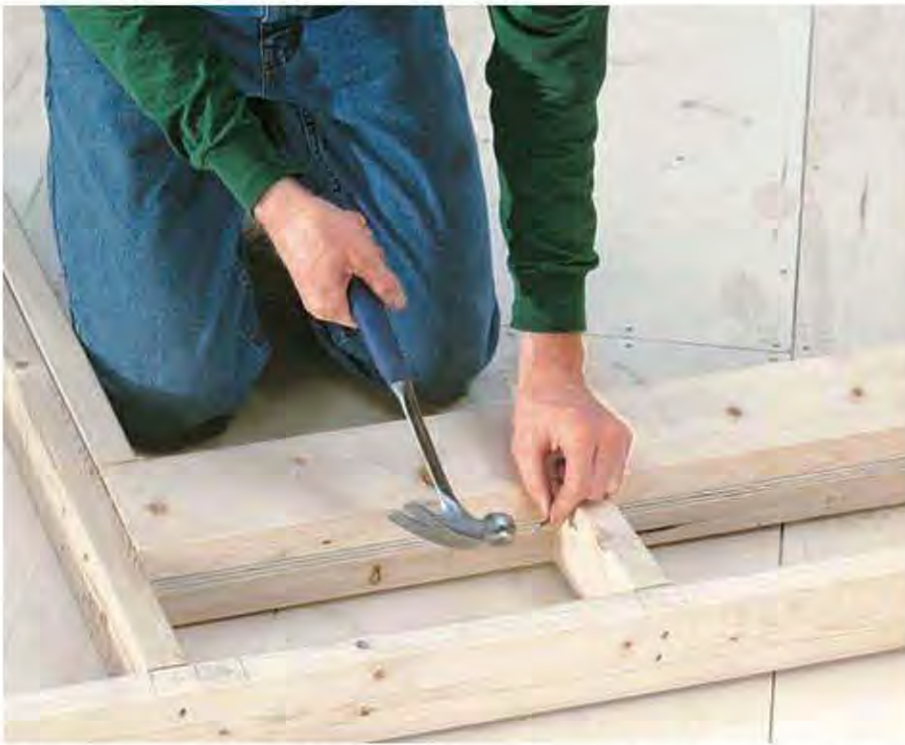
D. Frame the walls with 16d nails endnailed through the plates into the studs. Toenail cripples to headers with 8d nails.
