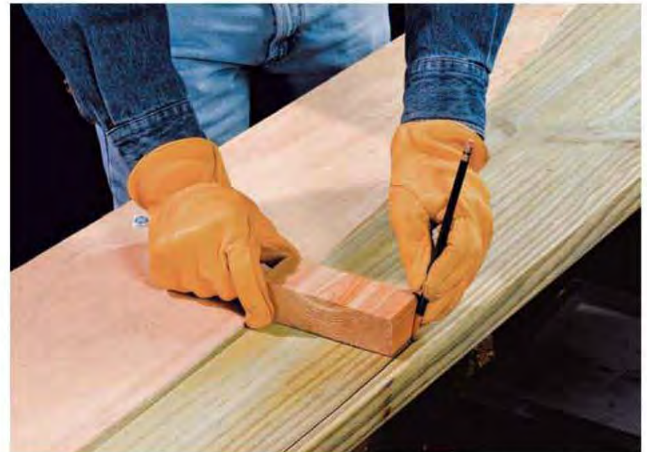
Cut a 2"-wide piece of 2 × 6 lumber and use it as a spacer to mark the outside curve for the inner tread.
