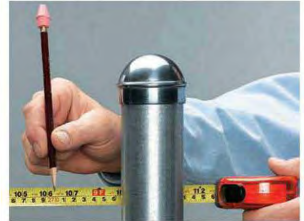
6. To fit the last piece of top stringer in the section, measure from where the taper begins on the previous piece to the inside back wall of the stringer end cup. Cut a piece of top stringer to fit.
