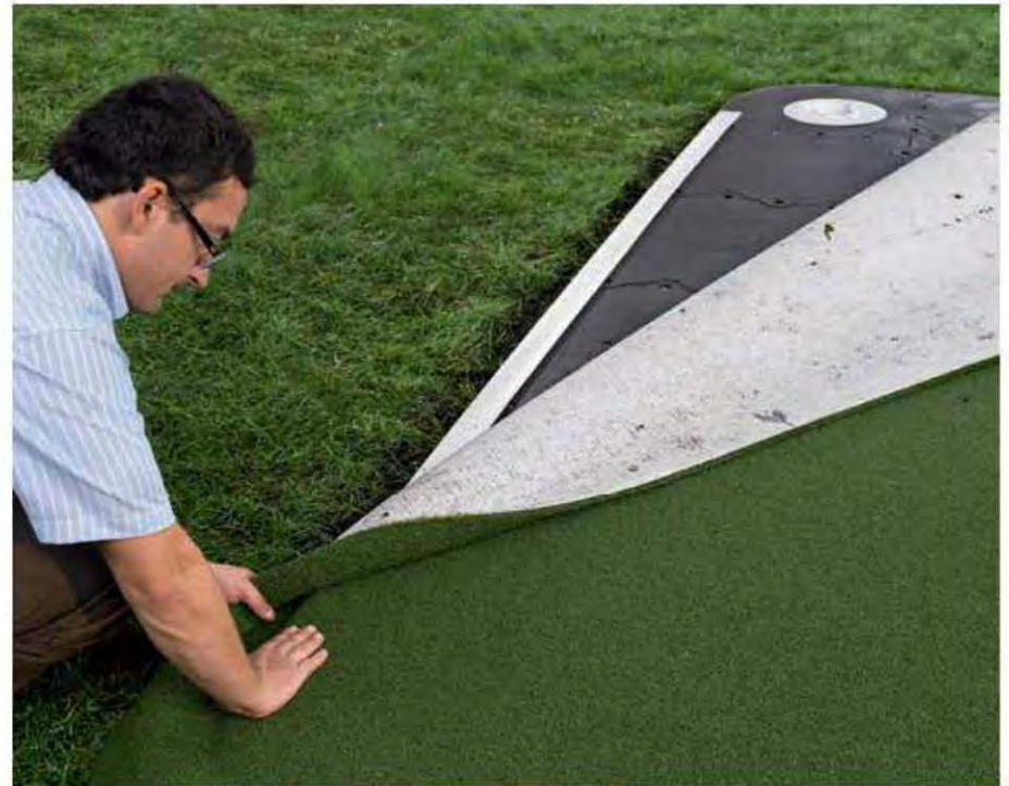
14. Fold back the edges of the turf. Apply double-sided carpet tape to the perimeter of the panel assembly. Peel off the tape's protective cover, then press the turf down onto the tape. Fold the excess turf over the edge of the panel assembly and down into the trench. If the turf bulges around a tight radius, make 3½" slashes in the edge of the turf and ease it around the curve.
