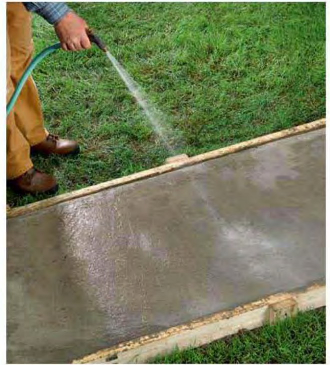
13. Keep concrete damp by spraying periodically with a fine water mist or cover with plastic sheeting for five to seven days.
