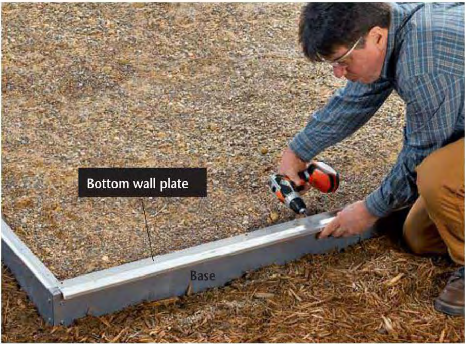
4. Attach the bottom wall plates to the base pieces so that the flanged edges face outside the greenhouse. In most systems, the floor plates will interlock with one another, end to end, with built-in brackets.
