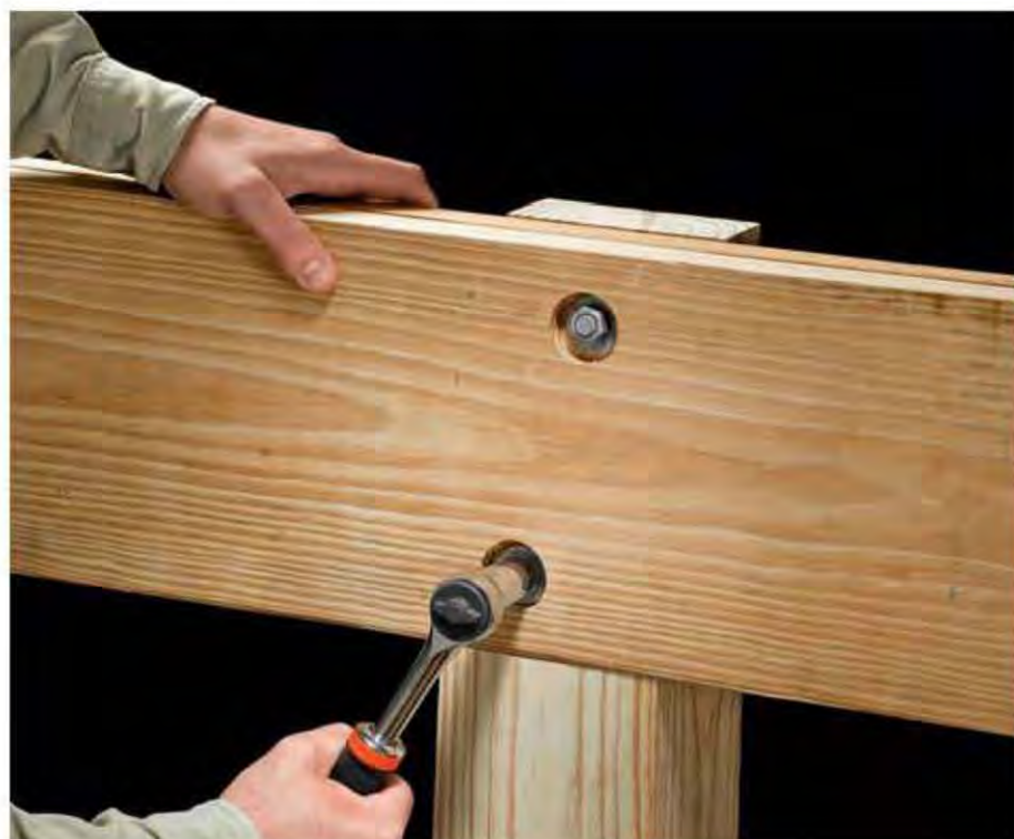
Use ½"-dia. or larger through bolts, washers, and nuts for fastening beams to posts or railing posts to joists. They should be galvanized or made of stainless steel for corrosion resistance.
