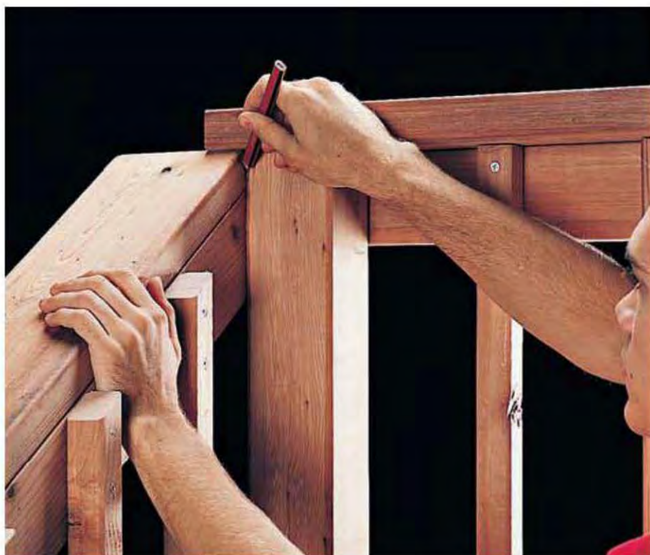
28. Measure and cut cap for stairway rail. Mark outline of post on side of cap and bevel cut the ends of the cap.
