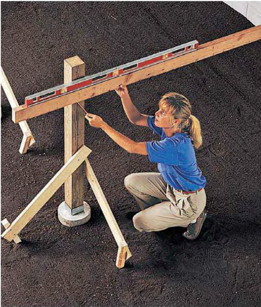
C. After the posts have been set in place and braced plumb, use a straight 2 × 4 and a level to mark the top of the beam on each post.
