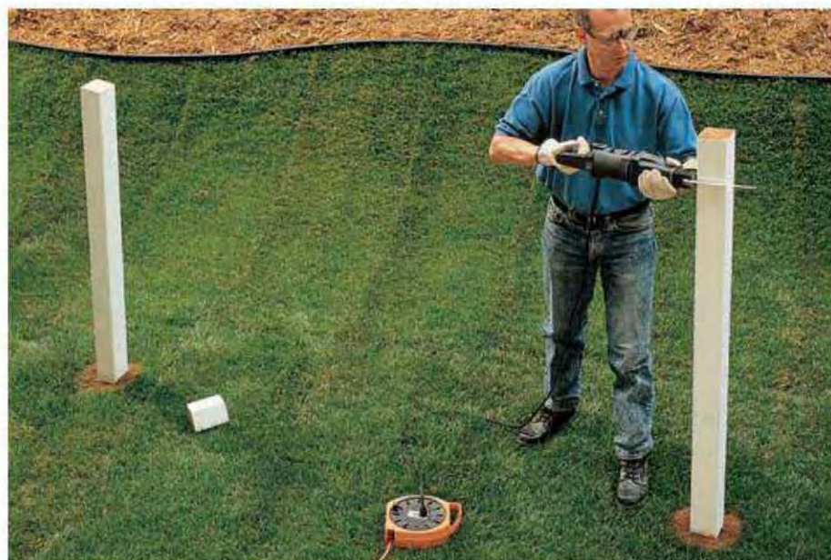
B. Set the posts, then mark cutoff lines and trim them to 48" above ground level.
