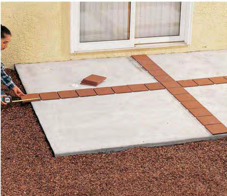
F. Adjust the tile to create a layout that minimizes tile cutting. Shift the rows of tiles and spacers until the overhang is equal at each end and any cut portions are less than 2" wide.
