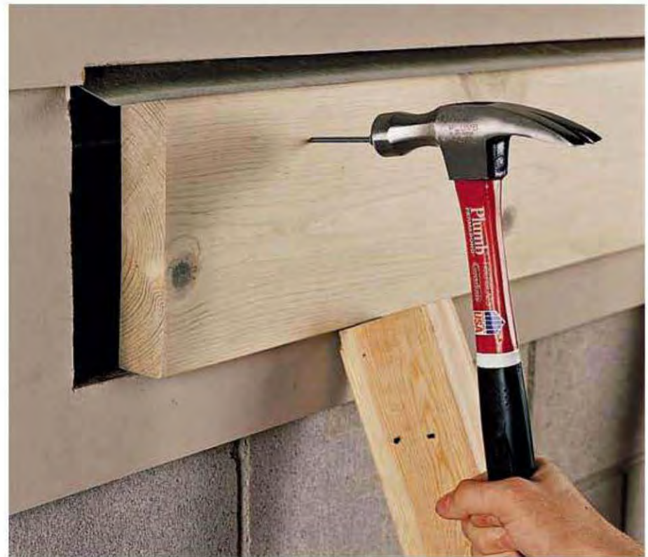
6. Center the ledger in the cutout, underneath the flashing. Brace in position, and tack ledger into place with 8d galvanized nails. Apply a thick bead of silicone caulk to crack between siding and flashing.
