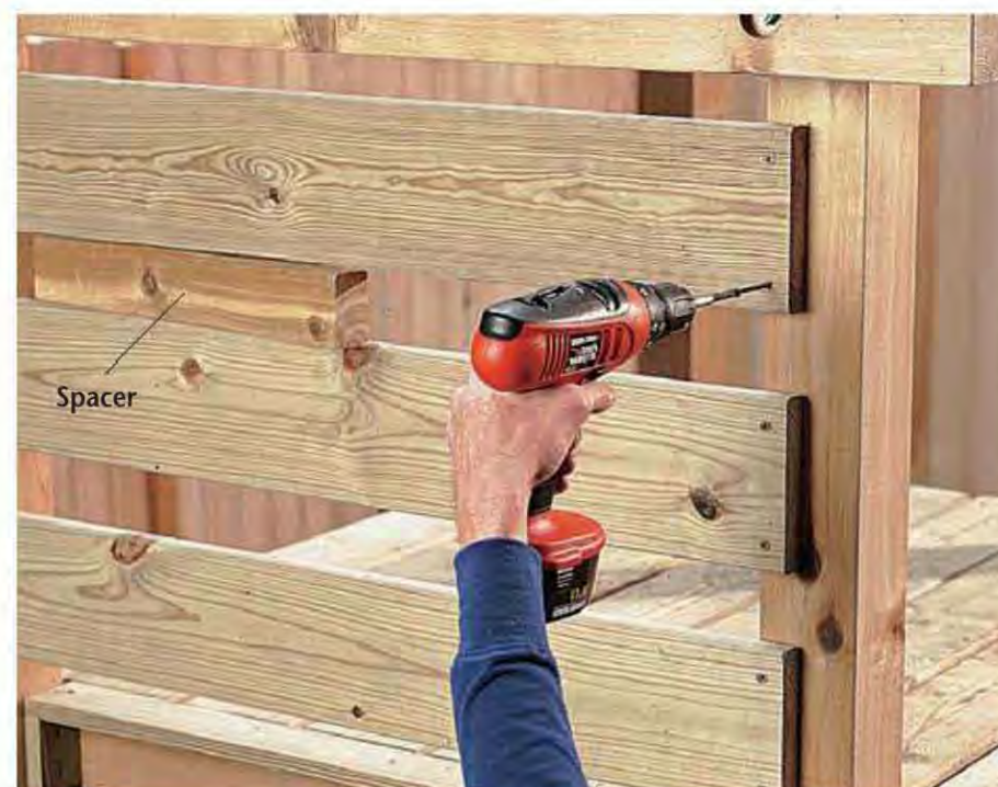
I. Install stringers between the posts in the clubhouse tower over any opening that does not house any accessories. Fasten to the posts with deck screws.
