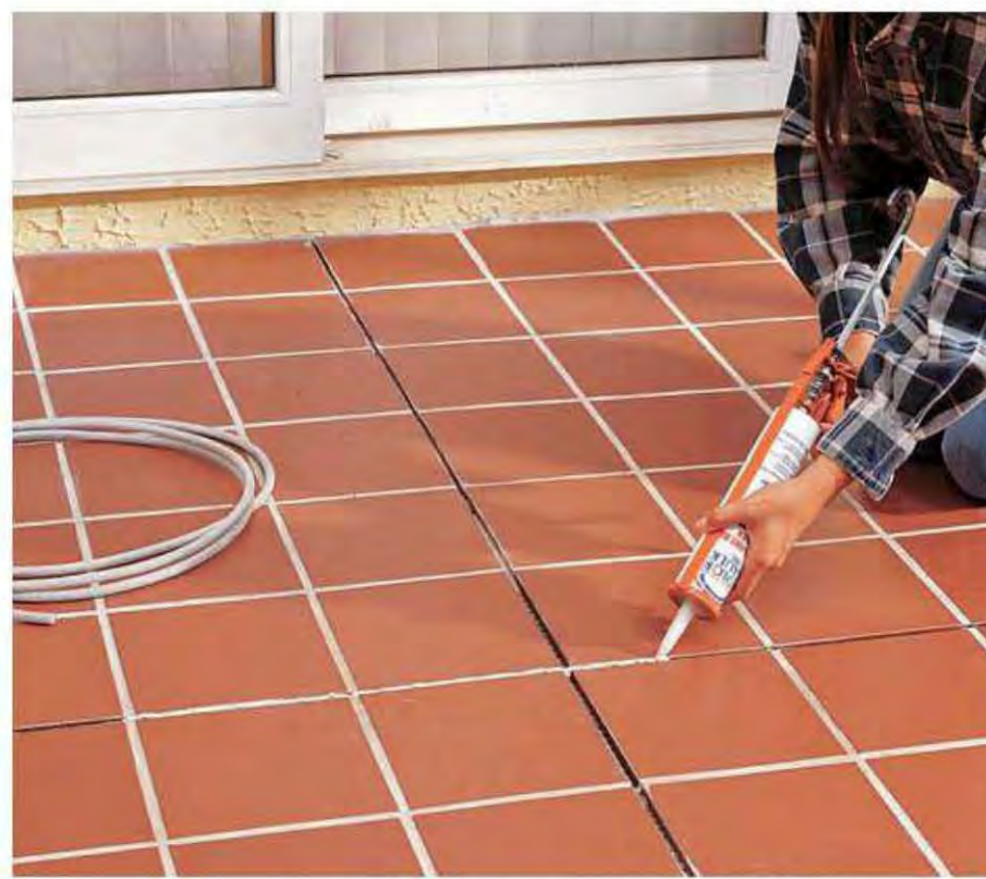
L. Remove the caulking backer rod, then fill the joints with caulk that is tinted to match the grout color. Apply grout sealer, then seal the entire surface with tile sealer after one to three weeks.
