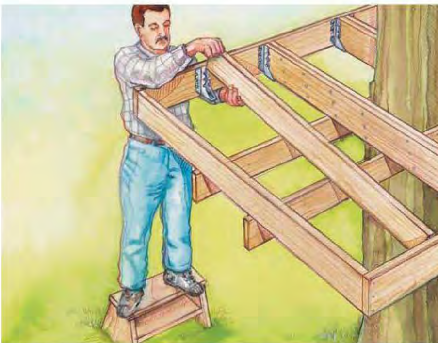
B. Mark the midpoints between the joists, install joist hangers, then set the joists in the hangers and nail them in place.
