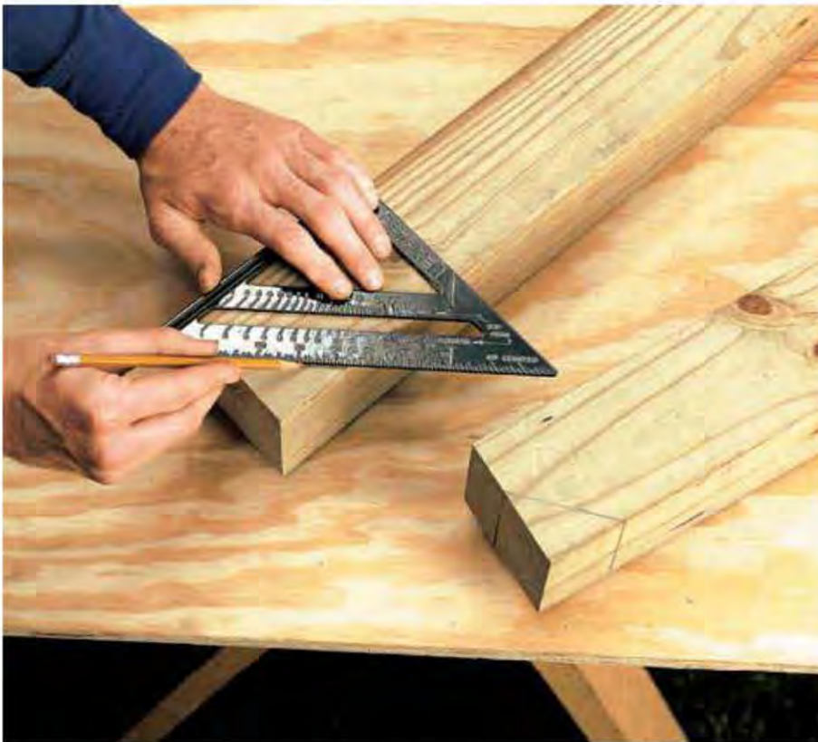
B. If desired, mark and clip the bottom corners of the skid ends. Use a square to mark a 45° angle cut.
