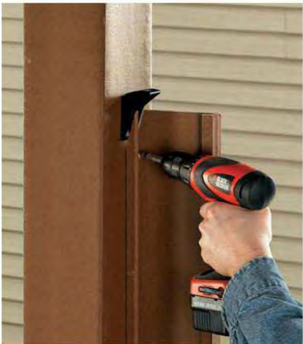
8. The initial siding strip fits inside the upper bracket and is screwed to the fence post.
