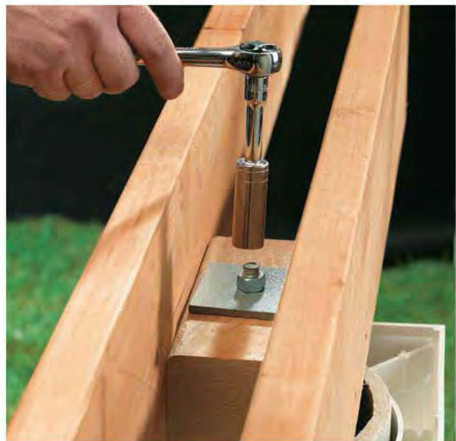
E. Center the column at both ends, then tighten the nut over the bearing plate to secure the entire assembly.
