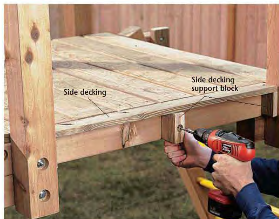
H. Position a support block flush with the bottom of the side decking and attach to the lower beam with a 3" deck screw. Attach the side decking to the block with 2\frac{1}{2} " deck screws.
