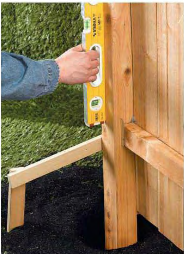
9. Plumb the post perpendicular to the fence line, making sure the panel is level. Brace the post, recheck for plumb and level, and then set the post the same way you set the first one.
