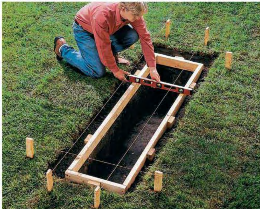
3. Build and install a 2 × 4 form frame for the footing, aligning it with the mason's strings. Stake the form in place, and adjust to level.
