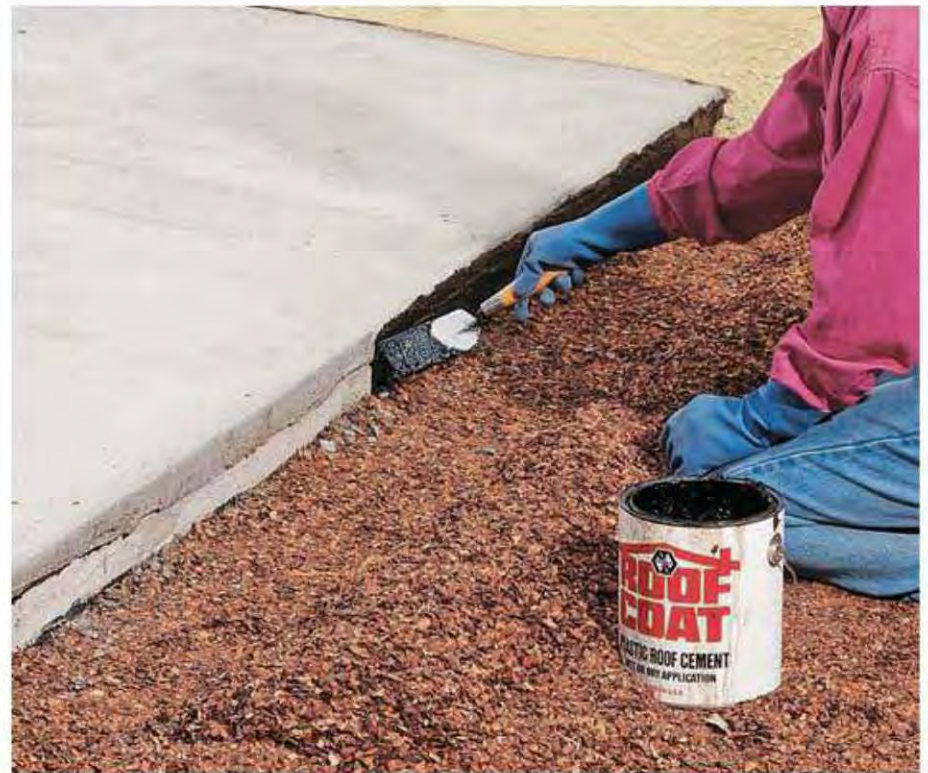
E. After curing is complete, remove the plastic, disassemble and remove the forms, and trim off the building paper around the sides. Apply roofing cement to two sides of the subbase.
