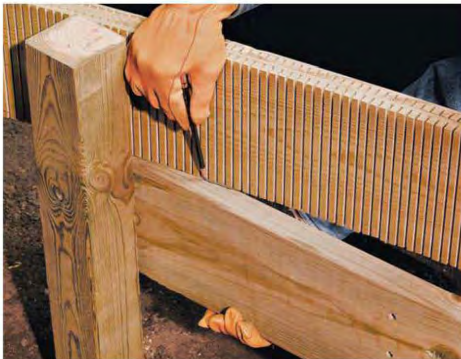
Mark the profile of the inner face of the curved rim joist on each end of the 2 × 8 for the inner joist at the curve. Cut the joist at the marks, then fasten to the posts with carriage bolts and to the curved rim joist with deck screws.
