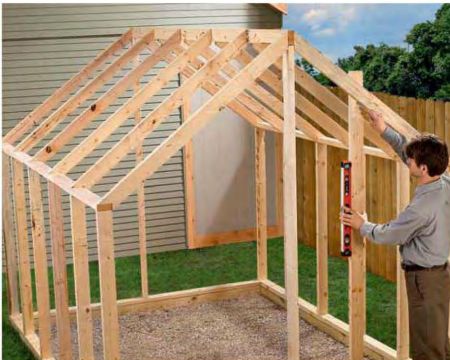
10. Mark the positions for the remaining end wall studs on the base plate. At each location, hold a 2 x 4 on end on the base plate and make it level and plumb. Trace a cutting line at the top of the 2 x 4 where it meets the rafter. Cut the studs and install them by driving screws toenail-style.
