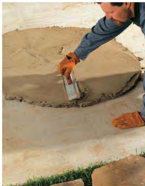
C. Move some of the stones aside, then apply mortar for setting the first few stones.
