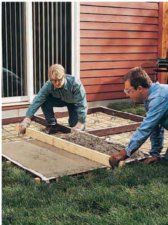
C. Pour concrete into the first quadrant and screed the concrete smooth with a 2 × 4 that rests on top of the form.
