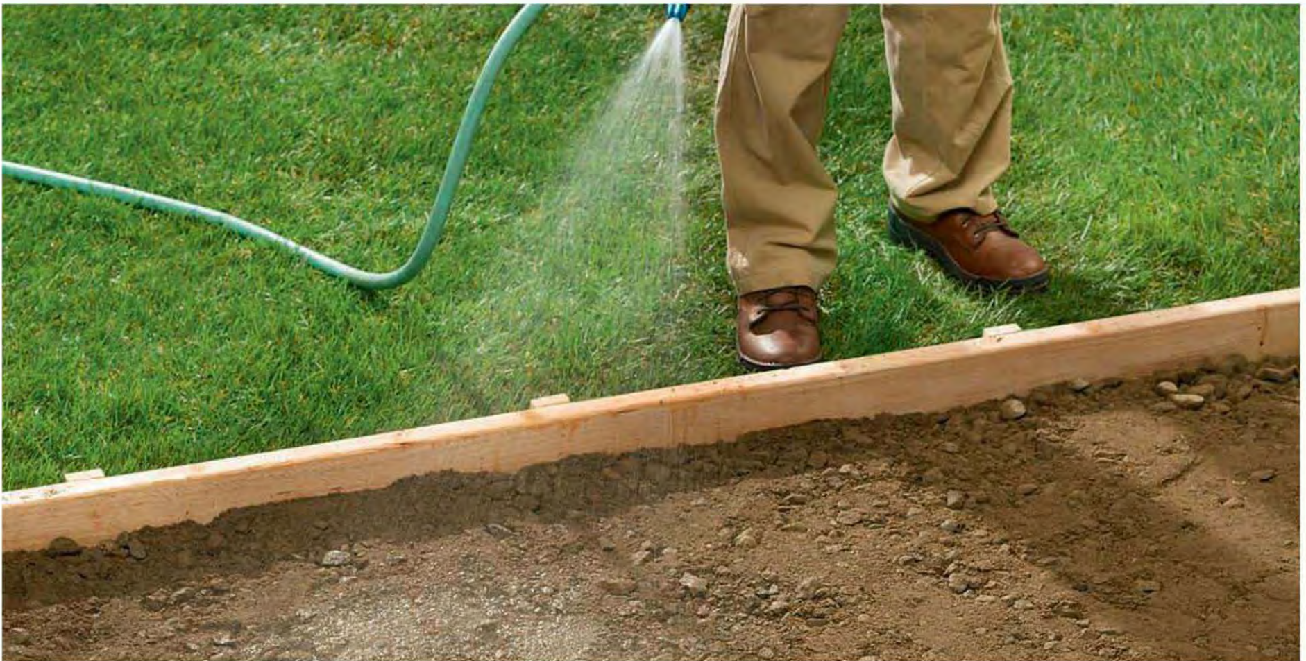
5. Prior to placing concrete, it is necessary to dampen the gravel subbase. Spray the subbase using a water hose until saturated but do not leave standing water.
