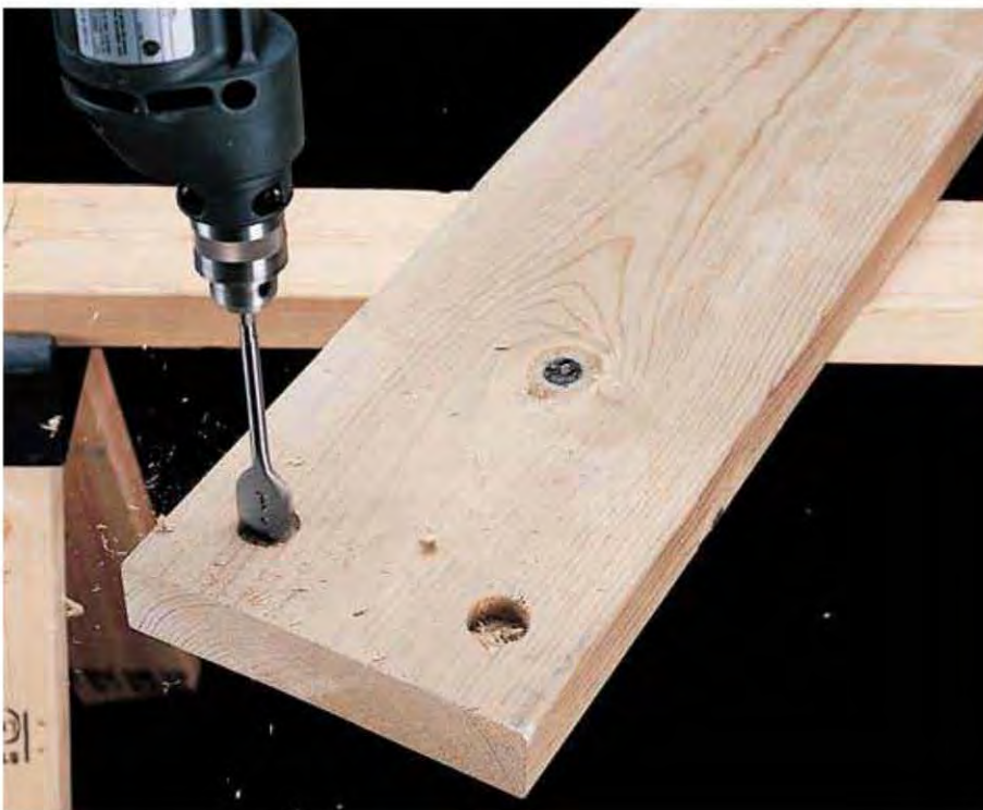
1. Measure and cut ledger. Ledger will be shorter than overall length of outline. Drill pairs of \frac{1}{4} " pilot holes every 2 feet in ledger. Counterbore each pilot hole to \frac{1}{2} " depth using a 1" spade bit.
