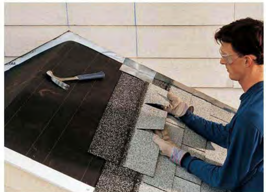
E. Continue to shingle and flash the roof, maintaining a regular shingle pattern with a consistent exposed area on the shingle tabs.
