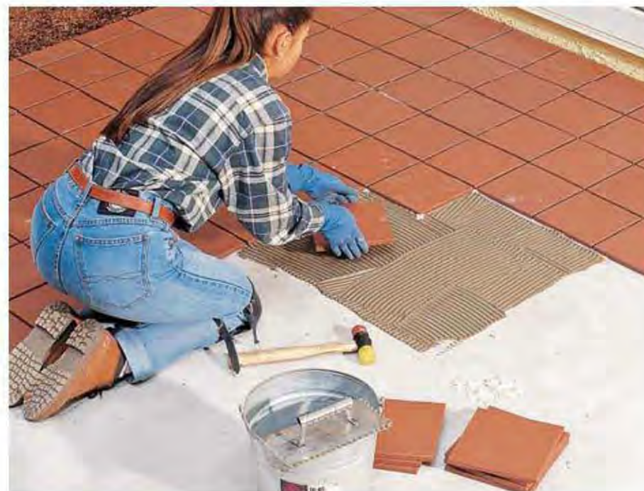
I. Fill in the remaining quadrants, using a straightedge to check joints occasionally. If any of the joint lines are out of alignment, compensate over several rows of tiles. After all tiles are set, remove spacers.
