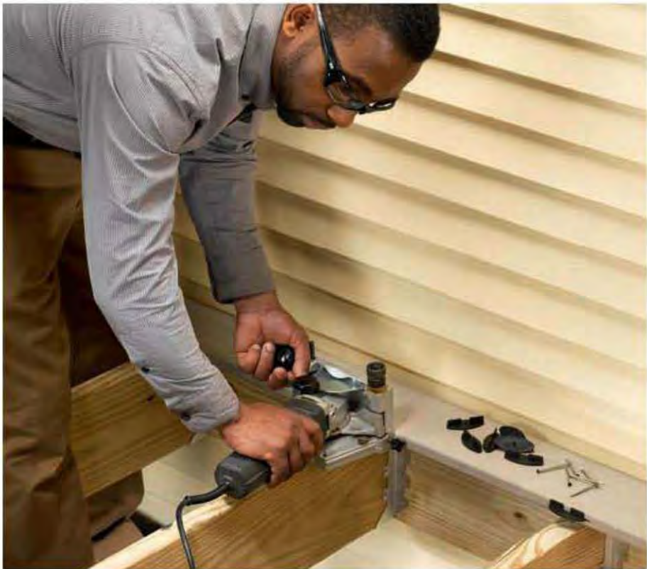
1. Cut a #20 biscuit slot into the edge of deck boards at each joist location using a biscuit joiner (plate joiner). Set the slot height so the bottom edge of the biscuit clip will touch the joist edge.
