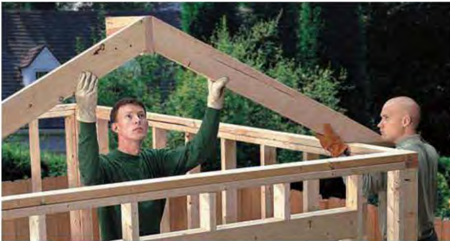
D. Test-fit the pattern and duplicate rafters using a 2× spacer to represent the ridge board.
