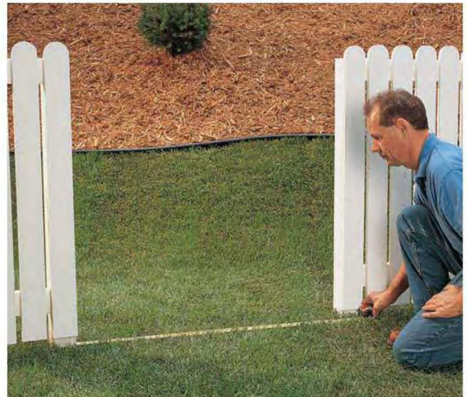
A. Make sure the gate posts are plumb, then measure the distance between them and calculate the dimensions of the gate.
