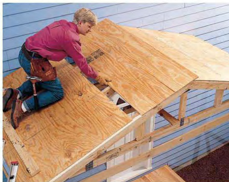
A. Install plywood roof sheathing, working from the rafter tails to the peak. Leave a \frac{1}{8} " gap between sheets and a \frac{1}{4} " at the peak.
