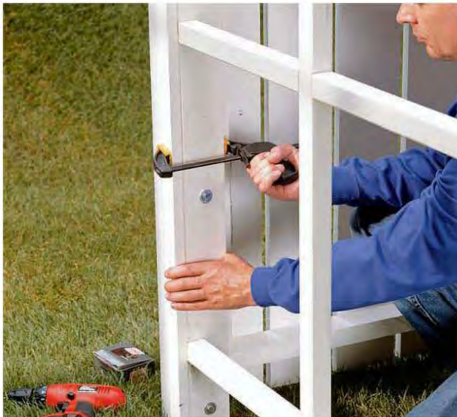
I. Clamp a 1 × 2 to the latch-side gate post and secure with 1½" galvanized deck screws.
