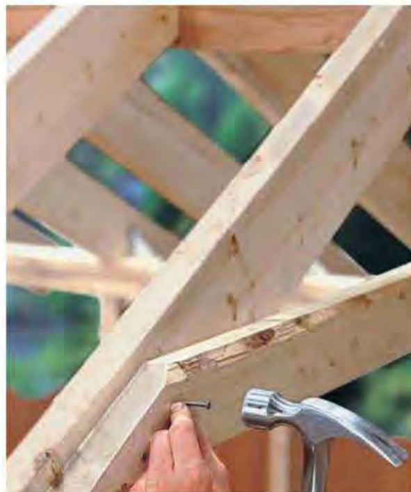
G. Angle-cut the ends of the collar ties to match the roof slope and facenail the ties to the rafters.
