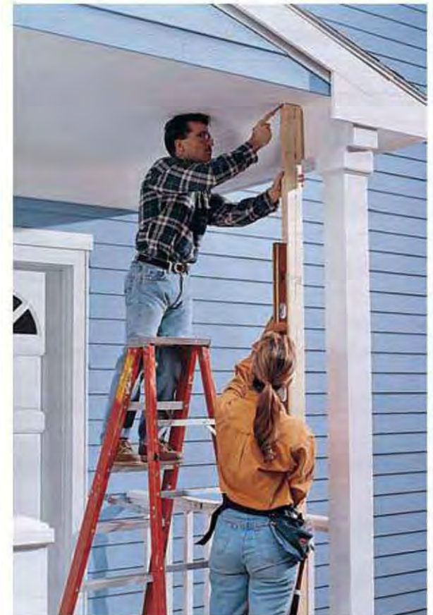
C. Mark the locations for the top plates on the ceiling directly above the sole plates using a straight 2 × 4 and a level.
