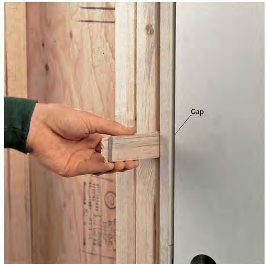
B. Shim the latch jamb, using the gap between the door and the jamb as a gauge. Make sure the gap is consistent.
