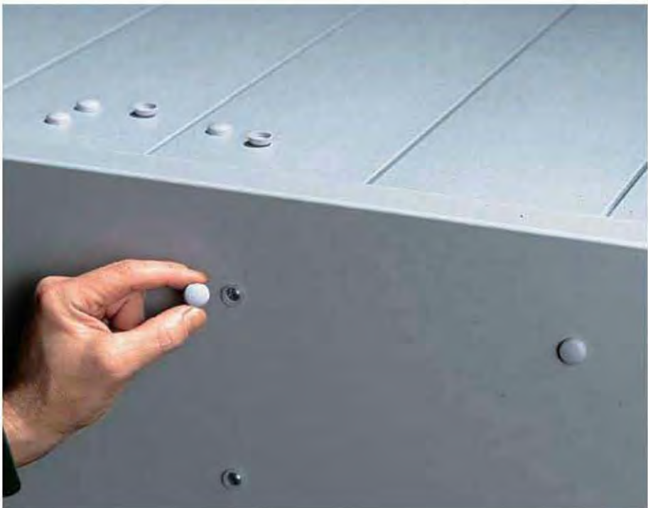
4. Use 2" galvanized deck screws to attach the pre-fabricated facing, covering the exposed hollow ends and creating a decorative trim. Cover the screw heads with the screw caps.
