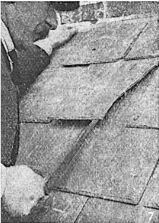
Fig. 7. How to remove old or broken slates with the tool shown above.
