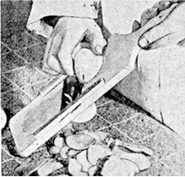
Potato Cutter which cuts fancy shapes, mainly for purposes of garnishing. Left, device for slicing potatoes finely and quickly for potato crisps.
