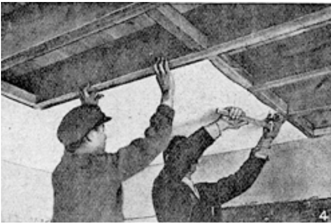
Panelling. Fig. 4. Applying the ceiling boards before panelling with strips of wood.
