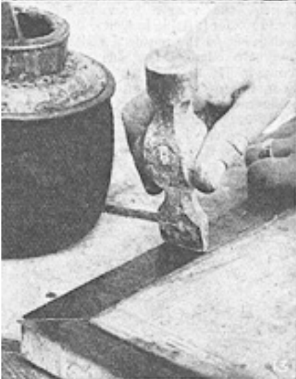
Veneering. Fig. 11. Raising one piece of veneer and removing waste after cutting with chisel. Fig. 12. Alternative method of holding hammer, with one hand; compare with Fig. 5. Fig. 13. Laying banding, using the back of an ordinary hammer to press out the superfluous glue.
