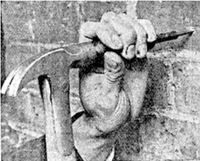
Fig. 1. Plug. Fig. 1. Making hole for fibre plug with borer.
