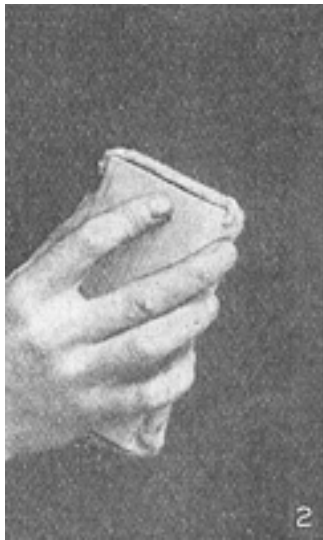
Varnishing a Door. Fig. 1. Working the first coat on the panels with a flat brush. Fig. 2. Using the felting pad between the two coats of varnish. The motion of the hand should be circular.
