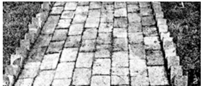
Path. Fig. 1. Making a brick path. The coarser soil is first rammed down, and above this the bricks are bedded, either in sand, as shown, or in mortar. Fig. 2. The finished path after grouting with cement.
