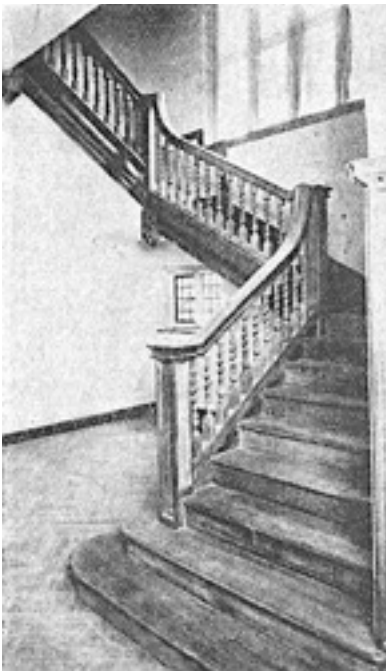
Staircase. Fig. 3. Well staircase of modern construction; a simple and dignified arrangement.
