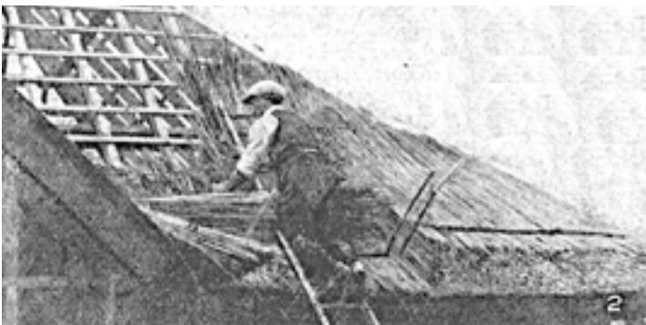
Thatching. Fig. 1. Roof prepared by nailing wooden runners to the joists. Fig. 2. Thatching begun by sewing the straw with twine to the runners. Fig. 3. Laying a plaited ridge roll, one way of finishing off the apex of the roof. (Courtesy of Boulton & Paul. Ltd.)
