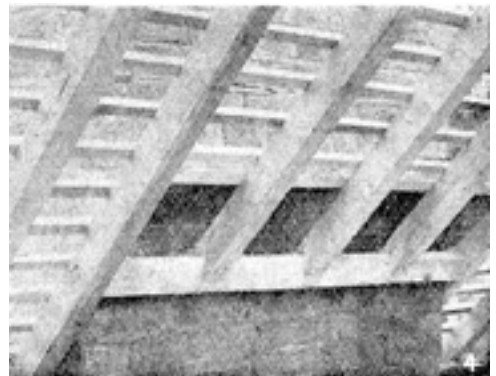
trimmed round a chimney stack.
