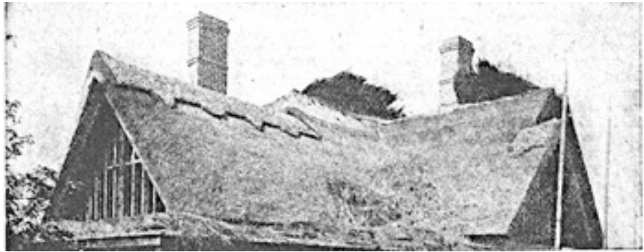
Fig. 4. Thatched roof nearing completion. Note the ornamental finish of the ridge stack, and how the thatch overhangs the gable ends of the roof. (Courtesy of Boulton & Paul, Ltd.)
