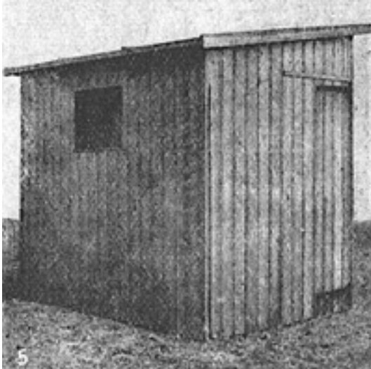
Shed. Fig. 3. Exterior view of a sectional span roof workshop or tool shed. Fig 4. The same partly erected, showing method of assembling the sections. Fig. 5. Useful lean-to shed made up on the same principle. (Courtesy of Alfred Turrell & Sons)
