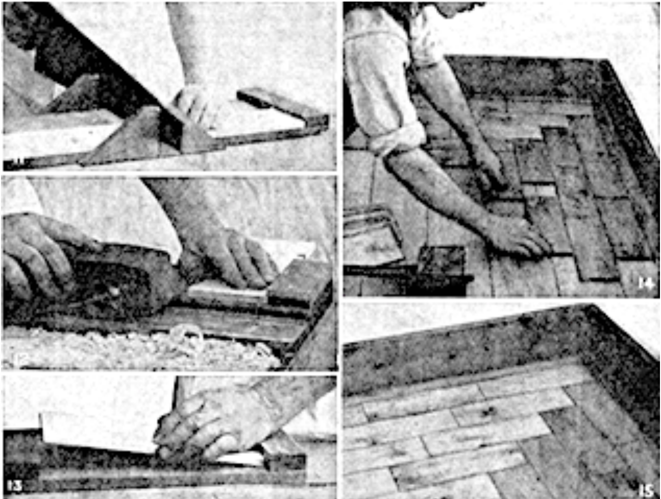
Parquet. Simple wood block flooring which the home worker can prepare. Fig. 11. Cutting strip to length with a sawing guide. Fig. 12. Planing the ends of the blocks. Fig. 13 Testing for length with a simple gauge. Fig. 14. Laying and fitting the blocks. Fig. 15. Corner of floor when completed.
