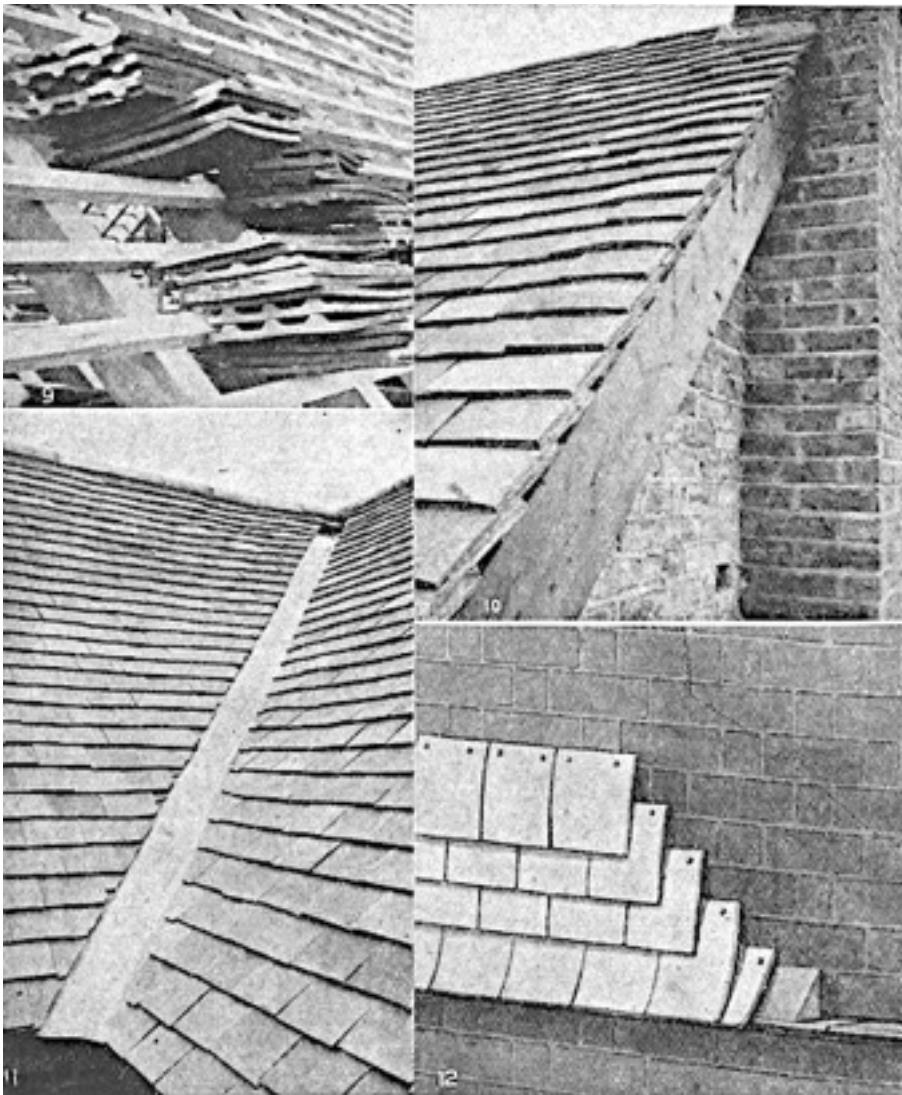
Tile. Fig. 9. Showing how to stack tiles on rafters ready for use. Fig. 10. Verge with tiles in place and cement fillet around chimney stack. Fig. 11. Tiles cut to form simple valley gutter. Fig. 12. Showing how lowest courses of tiles on a tile-hung wall should be tilted.
