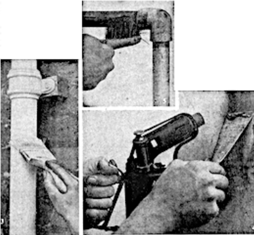
Paint. Fig. 3. Applying anti-rust priming to a rain-water pipe. Fig. 4. Process of burning and scraping off the old paint by means of a blow lamp and stripping-knife. Fig. 5. Cleaning radiator pipes with a wire brush before applying a new coat of paint.
