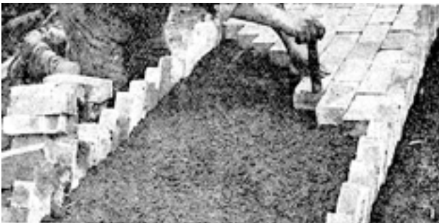
Path. Fig. 1. Making a brick path. The coarser soil is first rammed down, and above this the bricks are bedded, either in sand, as shown, or in mortar. Fig. 2. The finished path after grouting with cement.
