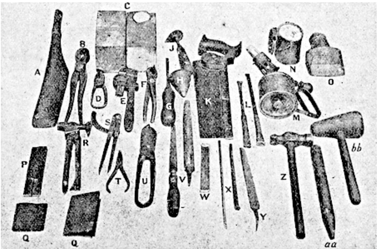
Plumbing. Fig. 1. Plumber's tools. A, dresser. B, gas tongs. C, wood blocks. D, snips. E, wrench. F, gas pliers. G, screwdriver. H, tan pin. J, shave hook. K, back saw. L, chisels. M, blow lamp. N, paste. O, stake. P, lead. Q, wiping cloths. R, combination wrench. S, compasses. T, pliers. U, shears. V, rasps. W, cold chisel. X, fixing points. Y, knife. Z, hammer; aa, opening rasp, bb, mallet.
