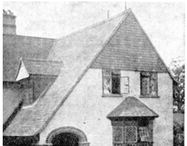
Top right, mansard type of roof. Right, tiled gable end with edge tiles arranged on Winchester underhang system.
