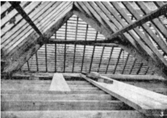
Roof: stages in construction. Fig. 1. Showing how ends of rafters and ceiling joists fit to the plate. Fig. 2. Valley board and common rafters in place.
