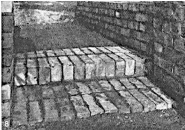
Fig. 7. How side walls are bonded together. Fig. 8. First two steps completed. Fig. 9. Heading course set on side wall and steps nearing completion.
