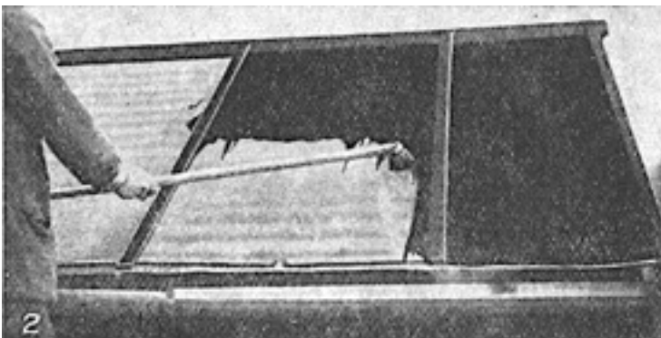
Fig. 2. Tarring a roof with a stiff-bristled brush fixed to a long handle.
