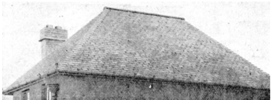
Pavilion roof, with four sides sloping to the ridge. Above valley roof on two semi-detached houses.
