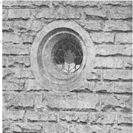
Circular window, an interesting combination of tooled stone with rock-faced stonework.
