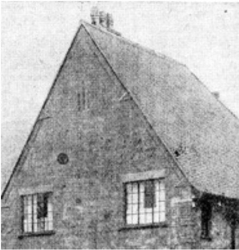
Top right, mansard type of roof. Right, tiled gable end with edge tiles arranged on Winchester underhang system.
