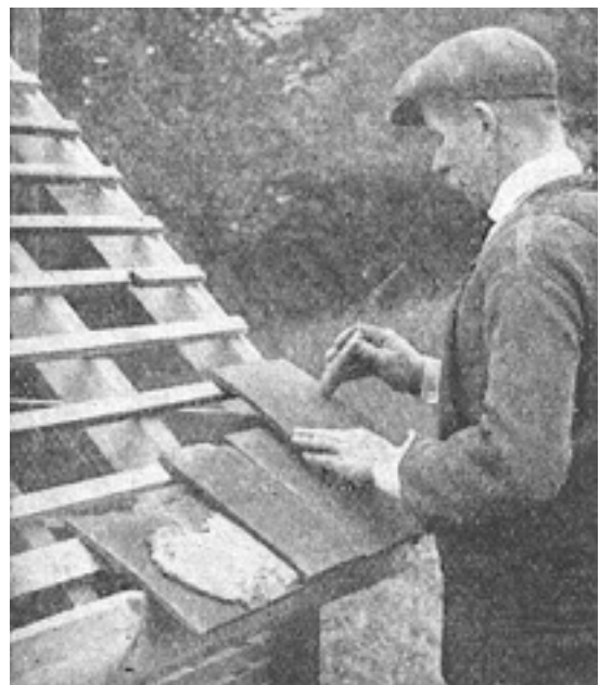
Tile. Fig. 8. Setting the tile-and-a-half tile for the start of the second course.
