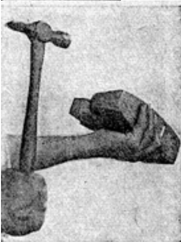
Left. Loosening the wedge of a smoothing plane.
