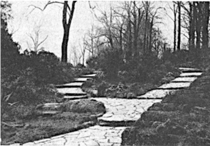
Steps. Fig. 1. Picturesque effect achieved by the use of crazy paving for a path which rises gradually in shallow steps. Fig. 2. Steps connecting different levels in a small garden; they are of crazy paving finished on the edges of the treads with hewn flagstone.
