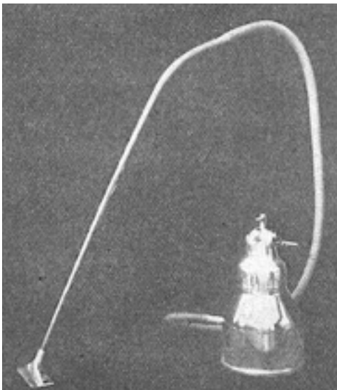
Fig. 3. In this model the usual type of dust-bag is replaced by a sanitary steel canister. Another fixture which makes for efficiency is the patent hinged nozzle. (Tellus Super Vacuum Cleaner Ltd.)
