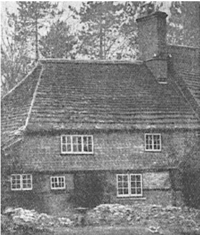
Stone. Fig. 6. Part of an old Sussex house with a picturesque roof consisting of thin slabs of Horsham stone.
