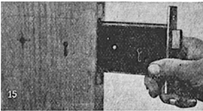
Fig. 15. Fitting mortise lock into door.
