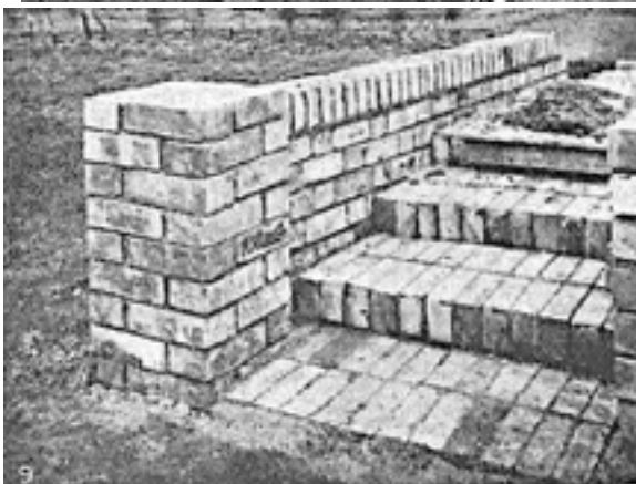
Fig. 7. How side walls are bonded together. Fig. 8. First two steps completed. Fig. 9. Heading course set on side wall and steps nearing completion.
