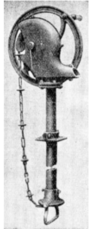
Fig. 7. Endless chain pump for thick liquids. (Joseph Evans & Sons. Ltd.)
