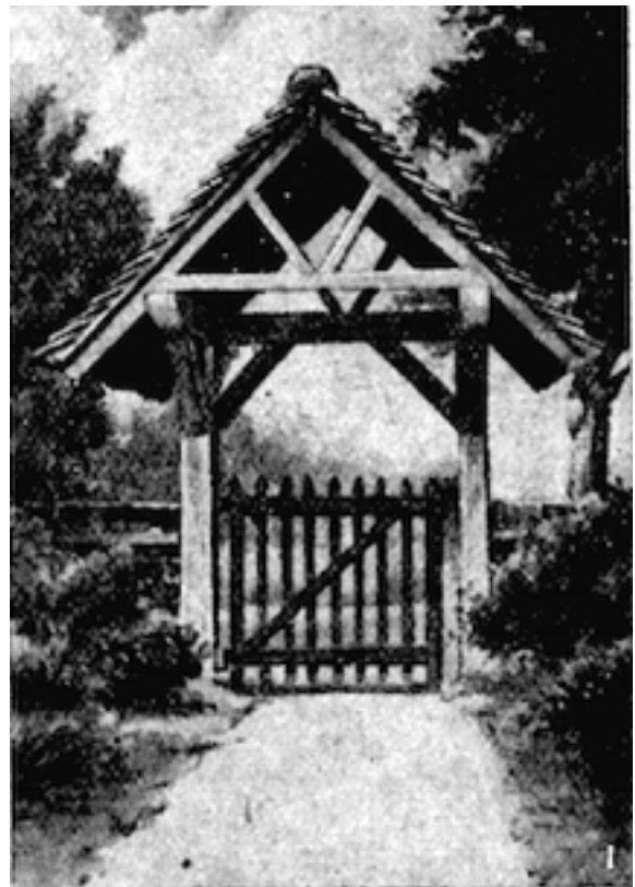
Lych Gate. Fig. 1. Lych gate with a tiled roof which can be easily built by the amateur worker.
