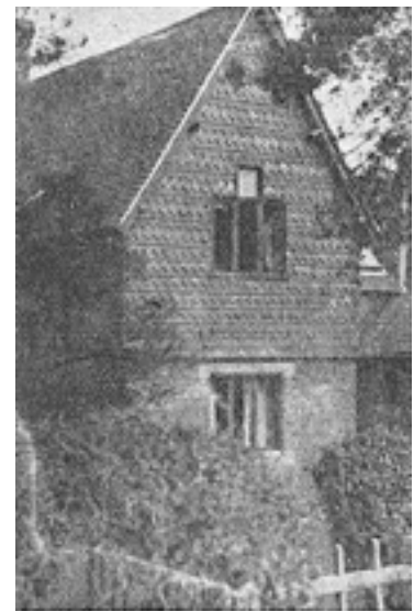
Fig. 13. Attractive effect of a cottage tile-hung with dark red sandfaced tiles of an ornamental pattern.
