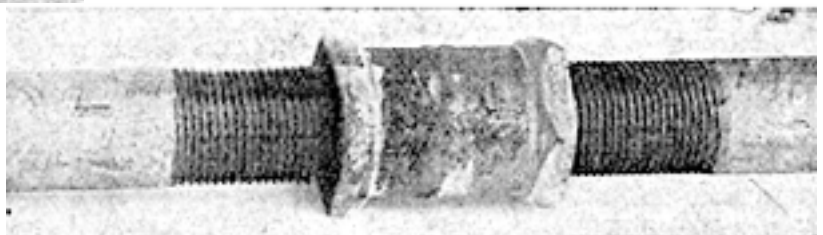
Left. Fig. 5. The pipe joint shown painted and being screwed up with the wrench.
