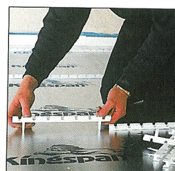
1 Press the pipe clips into place
