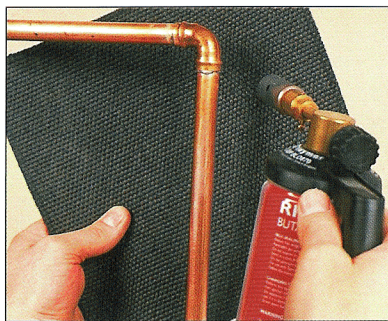
Heat the joint to melt the captive solder
