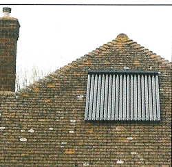
Mount collectors on a south-facing roof
