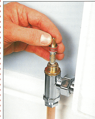
O-rings are housed in grooves in the valve spindle
