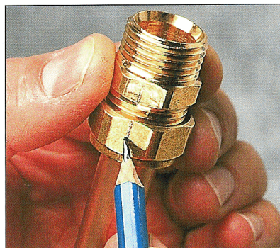
3 Mark the nut and joint with a pencil
