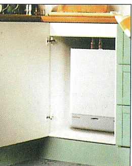
Locating gas boilers Modern boilers fit snugly into standard kitchen cupboards.
