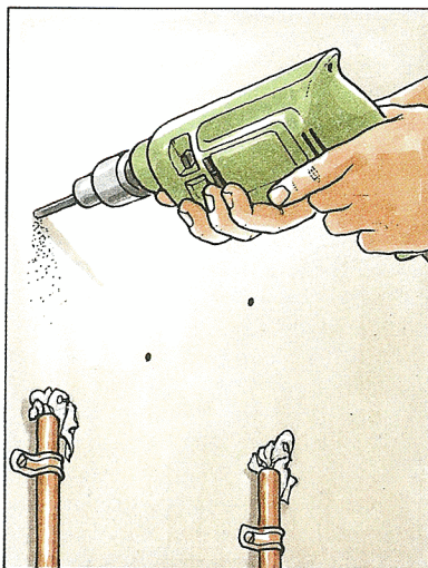
4 Drill and plug the holes
