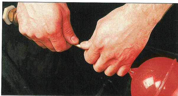
1 Straighten or bend a metal float arm
