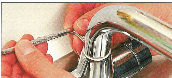
3 Remove the screw to release the mixer spout. You can use a cranked screwdriver (below) if the retaining screw is located behind the swivel spout.
