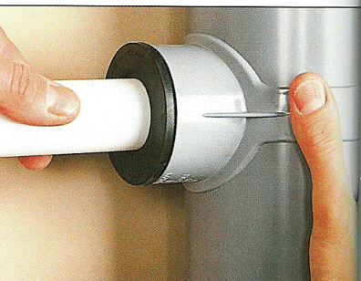
4 Push the waste pipe into the boss
