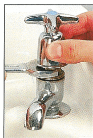
1 Loosen headgear nut
