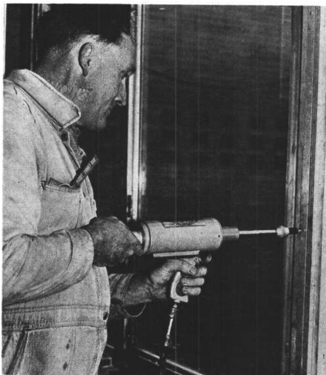
2 Fastening aluminium cover strips to prefabricated window frames with 'Chobert' rivets
