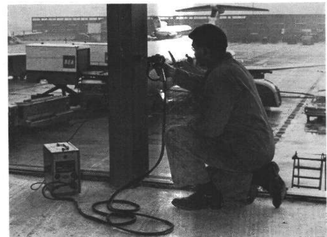
6 Threaded studs are fastened to window stanchions by capacitor discharge equipment
