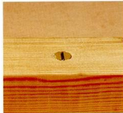
ABOVE: If all is well, the top face of the screw will be a clean fit, but fractionally lower than the surface of the wood.
