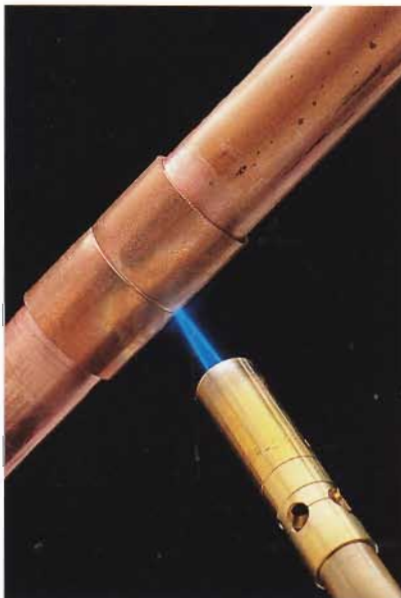
D. Heat the fitting until the flux begins to sizzle. Concentrate the tip of the torch's flame on the middle of the fitting.
