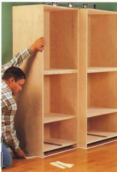
J. Shim under the side panels of the end units if necessary to align the top of each end unit with the center unit.
