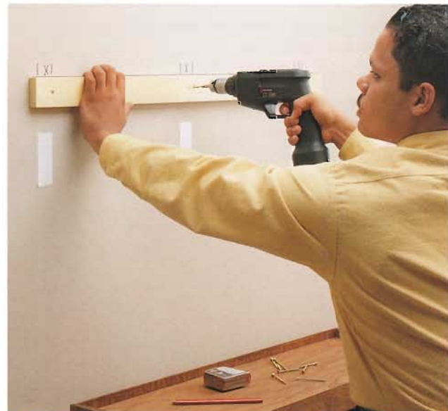
F. Install a temporary ledger strip so the top edge is flush with the reference line.
