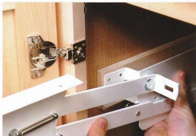
A. Mount wood spacers, then position each swing arm to make sure it will clear the door hinge and face frame.
