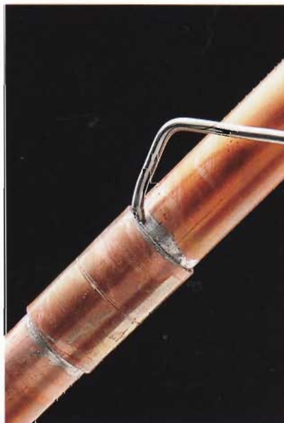
E. Push ½" to ¾" of solder into each joint, allowing capillary action to draw the liquefied solder into the joint.
