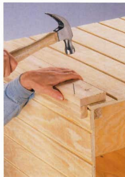
C. Attach the corner trim pieces flush with the edges of the corner battens, covering the plywood joints.
