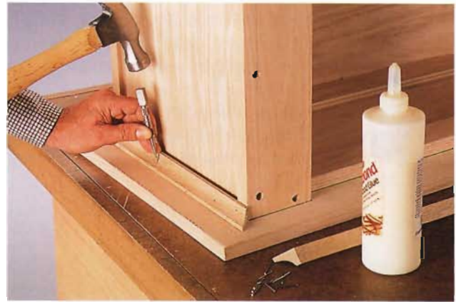
E. Miter-cut cove molding to cover the joint between the top panel and the carcass.
