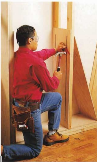
D. Install the lower risers on each side of the 2 × 4 support studs with 1½" finish nails.
