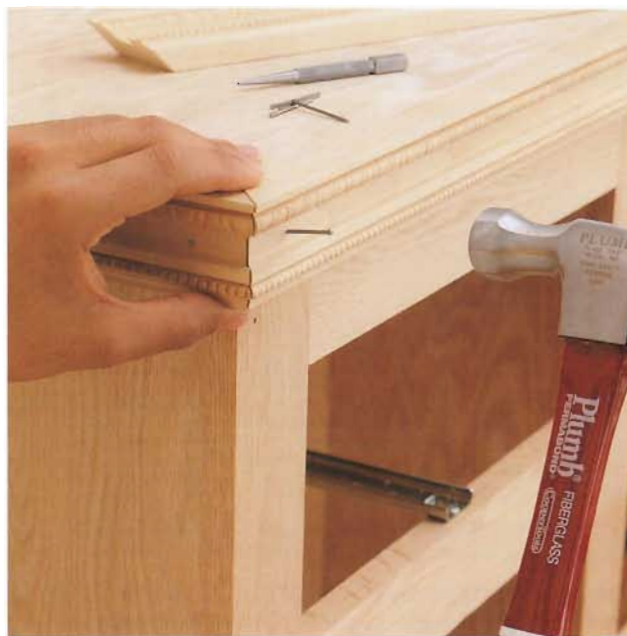
E. Cover the exposed edges of countertop with mitered ornamental molding.
