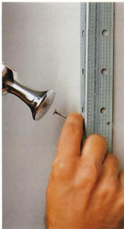
M. Install the corner bead with nails or screws driven every 8".
