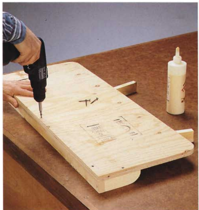
D. Attach the 1 x 2 skirt that frames the top of the top shelf, screwing the pieces together from below.
