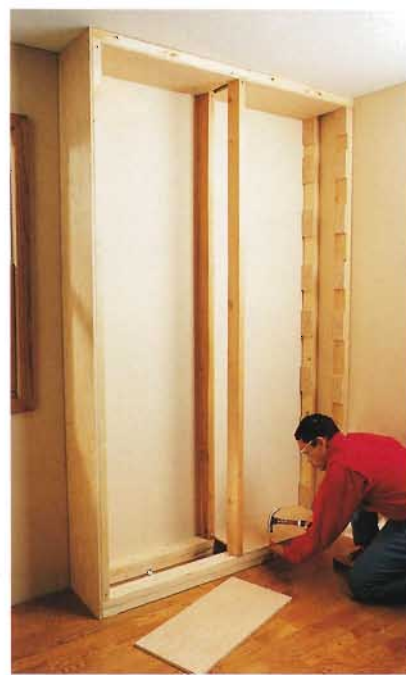
C. Attach the plywood top and bottom panels to the top and sole plates using 1½" finish nails.
