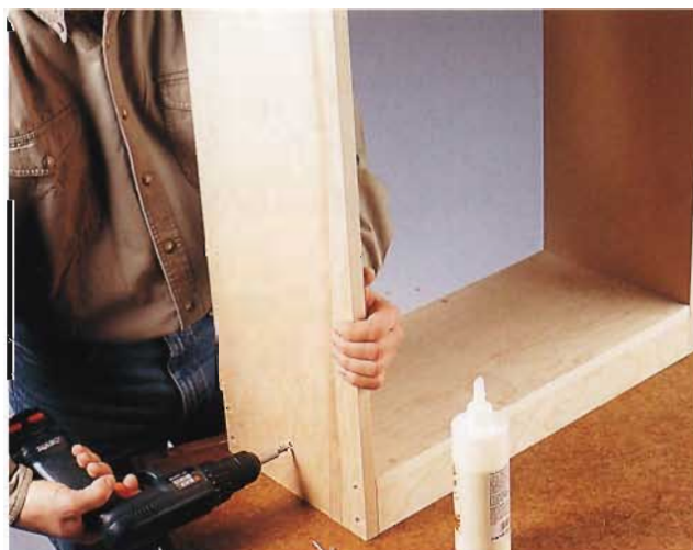
A. Attach the cupboard bottom by driving screws through the cupboard sides and into the edges.
