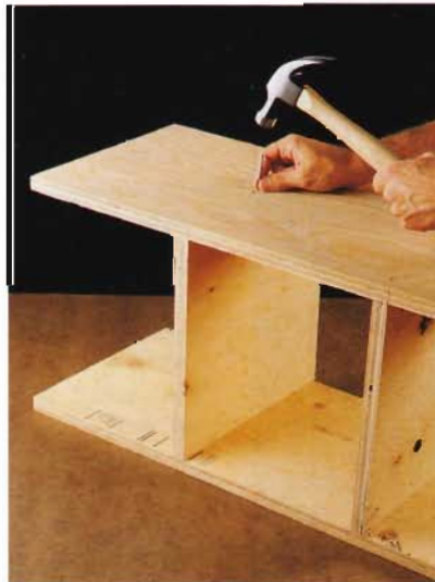
B. Assemble the central shelving unit, leaving the top open.
