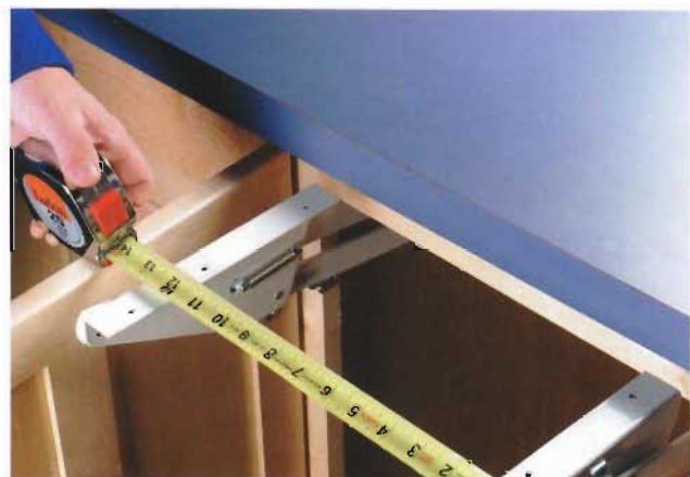
C. Determine the width of the shelf by measuring between the outer edges of the swing arm mounting flanges.
