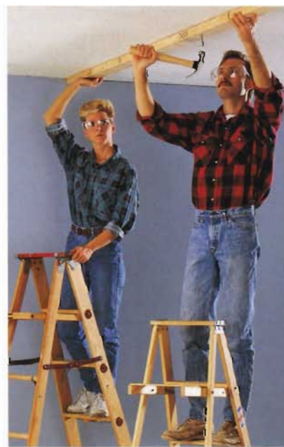
C. Install the top plates with 16d nails driven into the ceiling joists.
