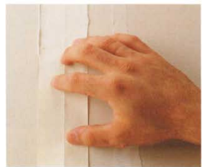
L. Press the wallboard tape into the compound and smooth out the tape with a 6" wallboard knife.
