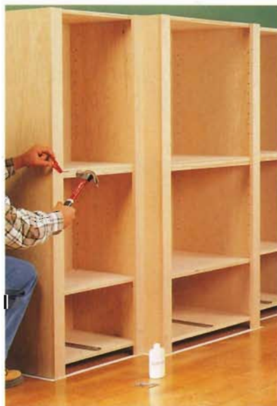
K. Measure and cut 1 × 3 vertical face frame stiles and attach them.
