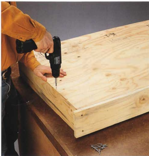
D. Cut the bottom panel to size, then fasten it to the box frame and divider.
