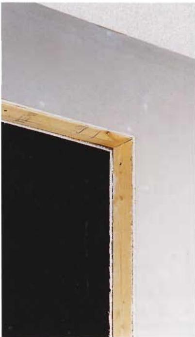
J. Plan the wallboard placement so that there are no joints at the corners of the door opening.
