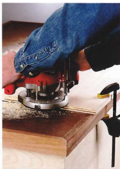
A. Use a router with a straightedge guide to cut the dado and rabbet grooves shown in the diagram on page 233.
