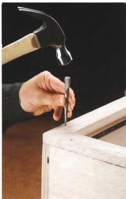
D. Install trim along the front edges of the cabinet, shelves, and side support, then use a nail punch to set the nails.
