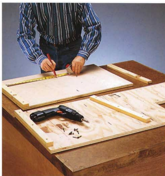
B. Measure up from the bottom cabinet cleats to mark positions for the other cabinet shelf cleats.
