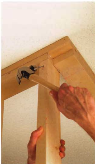
G. Toenail the corner stud assembly in place with 10d nails. Follow the Corner Detail drawing on page 257 for the exact placement of the studs.
