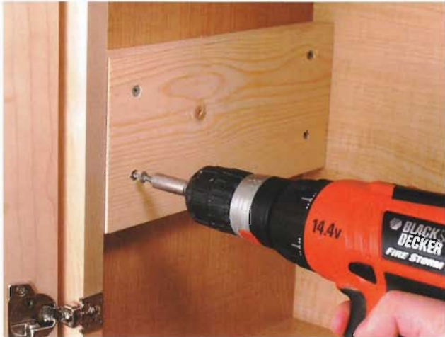
A. Fasten the spacers to the sides of the cabinet, using drywall screws.
