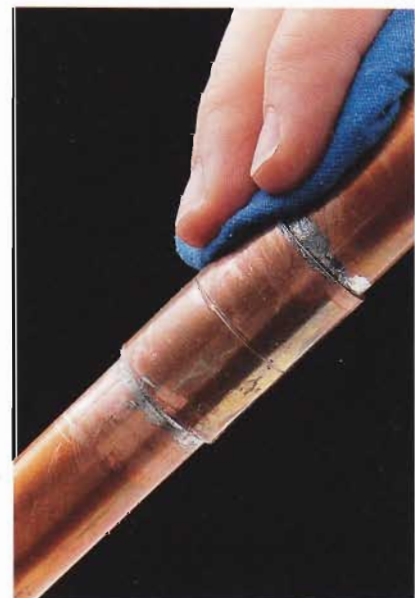
F. When the joint has cooled, wipe away excess solder with a dry rag. Be careful: Pipes will be hot.
