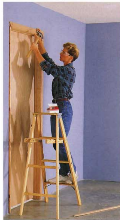
O. Install the door casings using 8d finish nails driven through pilot holes into the wall framing.
