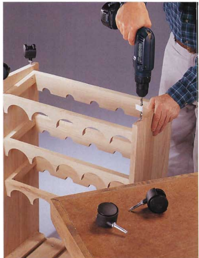
G. Drill holes for the casters in the bottom edges of the sides. Consider using a right-angle drill guide to ensure the holes are perpendicular to the sides.
