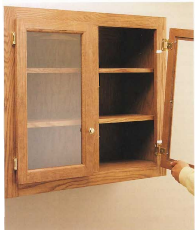
I. Install overlay doors and door hardware after the finish for the cabinet and doors is dry.
