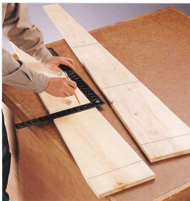
B. Use a framing square to mark reference lines for shelf placement on the standards.
