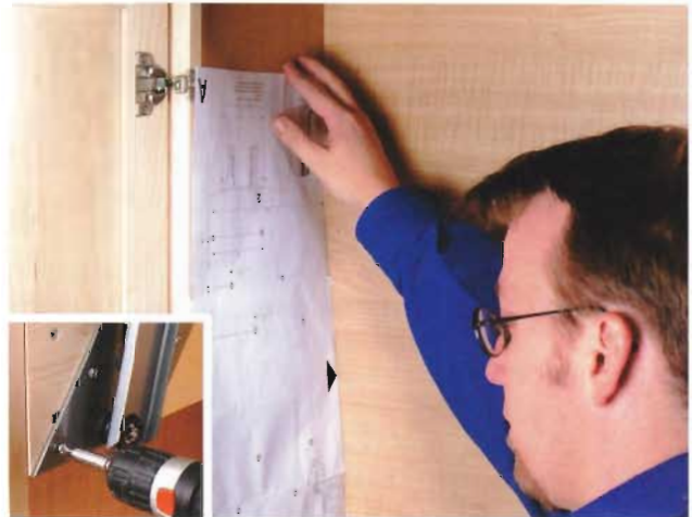
B. Use the manufacturer's template to mark the locations of the swing-arm mounting plates.
