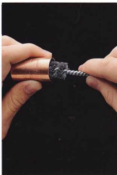
B. Clean the inside of the fittings with a wire brush.
