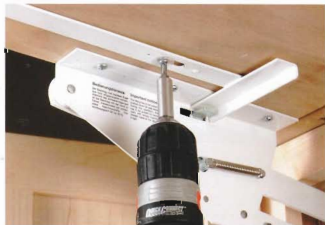
D. Fasten the locking bars to the bottom of the shelf, using the provided screws and spacers.
