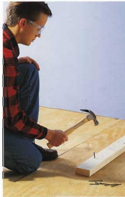
E. Install the sole plates with 10d nails driven every 16".
