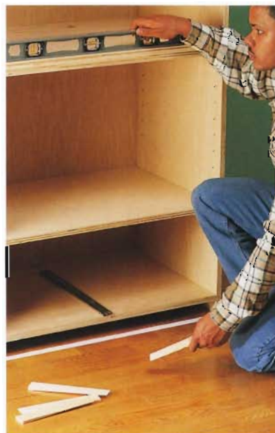
H. Shim under the sides of the center unit, if necessary, until it is level and plumb.
