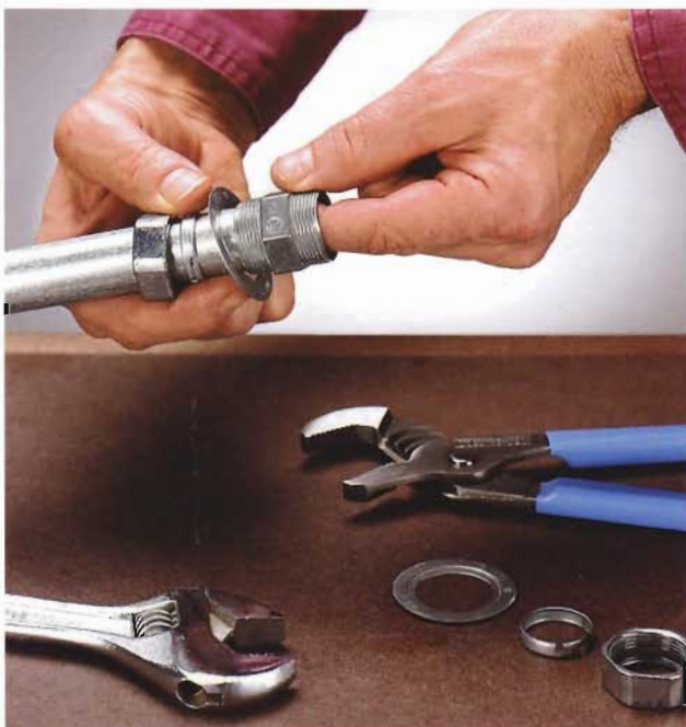
B. Insert the sanded pipe into the compression coupling, and tighten the fitting, using a channel-type pliers and an adjustable wrench.
