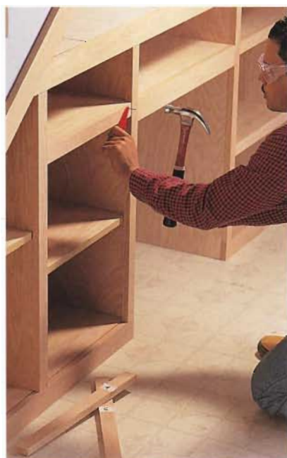
K. Measure and cut the stiles to size. Attach them with 2" finish nails, making sure the ends are flush with the bottom and countertop rails.
