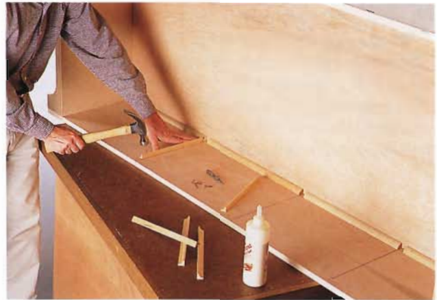
E. Attach the shelf cleats with glue and brads.
