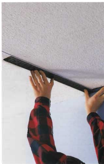
B. Check the chalk line with a framing square to ensure the layout is correctly placed.
