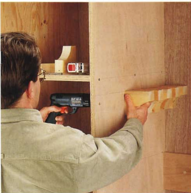
D. Attach the hangers by driving screws through the divider and into the ends of the hangers.
