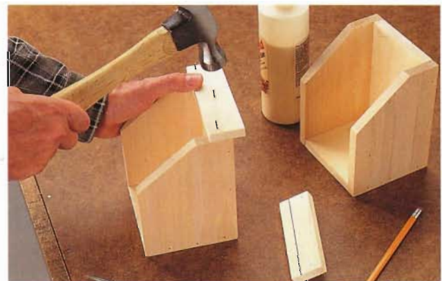
F. Attach the drawer fronts to the front edges of the sides and bottoms so they overhang the bottoms by \frac{1}{2} ".
