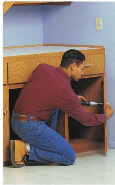
L. Hang the doors with \frac{3}{8} " semi-concealed hinges. See page 40 for more information.
