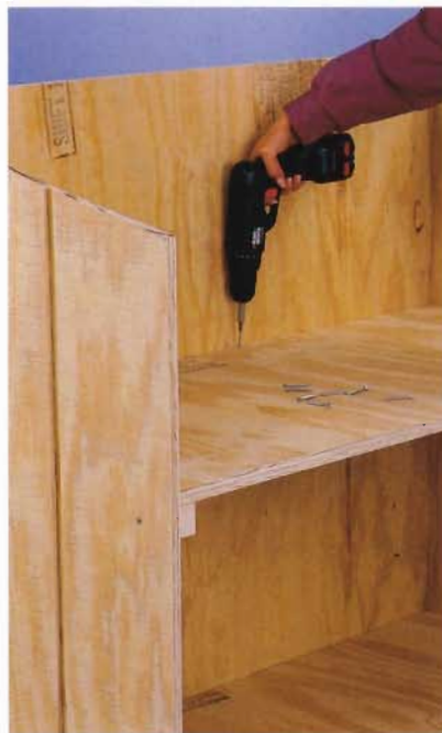
D. Place the shelf on top of the cleats and fasten with glue and screws.
