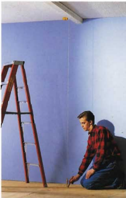
D. Take multiple plumb bob readings to determine the locations of the sole plates.
