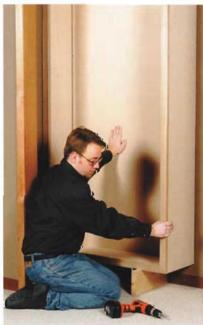
E. Mount the cabinet to the closet wall so its bottom edge is 6" above the floor.
