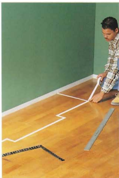
A. Use masking tape to mark the planned location of the entertainment center.
