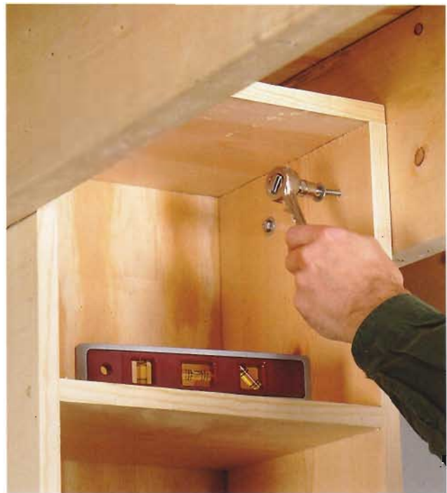
To build a deeper, stationary shelf, build the unit with wider lumber, and drive two \frac{1}{2} \times 2 " lag bolts through each side of the shelf and into the adjoining joists.
