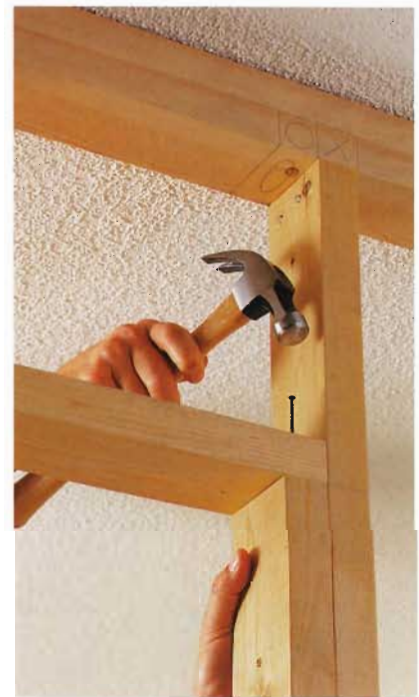
I. Drive 10d nails through the top of the header into the ends of the jack studs.
