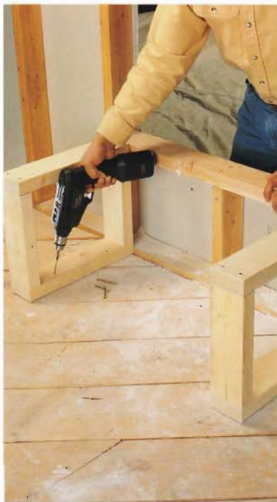
B. Set the pedestals inside the wall opening, even with the sides of the framed opening. Make sure they are level, and attach them to the floor.
