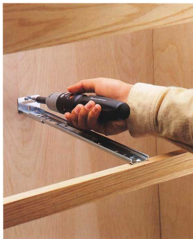
A. Mount the track for the drawer slide with the rear bracket when installing a drawer in an open cabinet.
