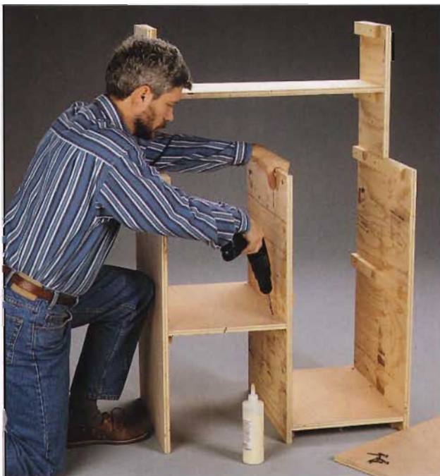
C. Attach the cabinet shelves and upper shelves to the sides and the divider to stabilize and strengthen the garden center.
