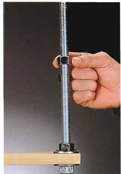
C. Thread nuts and washers onto the rod to position the shelves as desired.
