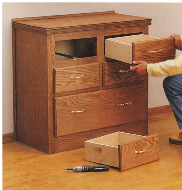
F. Finish the cabinet to match the wall cabinet. Install the drawer hardware after the finish has dried sufficiently.
