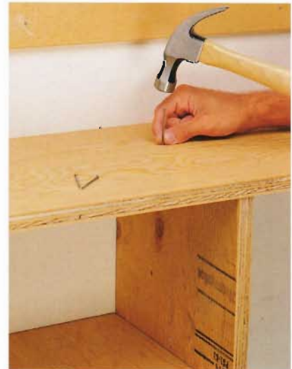
C. Install the upper shelves with 6d finish nails.
