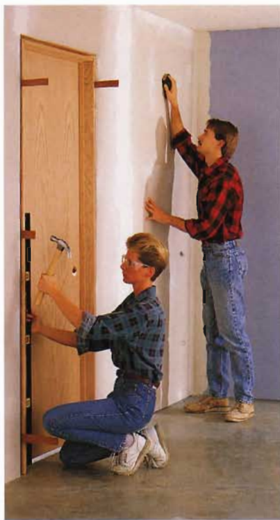
N. Drive shims between the jamb and the jack stud, spaced every 12".
