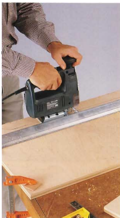
A. Use a jig saw and a straightedge as a guide to make the kick space cuts in the end and side panels.
