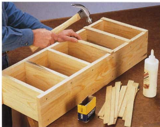
G. Using glue and 4d finish nails, attach the swing-out shelf sides.
