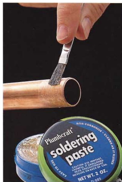
C. Brush a thin layer of flux onto the end of each pipe. Assemble the joint, twisting the fitting to spread the flux.
