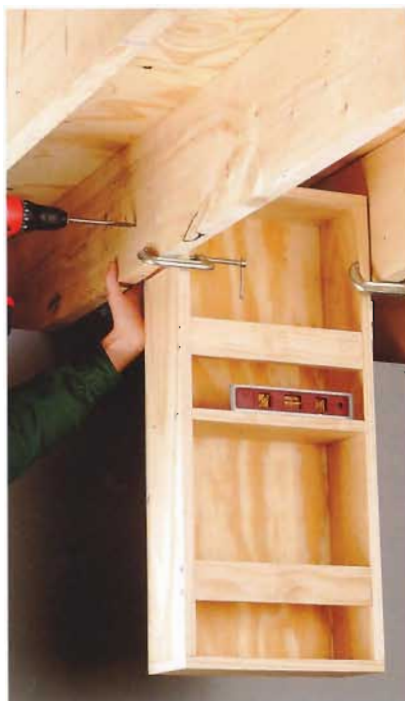
B. Clamp the shelf in place between the joists and drill holes for the carriage bolts.
