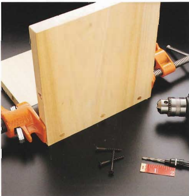
A. Clamp shelf A to shelf B and drill three equally spaced counterbored pilot holes through shelf A and into shelf B.
