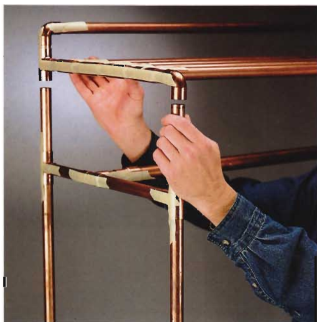
A. Test-fit each length together, making sure the pieces are cut to the proper length. Use masking tape to hold the joints in place.
