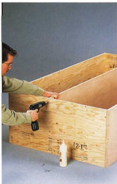
A. Install the divider panel between the top and bottom panels, separating the locker into an open area and a shelf area.
