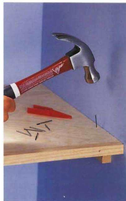
C. Attach the shelves to the cleats with 1 \frac{1}{2} " finish nails driven through pilot holes.
