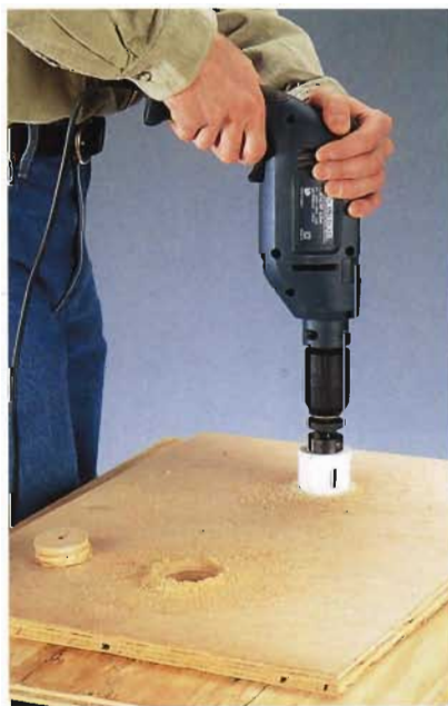
B. Using a hole saw, cut 2"-dia. holes in the shelves to keep balls from rolling inside the locker.
