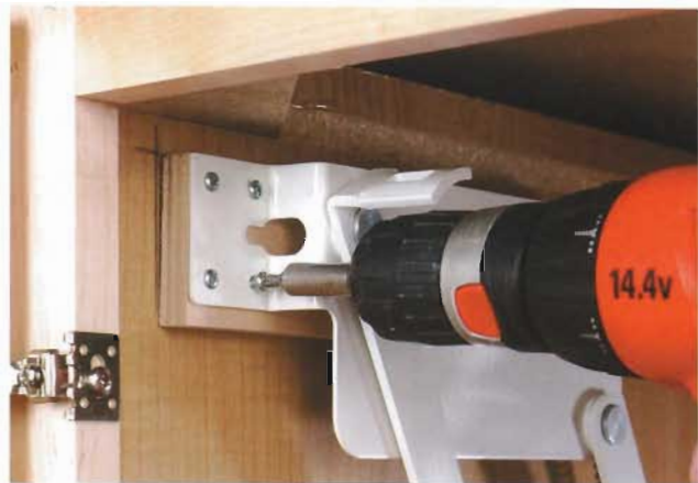
B. Mark the screw locations for the mounting plates on the spacers, then attach the swing arms
