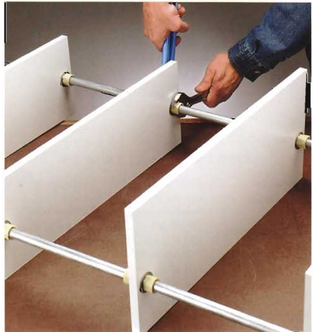
D. Use channel-type pliers and an adjustable wrench on both coupling nuts simultaneously to avoid loosening the opposite nut.
