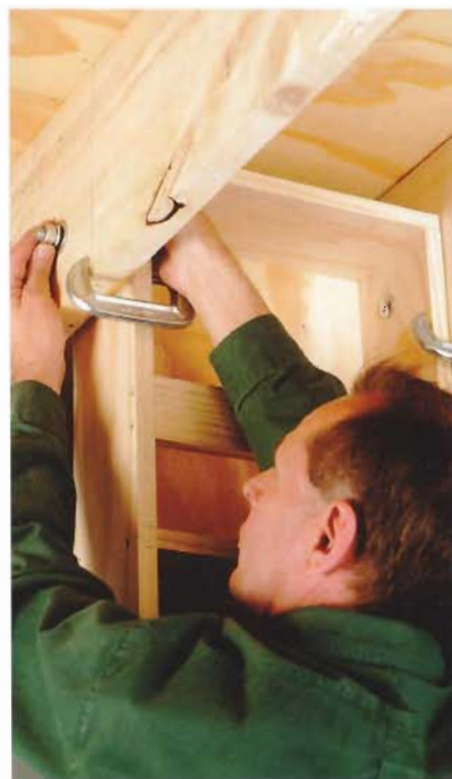
C. Insert a carriage bolt through the outer edge of a joist, then add a washer, lock washer, and hex nut.
