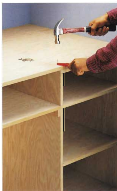
H. Install the countertop panel with 1½" finish nails driven through the countertop, into the cabinet sides.
