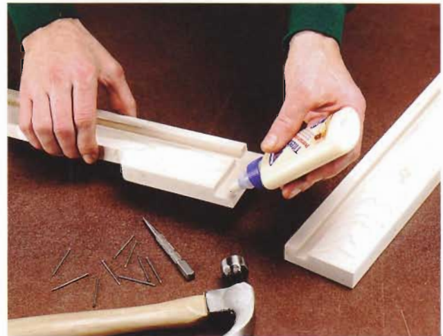
B. Use glue and finish nails to assemble the shelves. Clamp until the glue dries.
