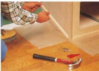
M. Install mitered ornamental molding along the top edge and base-shoe molding along the bottom edge of all the cabinets.
