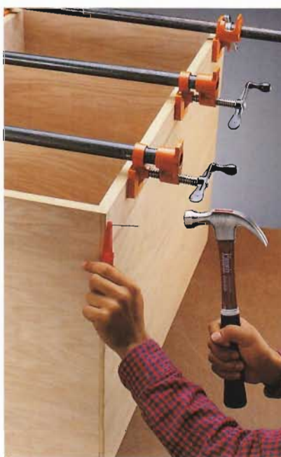
E. Reinforce each joint with 2" finish nails.
