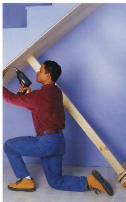
B. Use a 2 x 4 and some scrap wood to hold the understairs cover in place while you install it.
