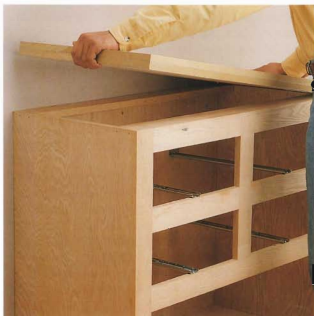
D. Set the two countertop panels on the cabinet, and anchor them with 2" screws driven up through the supports inside the cabinet.
