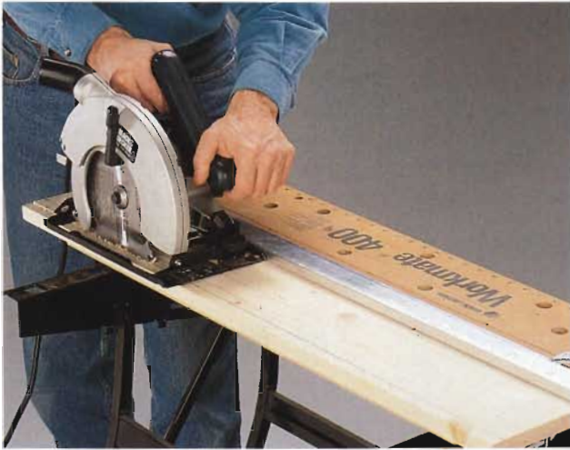
H. Use a circular saw with a straightedge as a guide to rip-cut the door boards to size.
