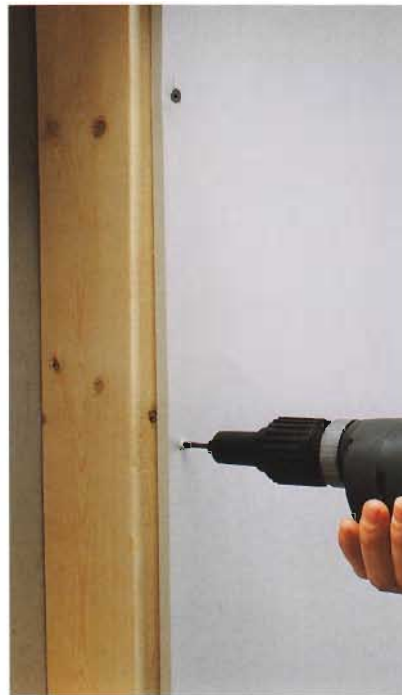
K. Install the panels using a screwgun and 1½" wallboard screws, spacing the screws every 10".
