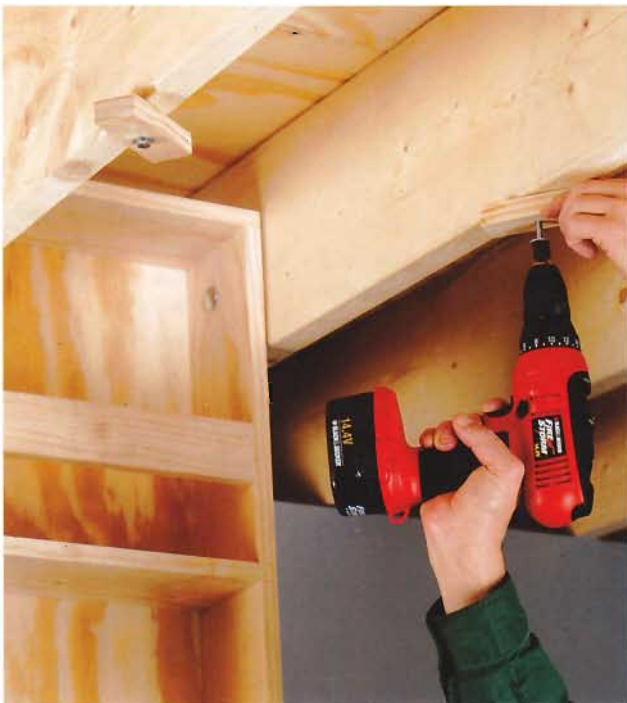
D. Screw plywood cleats into position to act as latches for the shelf.
