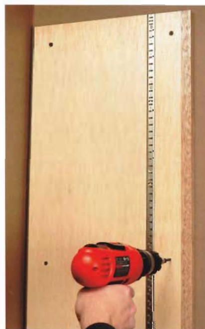
F. Install the side support at the cabinet height, then cut the closet rods to fit.
