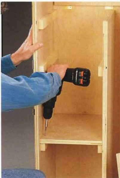
D. Attach the shelves by driving screws through the shelves into the cleats.
