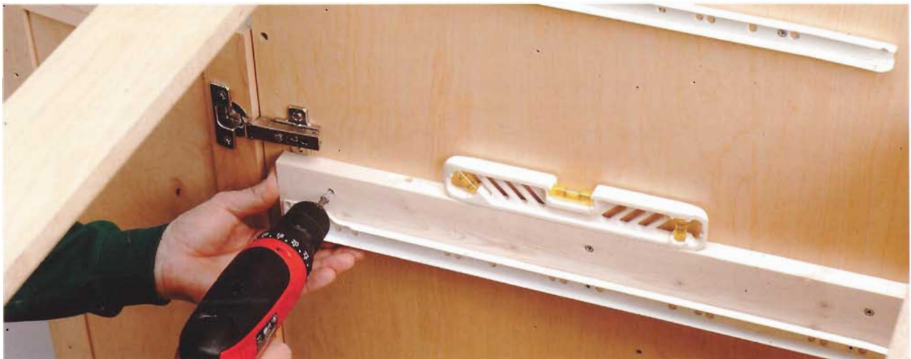
C. Mount glide-out rails to the bottom of the spacer strips, then attach the spacer strips to the interior walls. Attach the sliding rails to the bottom of the shelves, then install the shelves.
