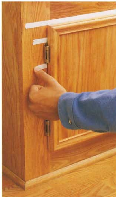
B. Position the door flush with the bottom edge of the reference line and mark the location of the top hinge with masking tape.
