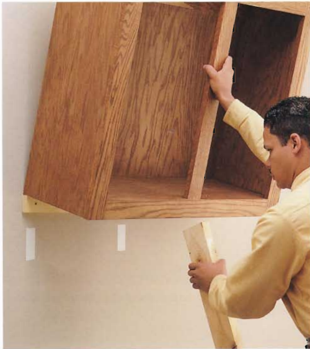
G. Set the cabinet on the temporary ledger and brace it in position with a 54"-long 2 x 4.
