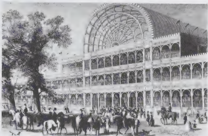
The Crystal Palace, 1851. The huge but graceful building was constructed from prefabricated iron and glass panels. It symbolized science, technology, and progress to the Victorians.
