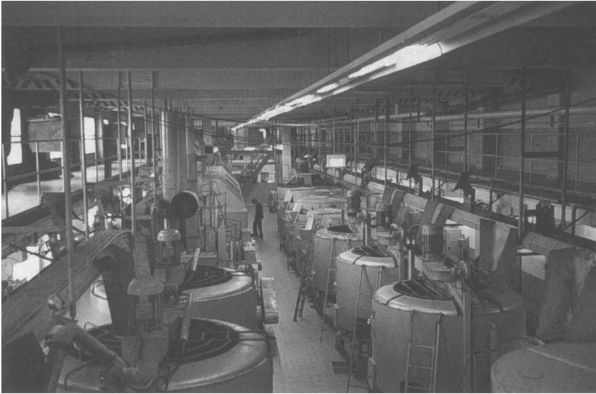
Figure 4.14 Picture of rotary conches
