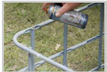
ABOVE:- Easier and a little more expensive alternative is to use pressure can paints. Easy and clean to use to freshen up the steel work..
