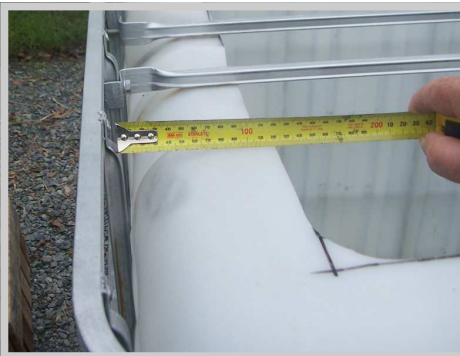
ABOVE:- Mark a line on all four sides. To guide your cut. This photo was taken after the plastic tank was put back in the cage and the top braces re fitted.
