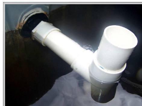
Above:- View showing how the made up assembly fits into the outlet fittings.
