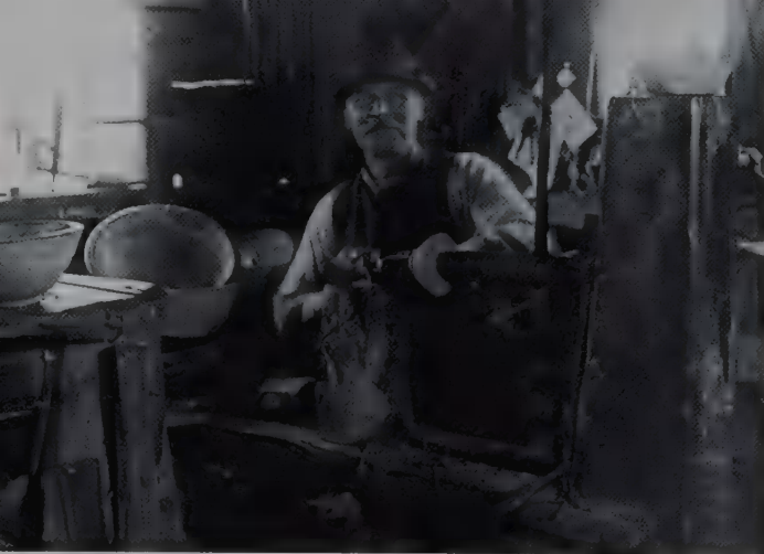
18. George Lailey, bowl-turner of Bucklebury, in the sunken hut with his pole lathe: an Iron Age tool still in use after the First World War.
