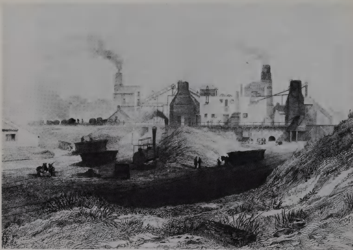
OLD HETTON COLLIERY, near Sunderland, by Thomas Hair c.1840. This big pit is fairly typical of the deep mines sunk in the northern coalfield to cope with escalating demand in the early years of the nineteenth century. The standard (4 feet 8½ inches) gauge railway connecting it with the sea was laid out by George Stephenson and two of his locomotives can be seen in the foreground.
