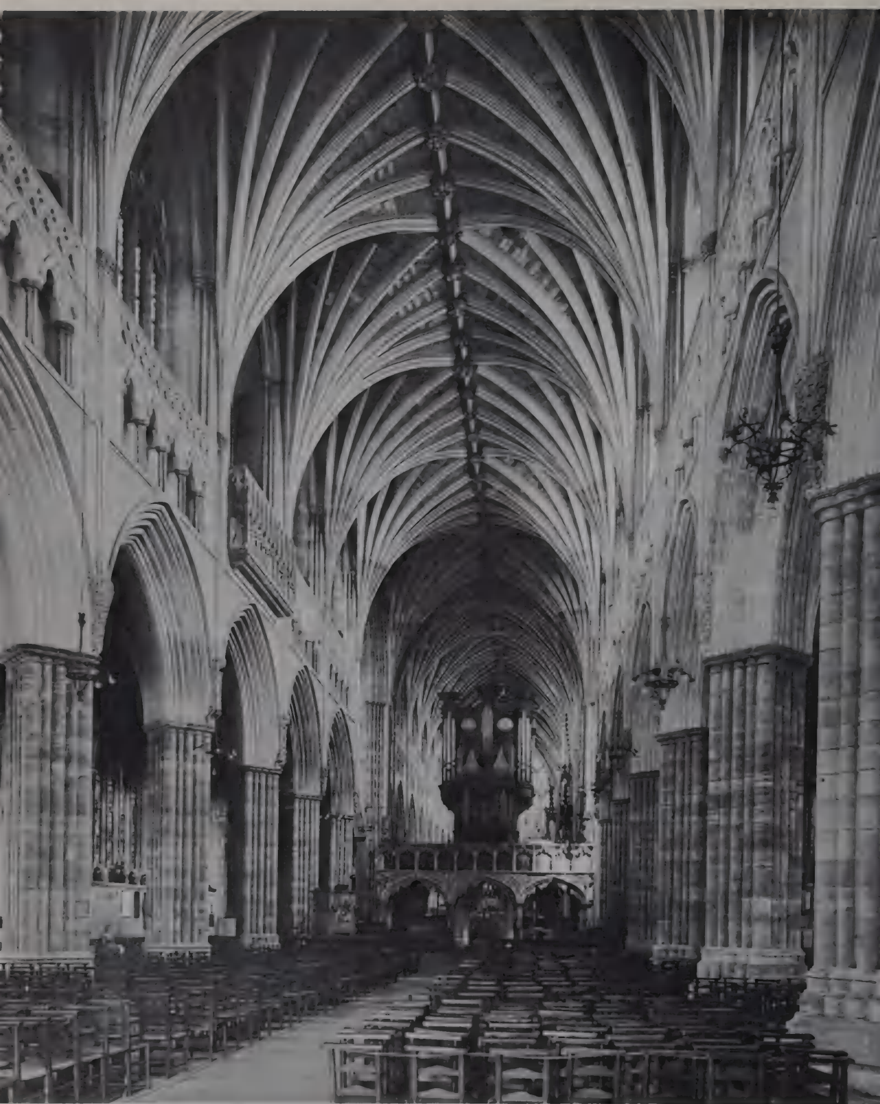
EXETER CATHEDRAL, early fourteenth century. The nave, looking east, is the longest unbroken vista of Gothic vaulting in the world (over 300 ft.). The solid pillars and exuberant vaulting create a symmetrical avenue of what appear as towering palm trees. Completed by 1360, mainly by Bishop Grandisson, and financed by the wealth of the English Church before the Black Death.
