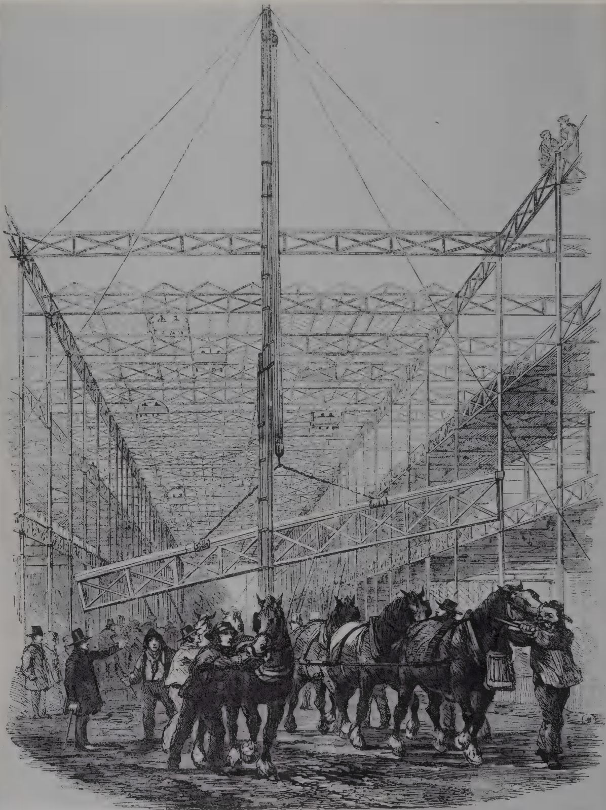
CRYSTAL PALACE, 1850. Using a horse-operated crane to raise the wrought-iron cross beams of the central avenue of the Crystal Palace. Joseph Paxton's design was a pioneer work of prefabrication; workers are already glazing the roof from trolleys. Site work started in August 1850, and was completed by May 1851.
