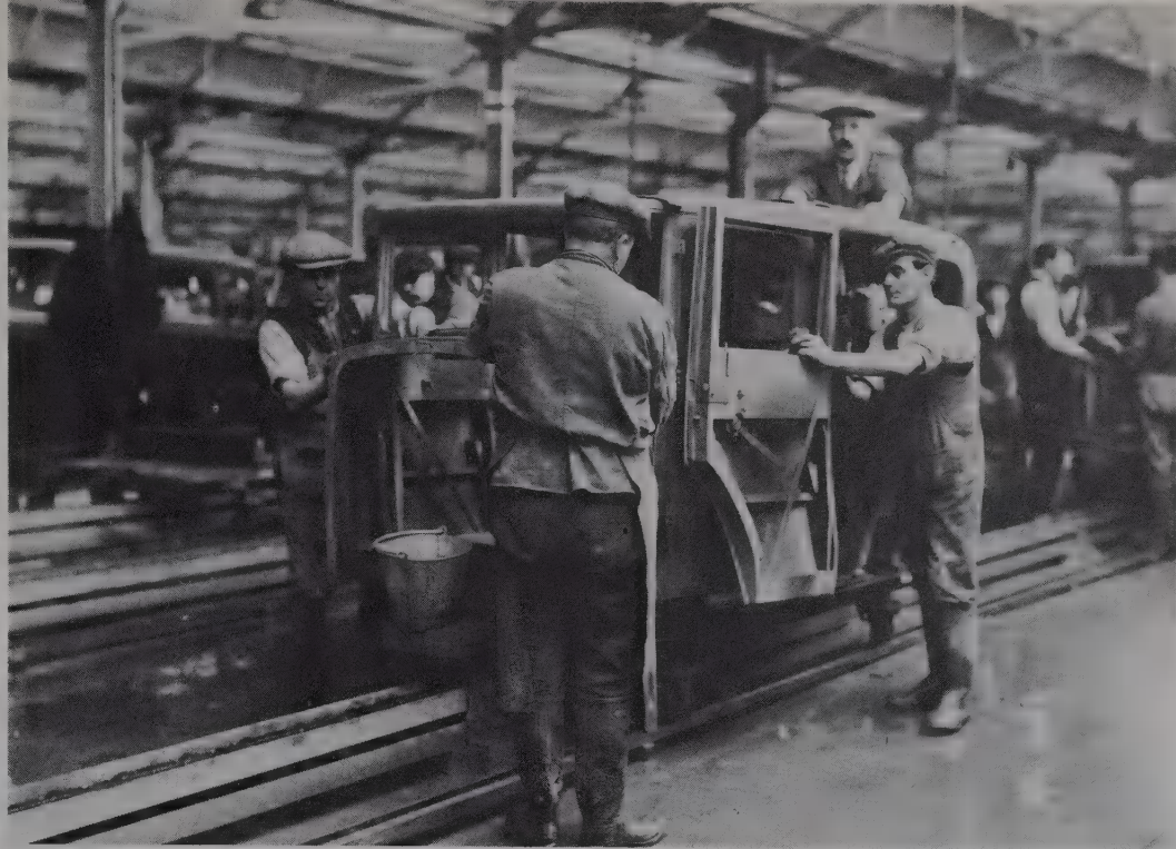
MASS PRODUCTION AT MORRIS MOTORS, COWLEY, OXFORD, 1929. Here the body foundation is being rubbed down after the first coat of paint. The car industry, pioneered by William Morris at Cowley and Herbert Austin at Longbridge, made a dramatic impact on British economic life and leisure patterns in the twenties.
