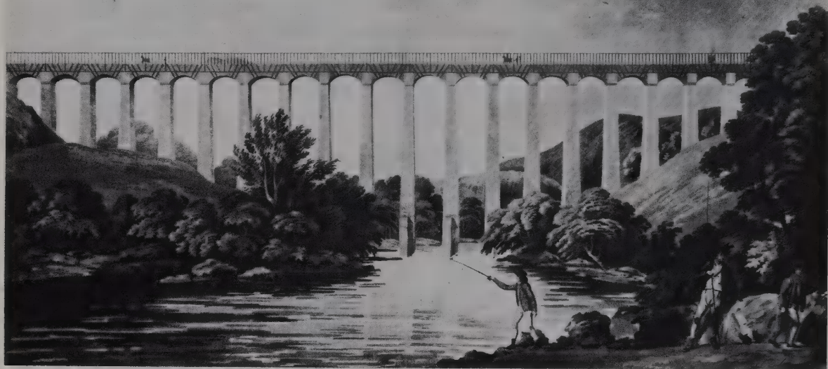
THOMAS TELFORD'S 'STREAM IN THE SKY'—the Pont-cysyllte aqueduct—carried the Llangollen canal 124 feet over the Dee in a cast-iron trough only 10 feet wide. It was probably the most spectacular piece of engineering of the early industrial revolution.
