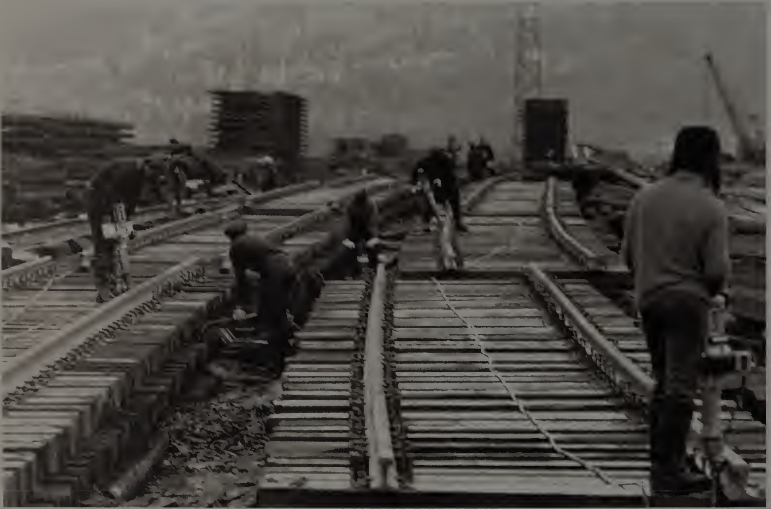
Baikalo-Amurskaya Railroad Workers, 1974— The railroad from Lake Baikal to the Amur region ran through rugged terrain in the far eastern part of the country. Note the use of a double layer of tracks, necessitated by the region's permafrost.
