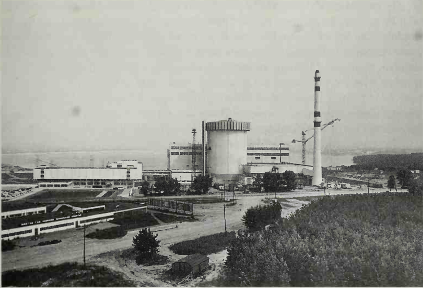
The fifth unit of the Novovoronezh Nuclear Power Station, a 1,000-megawatt pressurized-water reactor, completed in 1980. (Courtesy of Raissa Kuznetsova and the Kurchatov Institute)
