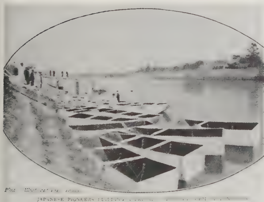
24 The Japanese indulged in novel logistic plans. These coolie-portable galvanised metal boxes when made into pontoons were built into bridges such as this one (25)
