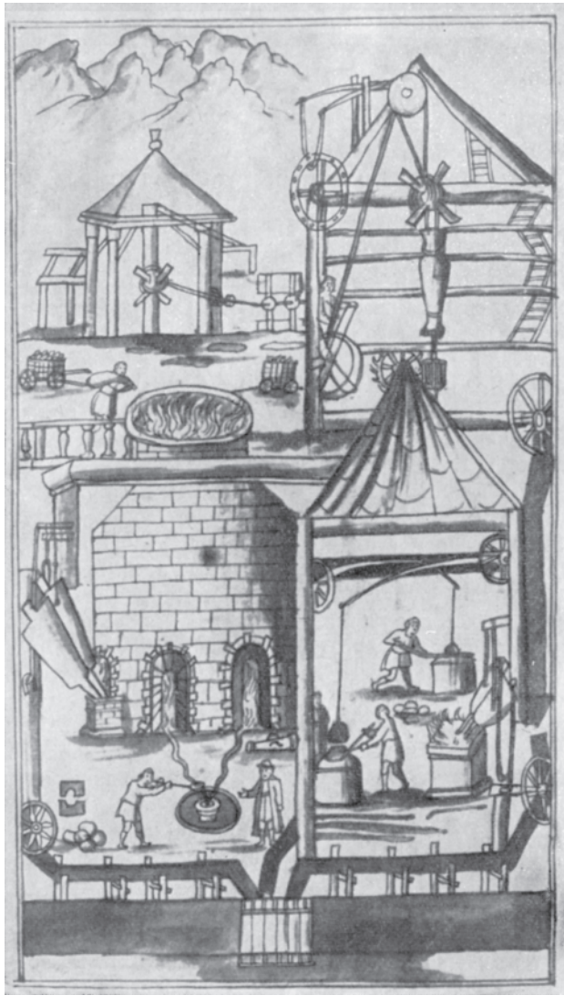
Figure 2 Drawing of a late seventeenth-/early eighteenth-century Siberian iron foundry with blast furnace. Note (a) the mountains in the background (almost certainly the Urals); (b) the large bellows on the left, serving the blast furnace; (c) the ingenious Heath Robinson apparatus of cogs, wheels and pulleys operating the power-hammers.
