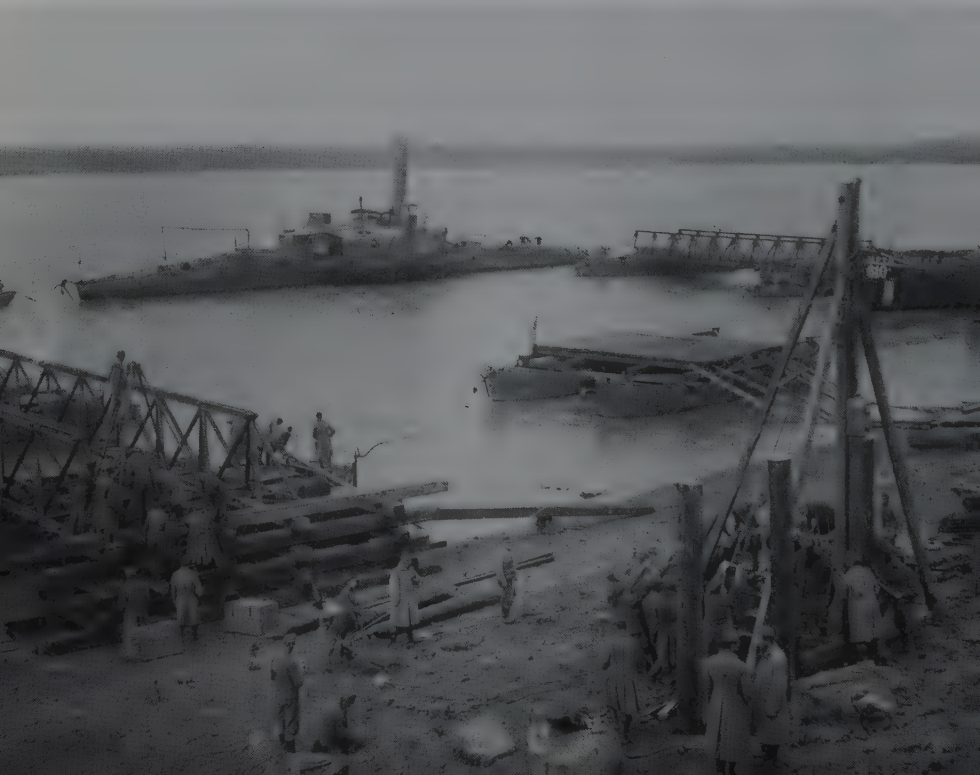
Building of the treadway bridge, November 1916 which enabled the crossing of the Danube River by Mackensen's Danube Army, from the Bulgarian bank near Svistov. (Photo by Robert Sennecke/ullstein bild via Getty Images)
