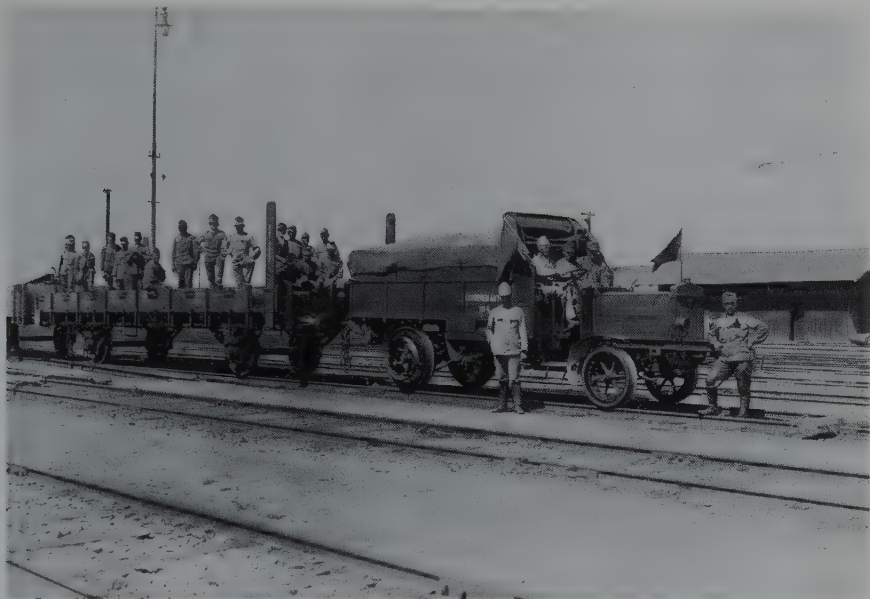
A rail vehicle of the k.u.k. Army on a railway station in Galicia, probably in 1915/16. The vehicle could also be used as truck on a road. (©ullsteinbild/TopFoto)
