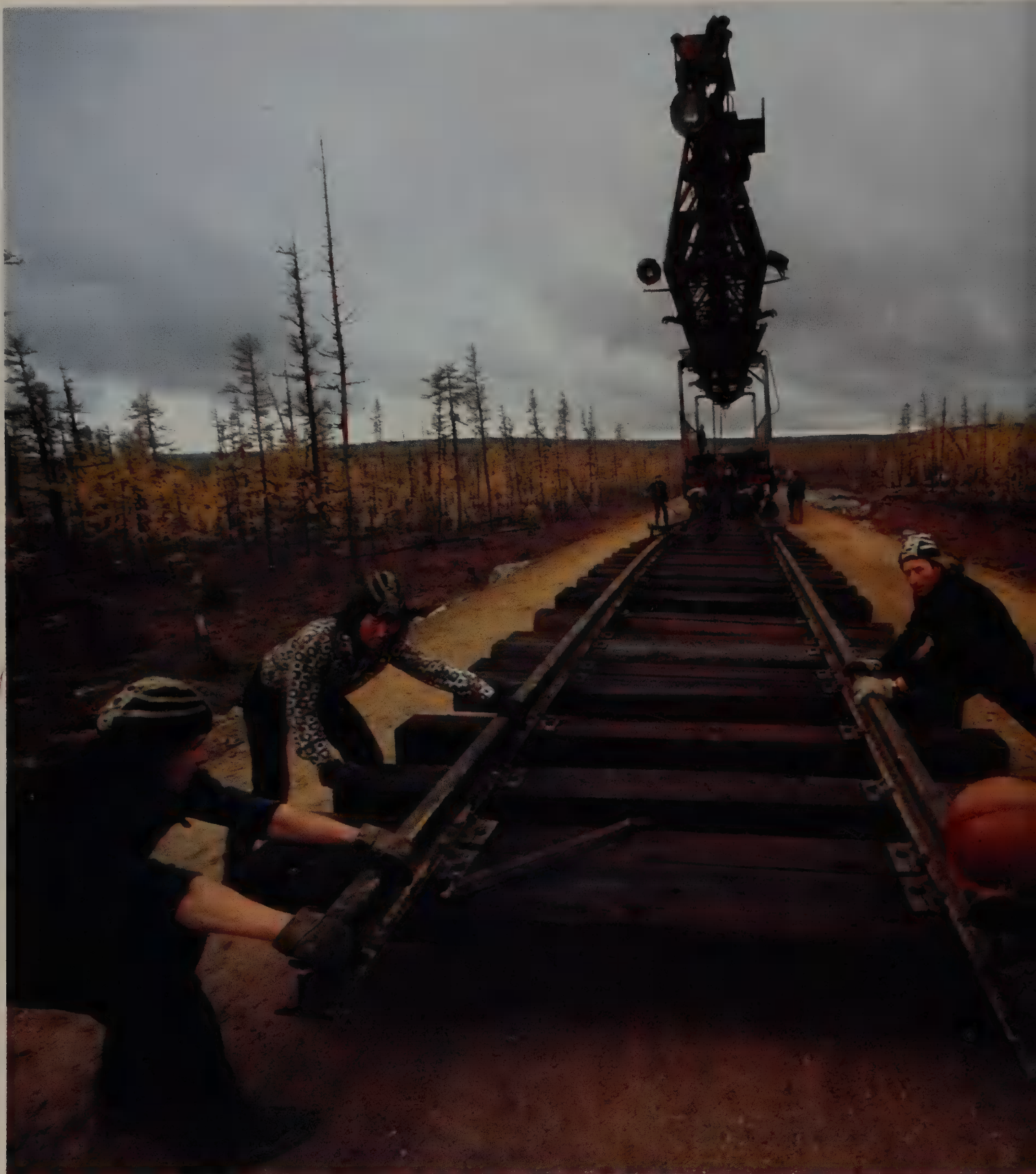
Siberian Yakuts — part of the labor force drawn from the local population — lay a prefabricated section of track with the aid of a crane.
