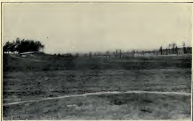
PREPARED RESERVE TRENCH
