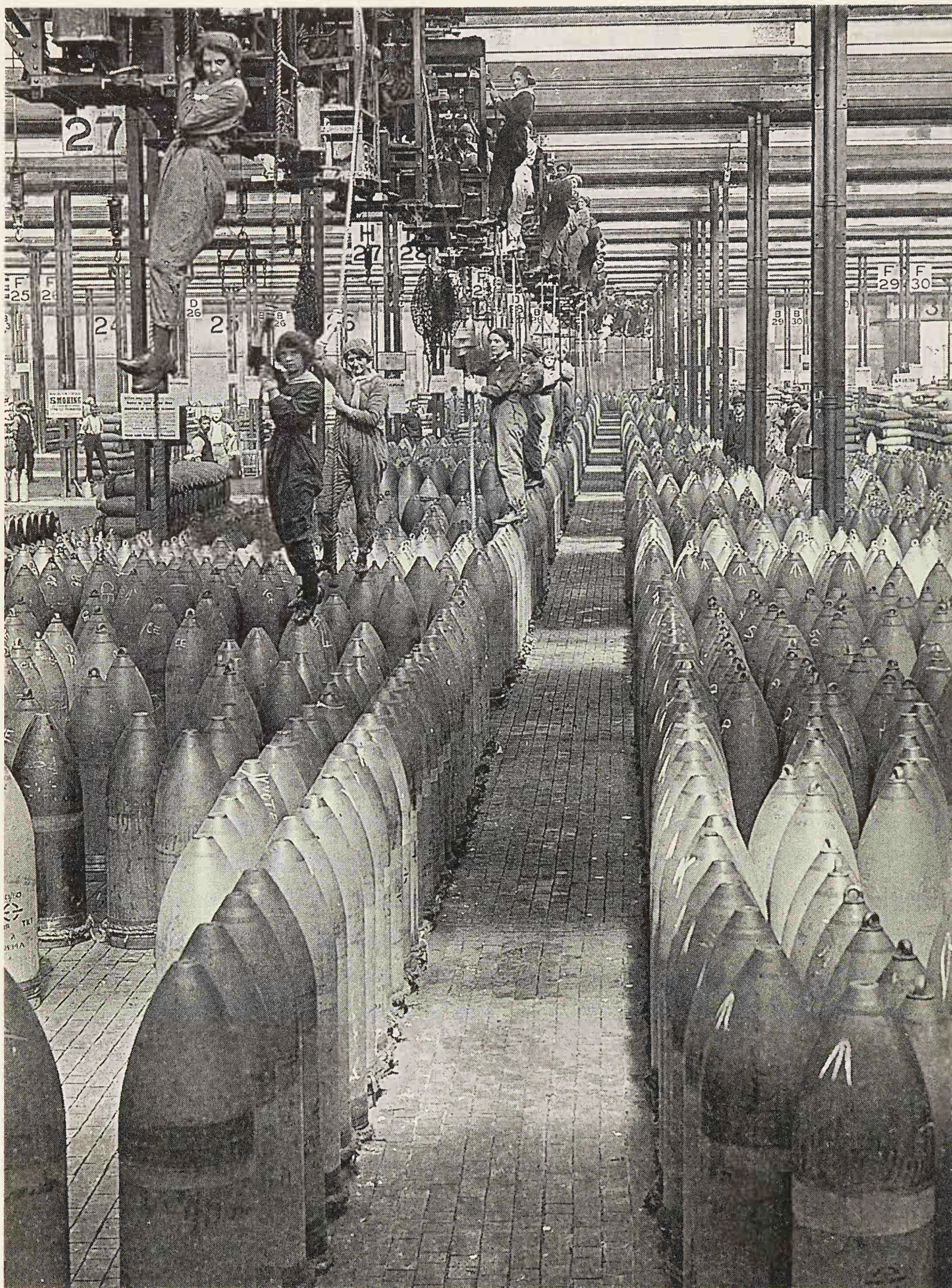
Women munitions workers in the shell-filling factory at Chilwell near Nottingham. The wood-block floor was designed to prevent sparks, but there were several explosions, one of which gutted this building; it was rebuilt immediately.
