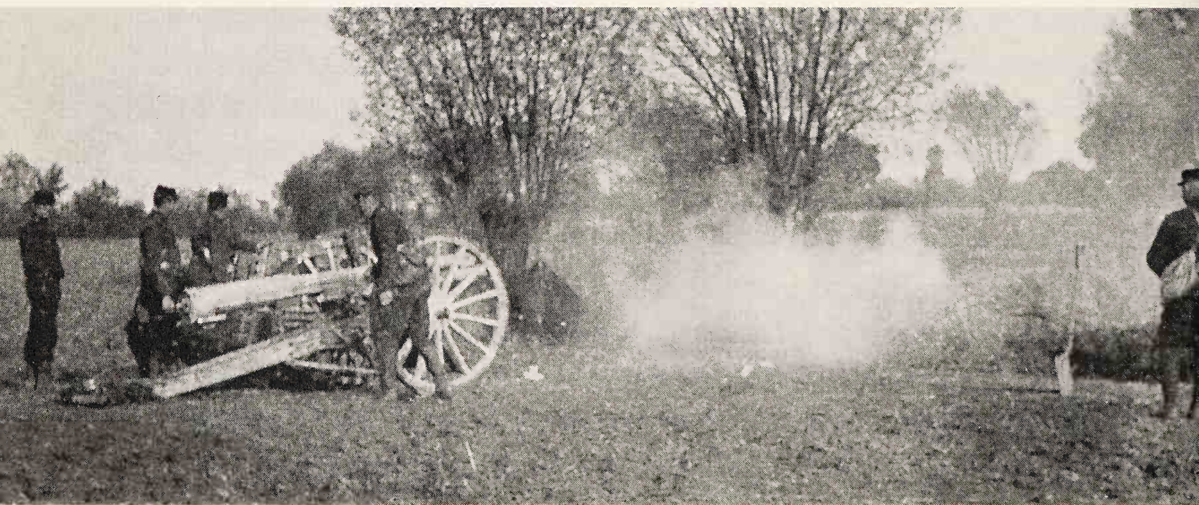
A French 75 mm field gun showing the barrel at full recoil after firing. France was pitifully short of modern heavy guns.
