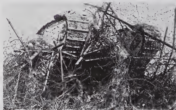
LEFT Tanks were expected to crush wire and, often using ropes and grapnels, to clear avenues for attacking infantry.
