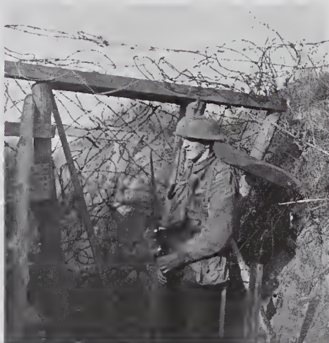
Trenches were equipped with a variety of 'bomb stops' to prevent an enemy who entered the trench grenading his way along it. This barbed wire gate, in the Cambrin sector held by 1/7 Sherwood Foresters in September 1917, could be shut to bar an attacker's progress. The sentry is wearing 1914 pattern leather equipment.
