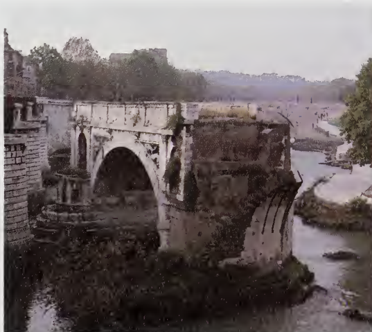
The Ponte Rotto ( Broken Bridge ), Rome—the remains of the Pons Aemilius, showing the construction of arch.
