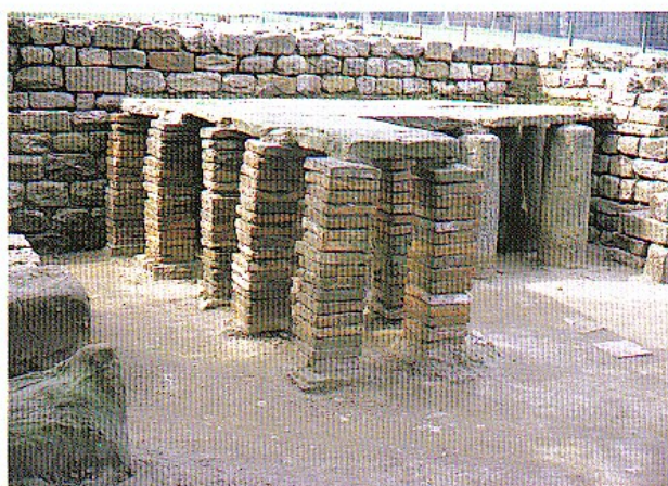
A hypocaust, a heating system under the floor
