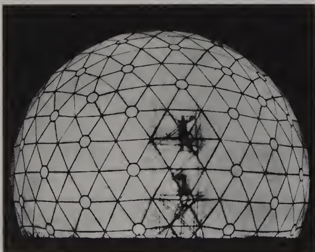
Fig. 9-11. A geodesic dome built on a plan of a T = 12 icosahedral surface lattice.
