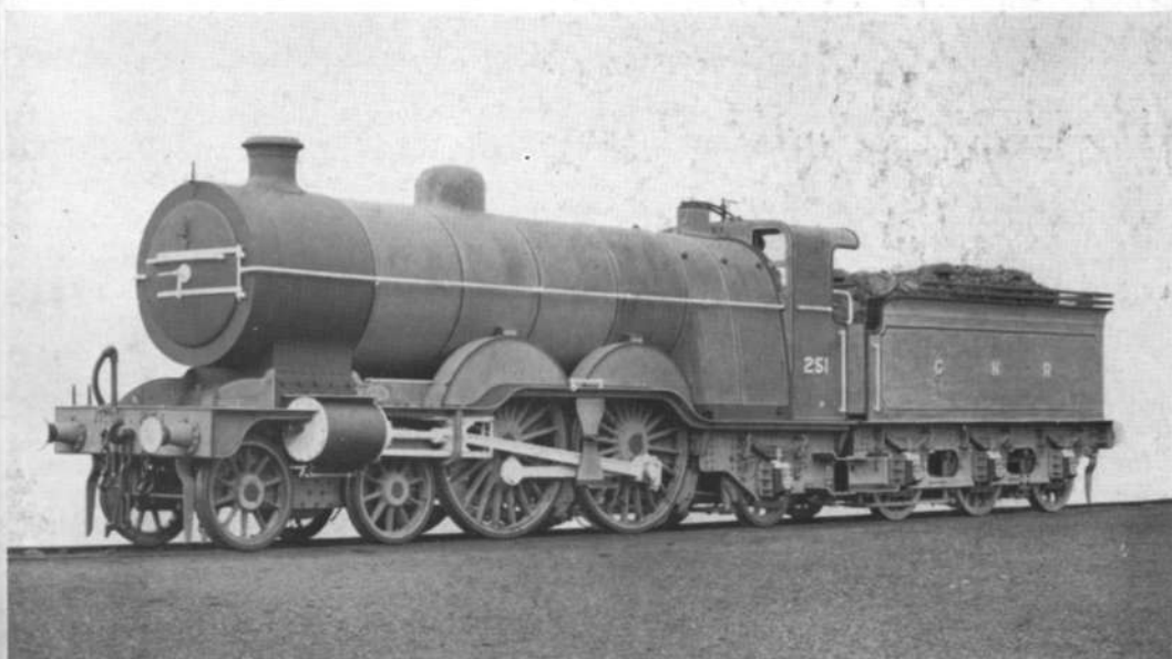
No. 251, the first Atlantic with large boiler and wide firebox, built at Doncaster in 1902.
