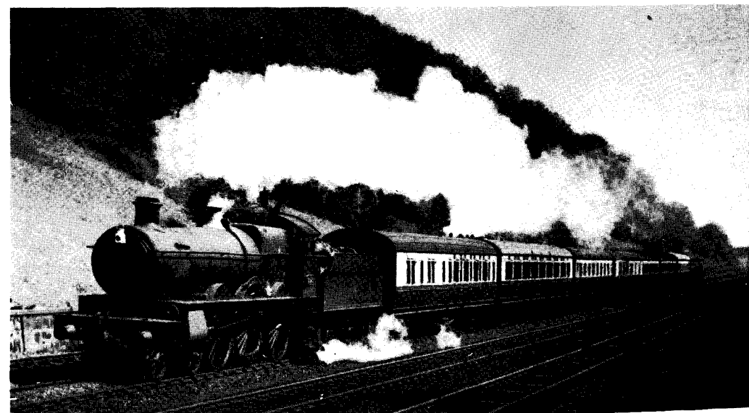
Albion at work, about 1930, with standard boiler and top feed. [M. W. Earley.
