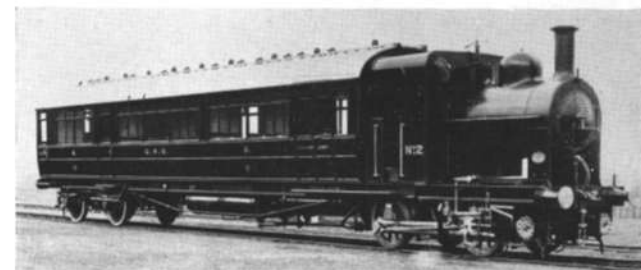
Ivatt's 0-8-2 condensing suburban tank, No. 116, as first built in 1903 with long tanks, which probably prompted this short-lived advertising scheme. The pictorial poster shows No. 990 with a train of 6-wheel-bogie carriages.
