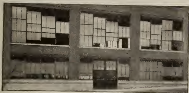
LUPTON COUNTERBALANCED SASH 2-sash and 3-sash high
