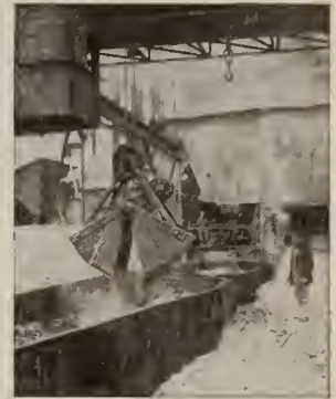
BLAW BULLDOG BUCKET REHANDLING BLAST FURNACE SLAG
