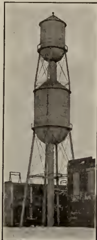
ERECTED AT THREE RIVERS, QUE. Capacity 50,000 gals., height, 149 ft. Capacity 120,000 gals., height, 100 ft.
