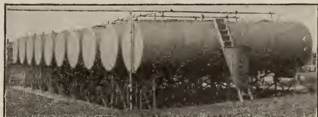
FOUR SINGLE, THREE DOUBLE AND THREE TRIPLE COMPARTMENT CYLINDRICAL, HORIZONTAL OIL STORAGE TANKS ON STRUCTURAL STEEL SUPPORTS
