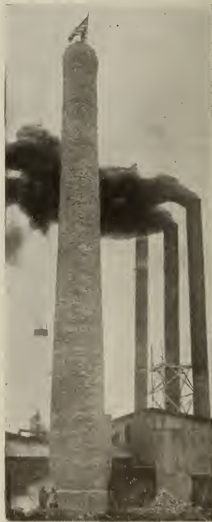
COMMON BRICK CHIMNEY 125 FT. HIGH BUILT BY AMERICAN CHIMNEY CONSTRUCTION CO. FOR THE LOVINGTON COAL MINING CO., LOVINGTON, ILL.
