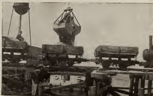
No. A-1675. HAYWARD CLAM SHELL BUCKET WITH ORE BOWL Rehandling contractor's materials. Note the clean, accurate dump
