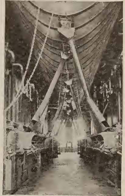
VIEW OF BROWNHOIST COAL BIN SHOWING DISTRIBUTING SPOUTS
