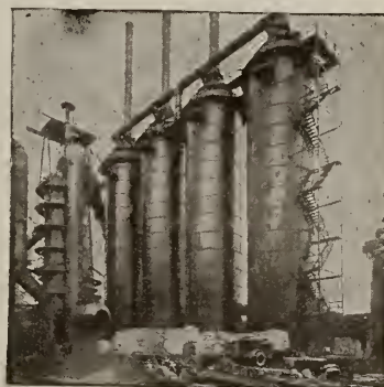
HOT BLAST STOVES INSULATED WITH SIL-O-CEL BRICK
