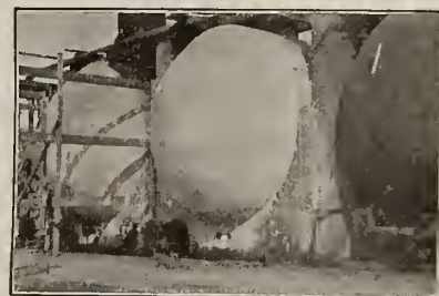
OIL STILLS INSULATED WITH SIL-O-CEL INSULATING BRICK
