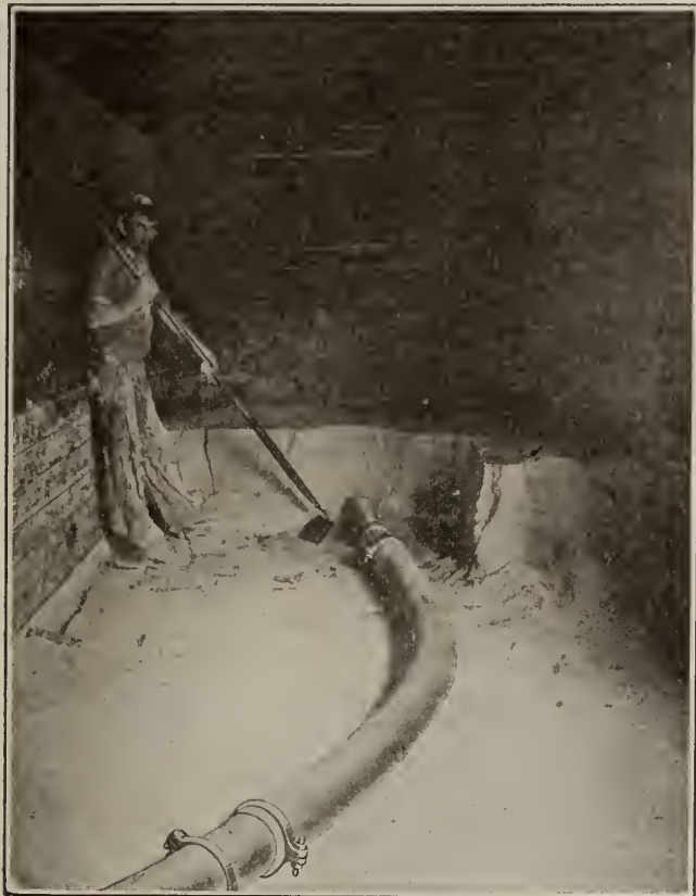
AIRVEYOR USED AS A PNEUMATIC CAR UNLOADER HANDLING SODA ASH
