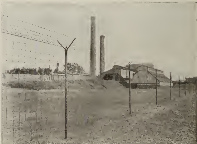
PLATE NO. E3695. SQUARE MESH FENCE, ERECTED FOR MERCK & CO., RAHWAY, N. J. Height.....8 ft. Posts.....Galvanized Anchor posts Fabric.....No. 9 galvanized wire, woven into rectangular mesh Equipped with arms and 7 strands of barbed wire
