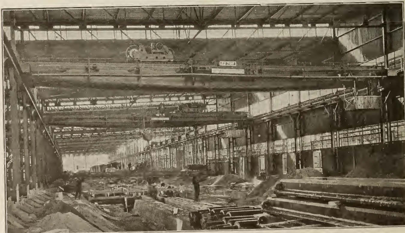
CHESAPEAKE ELECTRIC TRAVELING CRANES IN PLANT OF EASTERN ROLLING MILLS CO., BALTIMORE, MD. Capacity of each, 25 tons, with 10-ton auxiliary hoist
