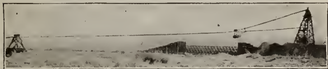
DAM AND RESERVOIR CONSTRUCTION—In dam or reservoir construction a stationary mast or movable tower can be used, depending on local conditions. The mast or tower is located behind the proposed dam. The dam is built up by depositing the material excavated from the proposed basin.
