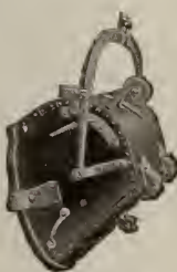
Side- and Back-lever Catch for Coal Hoisting
