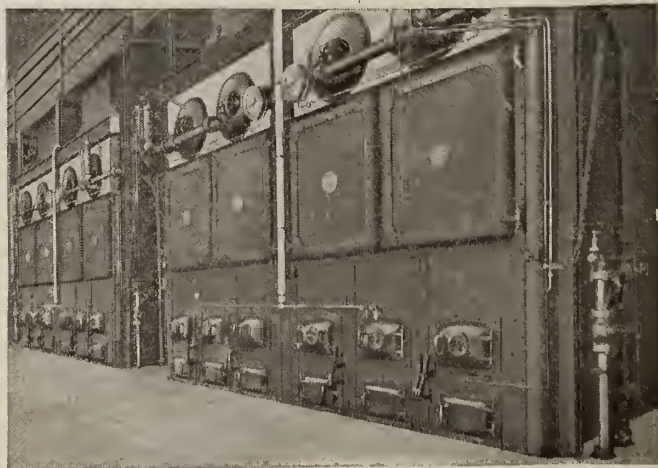
TWELVE 410 H. P. KEELER WATER TUBE BOILERS, ISTHMIUS OF PANAMA Built for the United States Government
