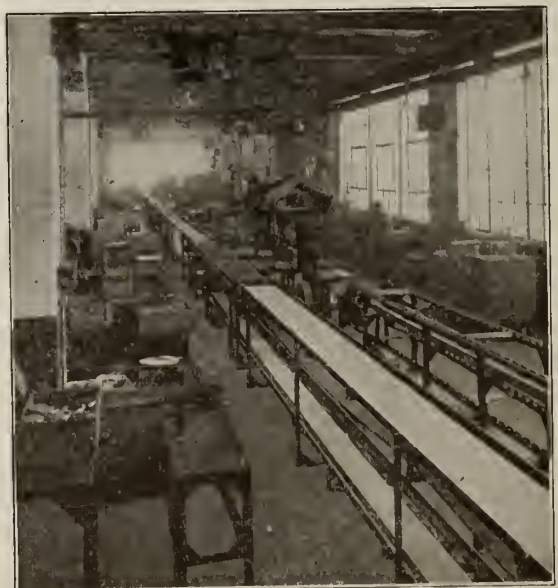
PORTION OF A COMPREHENSIVE CONVEYING AND ELEVATING SYSTEM INSTALLED IN PLANT OF AMERICAN CAN CO., MAYWOOD, ILL.
