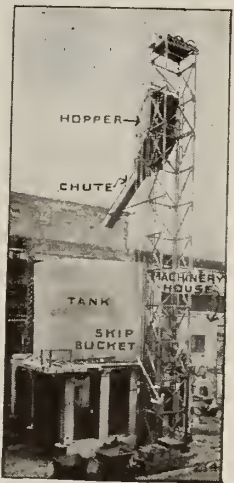
SKIP HOIST INSTALLATION
