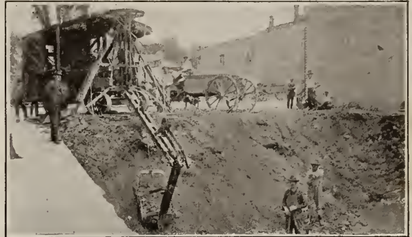
DRAG-DITCHER SCOOP, USED IN DITCHING, BACKFILLING AND CELLAR DIGGING, (MODEL 3)
