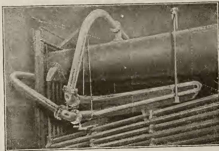
FIG. 1. TYPICAL INSTALLATION OF FOSTER SUPERHEATER IN BABCOCK & WILCOX WATER TUBE BOILER
