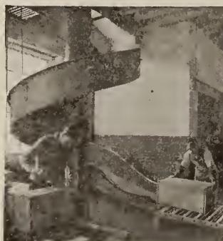
Lamson spiral chutes carry a steady stream of packages vertically downward, quickly and without attention and without damage
