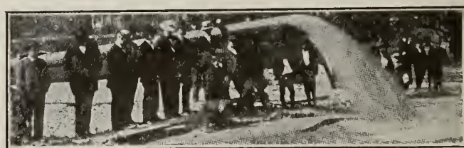
FIG. 4. ASPHALTED PRESSURE PIPE DISCHARGING SAND AND GRAVEL 1¼ MILES FROM SUPPLY Raising the level of the ground. Using 6,600 ft. of 12-in. No. 12 pipe
