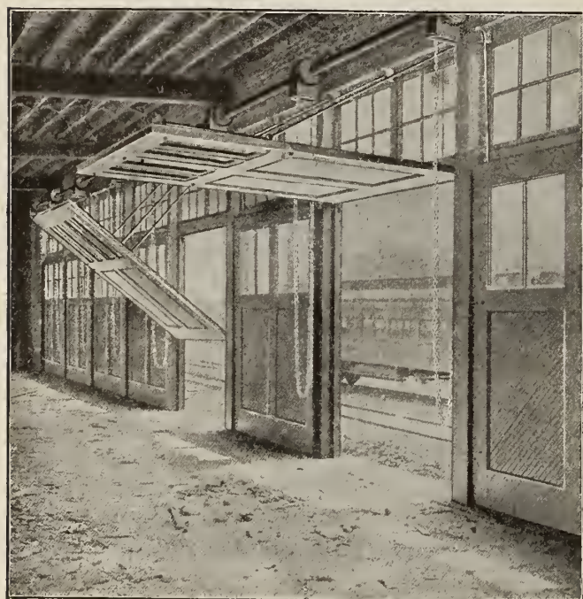
SLIDING SWING DOORS IN FREIGHT SHED OF CHICAGO & NORTHWESTERN R. R. CO., MADISON, WIS.
