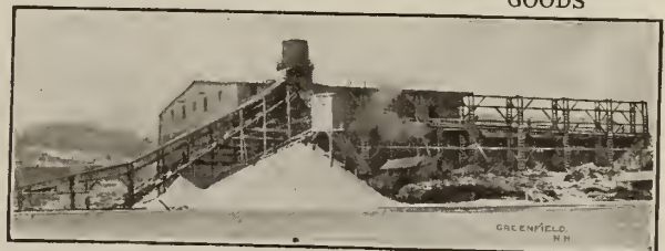
CONVEYOR AND ROPE DRIVE CHIP CONVEYOR The run on the gallery is wide and is provided with two single chains with flights side by side
