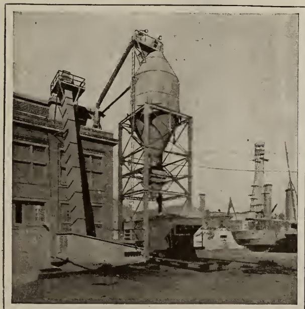
PNEUMATIC CONVEYOR FOR HANDLING ASHES FROM BOILER HOUSE TO STORAGE TANK OUTSIDE
