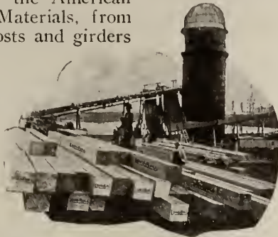
LONG-BELL TIMBERS MADE OF LONG-LEAF SOUTHERN PINE Can be supplied in lengths up to 60 ft., either creosoted or untreated
