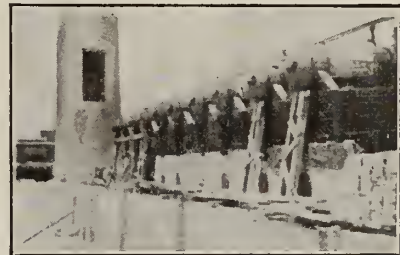
Boiler Settings for 10 Water Tube Boilers, Charleston, S. C.
