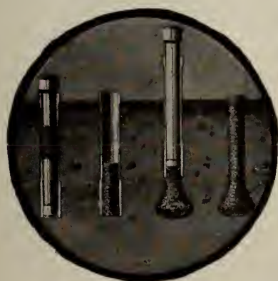
METHOD OF INSTALLING MACARTHUR PEDESTAL PILES
