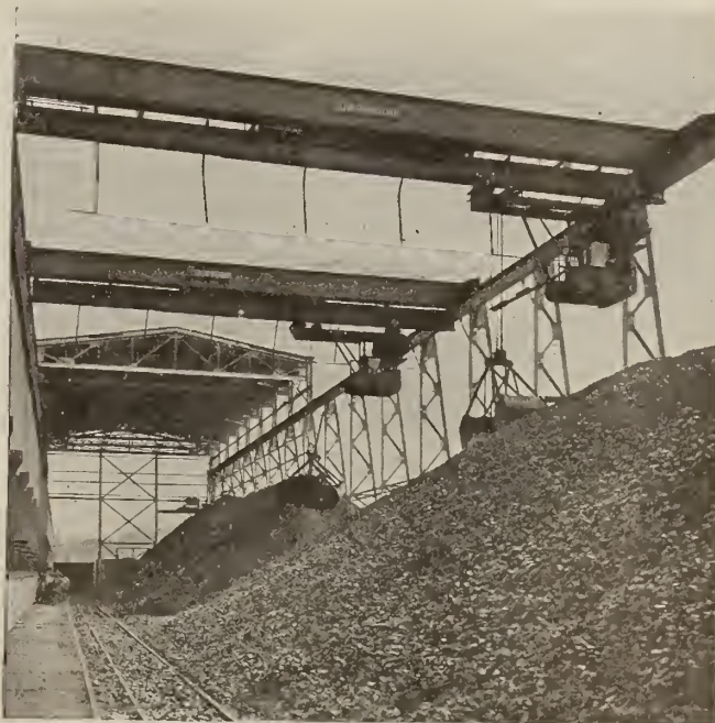
TWO FORM 19-13 MONORAIL HOISTS OPERATING ON TRANSFER CRANES
