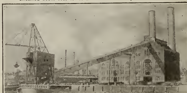
PUBLIC SERVICE CORPORATION, PERTH AMBOY, N. J. Electric hoisting tower with inclined belt conveyor to bunkers. Capacity on acceptance test, 240 tons per hour
