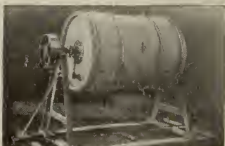
SPECIAL MIXING TANK WITH STEEL SPIRAL STIRRERS
