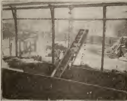
TYPE B CONVEYOR SUSPENDED FROM TROLLEY
