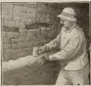
SHOWING HOW EASILY PLIBRICO CAN BE PUT IN
