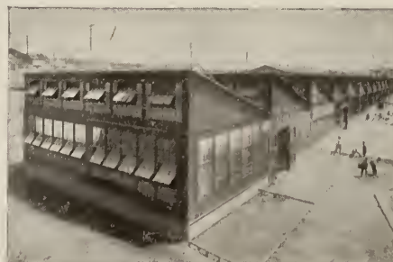
50 x 500-FT. SAWTOOTH TYPE TRUSCON STANDARD BUILDING
