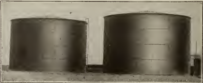
MOLASSES TANKS, GREAT WESTERN SUGAR CO., GERING, NEBR. Diameter, 35 ft.; height, 23 ft.
