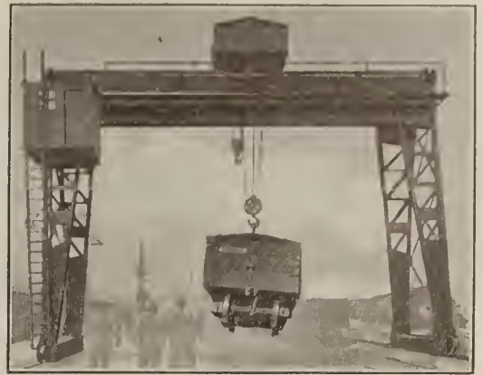
30-TON, 4-MOTOR GANTRY CRANE, PENNSYLVANIA R. R. LINES, CLEVELAND, OHIO 42-foot span
