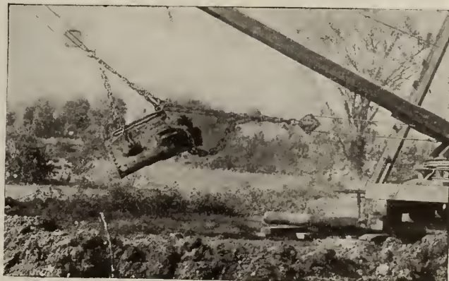
No. A-1839. HAYWARD DRAG SCRAPER BUCKET Digging in hard-pan. Note the full load cleanly carried
