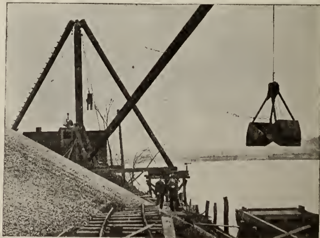
BLAW SPEEDSTER BUCKET REHANDLING SAND AND GRAVEL FROM BARGE
