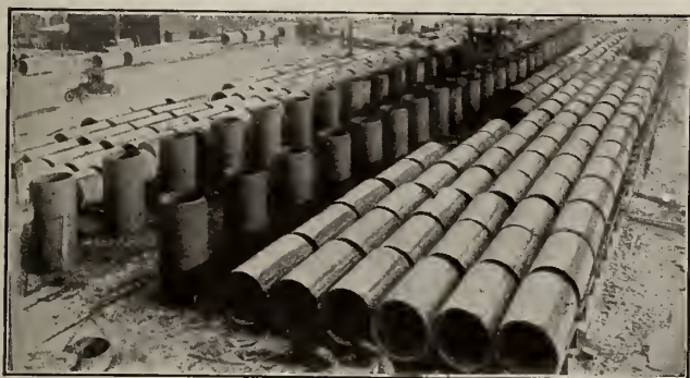
A LOCK-JOINT PLANT MAKING 42-INCH PRESSURE PIPE
