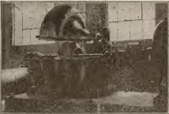
18-INCH TYPE "S" PUMP IN IRRIGATION PUMPING STATION Cover raised showing split casing feature
