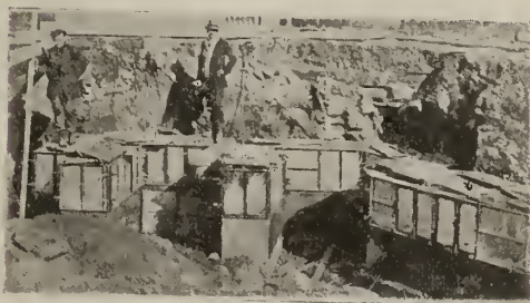
METAFORMS ON BASEMENT FOUNDATION
