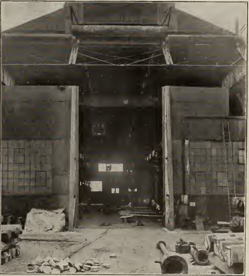
MOTOR DRIVEN DOORS, 60 x 40 FT., WITH AUTOMATIC STOPS Designed and erected by CORNELL IRON WORKS
