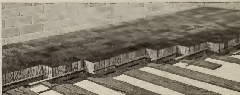
FIG. 3. BLOXONEND ON FLAT STRIPS OVER NEAT CONCRETE
