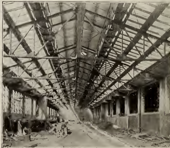
"FEDERAL" ALL-GLASS SLAB ROOF Great Western Smelting and Refining Co., Chicago, Ill.
