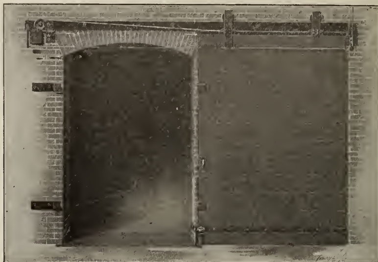
"AJAX" SLIDING DOOR EQUIPPED WITH AUTOMATIC CLOSING DEVICE
