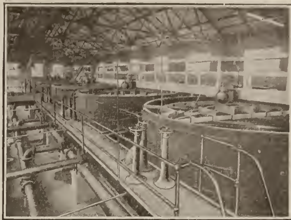
A 3,000,000-GALLON "PERMUTIT" FILTRATION PLANT
