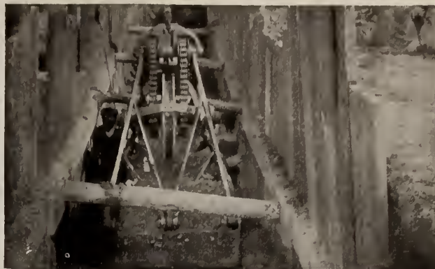
No. A-1645. HAYWARD CLASS "H" MULTI-POWER CLAM SHELL BUCKET (1½ CU. YDS.) Working between sheeting 10 ft. apart and digging in sand, loam and gravel
