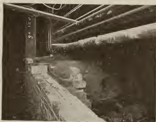
INSULATING A BOILER SETTING WITH NONPAREIL INSULATING BRICK
