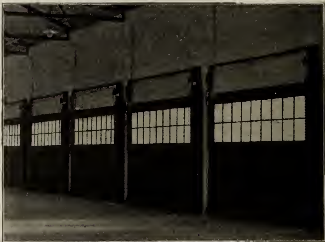
NORFOLK & WESTERN FREIGHT HOUSE, NORFOLK, VA. Installation of Kinnear bifolding door, type No. 1
