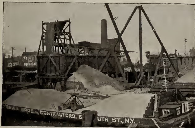
No. C-355. HAYWARD CLAM SHELL BUCKET Unloading crushed stone from barges
