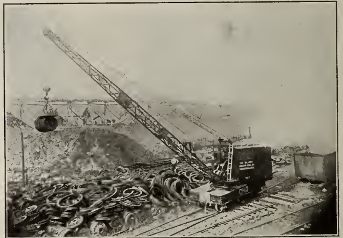
20-TON CAPACITY, 8-WHEEL CRANE, WILKOFF IRON & STEEL CO., YOUNGSTOWN, OHIO Used for handling heavy material about their scrap yards. Equipped with magnet and generator
