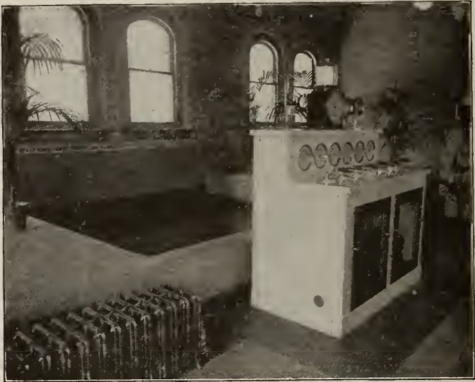
OPERATING TABLE CONTROLLING CONCRETE GRAVITY FILTER
