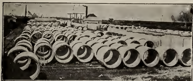
66-INCH PRESSURE PIPE MADE AT WINNIPEG PLANT FOR GREATER WINNIPEG WATER DISTRICT
