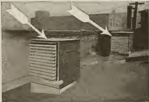
TWO 36-IN. ILG POWER ROOF VENTILATORS INSTALLED ON ROOF AND DIRECTLY CONNECTED TO HOODS OVER FURNACES, IN PLANT OF AMALGAMATED METALS CO., CHICAGO, ILL.
