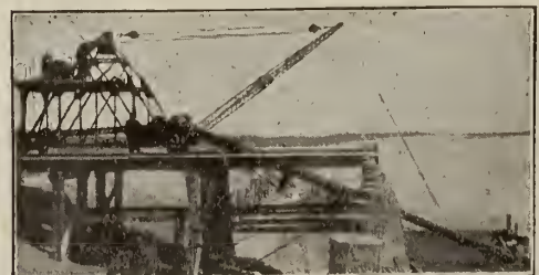
LARGE SELF-PROPELLED BOAT UNLOADER FOR HANDLING GENERAL CARGO BETWEEN BOATS AND CARS
