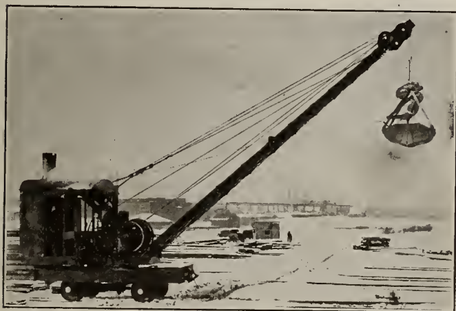
10-TON 4-WHEEL STANDARD BUFFALO LOCOMOTIVE CRANE AND 1-CU. YD. BUFFALO STANDARD CLAMSHELL BUCKET IN USE BY A LARGE BUFFALO STEEL COMPANY
