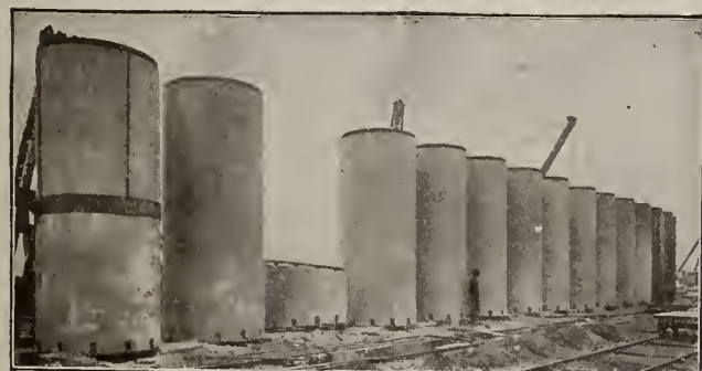
72-INCH SUBAQUEOUS PIPE LAID IN LAKE ERIE
