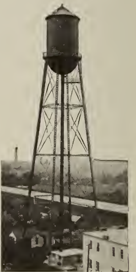
TANK AND TOWER. STUDEBAKER BROS. MFG. CO., SOUTH BEND, IND. 150,000 gals., 206 ft. high
