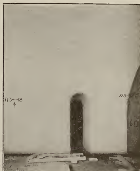
Before being Waterproofed SAME POINT IN PENNSYLVANIA TUNNELS BEFORE AND AFTER BEING WATERPROOFED WITH "COW BAY" WATERPROOF CEMENT
