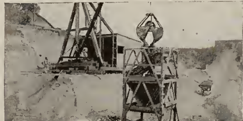
HAISS "CONTRACTOR" BUCKET DIGGING IN A SAND PIT
