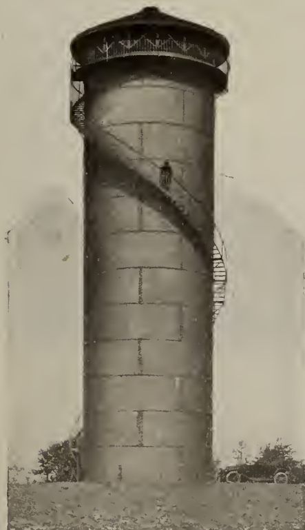
STANDPIPE FOR CONNECTICUT AGRICULTURAL COLLEGE Diameter, 25 ft.; height, 80 ft.
