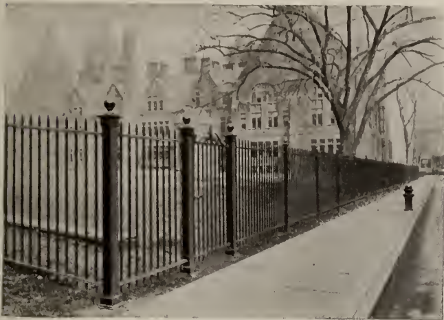
PLATE NO. E4617. ELECTRICALLY WELDED IRON RAILING, ERECTED FOR THE HARTFORD HIGH SCHOOL, HARTFORD, CONN.
