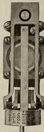
POSITIVE THERMOSTAT Showing inside mechanism
