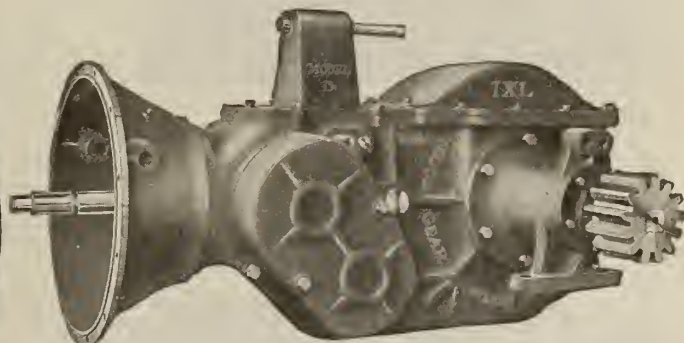
MODEL D FOOTE-IXL TRACTOR TRANSMISSION
