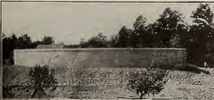
REINFORCED CONCRETE RESERVOIR, BADEN, N. C. Capacity, 1,000,000 gals.
