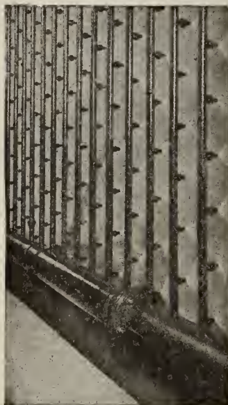
SPRAY CHAMBER VIEW OF WEBSTER APPARATUS
