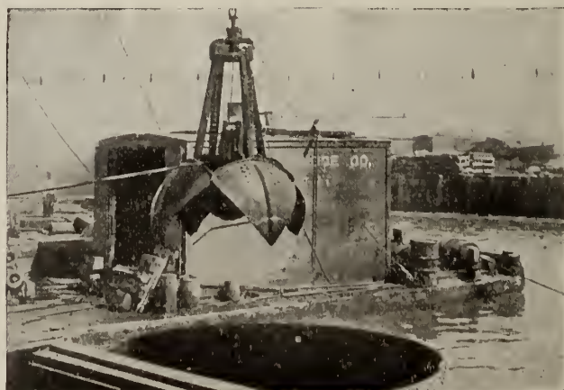
No. A-2648. HAYWARD ORANGE PEEL BUCKET Excavating material from within a caisson as it is being sunk
