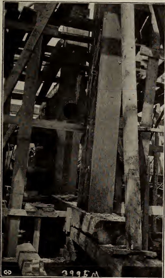
OAK STERN POST AND RUDDER POST OF WOODEN SHIP Photo by U. S. Forest Products Laboratory
