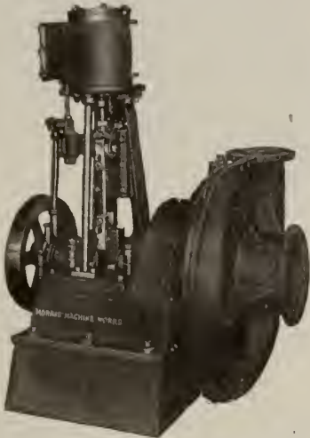
STANDARD SIDE SUCTION STEAM PUMP
