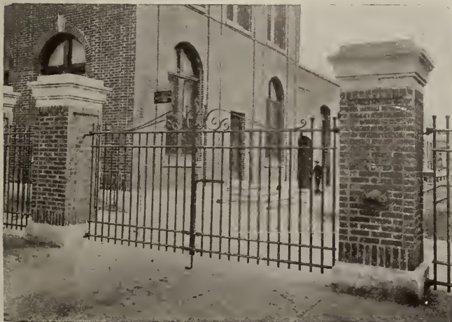
PLATE NO. E4606. ELECTRICALLY WELDED DOUBLE GATES AT THE FACTORY OF THE DURATEX COMPANY, NEWARK, N. J.
