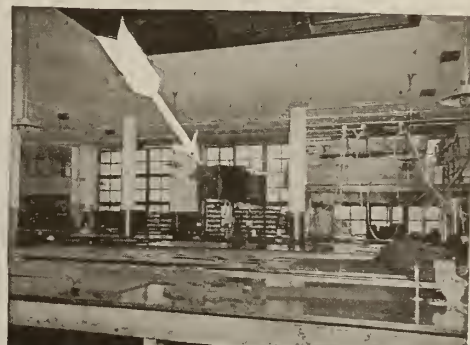
CEILING TYPE 24-IN. ILGAIR UNIT HEATER BLOWING IN TEMPERED OUTSIDE AIR FOR VENTILATION, "HOUSE OF KUPPENHEIMER," CHICAGO
