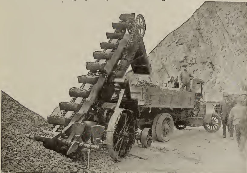
"PATH DIGGING" WAGON LOADER LOADING 5 CU. YDS. OF 2-IN. CRUSHED STONE IN 5 MINUTES
