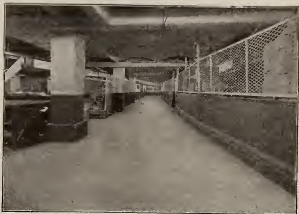
HEAVY DUTY TROEGERLITH COMPOSITION FLOORING INSTALLED IN WAREHOUSE OVER ROUGH CONCRETE UNDERFLOORS
