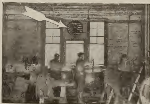
EXHAUSTING STEAM AND ACID VAPOR IN STAR CLEANING CO., CHICAGO, USING 24-IN. SELF-COOLED MOTOR PROPELLER FAN EQUIPPED WITH AUTOMATIC SHUTTER
