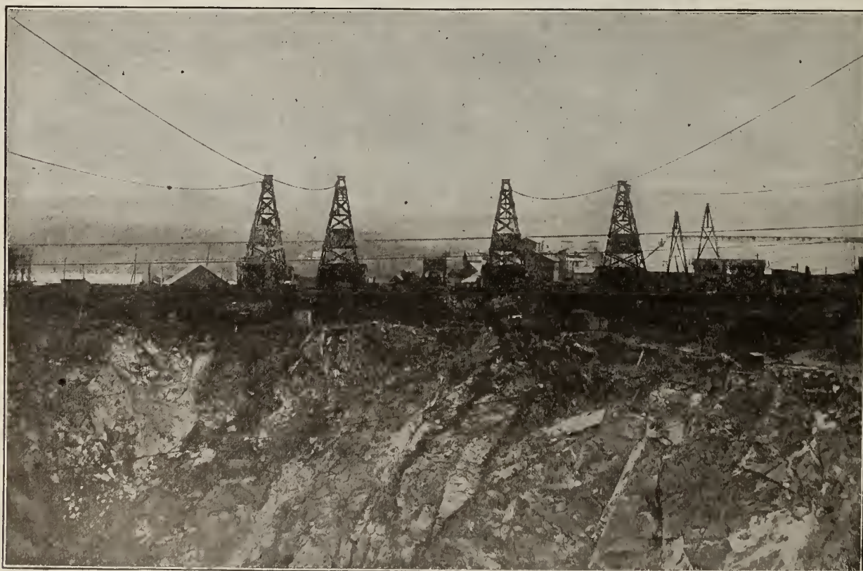
FLORY CABLEWAYS INSTALLED BY THE ASBESTOS CORPORATION OF CANADA
