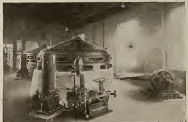
300-KV-A WATER WHEEL GENERATOR VIRGINIA COTTON MILLS
