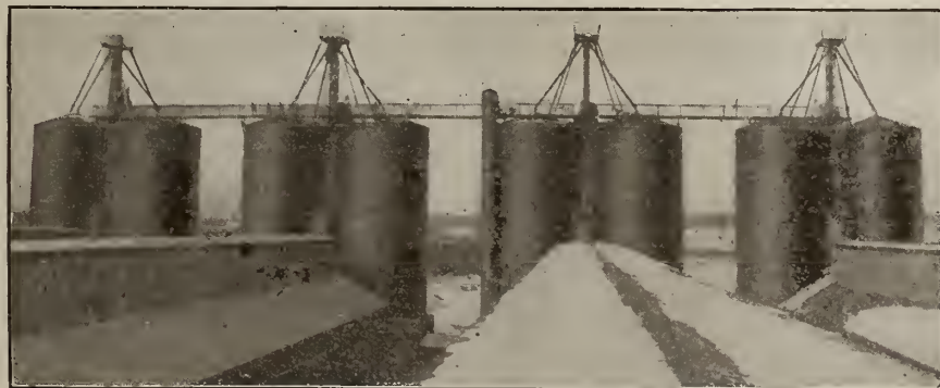
EIGHT ALUMINUM ORE BINS, 34 FT. DIAMETER BY 70 FT. HIGH Aluminum Company of America, Massena, N. Y.
