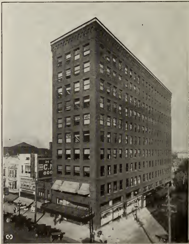
THE RENKERT BUILDING, CANTON, OHIO, FACED WITH VITRIFIED PAVING BRICK
