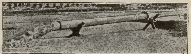
SECOND-HAND PIPE USED FOR DISCHARGE LINE
