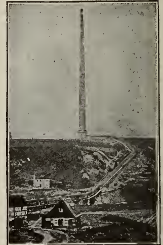
HEINICKE CHIMNEY SERVING A SMELTER Height, 460 ft.; clear diameter at top, 8 ft. Built 1889
