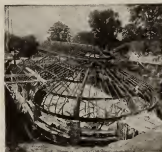
STEEL FRAME READY FOR PYROBAR
