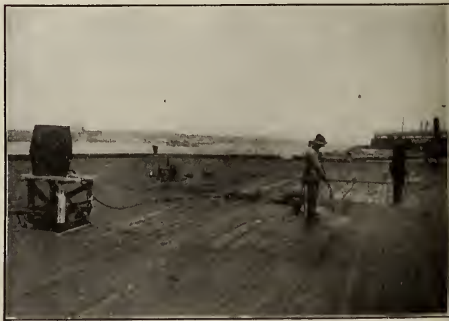
APPLYING LETTENY WITH SPRAYING MACHINE TO UNDER-PLANKING OF NEW YORK CITY PIER
