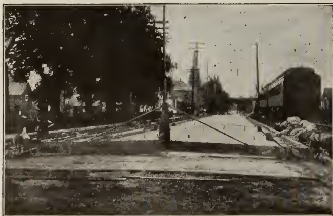
REINFORCED CONCRETE PAVEMENT, CONNERSVILLE, IND. W. F. RIDPATH, City Engineer GREENWOOD, CONNOR, BOOTS & GANT, Contractors 585 sq. ft. Triangle Mesh Reinforcement used
