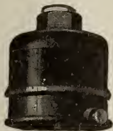
HOLDER-SOCKET WITH PORCELAIN BUSHING FOR REINFORCED DROP CORD SUSPENSION
