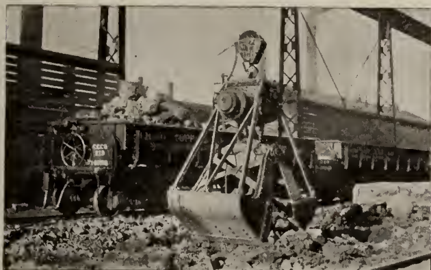
No. C-495. HAYWARD ELECTRIC MOTOR BUCKET (3 CU. YDS.) Loading broken open hearth slag into cars
