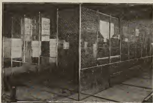
PAGE STANDARD WIRE LINK INSIDE PANEL PARTITION Note self-supporting construction. No light is lost here
