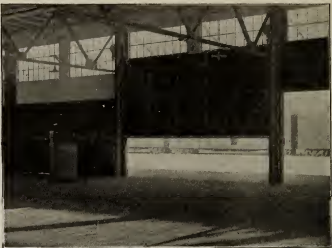
SANTA FE FREIGHT SHED, LOS ANGELES, CAL. Equipped with Kinnear vertical sliding doors. Interior view showing three positions of the door
