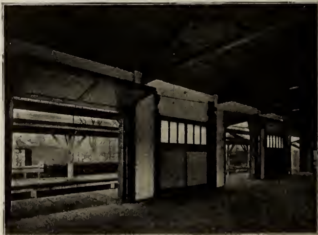
PENNSYLVANIA FREIGHT HOUSE, CAMBRIDGE, OHIO Installation of Kinnear bifolding door, type No. 1
