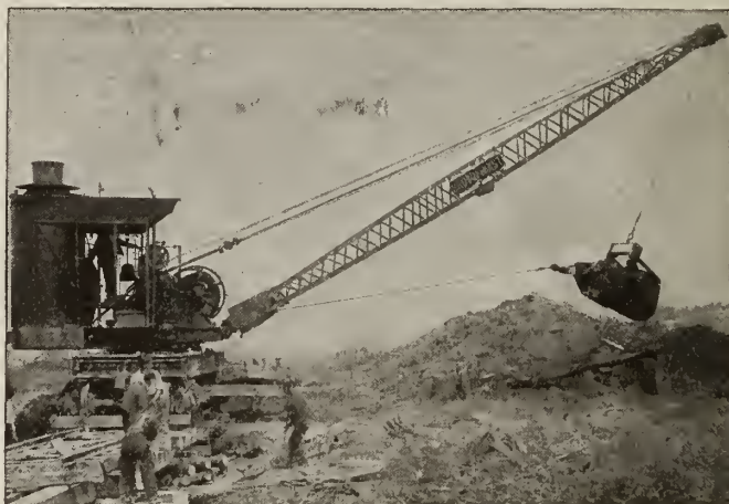
No. 4 CRANE EQUIPPED WITH DRAGLINE BUCKET
