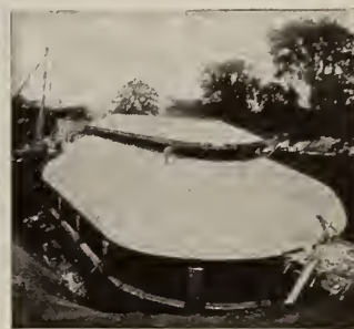
PYROBAR APPLIED TO STEEL
