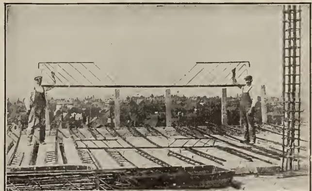
RIVET GRIP FABRICATED UNIT BEAM FRAMES Note simplicity in handling
