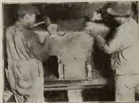
PLIBRICO CAN BE MOULDED TO FIT ANY PLACE IN FURNACE OR SETTING
