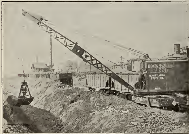
25-TON CAPACITY, 8-WHEEL CRANE, PENNSYLVANIA STEEL CO., STEELTON, PA. Equipped with orange peel bucket
