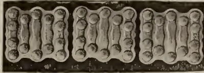
OUTSIDE OF CRESCENT JOINT SHOWING CRESCENT PLATES AND CRESCENT RIVETS
