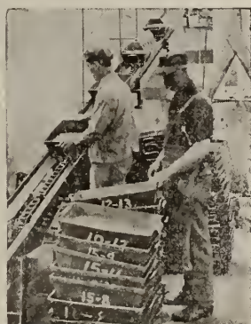
Tote boxes of small parts carried by gravity or by this chain conveyor
