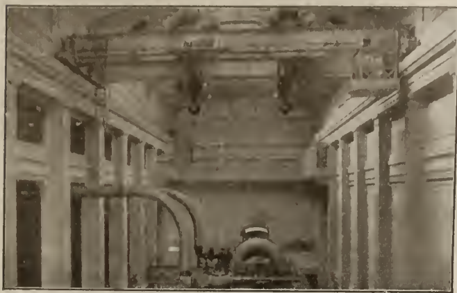
160-TON TRAVELING CRANE IN POWER PLANT OF PHILADELPHIA ELECTRIC CO.
