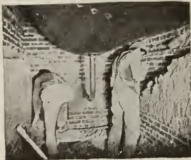
APPLYING BETSON'S PLASTIC FIRE BRICK FURNACE LINING
