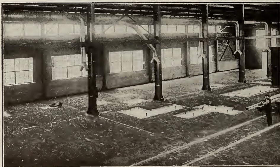
SHOWING METHOD OF LAYING FLOOR ALONG TRACKS AND AROUND MACHINERY FOUNDATIONS
