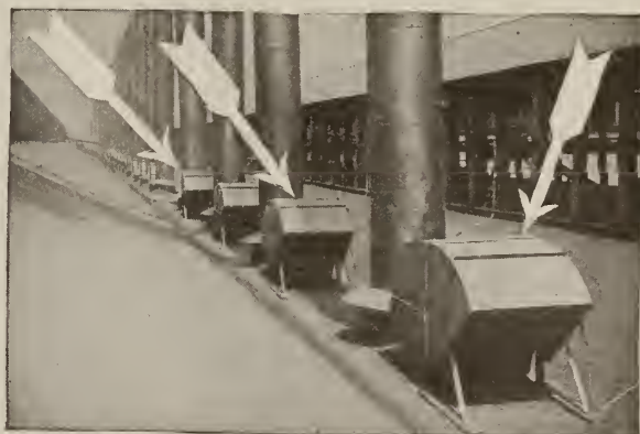
FORTY-FOUR 42-IN. ILG SELF-COOLED MOTOR PROPELLER FANS COOLING MEN WORKING AT FURNACES, McKEESPORT (PA.) TIN PLATE CO.
