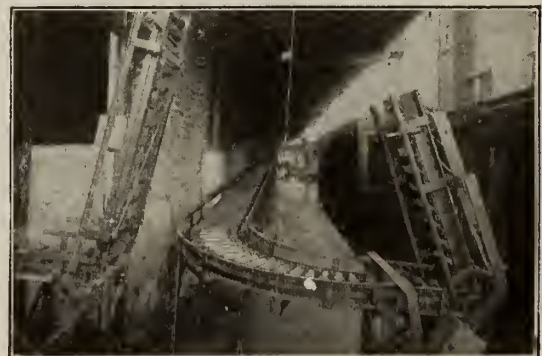
DOW GRAVITY CONVEYOR ON SHIPPING PLATFORM Note hinged sections
