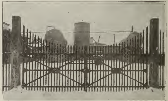
ANGLE IRON PICKET FENCE SHOWING CONCRETE POSTS IN USE
