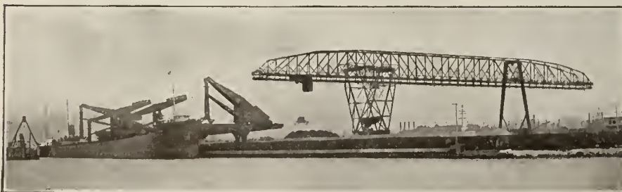
ORE BRIDGE PENNSYLVANIA R. R. DOCKS, CLEVELAND, OHIO Serves dock space 612 ft. deep and carries a 15-ton bucket. Transfers ore, weighing while handling. Capacity, 800 tons per hour
