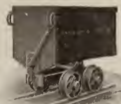
FIG. 403. MINE CAR FOR HEAVY WORK This type is built in capacities ranging from 12 to 27 cu. ft.
