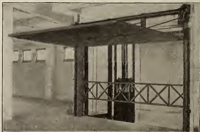
SWING SLIDING DOORS, DUQUESNE FREIGHT SHEDS, PENNSYLVANIA RAILROAD, PITTSBURGH, PA.
