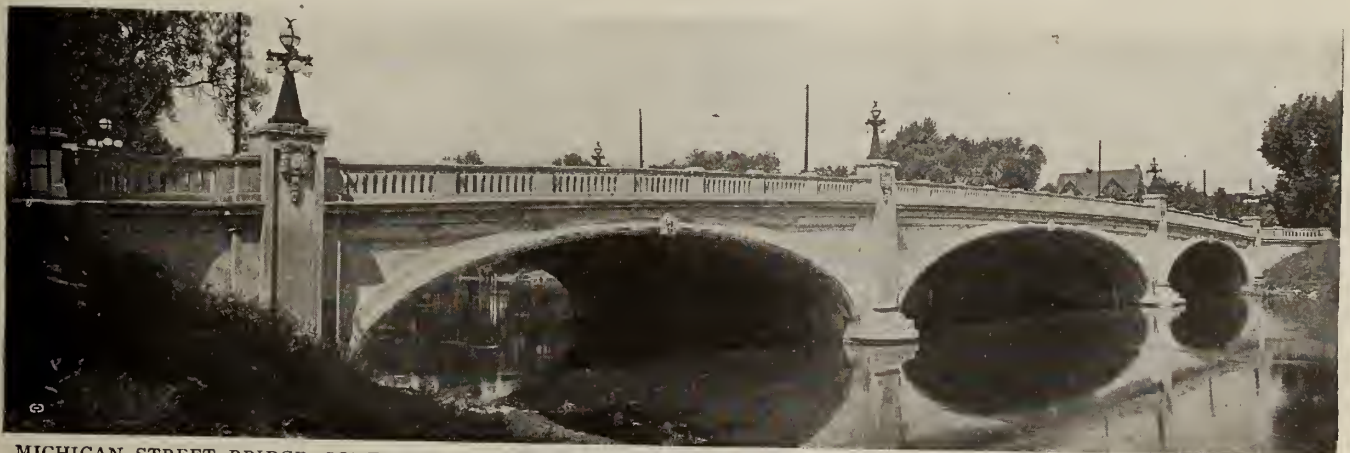
MICHIGAN STREET BRIDGE, SOUTH BEND, IND., BUILT OF REINFORCED CONCRETE FACED WITH INDIANA LIMESTONE CHARLES W. COLE, Architect and Engineer, South Bend, Ind.
