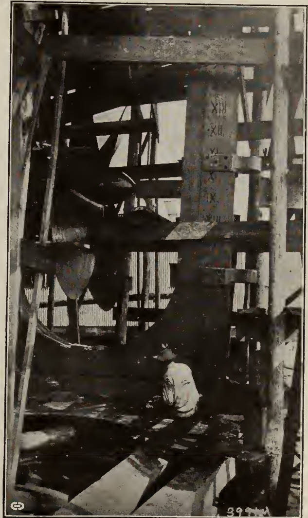
PROPELLER AND OAK STERN POST OF WOODEN SHIP The propeller shaft runs through oak shaft logs and the stern post shown in illustration to left
