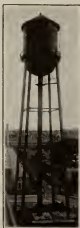
ELEVATED STEEL TANK, EAST YORK, PA., AMERICAN CHAIN CO. Capacity, 100,000 gals., height, 100 ft.
