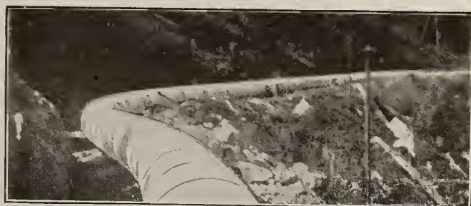
VIEWS OF 42-INCH "LOCK-JOINT" PIPE FOR SOOKE LAKE WATER SUPPLY, VICTORIA, B. C.
