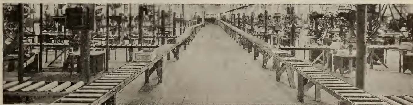
A completely equipped shop. Parts and products from every machine are carried on Lamson conveyors to the two main line conveyors, which in turn carry them to the packing and shipping departments
