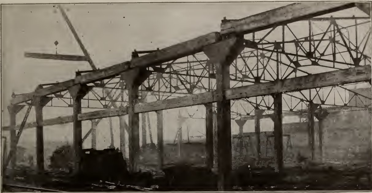
REINFORCED CONCRETE PIECE CONSTRUCTED COLUMNS AND GIRDERS Being erected in place by Union Stock Yard & Transit Co., Chicago. Triangle Mesh Reinforcement used
