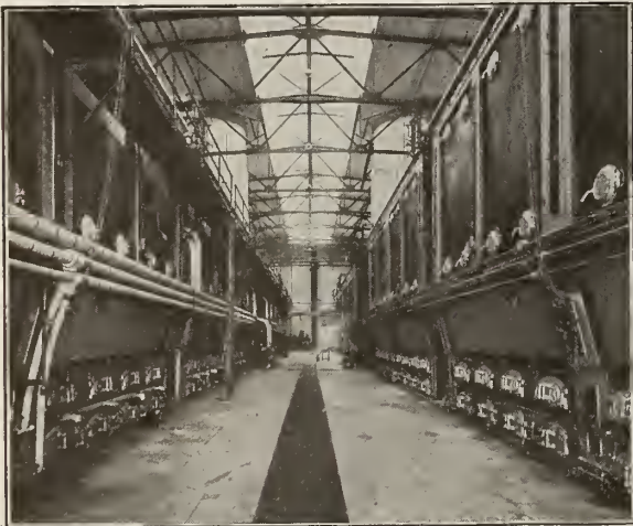
BOILER PLANT OF A LARGE PUBLIC SERVICE CORPORATION, EQUIPPED WITH HAMMEL BURNERS AND FURNACES
