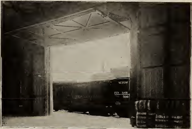
INTERIOR VIEWS SHOWING KINNEAR BIFOLDING DOORS, TYPE NO. 2, IN CLOSED AND OPEN POSITIONS
