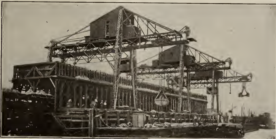
THREE SAND UNLOADER CRANES, INSTALLED FOR THE U. S. GOVERNMENT FOR USE ON THE PANAMA CANAL Equipped with 4-yard buckets.
