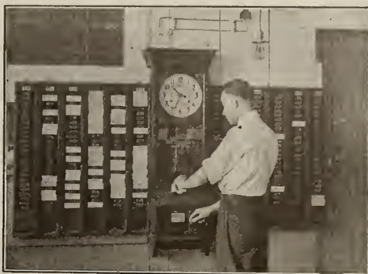
ANY MAKE OF TIME RECORDER CAN BE SYNCHRONIZED OR ELECTRICALLY DRIVEN BY THE "STANDARD" SYSTEM
