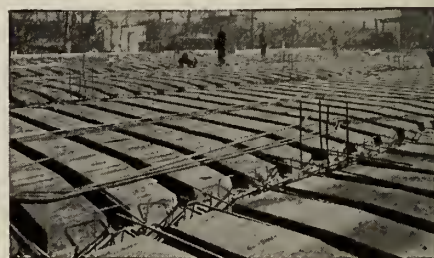
MEYER STEELFORMS WITH REINFORCEMENT IN PLACE READY FOR CONCRETING
