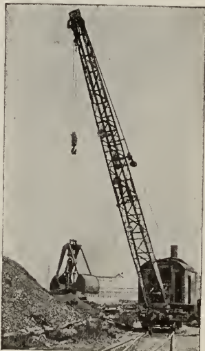
BLAW SINGLE LINE BUCKET, HOOK-ON TYPE
