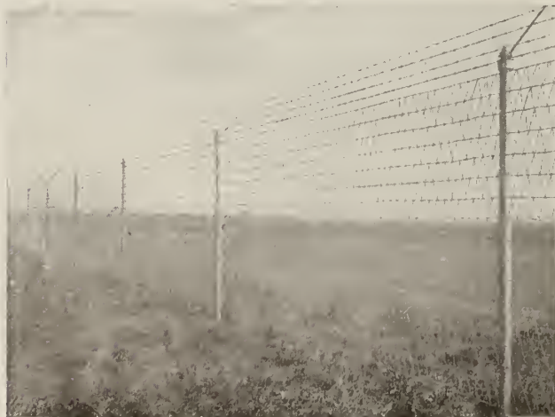
PLATE NO. E3533. TRIANGULAR MESH FENCE, ERECTED FOR THE AMERICAN AIRCRAFT COMPANY AT COPIAGUE, N. Y. Height.....8 ft. Posts.....Galvanized Anchor posts Fabric.....Triangular mesh 2 x 4 in. Equipped with arms and 4 strands barbed wire (Specifications and details on preceding page)
