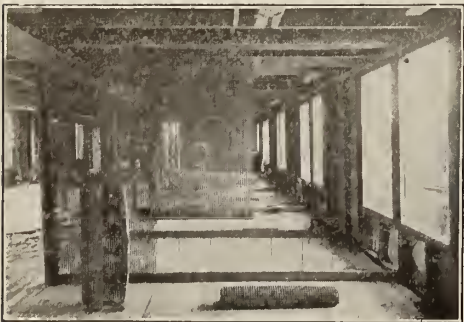
METHOD OF ERECTING WIRE SUPPORTS FOR 2-IN. MONOLITHIC PARTITIONS ON BRIKLATH
