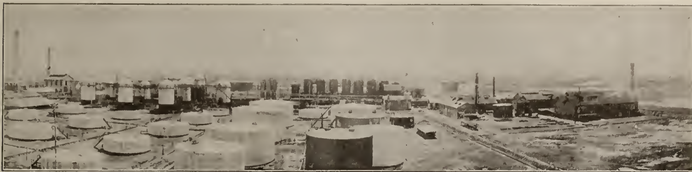
THE TEXAS COMPANY'S REFINERY, PORT ARTHUR, TEX. (Continuous with view on opposite page) barrels up to and including those of 55,000-barrel capacity; 30 filter tanks; 4 dump tanks; 2 receiving tanks; 26 filling tanks; 5 separator tanks; 22 exchanger tanks; 16 steam drums; 11 grease tanks, some steam jacketed; acid tanks, kettles, and many other steel plate products. This refinery is one of the largest in the world
