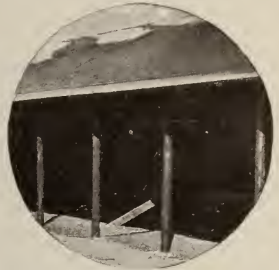
LONG-BELL CREOSOTED BARN POLES AS USED IN GARAGE CONSTRUCTION
