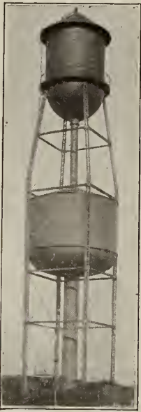
TANK OF PROC-TER & GAMBLE, HAMILTON, ONT. Capacities, 50,000 and 100,000 gals. Heights, 100 and 50 ft. to bottom
