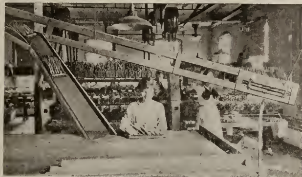
In textile mills, Lamson conveyors carry bobbins, laps, raw cotton, finished cloth, etc. Lower belt of this 2-way conveyor brings empty silk quilts to filling machines. Upper belt returns filled quilts
