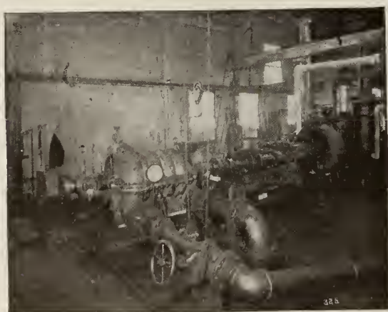
FIG. 325. TESTING A LEA-COURTENAY 8-IN., 5-STAGE, ALL-BRONZE PUMP—ONE OF TWO FURNISHED A LARGE PENNSYLVANIA COAL COMPANY
