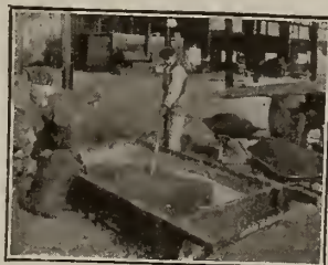
MIXING REFRACTORY MA- TERIALS WITH HYTEM- PITE FOR RAMMED-IN LININGS
