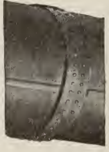
FIG. 6. BUTTSTRAP JOINT
