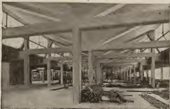
Pond Truss over Domestic Engineering Co. Building, Moraine (near Dayton) Ohio.
