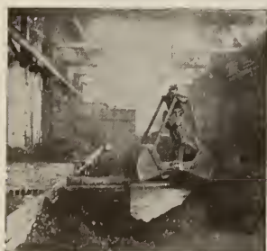
BLAW SINGLE LINE BUCKET HANDLING COAL FROM PILE TO STOKER HOPPERS
