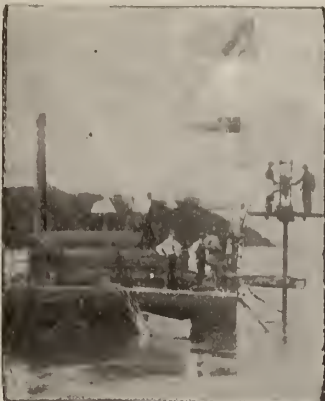
SULLIVAN DIAMOND DRILL TESTING A BRIDGE SITE ON THE ST. LAWRENCE RIVER
