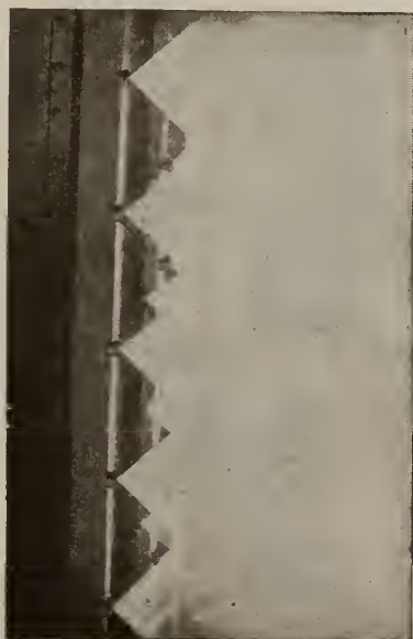
AIR WASHER SPRAY IN OPERATION
