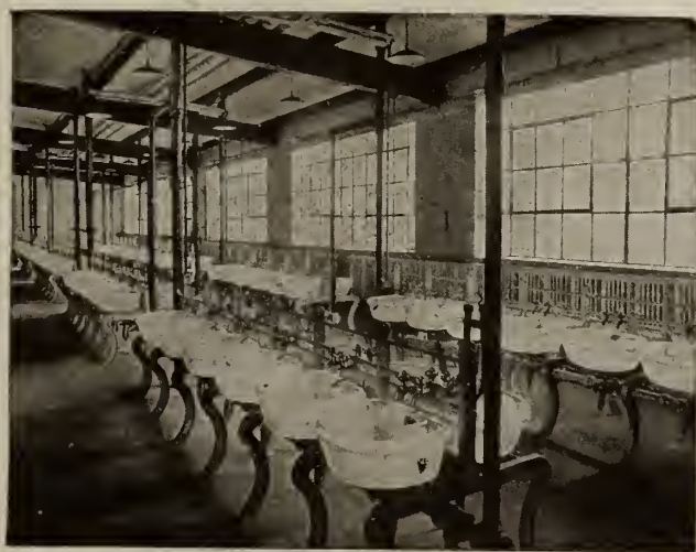
RANGE OF SOLID PORCELAIN "IDEAL" FACTORY LAVATORY BASINS WITH INTEGRAL SOAP HOLDERS
