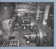
As part of the elaborate installation essential to the operation of 1,438 Hudson  $\psi$  Manhattan trains per day, these three substations convert electric power to the proper voltage.
