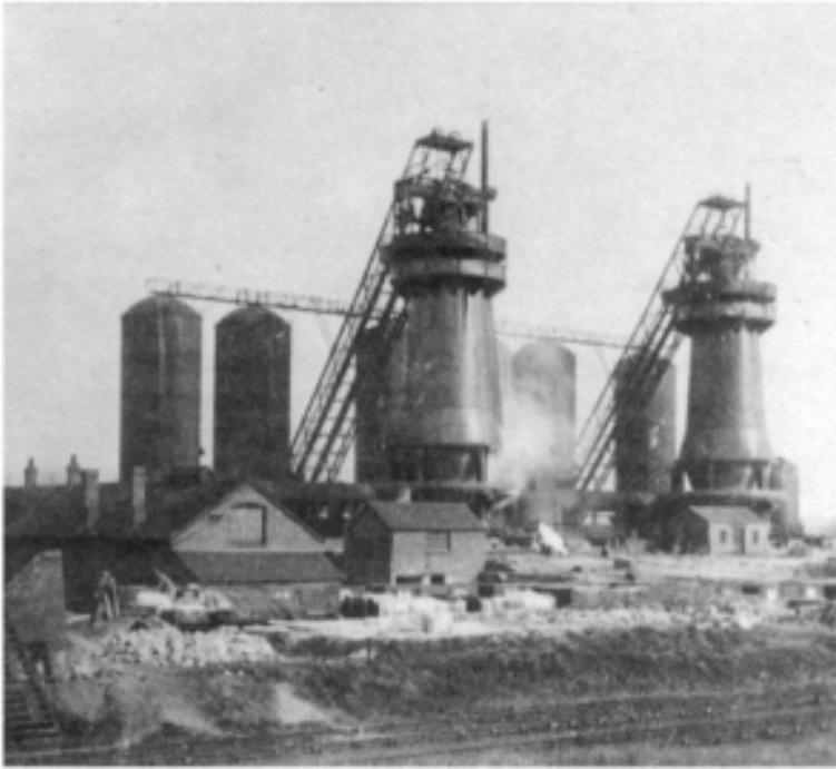
Figure 2.1: From c. 1900 the mechanically-charged blast furnace began to be adopted widely. These two were at Corby, Northamptonshire. The photograph was taken in 1918. Author's collection.
