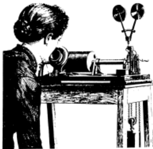
Figure 15.3: Cylinder phonograph for recording and transcribing dictation; the governor regulated the speed of the weight-driven 'motor'.
