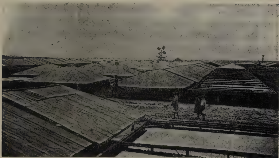
One of the last Cape Cod saltworks still in operation in Yarmouth in the late nineteenth century with vats full of brine and rolling roofs open. An operating windmill is in the background. The Snow Library, Orleans, Massachusetts
