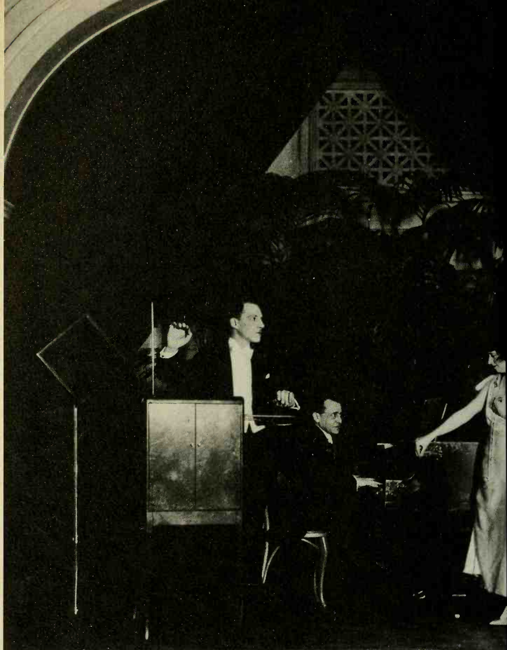
Léon Thérémin (left) giving an early demonstration of the electronic instrument which he developed in 1924. Its sound production was controlled by movements of the hand around the upright pole.
