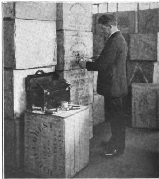
Extracting the sample with wire rake.
