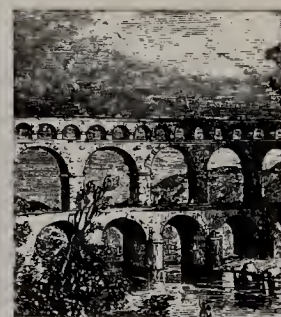
2-8. Roman bridges, part of their road network, were frequently constructed of arches to span rivers.
