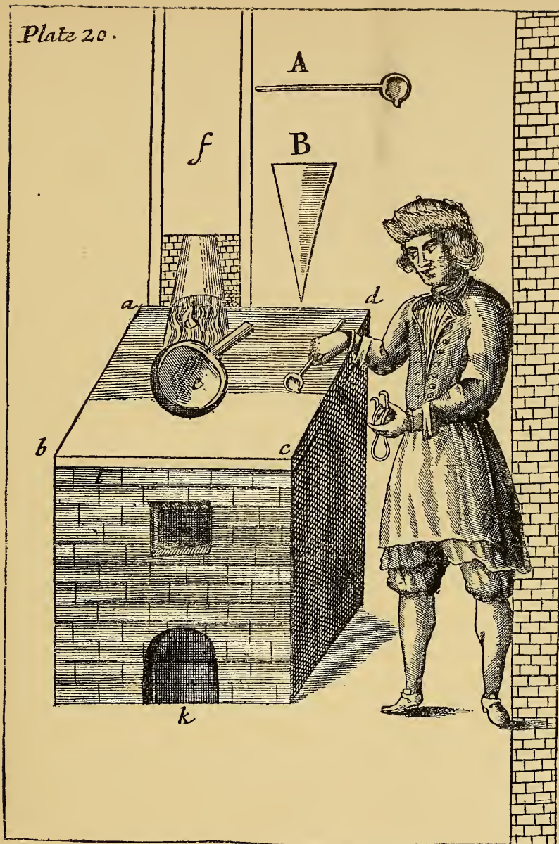
25. Letter-founding in 1683. (From Moxon's Mechanick Exercises .)
