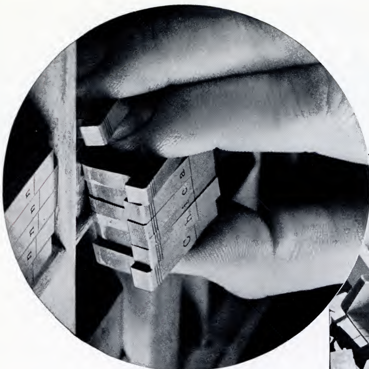
Showing half a dozen Ludlow matrices "gathered" in one operation
