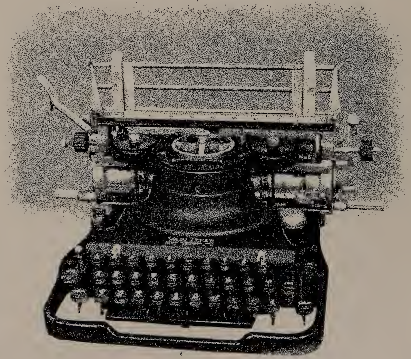
1-1. The original Varityper, c. 1930, was the first typewriterlike composer. The keys are arranged like those of a typewriter but accommodate extra symbols for typesetting with a super shift, an extra shift above the capital letters. Later models provide variable spacing, pressure control for the many different sizes and weights of type fonts, and a rail shift for four different sizes, with adjustable linespacing in point sizes. The Varityper also provides type justification by means of a mechanical counter. These controls provide for type composition.
