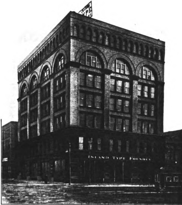
Saint Louis Office and Factory
