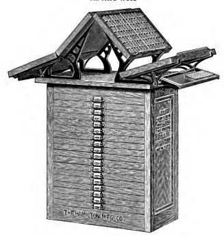
Specially designed for placing in front of a window, as it does not obstruct the light, of which the cases on top get the full benefit. Two men may work undisturbed at the sides, while the job cases in front are convenient for other men. The top is flat, and useful for holding tied-up type.
