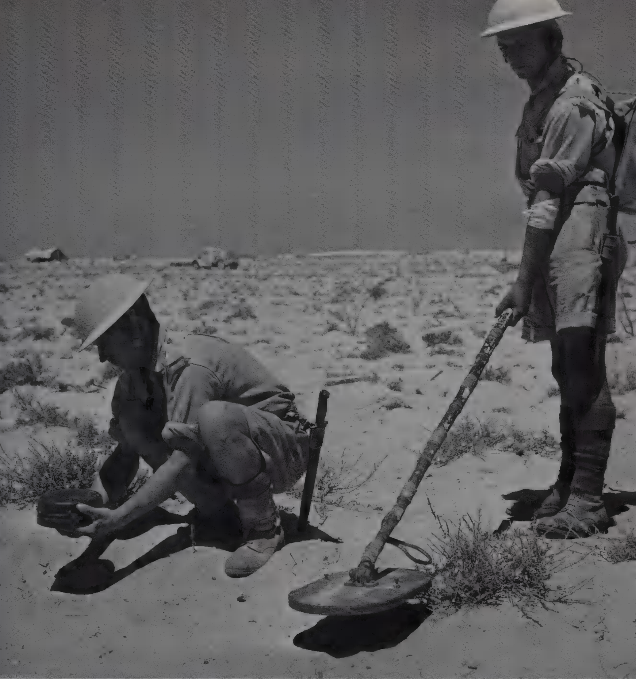
Royal Engineers training with a mine detector. The sapper on the right is alerted to a mine by a sound in his earphones.
