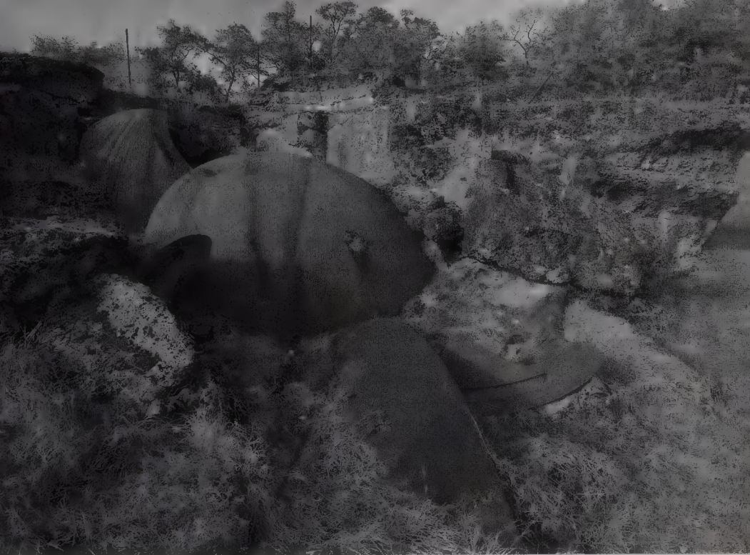
5. Thor's anvil. A cupola at Loncin, one of the forts protecting Liège, smashed by German heavy guns in August 1914.
