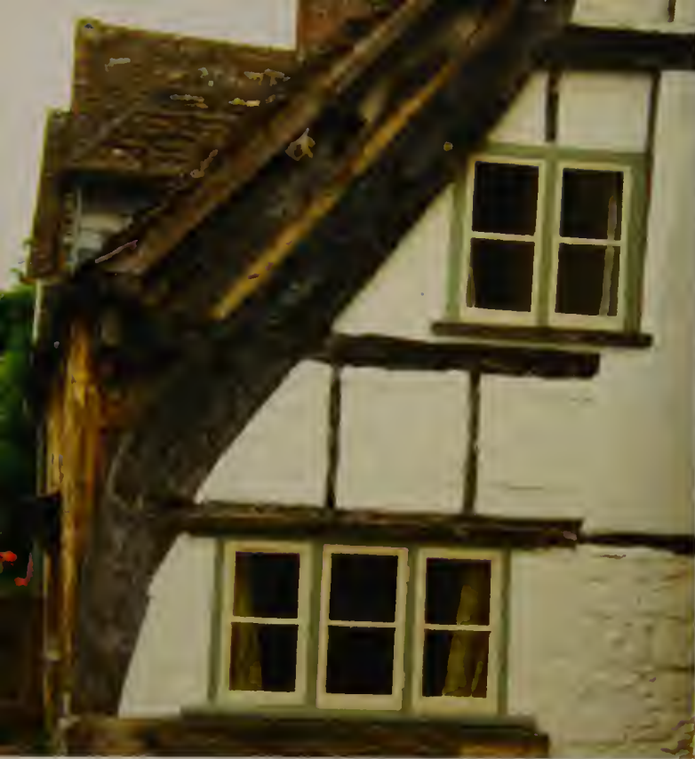
Cruck-beam construction was real leading-edge carpentry technology of the day
