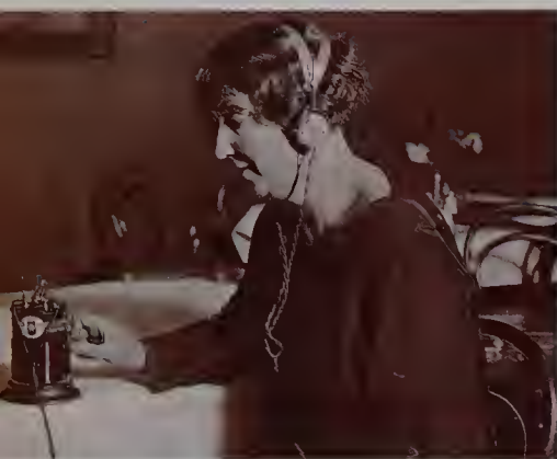
Listening in' on a cat's whisker and crystal set during the Twenties
